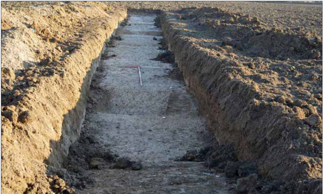
Plate 8: Trench 43, looking south-east
