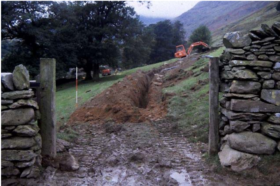
Plate 8: General view of pipeline, looking east along the easement
