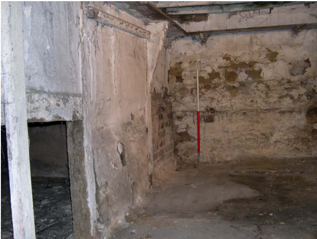
Plate 17: General view of ground floor Room 5
