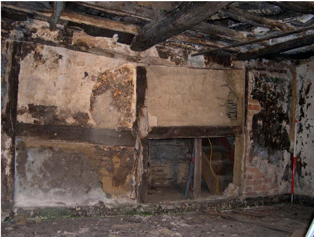
Plate 15: Timber-framed north wall of ground floor Room 3
