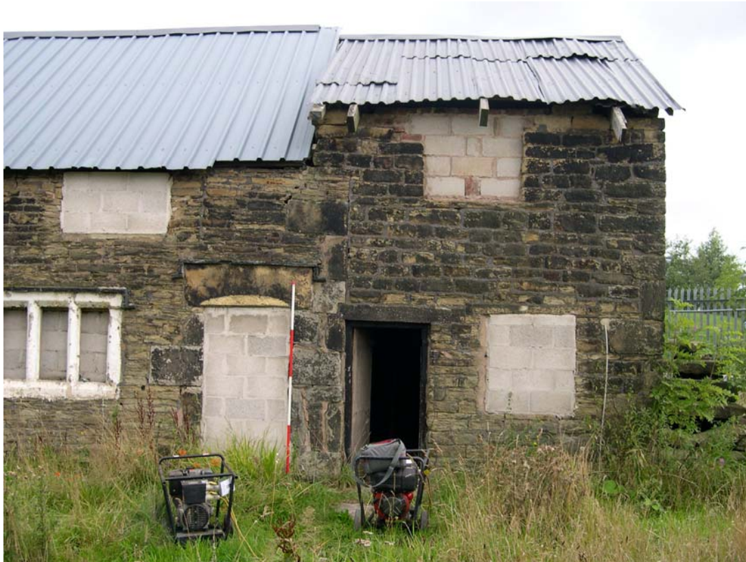
Plate 6: East end of the front (south) elevation
