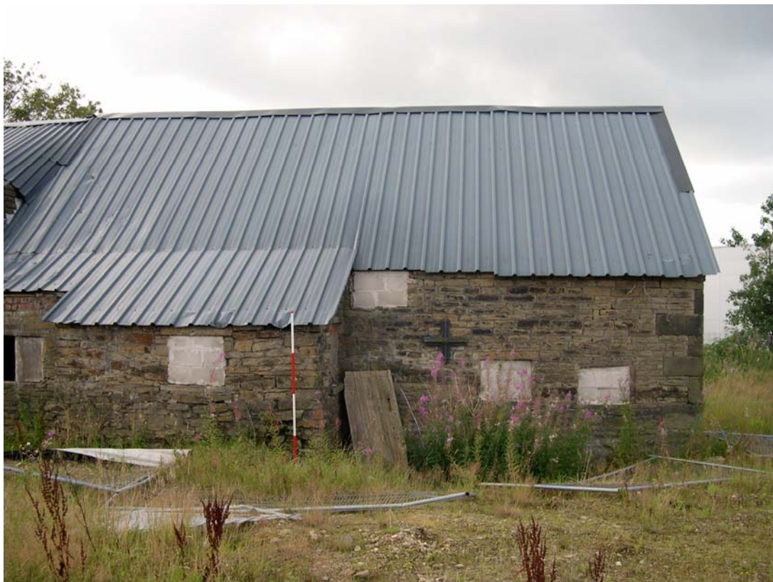
Plate 9: West end of north (rear) elevation
