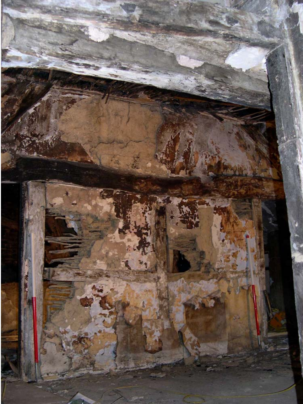
Plate 28: East wall of first floor Room 2
