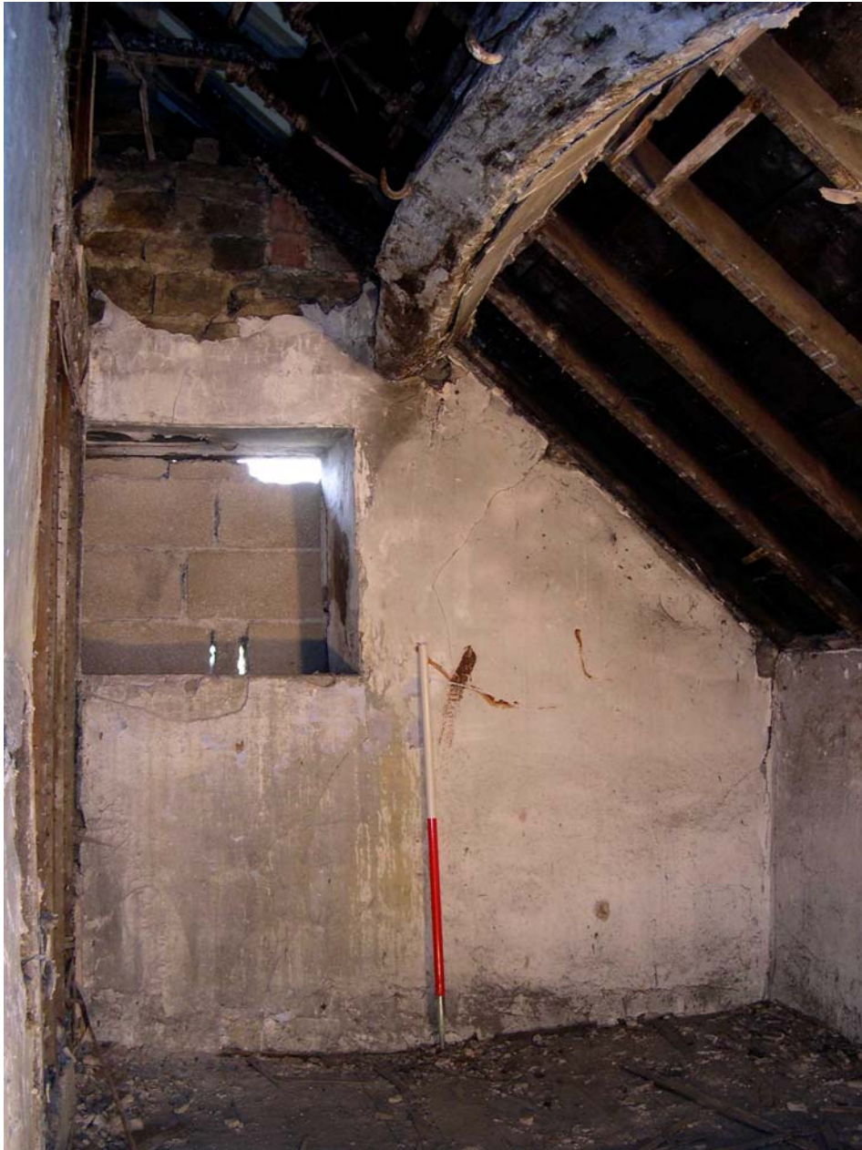
Plate 34: West elevation of first floor Room 4
