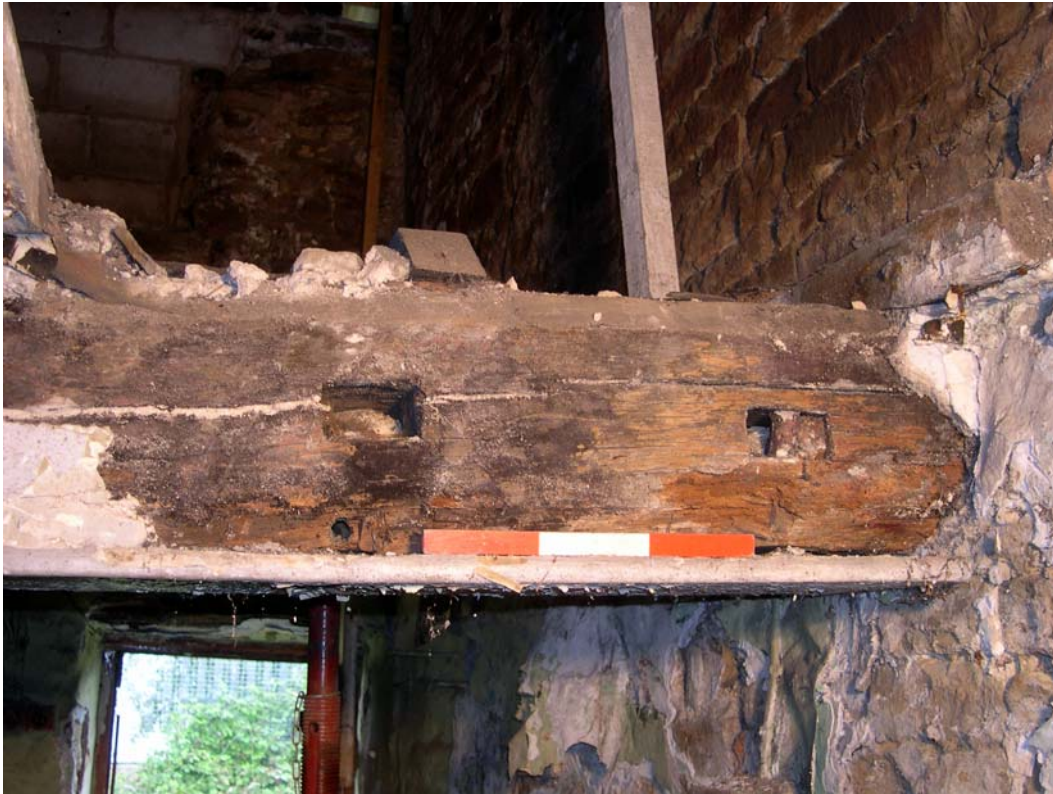
Plate 12: Empty socket holes in ceiling of ground floor Room 1
