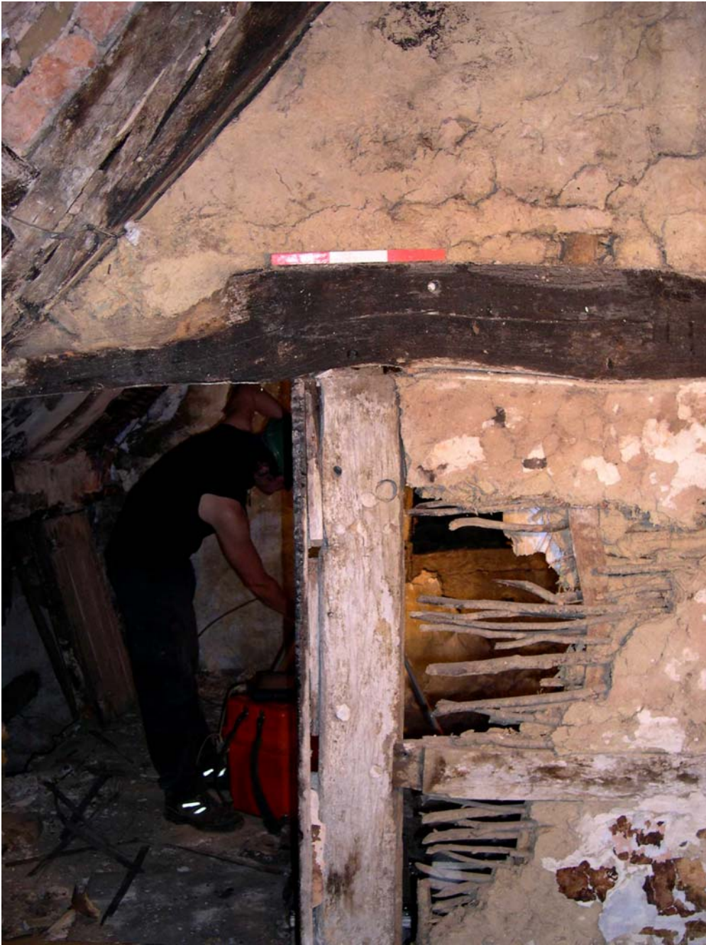
Plate 31: Detail of peg holes and joints in east wall of first floor Room 2
