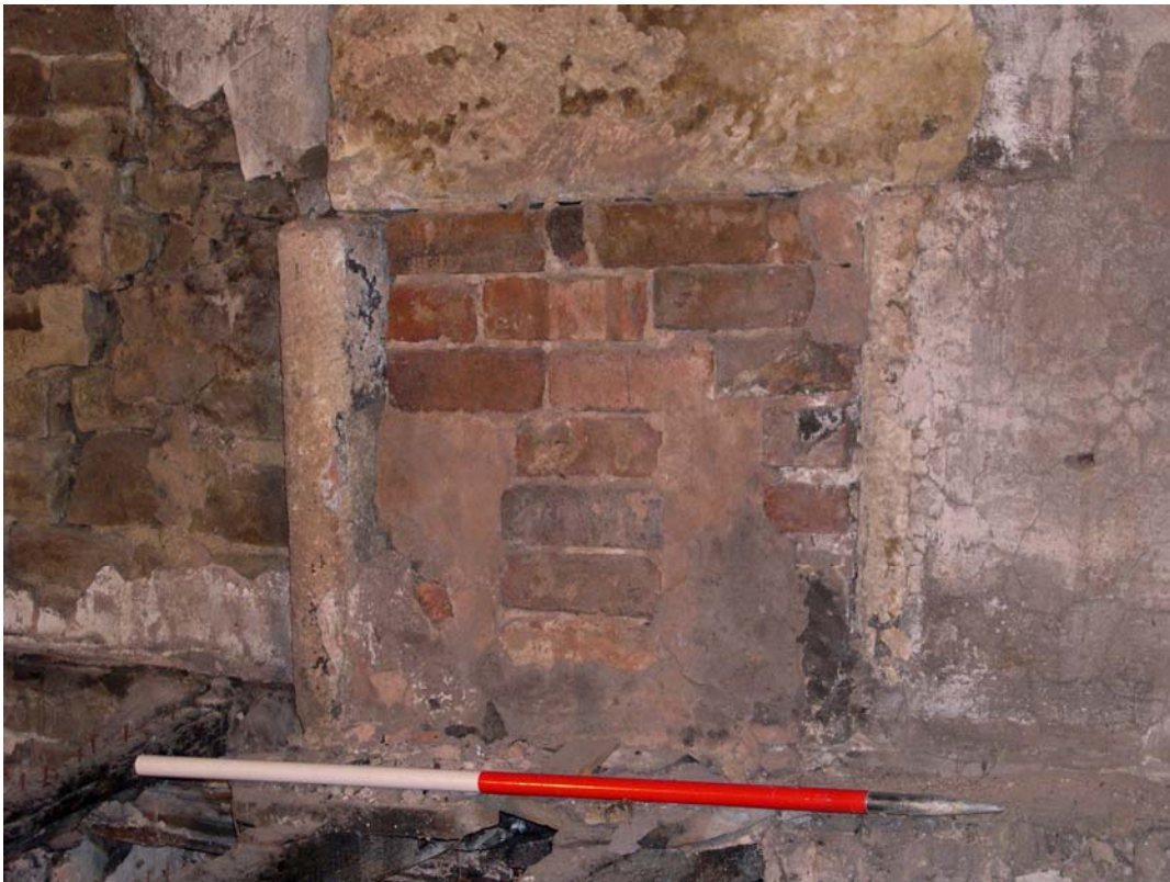
Plate 33: Fireplace in west elevation of first floor Room 3
