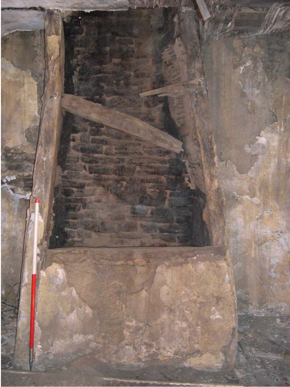
Plate 26: Front of firehood in first floor Room 1
