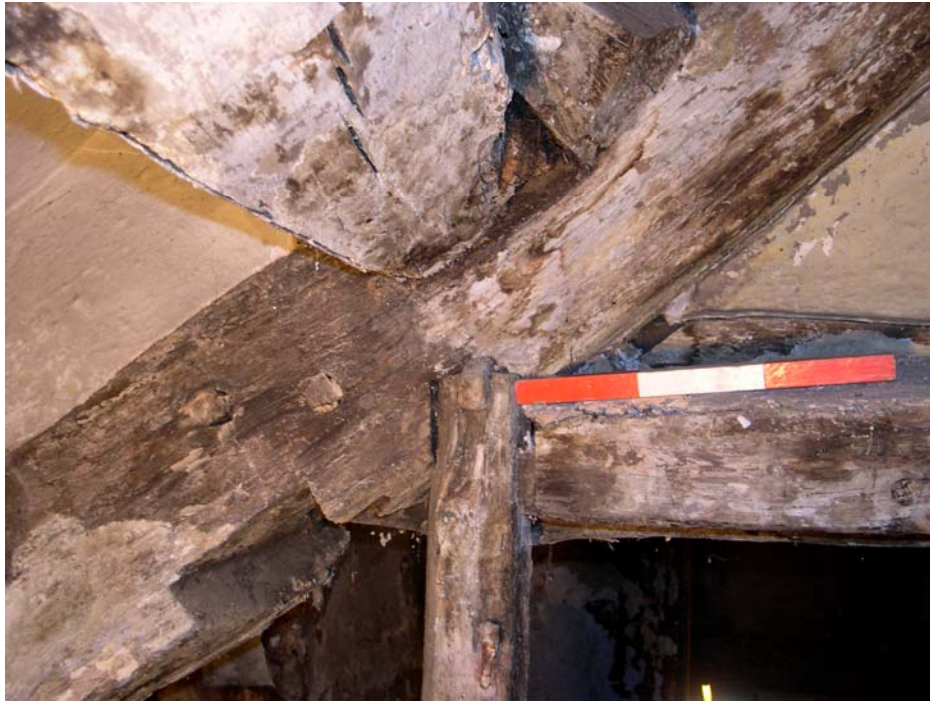
Plate 35: Joints of timbers to roof in east wall of first floor Room 4
