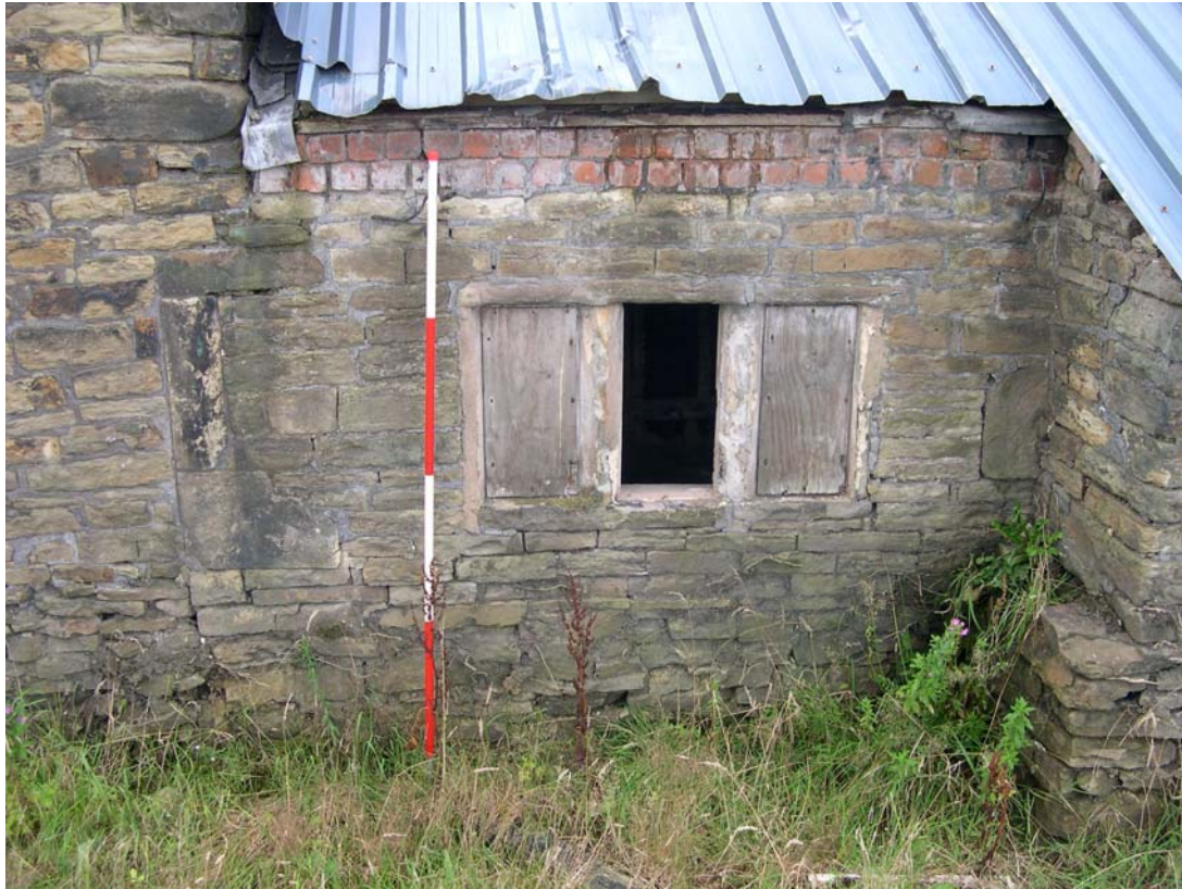
Plate 10: Detail of partial outshut in rear elevation
