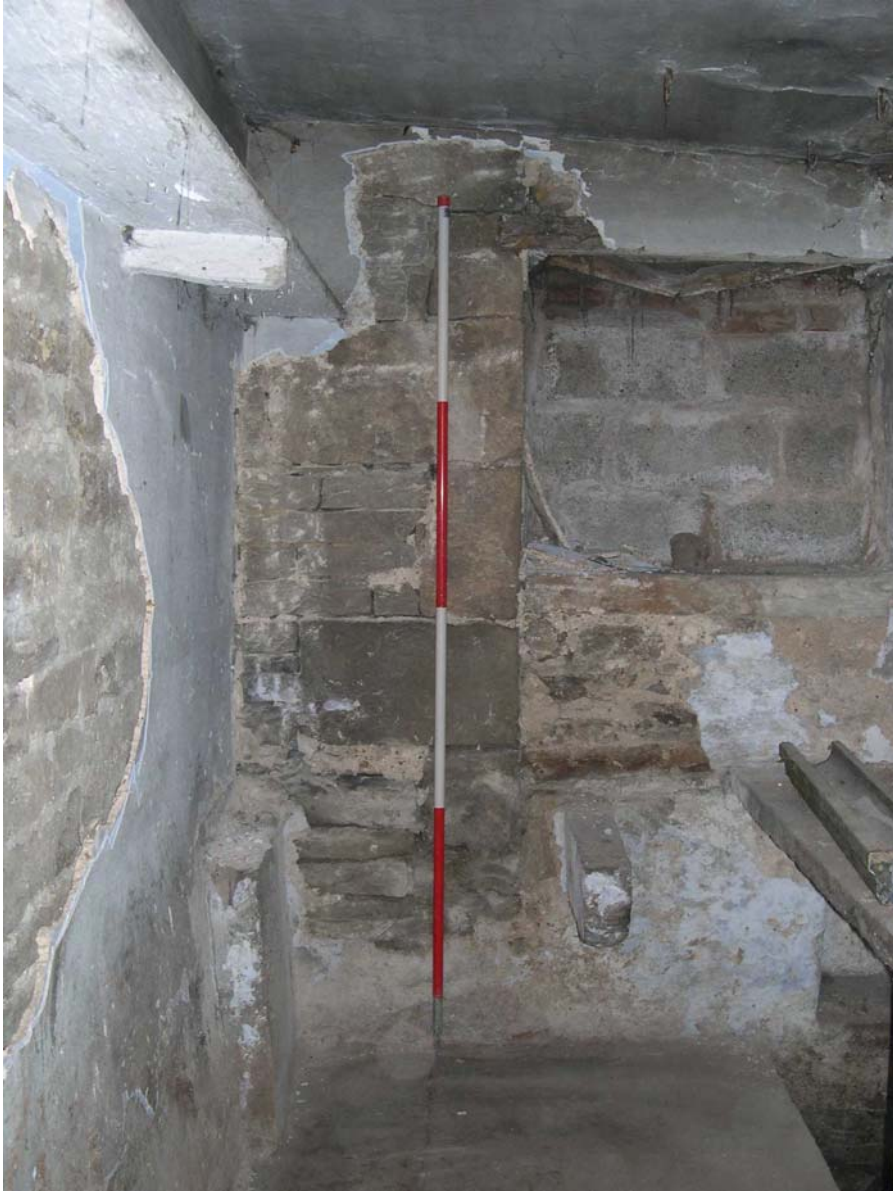
Plate 18: Quoins revealed in ground floor Room 6
