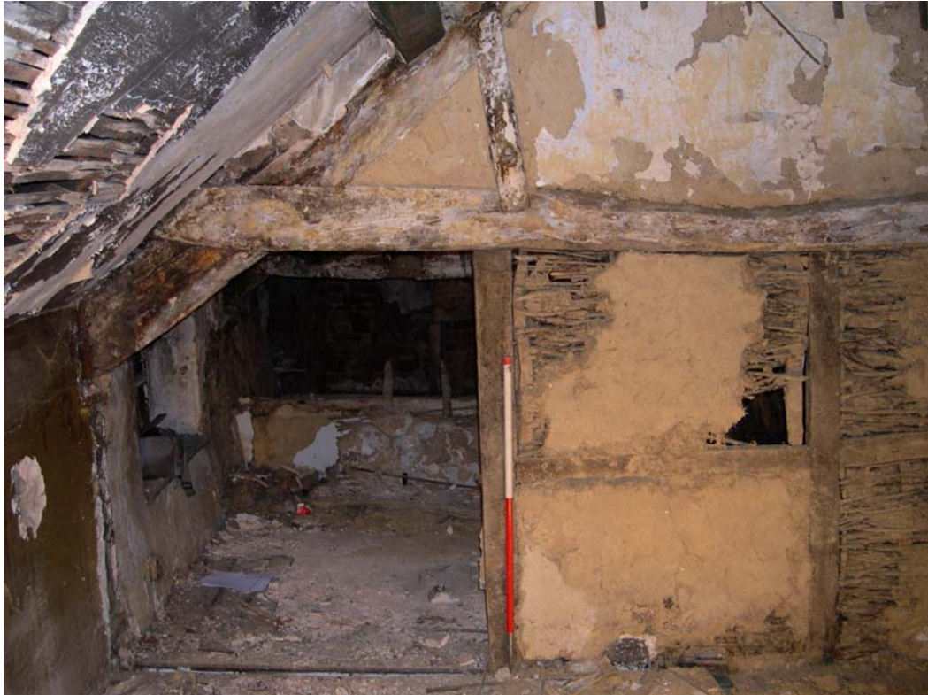
Plate 22: West wall of first floor Room 1, south end
