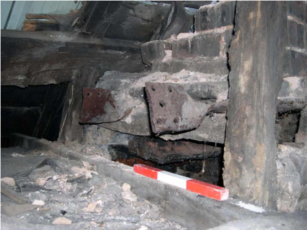
Plate 27: Chimney stack above firehood in roof space, supported by iron plates and sandstone pad
