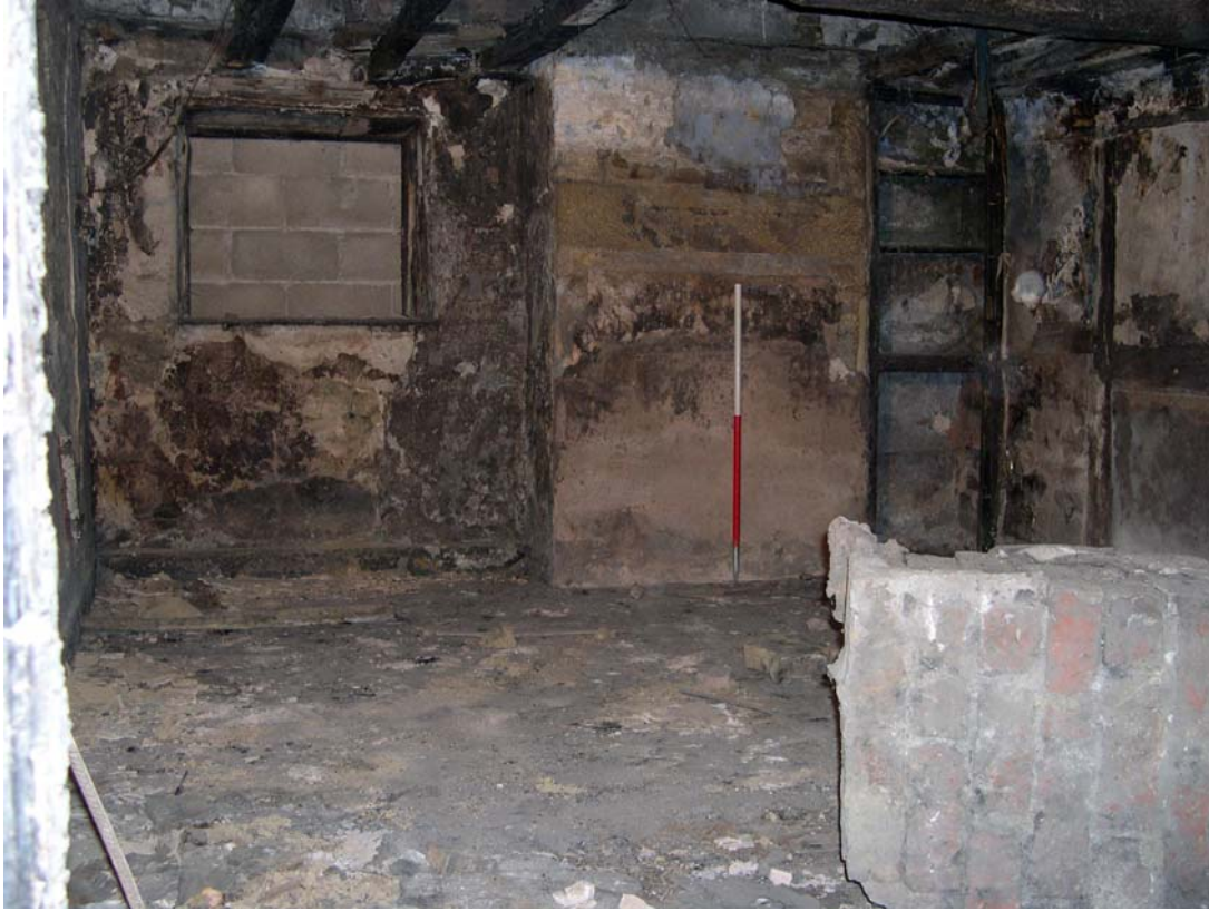
Plate 16: Fireplace in west elevation of ground floor Room 3
