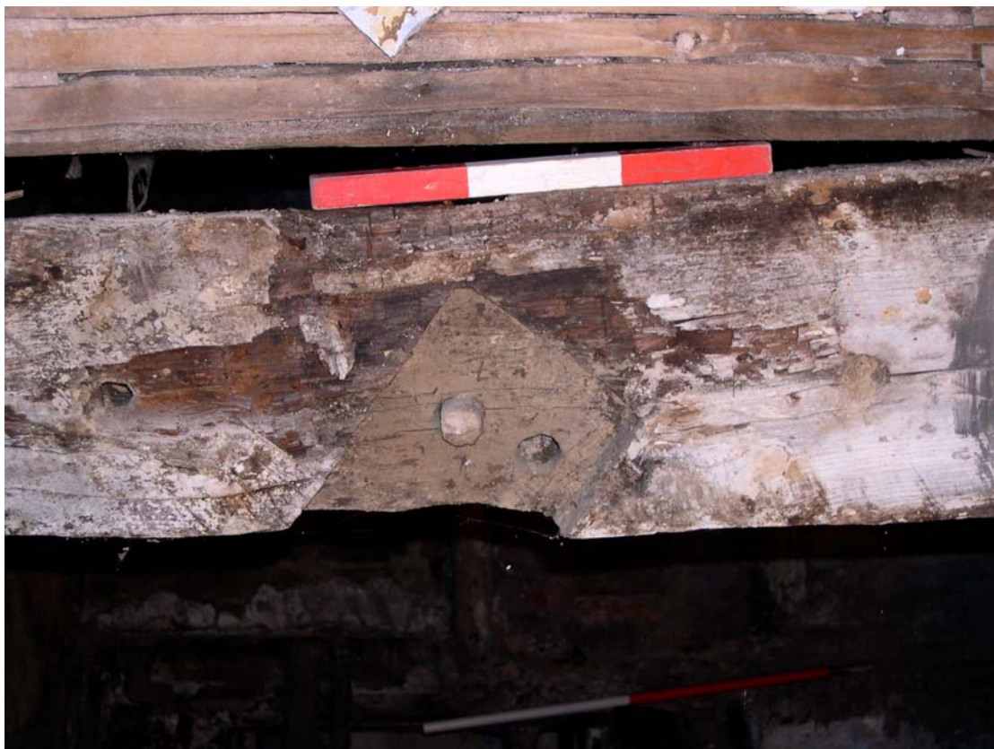
Plate 30: Empty joist slot in west wall of first floor Room 2
