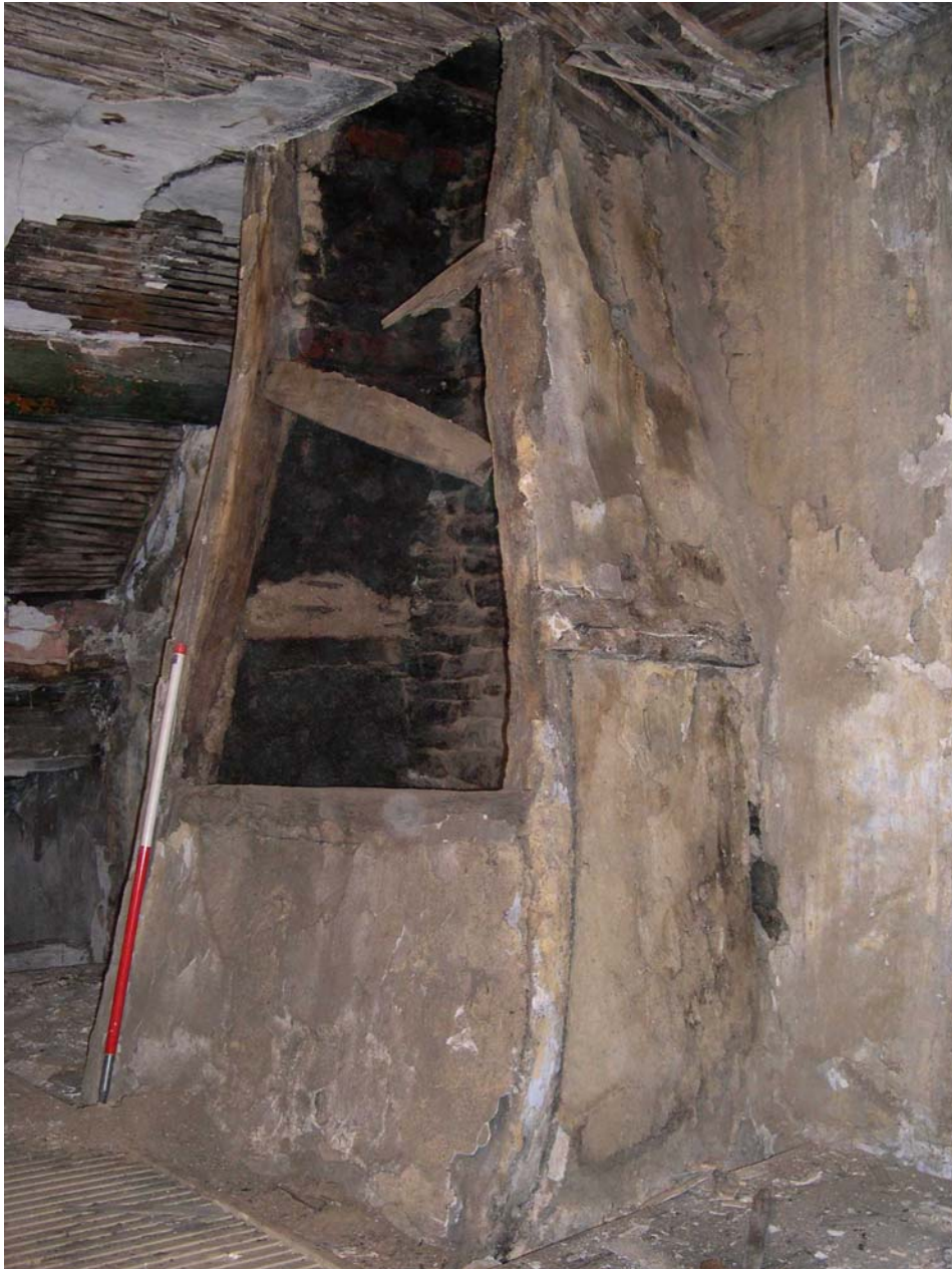
Plate 24: South side of firehood in first floor Room 1
