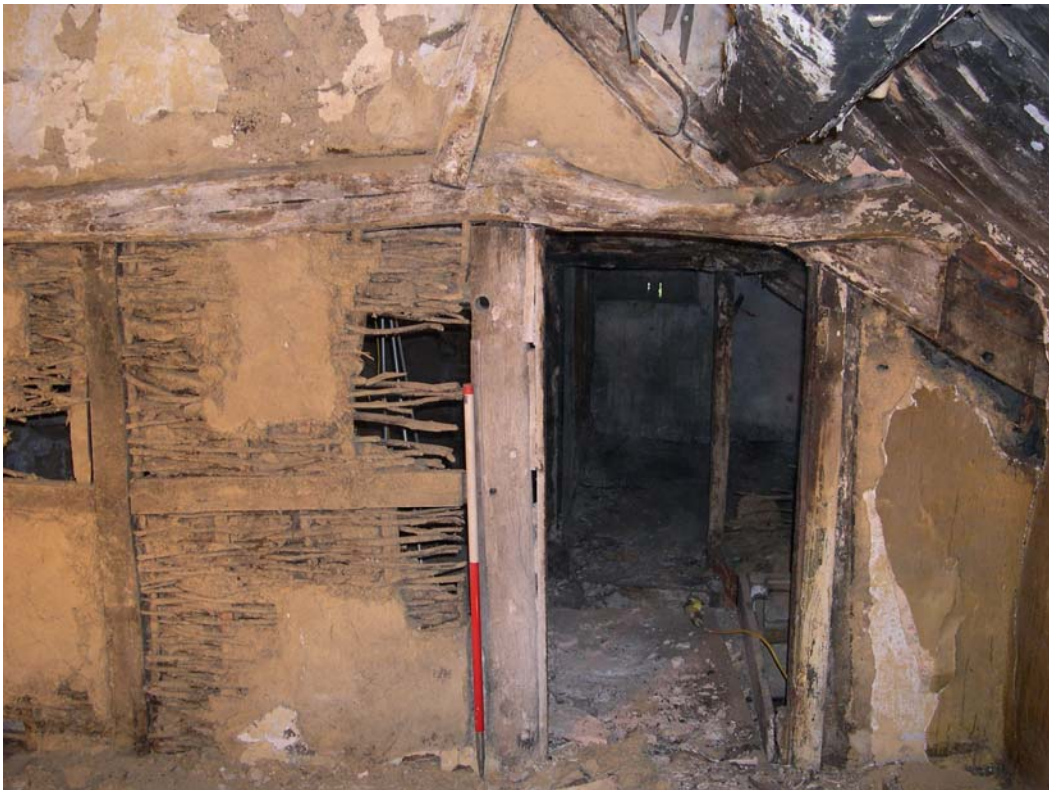
Plate 23: West wall of first floor Room 1, north end
