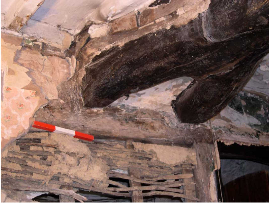
Plate 14: Forked north end of bressumer beam in ground floor Room 2
