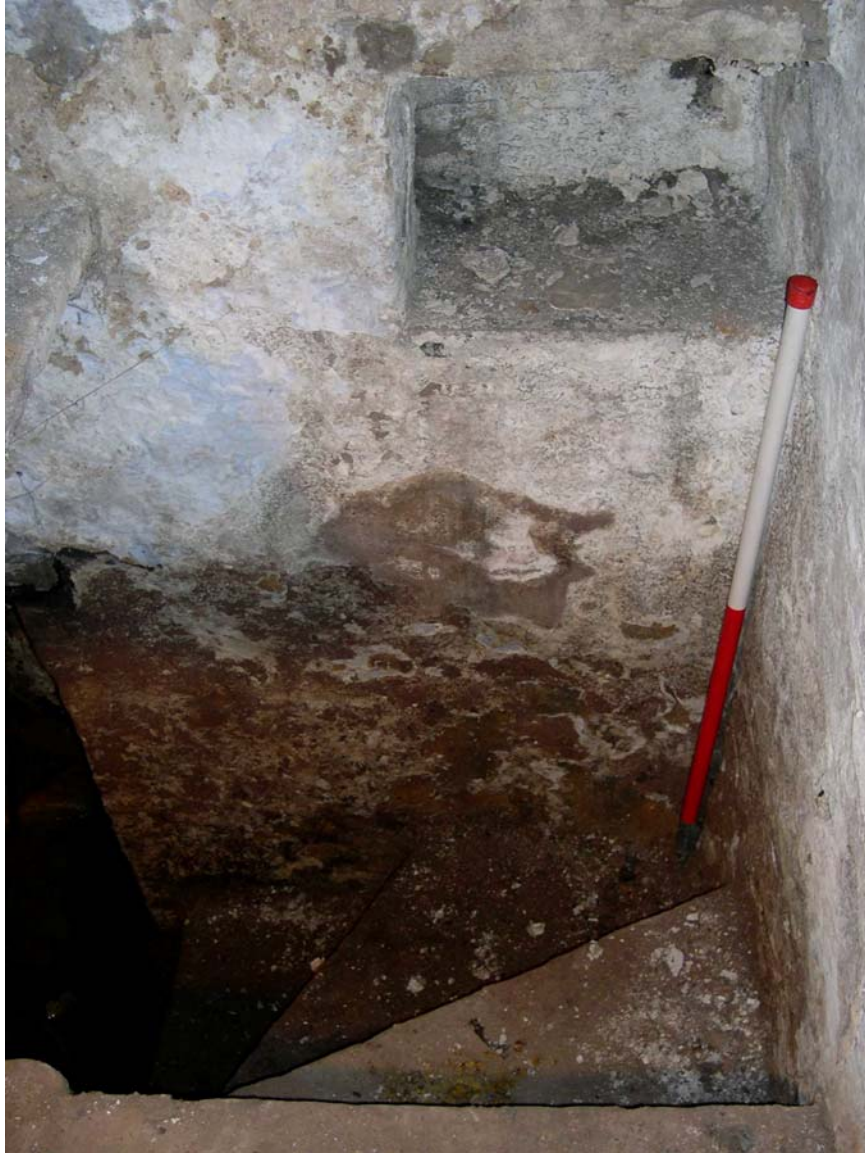
Plate 19: Stairs and alcove in ground floor Room 6
