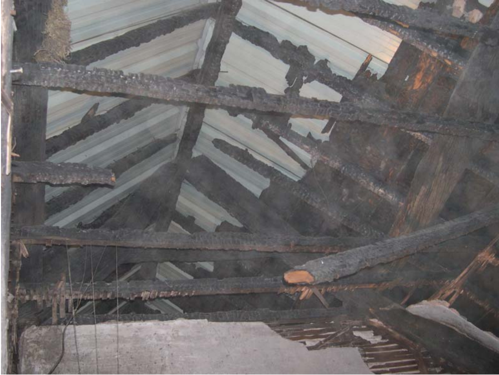
Plate 32: Remains of fire damaged roof over first floor Room 3
