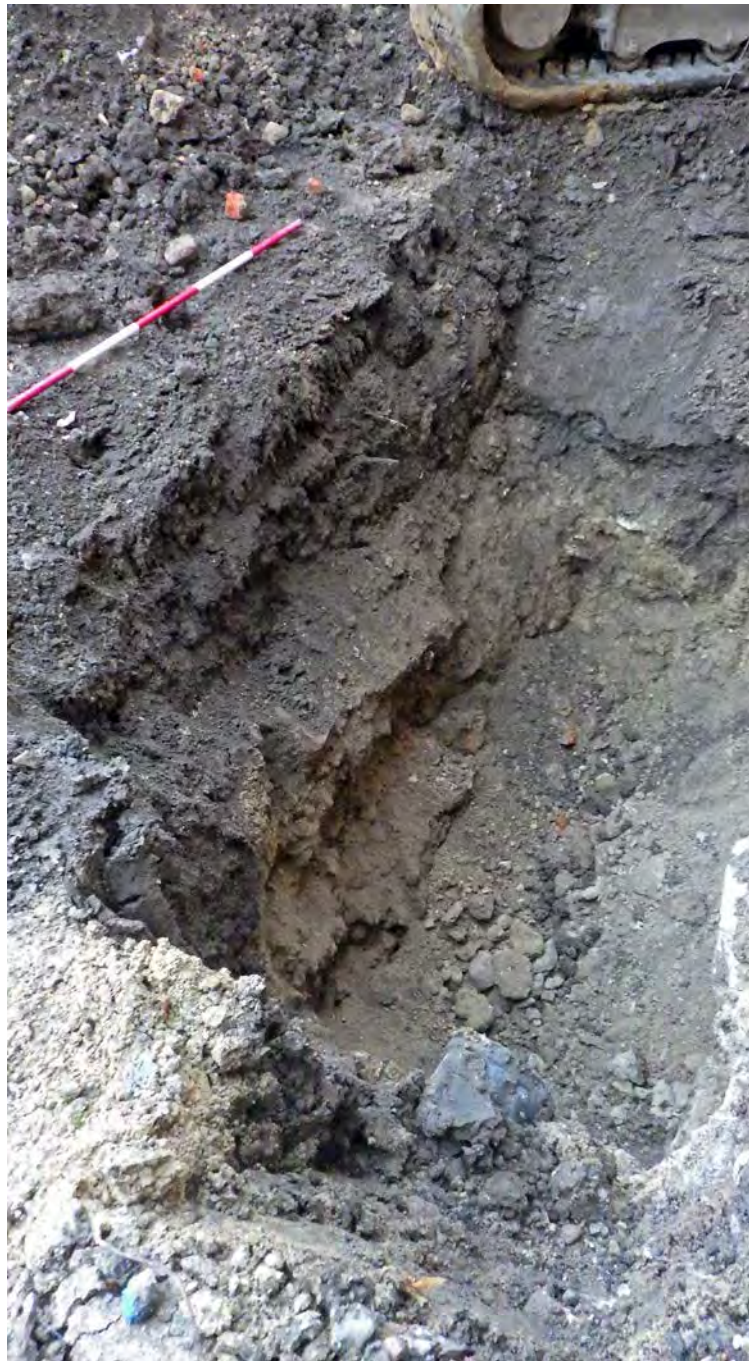
Plate 13: Chavasse Quad, section of test pit to investigate the foundations of the north wall of New Road Baptist Church, facing north-east
