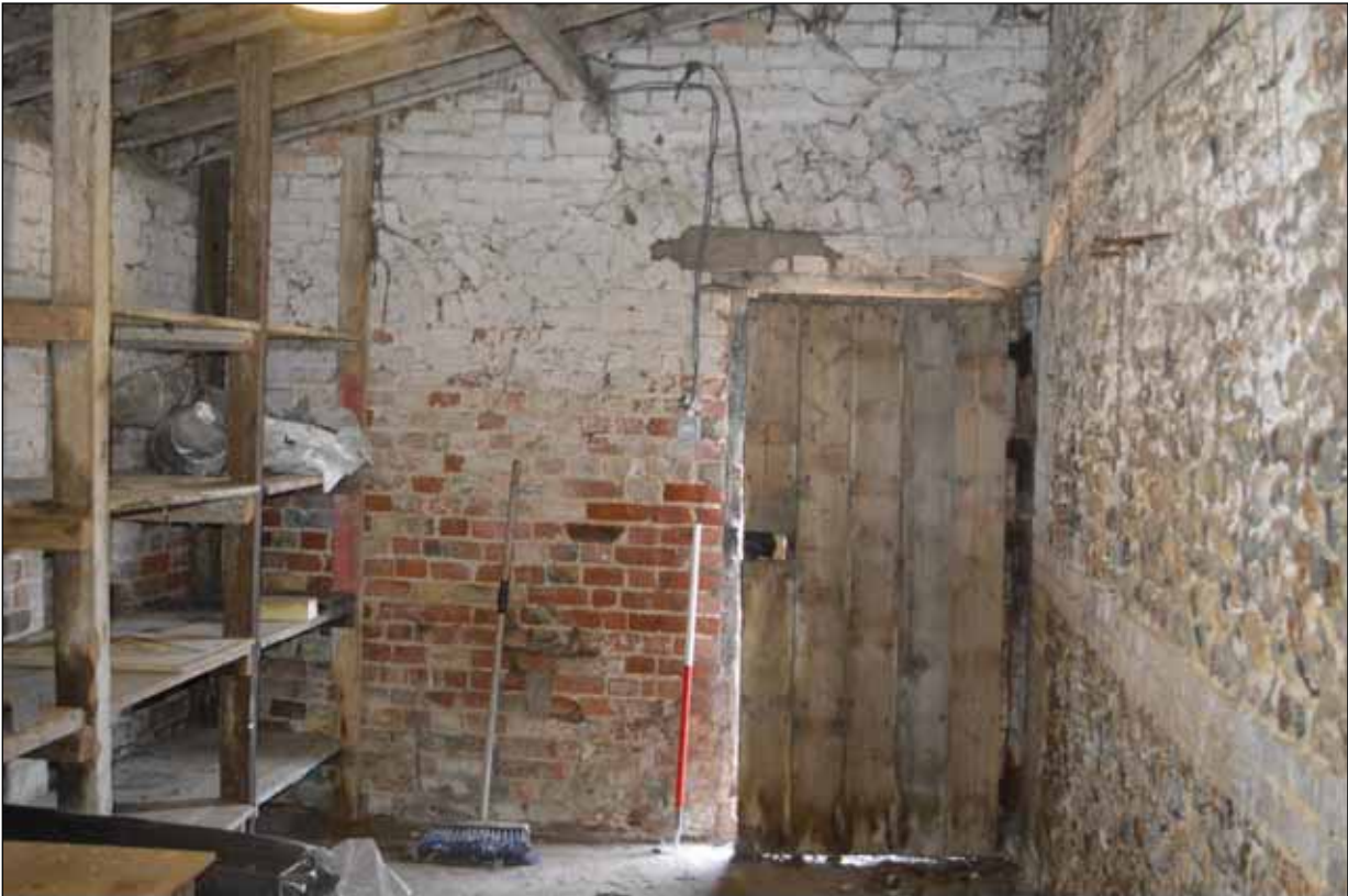
Plate 90: Internal view of the extension to Building 6a viewed from the south-east
