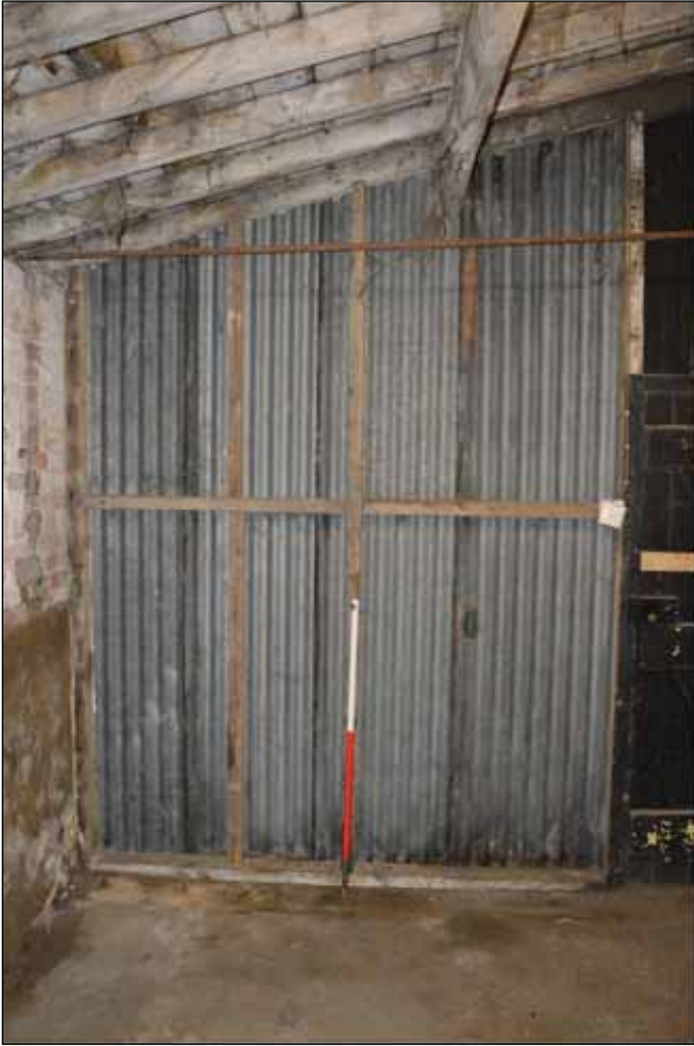
Plate 96: Detail of corrugated tin partition to Building 6a viewed from the south-west
