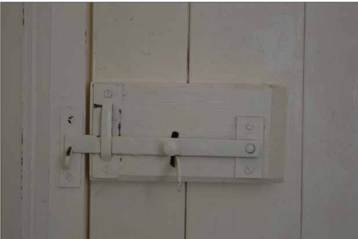
Plate 47: Building 5 - Detail of latch to toilet door (room 1)
