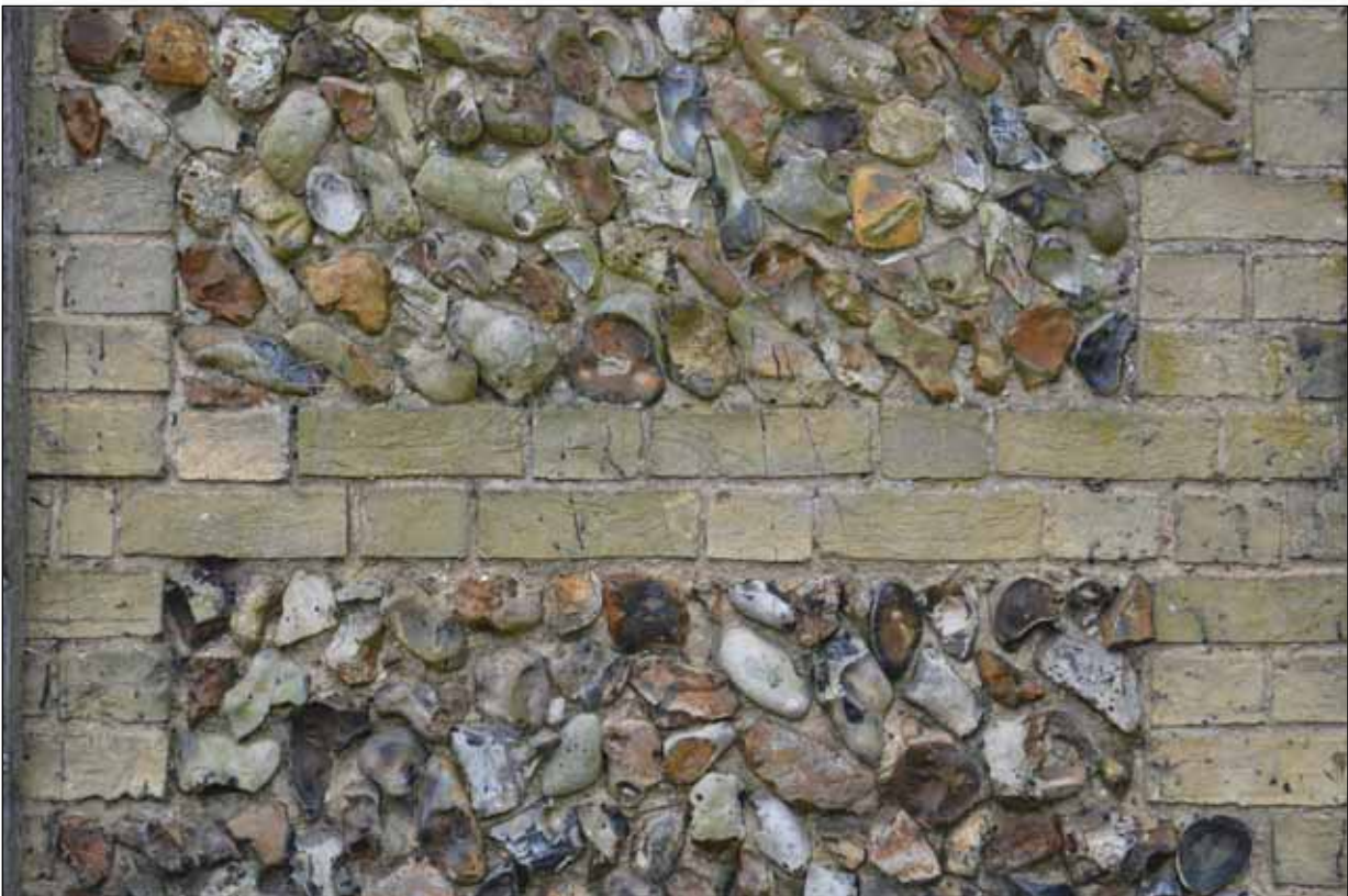
Plate 23: Building 4 - Detail of flint and brick lacing located on north-east elevation
