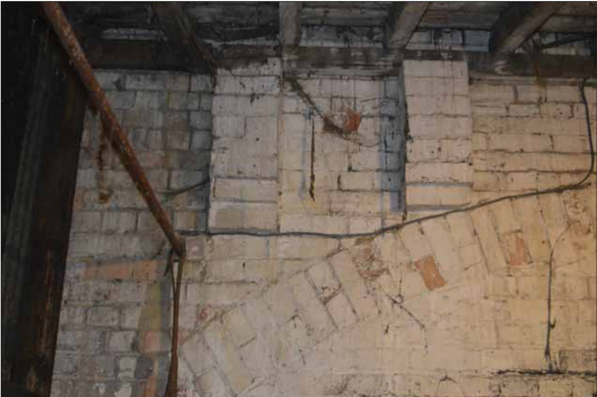
Plate 98: Detail of brick supports above blocked arch to the south-east wall of Building 6a
