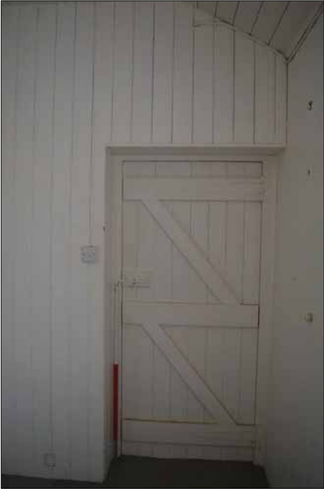
Plate 46: Building 5 - Door to office seen from kitchen area (room 1)
