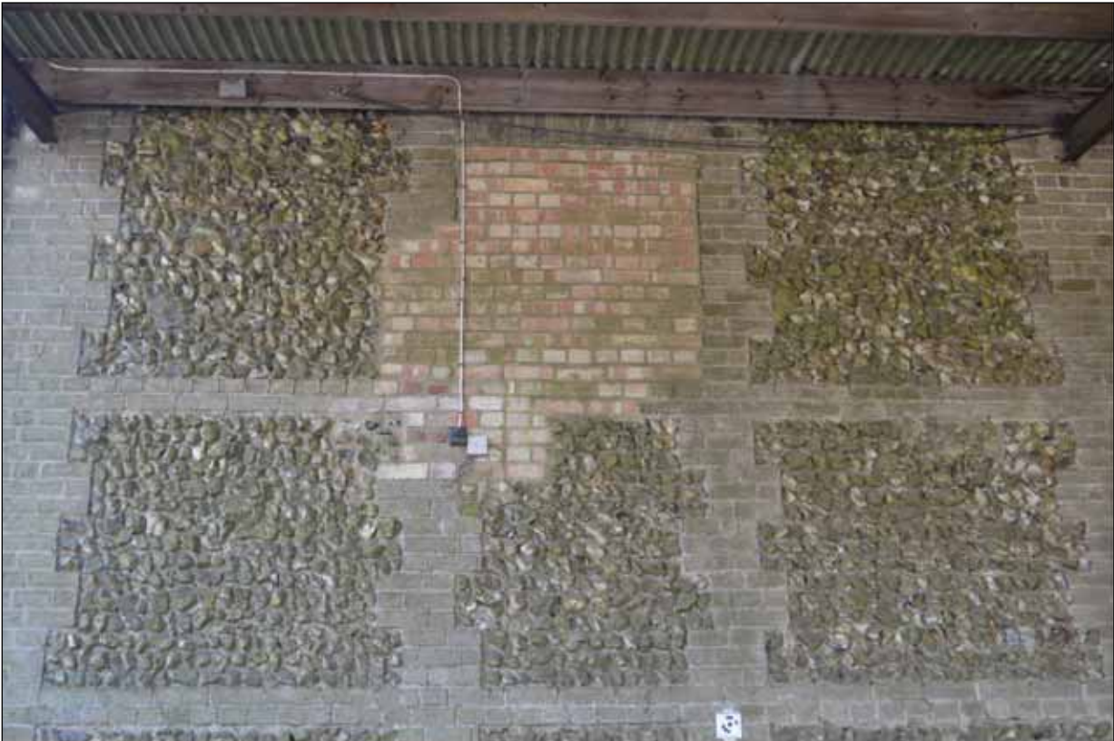
Plate 114: Building 8 - Detail of blocked window to the north-west elevation
