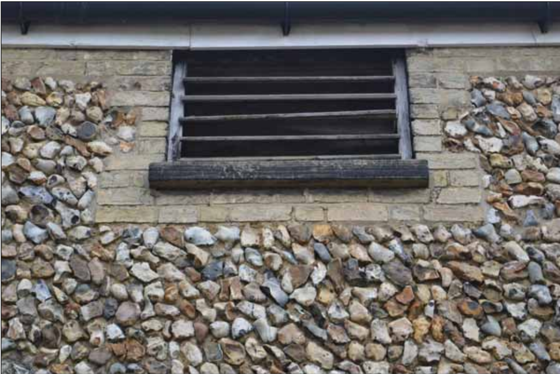
Plate 66: Building 6 - Detail of eave high ventilation window
