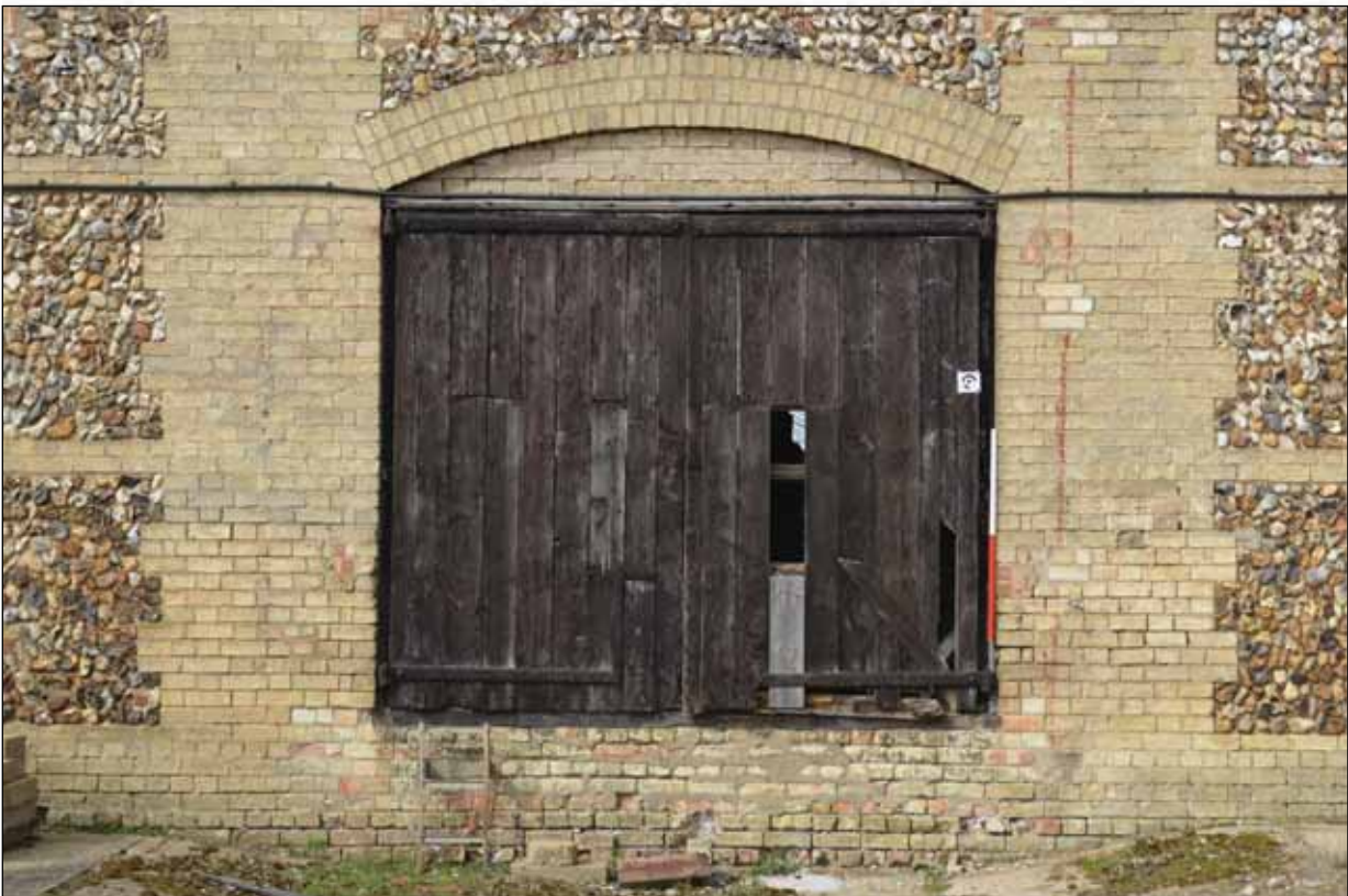
Plate 113: Building 8 - Doorway to south-east elevation
