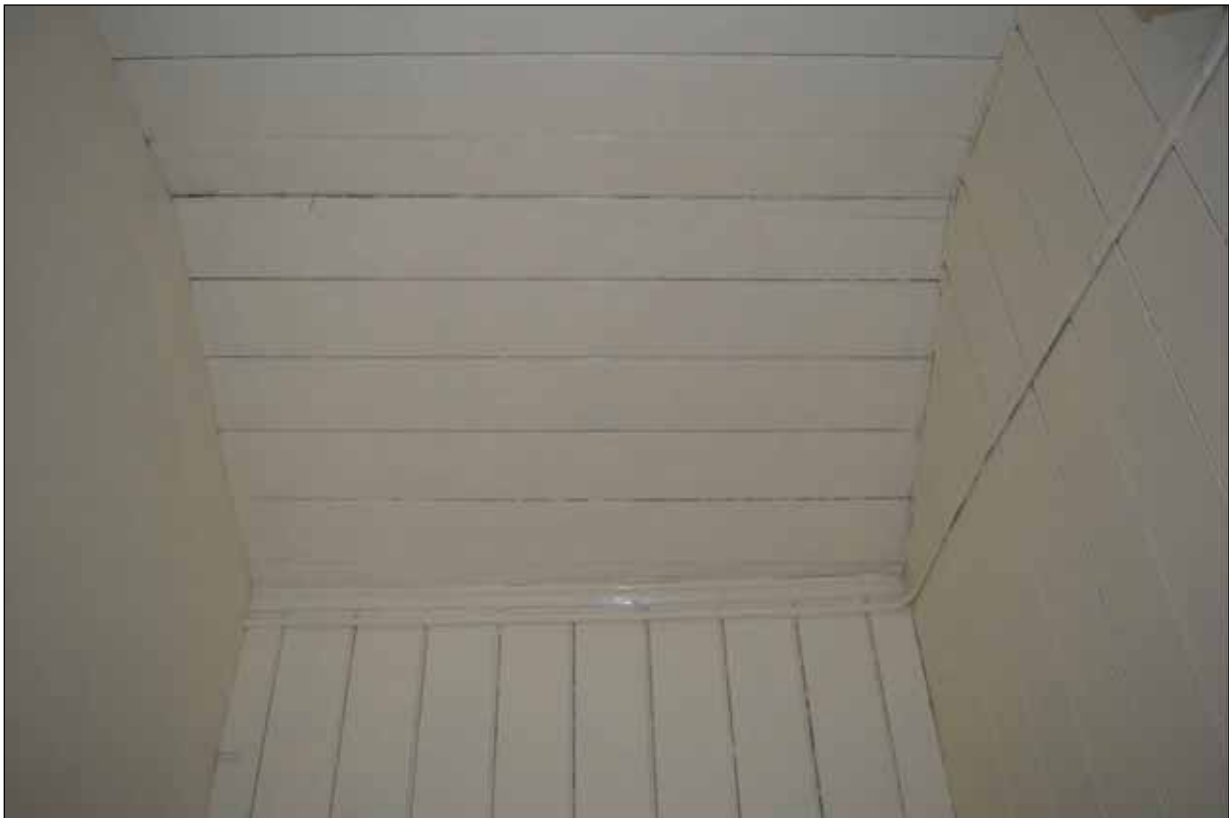
Plate 48: Building 5 - Detail of hip roof and tongue and groove wall and ceiling covering (room 1)
