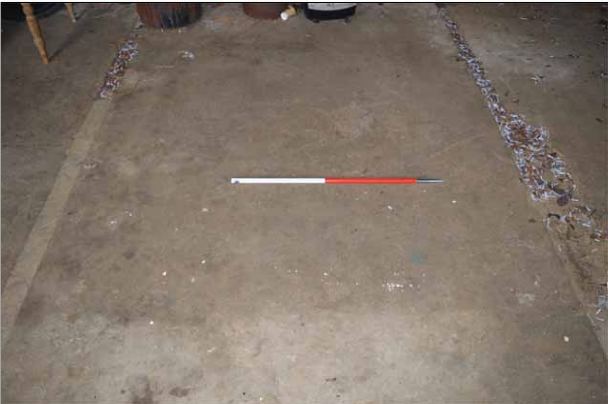
Plate 33: Building 4 - Floor surface showing stable wall divisions
