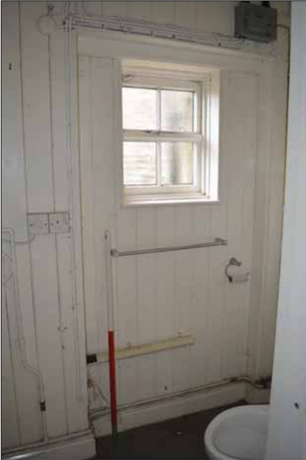
Plate 44: Building 5 - Internal view of window located to the northern end of the building
