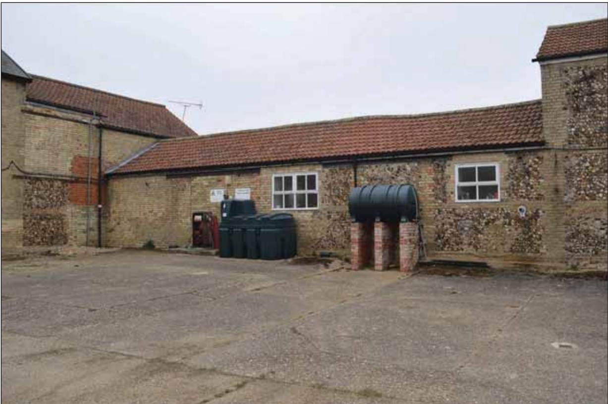
Plate 69: Building 6 - Western end of building showing in-filling viewed from the south
