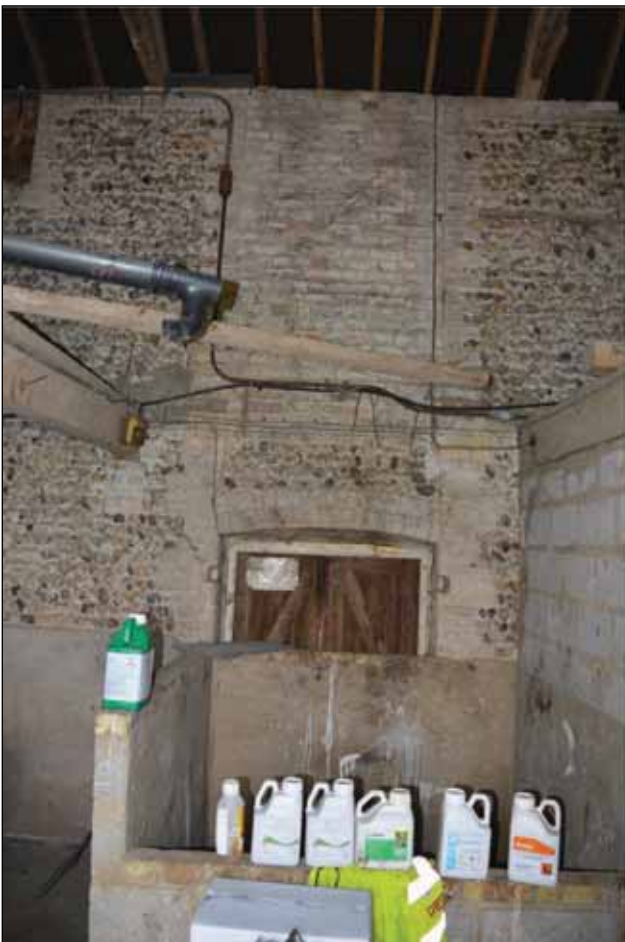
Plate 75: Building 6 - Internal view of the south-west elevation showing detail of blocked door (room a)
