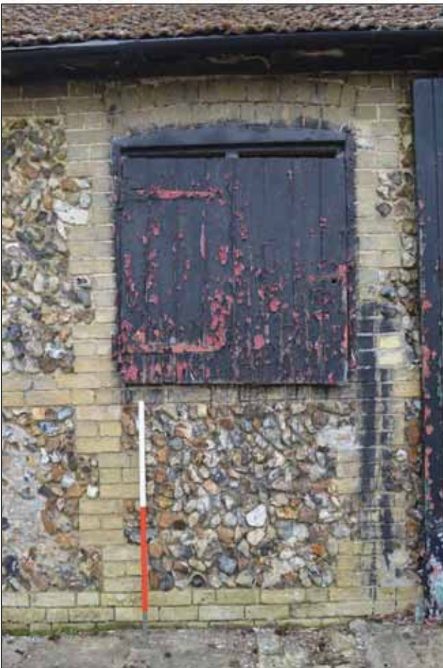
Plate 25: Building 4 - Detail of wooden shutter on the north-east elevation
