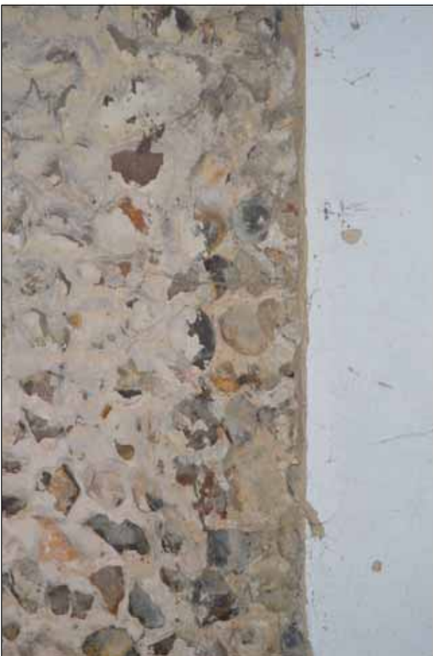
Plate 35: Building 4 - Detail of flint wall
