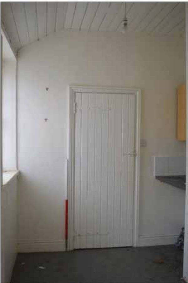
Plate 45: Building 5 - Internal wooden door located to the northern end of the building
