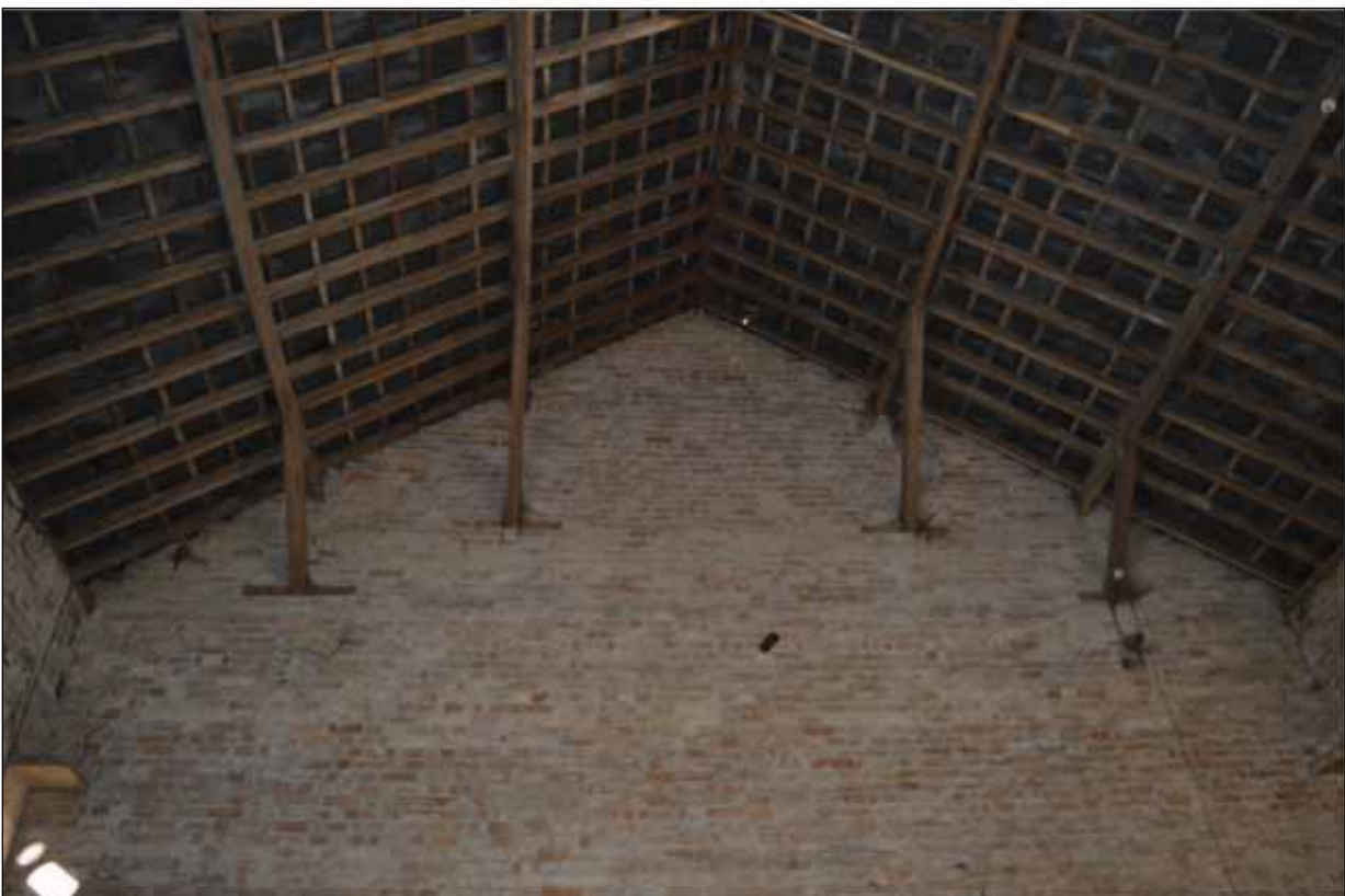
Plate 125: Building 8 - Detail of roof structure to the north eastern elevation viewed internally
