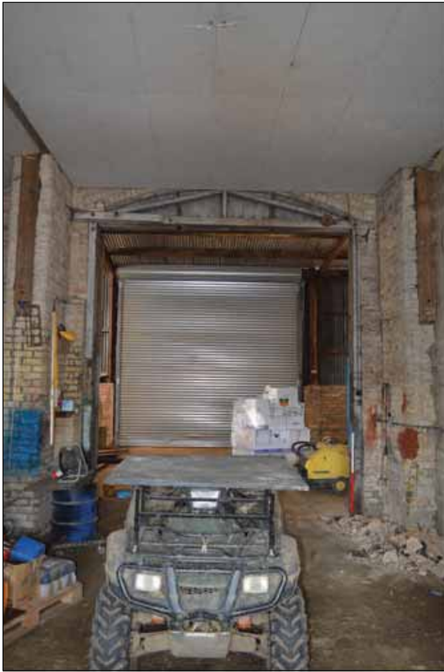
Plate 130: Modern metal shutter to the north-west elevation of Building 8
