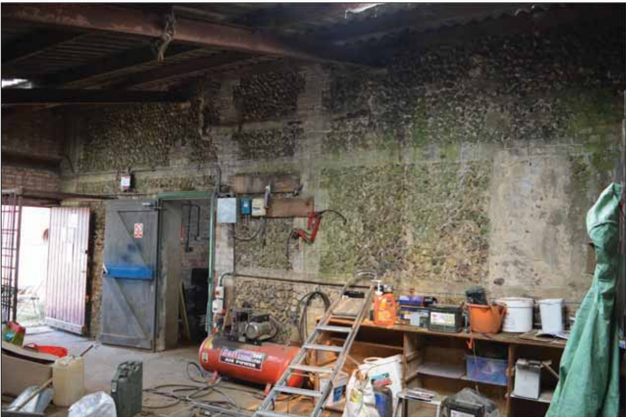
Plate 133: South-west elevation of Building 8 seen internally from modern lean to
