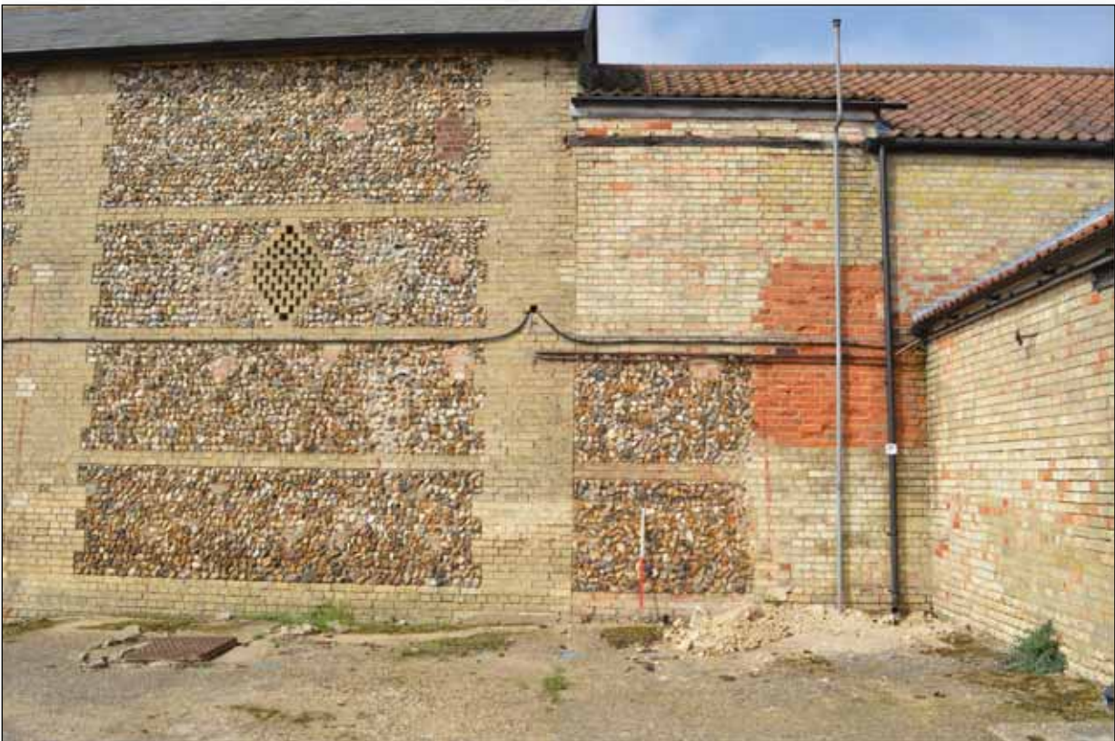
Plate 109: North-east end of Building 8 showing later brick in fill
