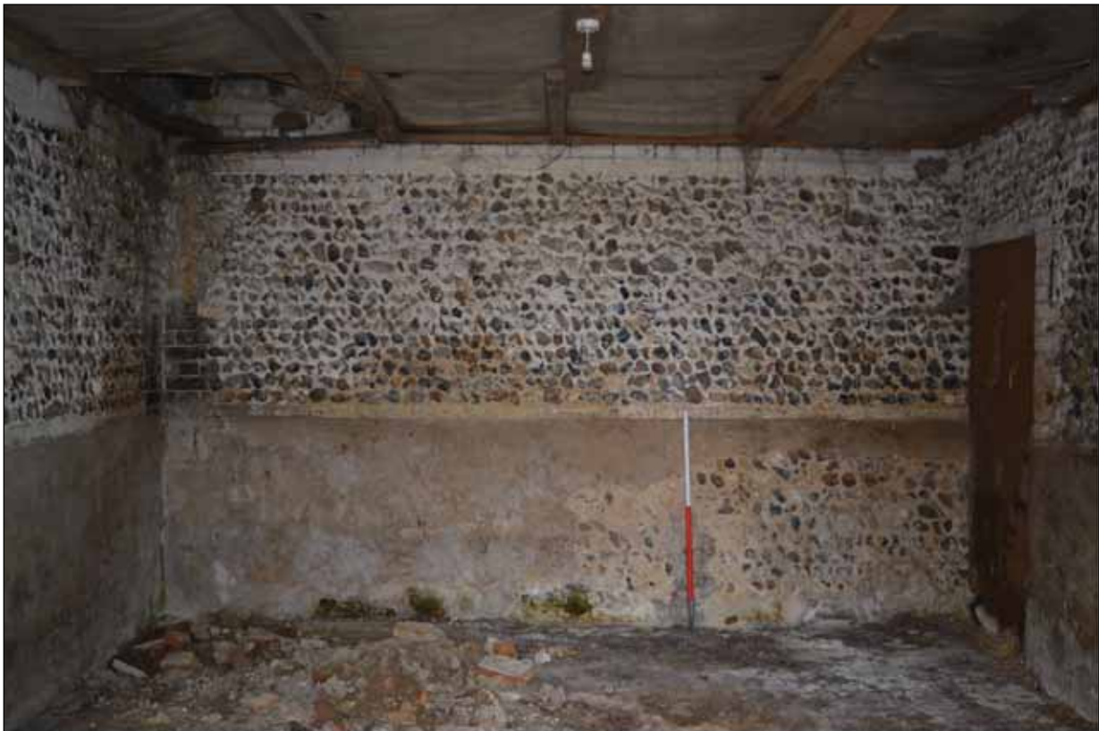
Plate 16: Building 4 - Internal view of the stable viewed from the north-east
