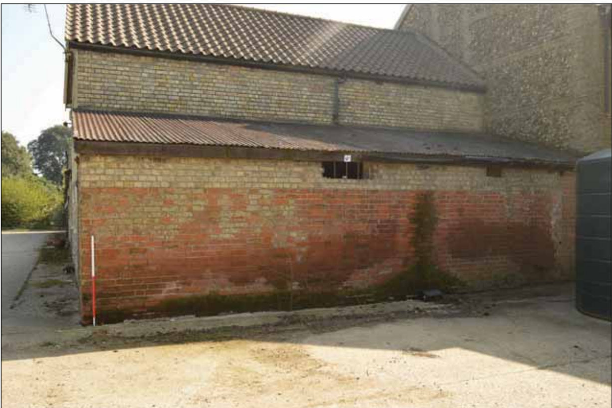
Plate 87: Extension to the north-west end of Building 6a viewed from the north-west
