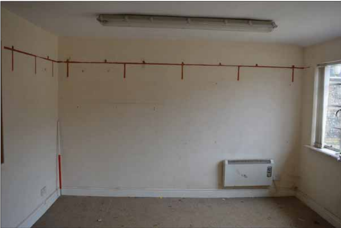
Plate 57: Building 5 - South-western wall of building (room3)
