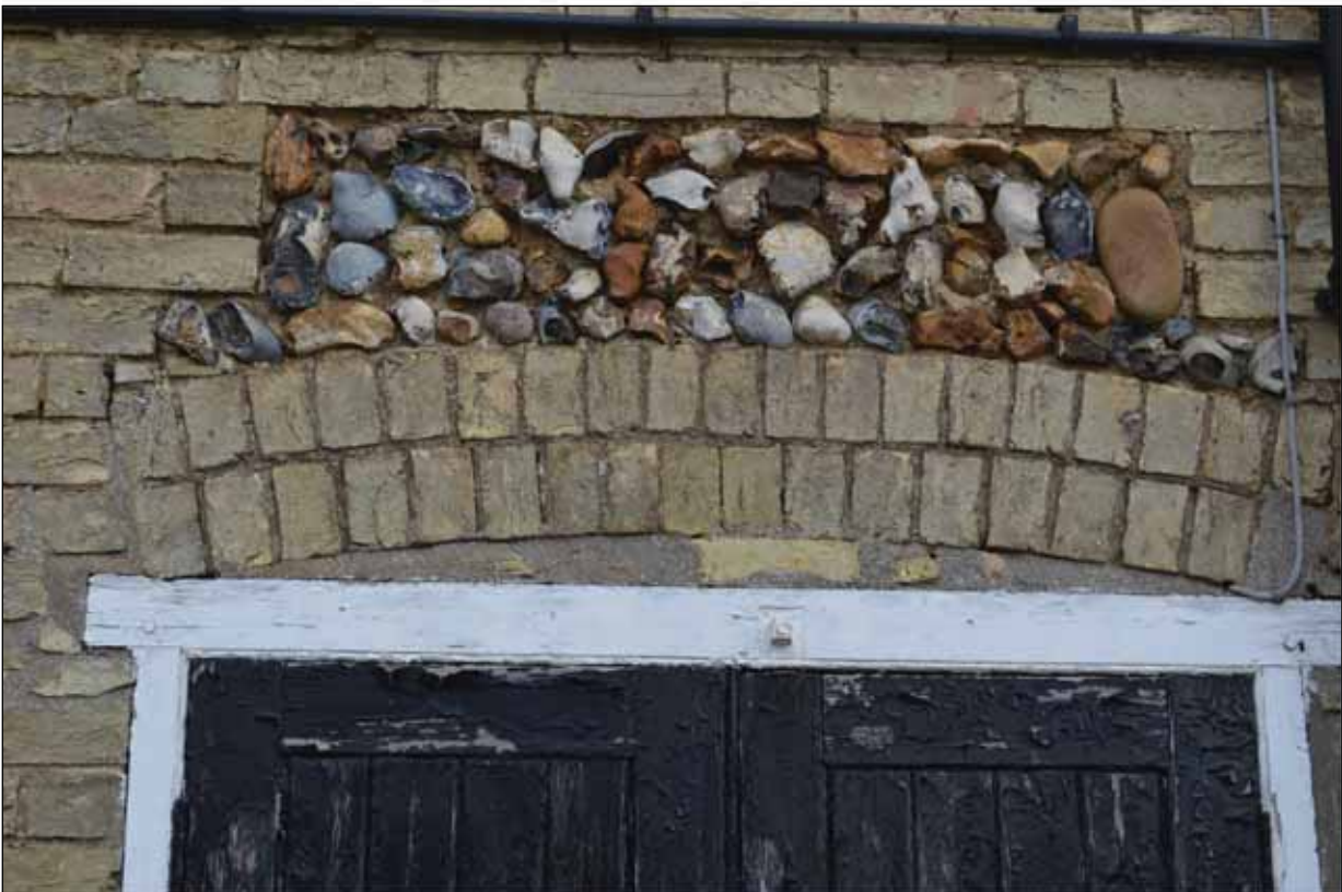
Plate 65: Building 6 - Detail of flint dressing
