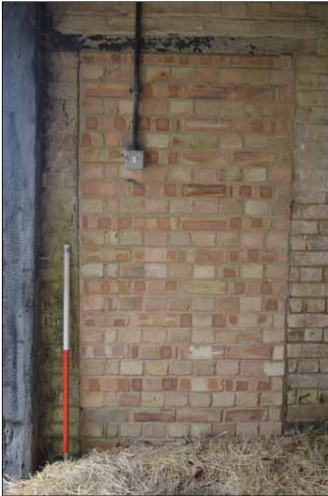
Plate 106: Blocked door to the south-east wall of Building 7
