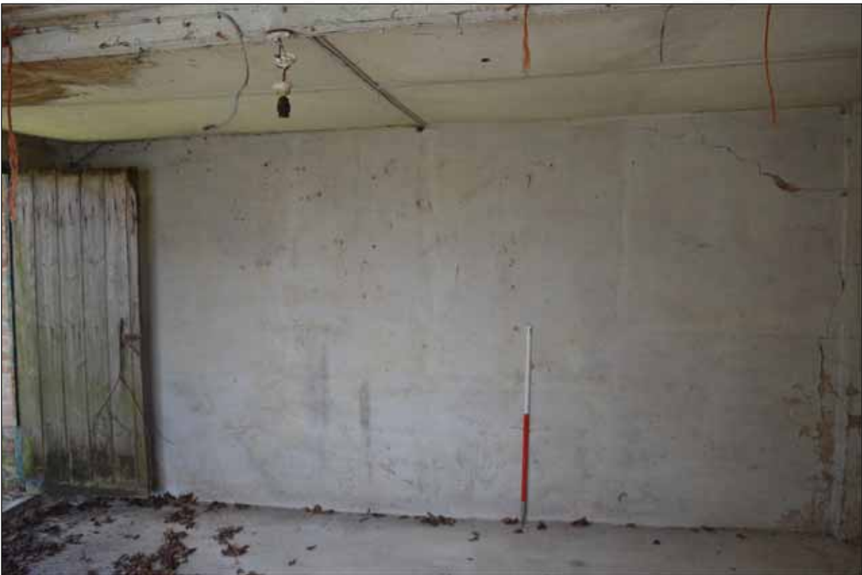
Plate 141: Wall to north-east wall of Building 11 viewed internally
