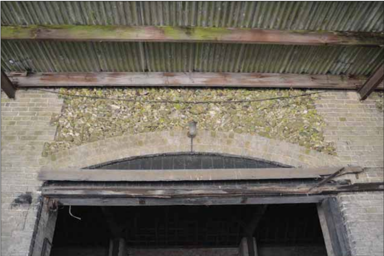
Plate 118: Building 8 - Brick arch and flint work above door to north-west elevation
