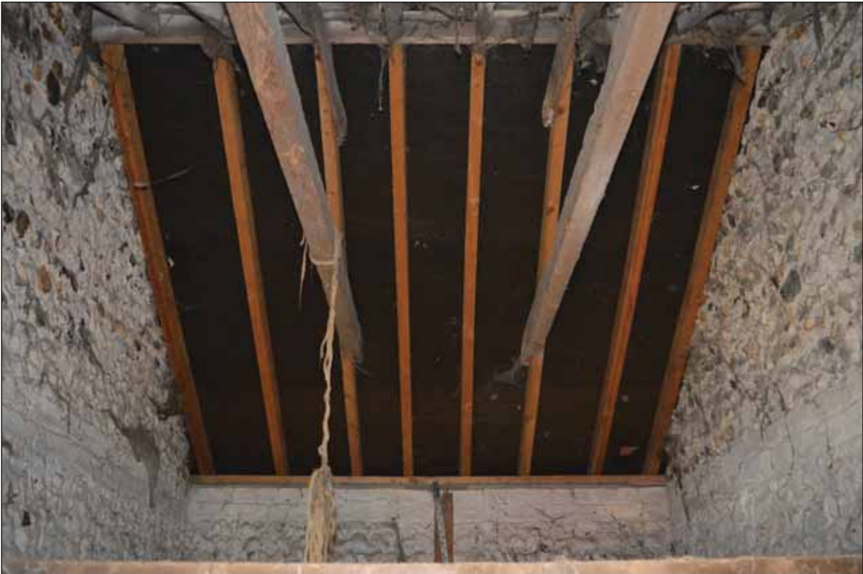
Plate 62: Building 5a - Detail of roof structure
