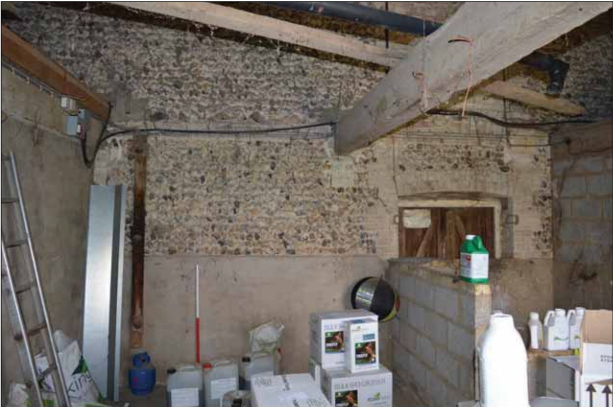
Plate 76: Building 6 - Detail of flint and rendered wall to the south-west elevation
