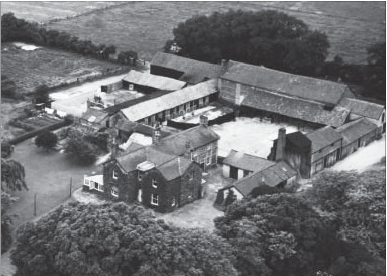
Figure 6: Aerial photograph of Hill House Farm from the south-west
