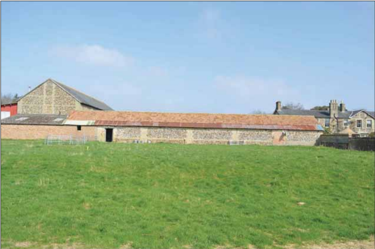
Plate 22: Rear of Building 4 viewed from south-west
