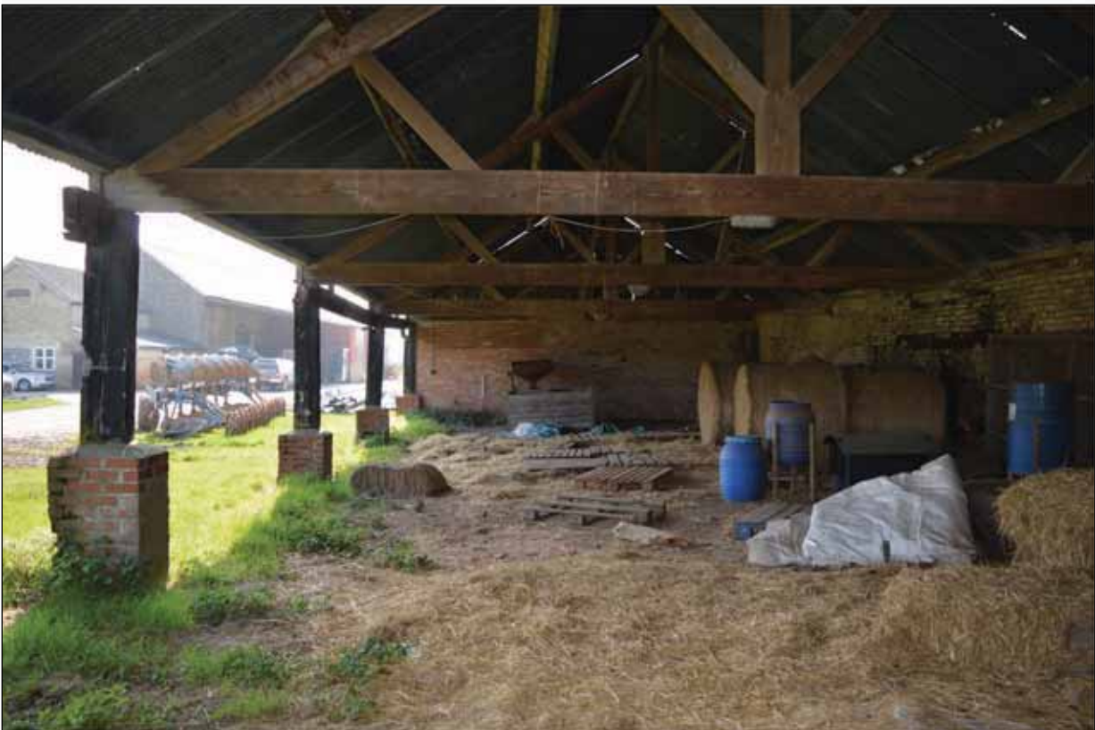
Plate 9: Building 1 - Internal view of the southern end of the building viewed from the north-east
