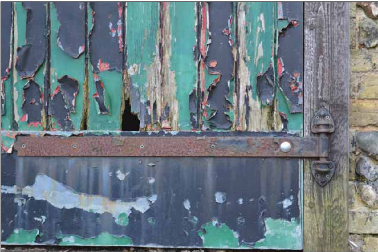
Plate 28: Building 4 - Detail of strap hinge on door to the north-east elevation
