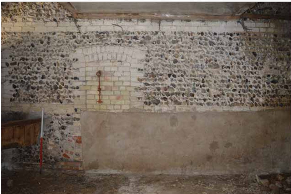
Plate 17: Building 4 - Internal view of the eastern wall
