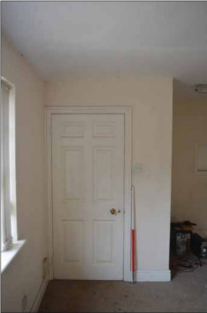
Plate 56: Building 5 - Door leading to foyer on north-eastern wall (room 3)
