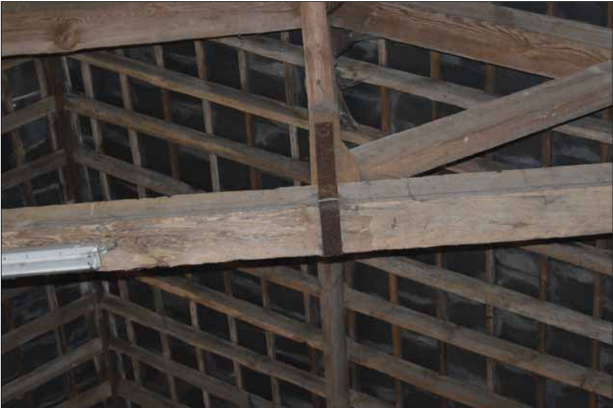
Plate 128: Detail of iron banding to trusses in Building 8
