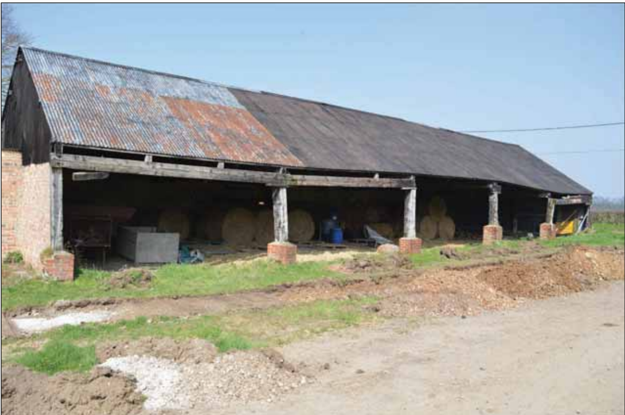
Plate 5: Building 1 - Open fronted viewed from the south
