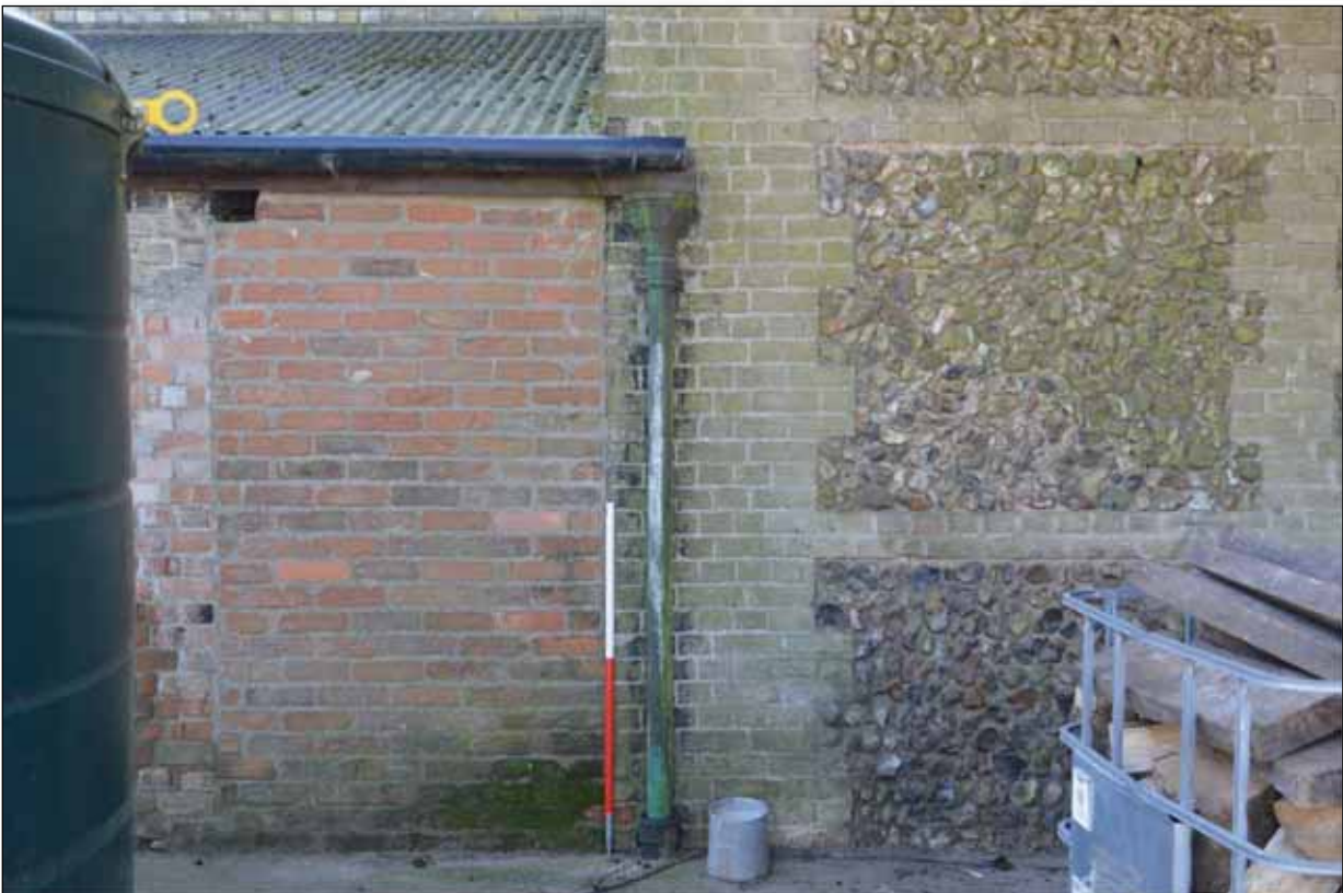
Plate 89: Building 6a - Detail of blocked door
