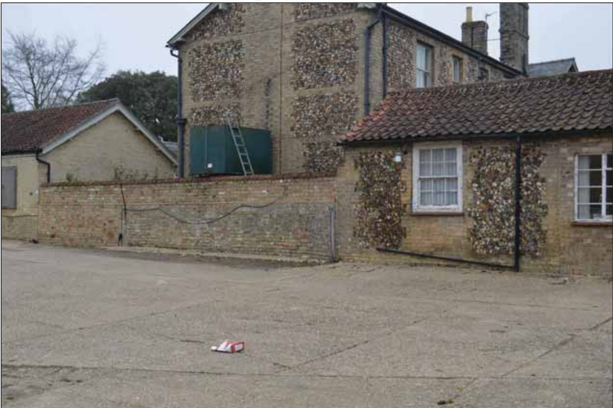
Plate 41: Building 5 - Detail of added wall to the northern end of the building
