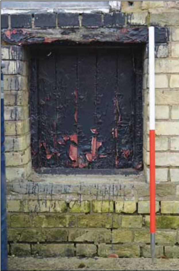
Plate 26: Building 4 - Detail of recessed window and wooden shutter on north-east elevation
