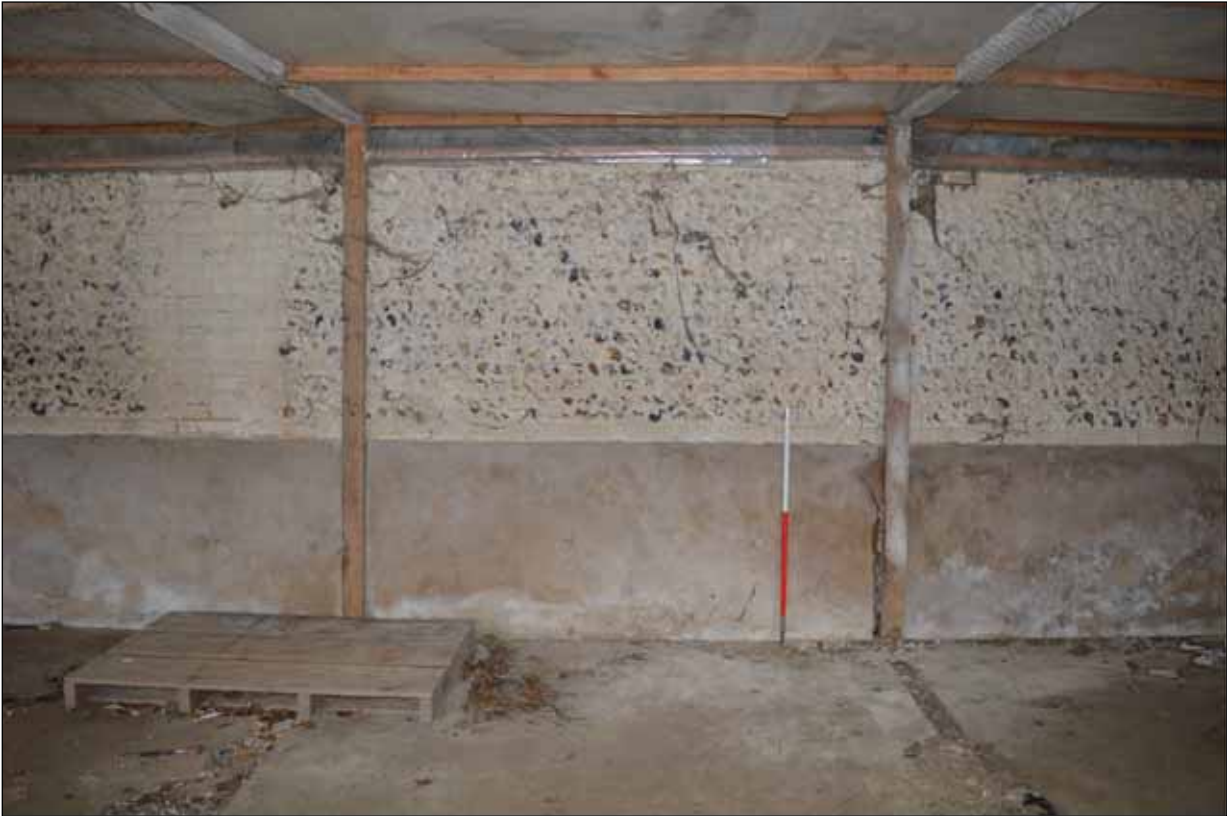
Plate 34: Building 4 - Internal view of wall to the rear of the building
