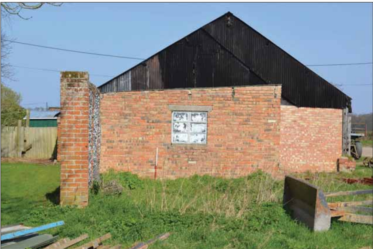
Plate 137: Building 11 and perimeter wall viewed from the south-west
