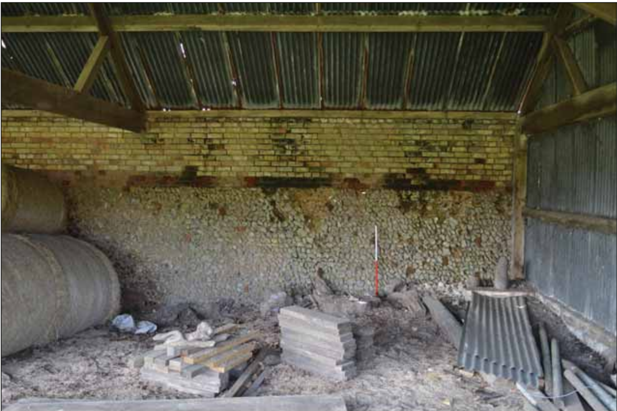
Plate 12: Building 1 - Rear wall viewed internally from the east
