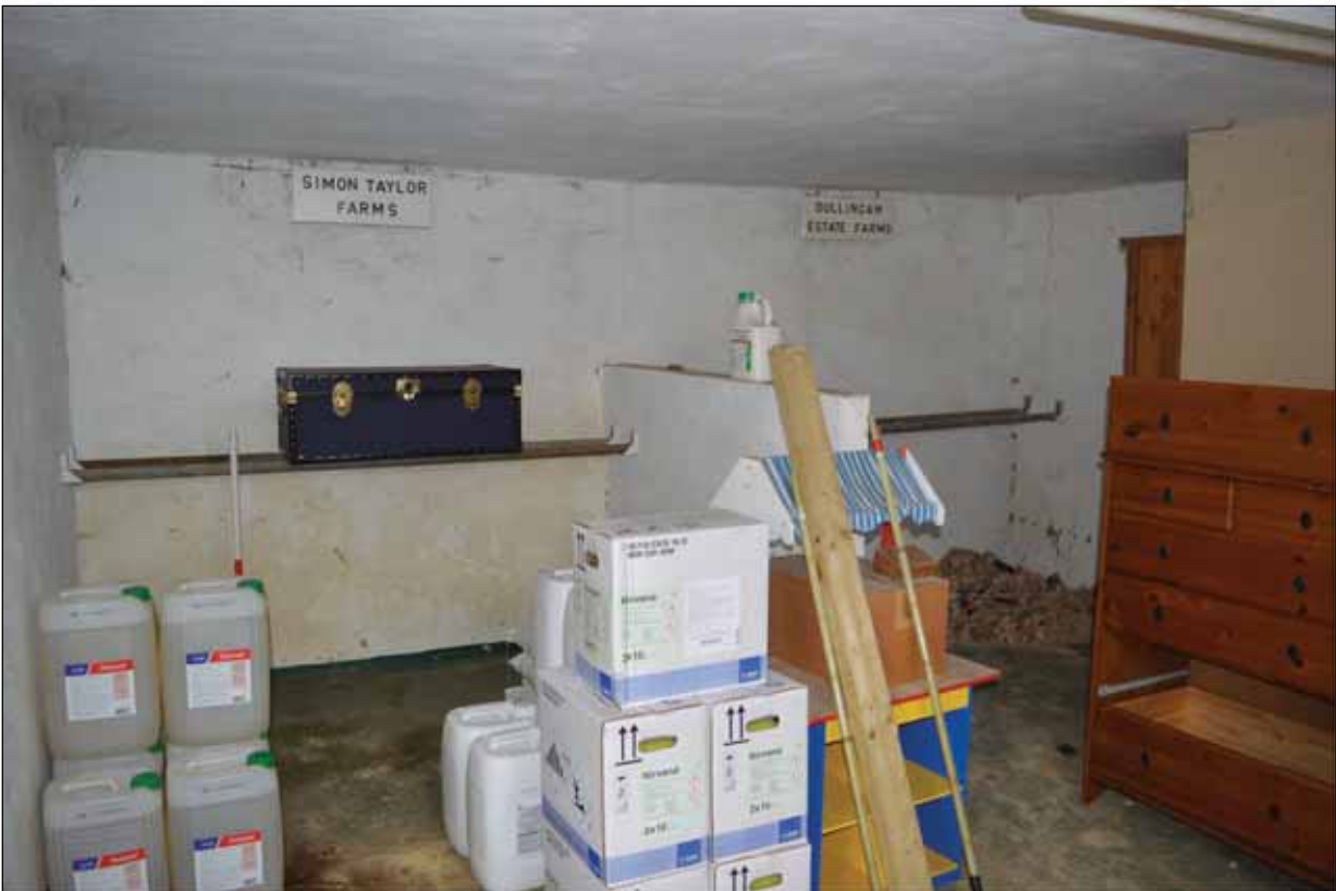
Plate 81: Internal modern stud wall and plaster boarding to Building 6 (rear wall)
