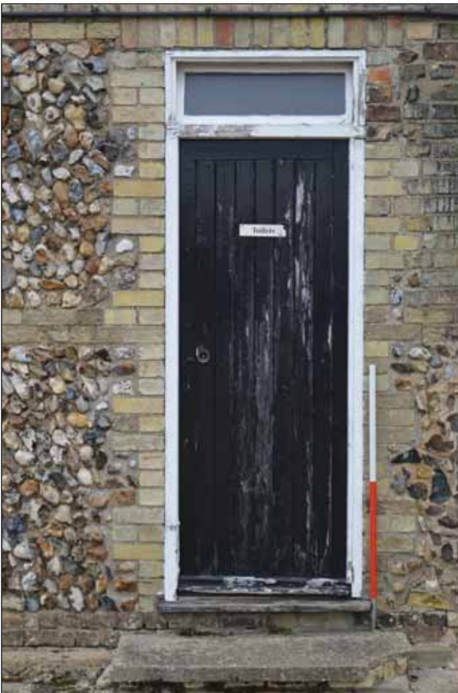
Plate 67: Building 6 - Detail of door to the east end of the building
