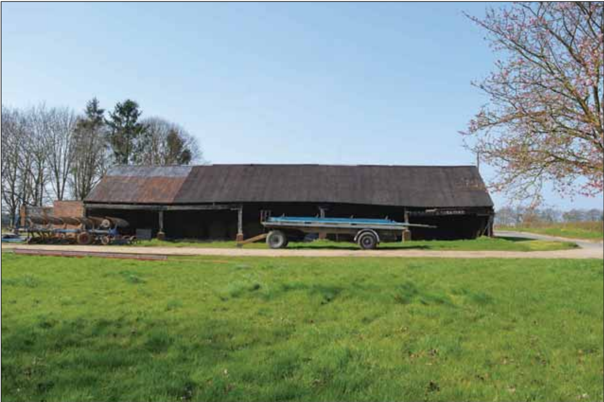
Plate 4: Building 1 viewed from the south-east
