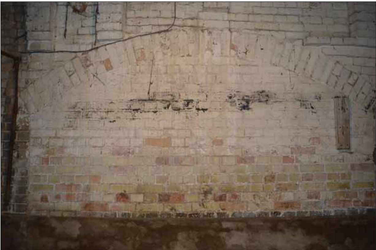
Plate 99: Blocked arch to the south-east wall of Building 6a
