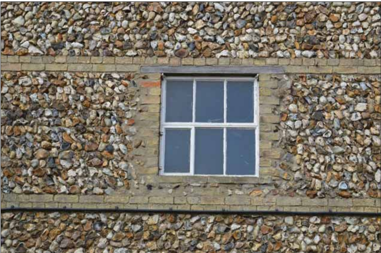
Plate 111: Building 8 - Detail of metal window to the south-east elevation
