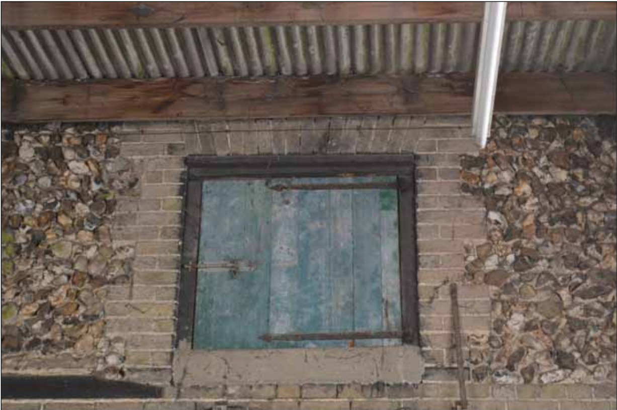
Plate 134: Door located at first floor level to south-west elevation of Building 8
