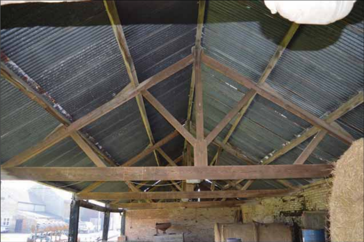
Plate 10: Building 1 - Detail of roof structure viewed from the north-east
