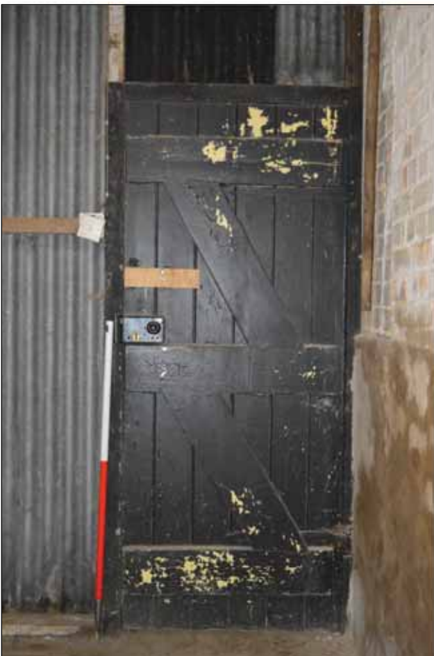
Plate 95: Building 6a - Detail of wooden door viewed from the south-west
