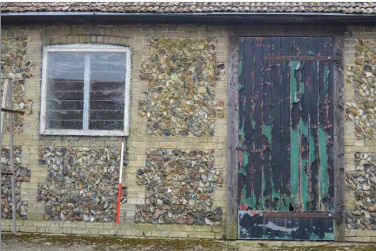
Plate 27: Building 4 - Window and door to the north-east elevation
