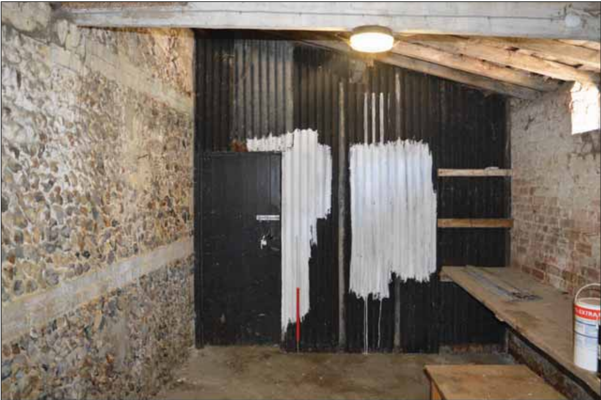
Plate 94: Corrugated wall and wooden door internally to Building 6a
