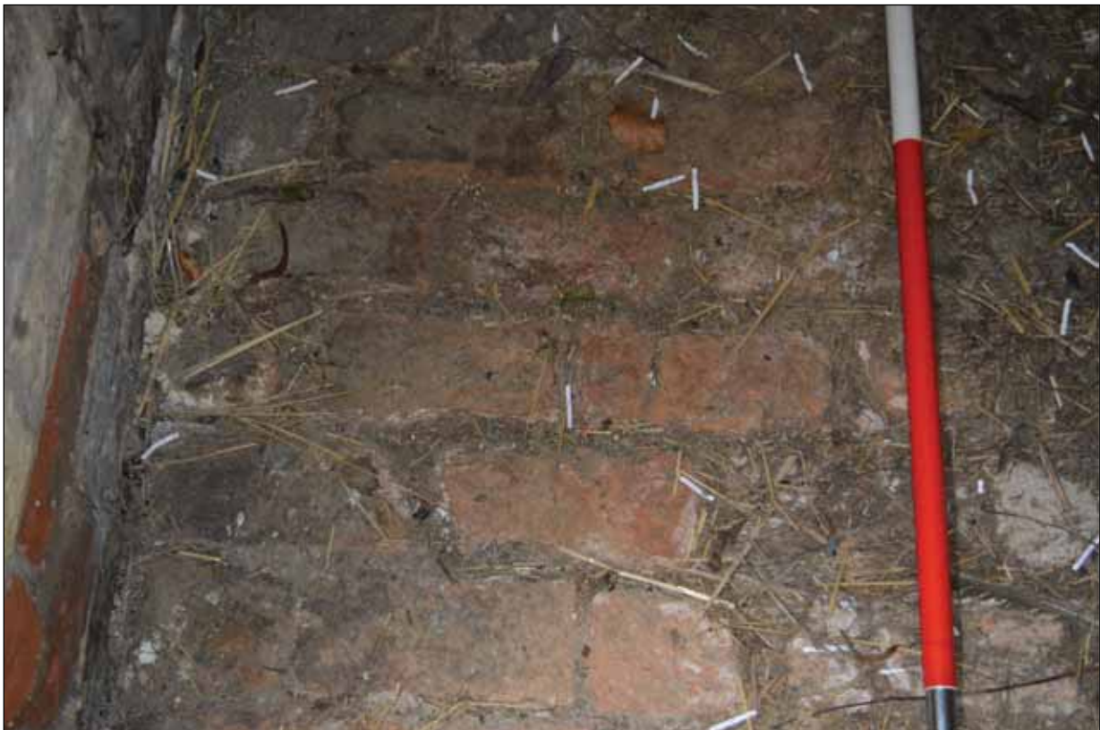
Plate 19: Building 4 - Detail of brick floor within the stable
