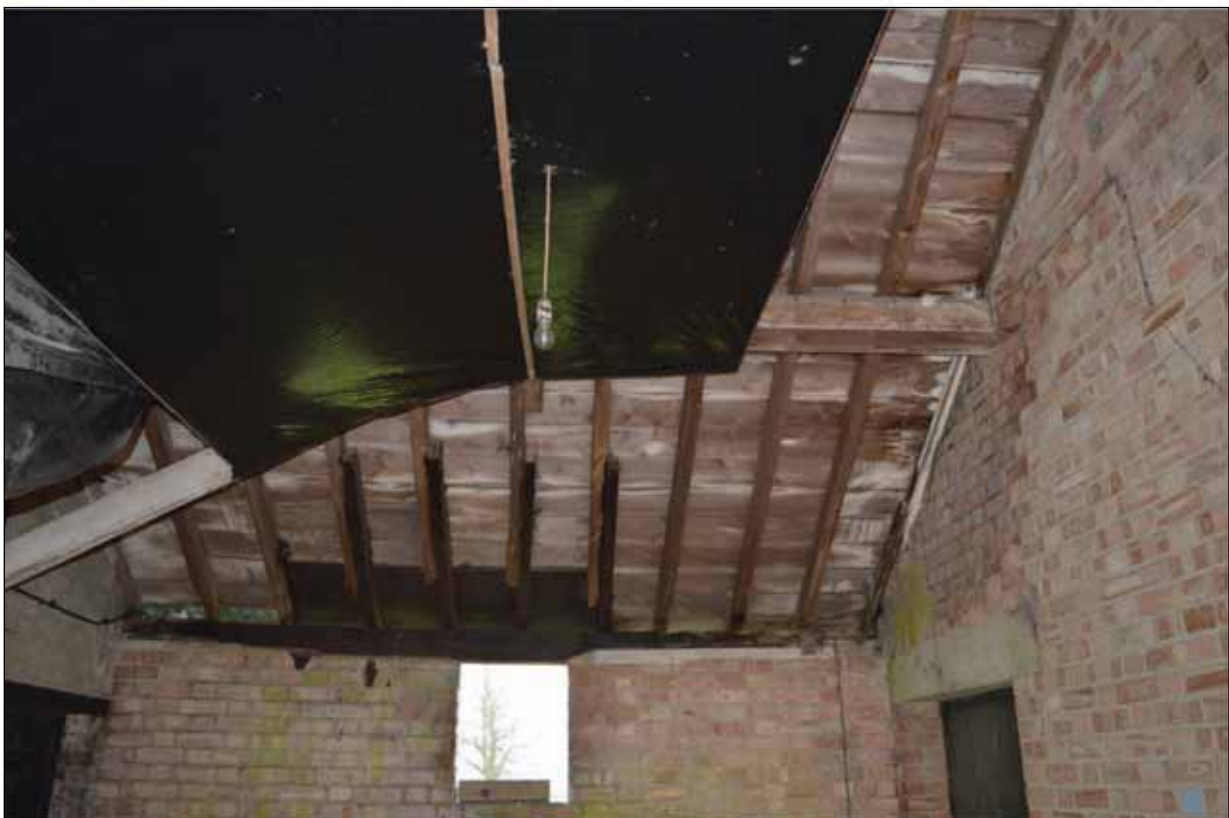
Plate 107: Detail of modern roof structure to Building 7
