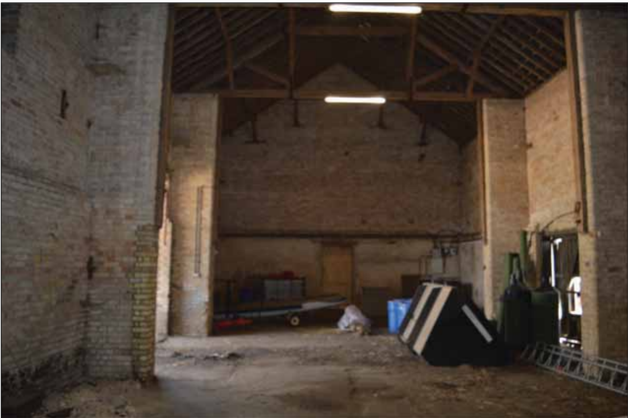
Plate 123: Internal view of the north-east elevation of Building 8
