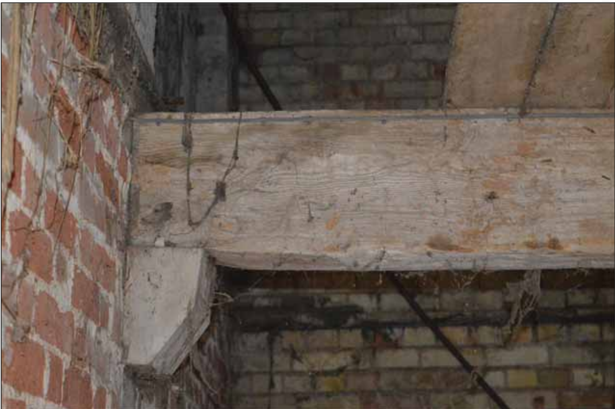
Plate 77: Building 6 - Detail of machine cut beam (room a)
