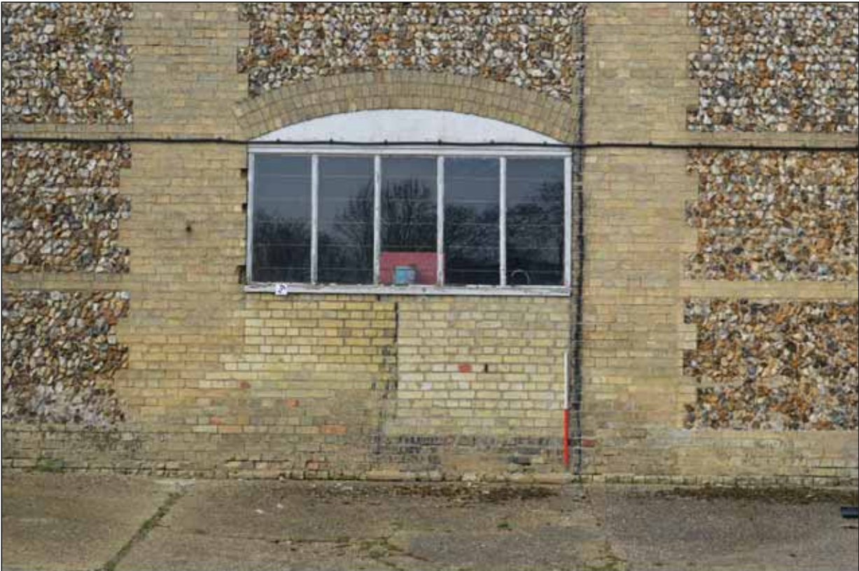
Plate 112: Building 8 - Detail of window in a blocked arch to the south-east elevation
