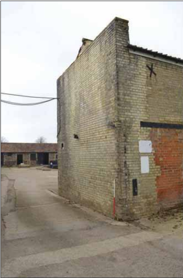
Plate 72: South-east facing wall at the end of Building 6 viewed from the north-east
