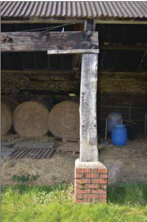
Plate 11: Building 1 - Brick pier with re-used upright viewed from the south-east
