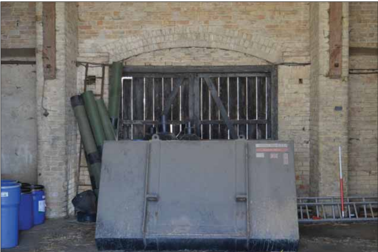
Plate 117: Building 8 - Internal view of double doors to south-east elevation
