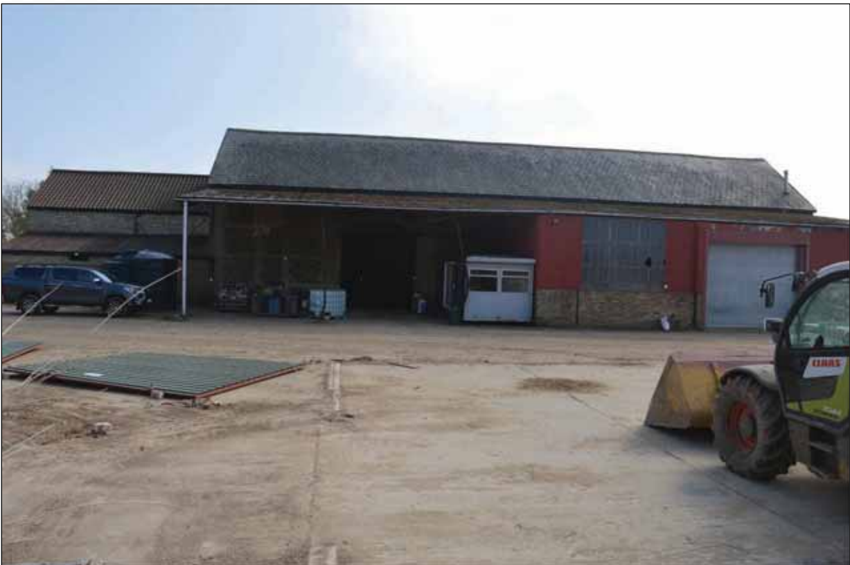
Plate 135: Building 10 - Modern lean to attached to the north-west elevation of Building 8
