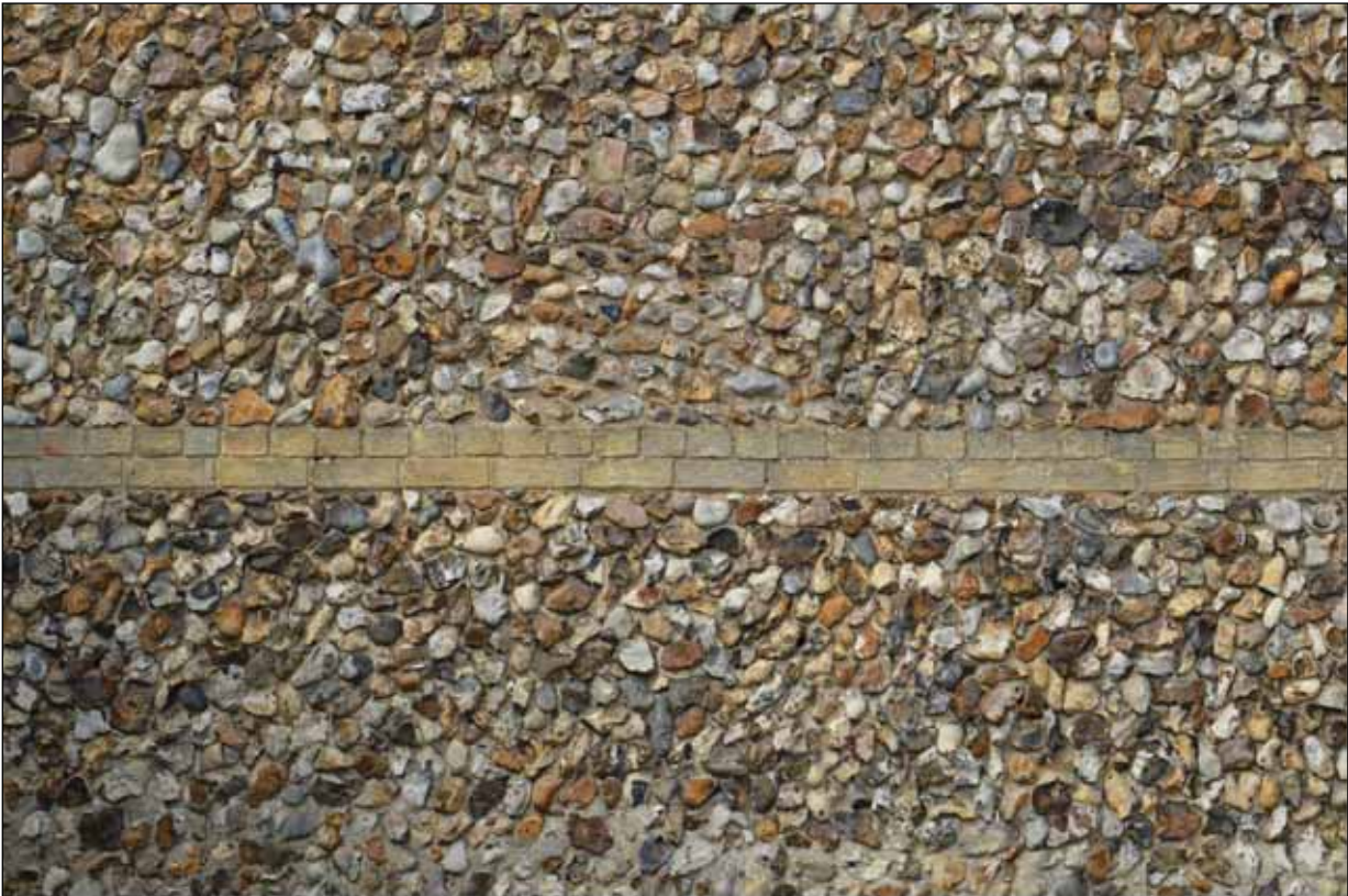
Plate 110: Detail of flint work and brick lacing bands to Building 8
