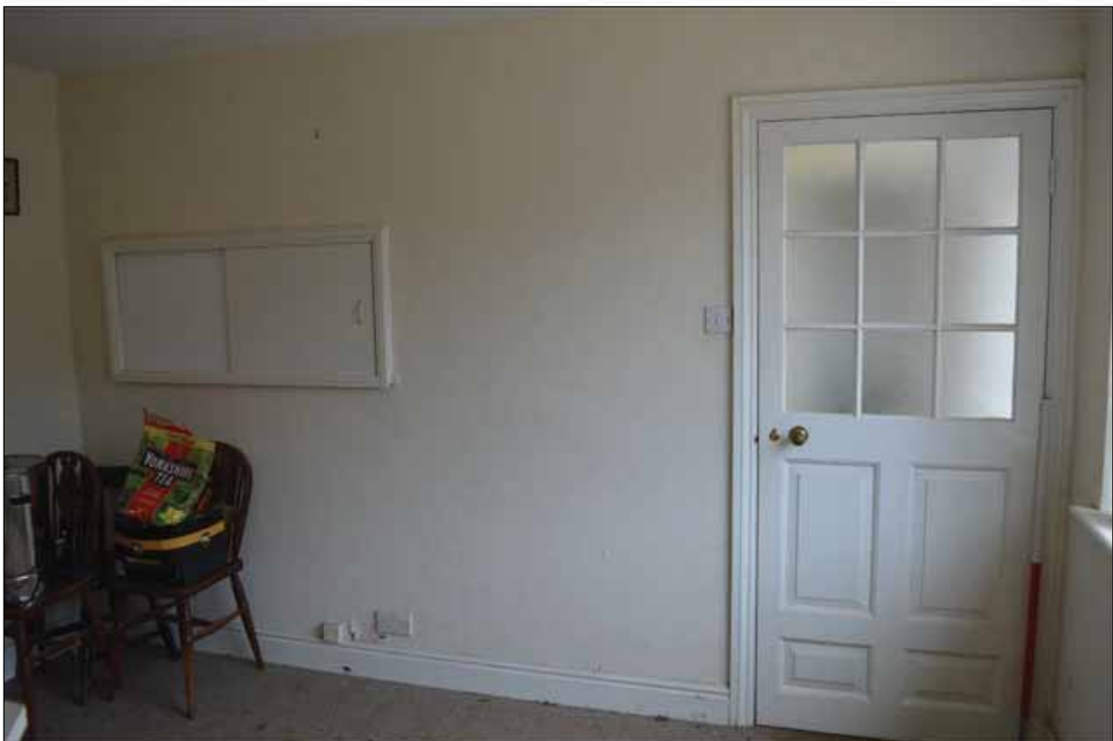
Plate 49: Building 5 - South-western stud wall of office showing door and hatch (room 2)
