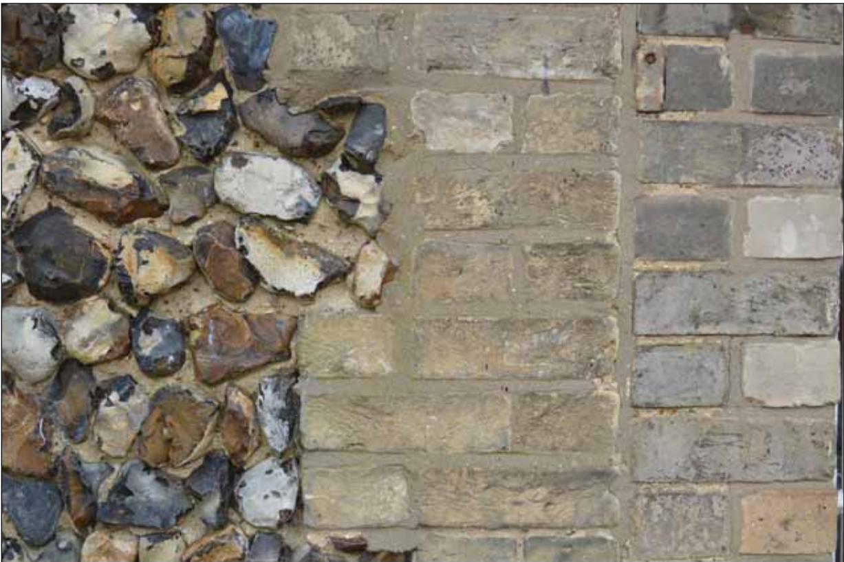
Plate 42: Building 5 - Detail of brick and flint work
