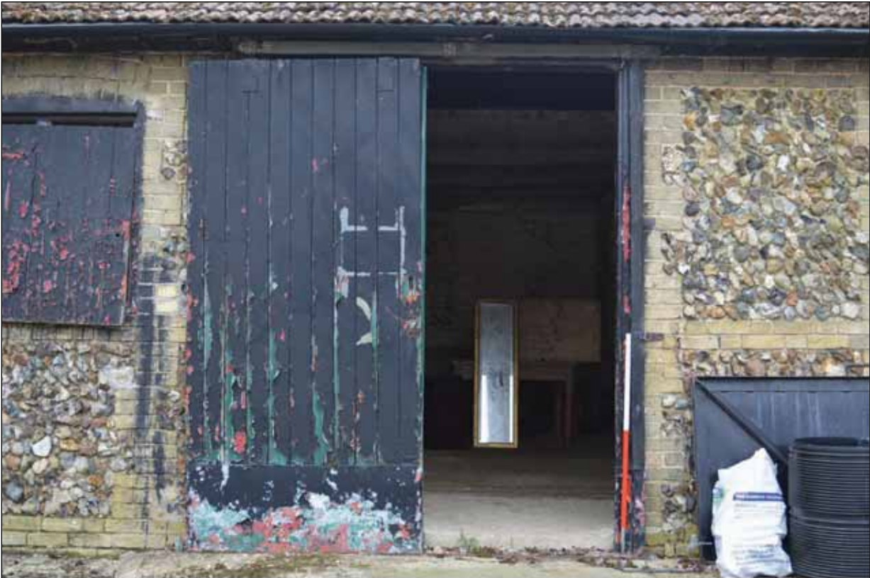
Plate 24: Building 4 - Double wooden doors located on the north-east elevation
