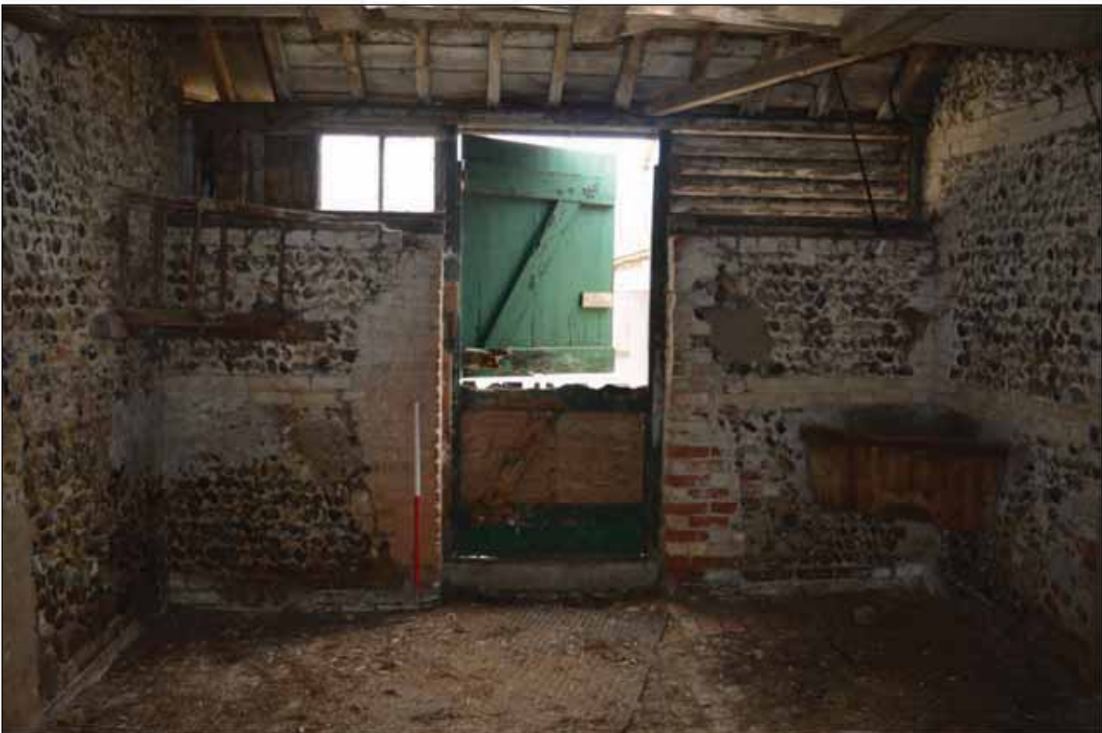
Plate 15: Building 4 - Internal view of stable door to the eastern end of the range
