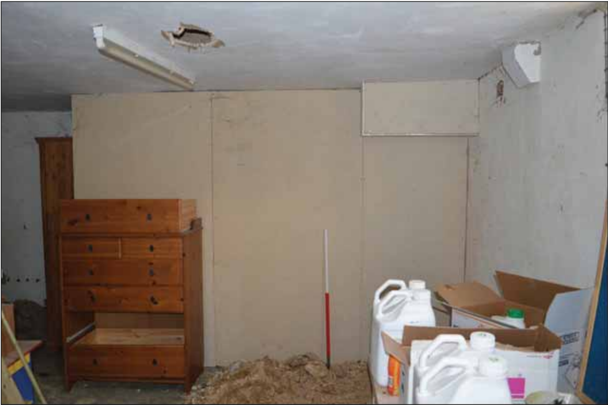
Plate 80: Internal modern stud wall and plaster boarding to Building 6 (room a)
