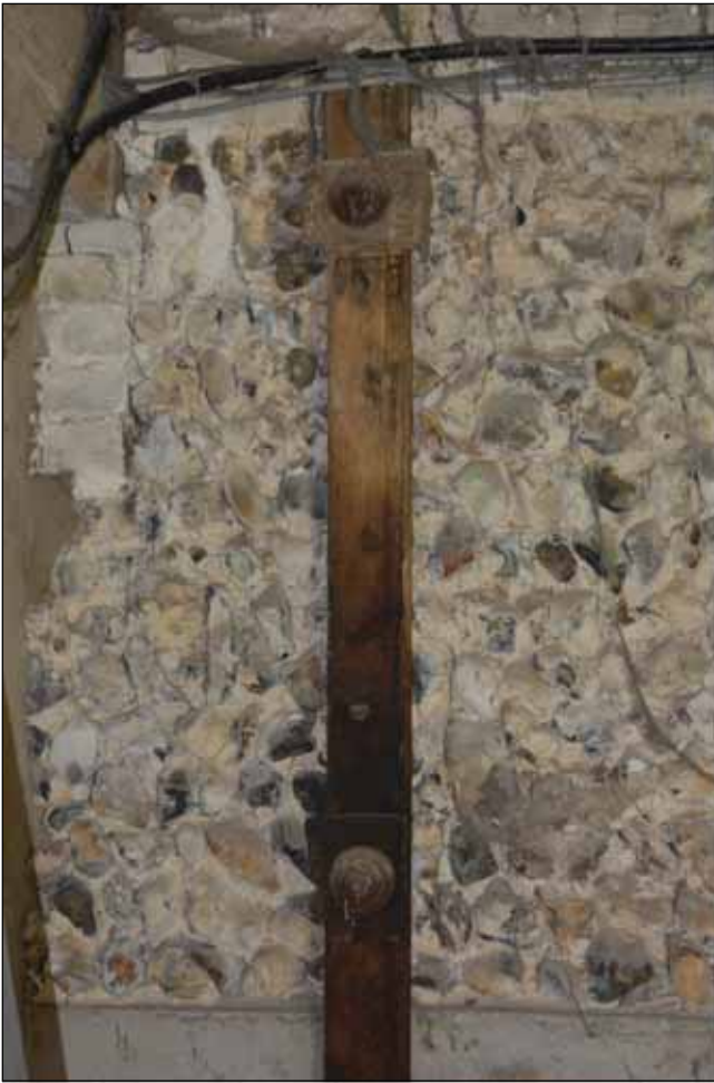
Plate 78: Building 6 - Detail of brace to rear wall (room a)
