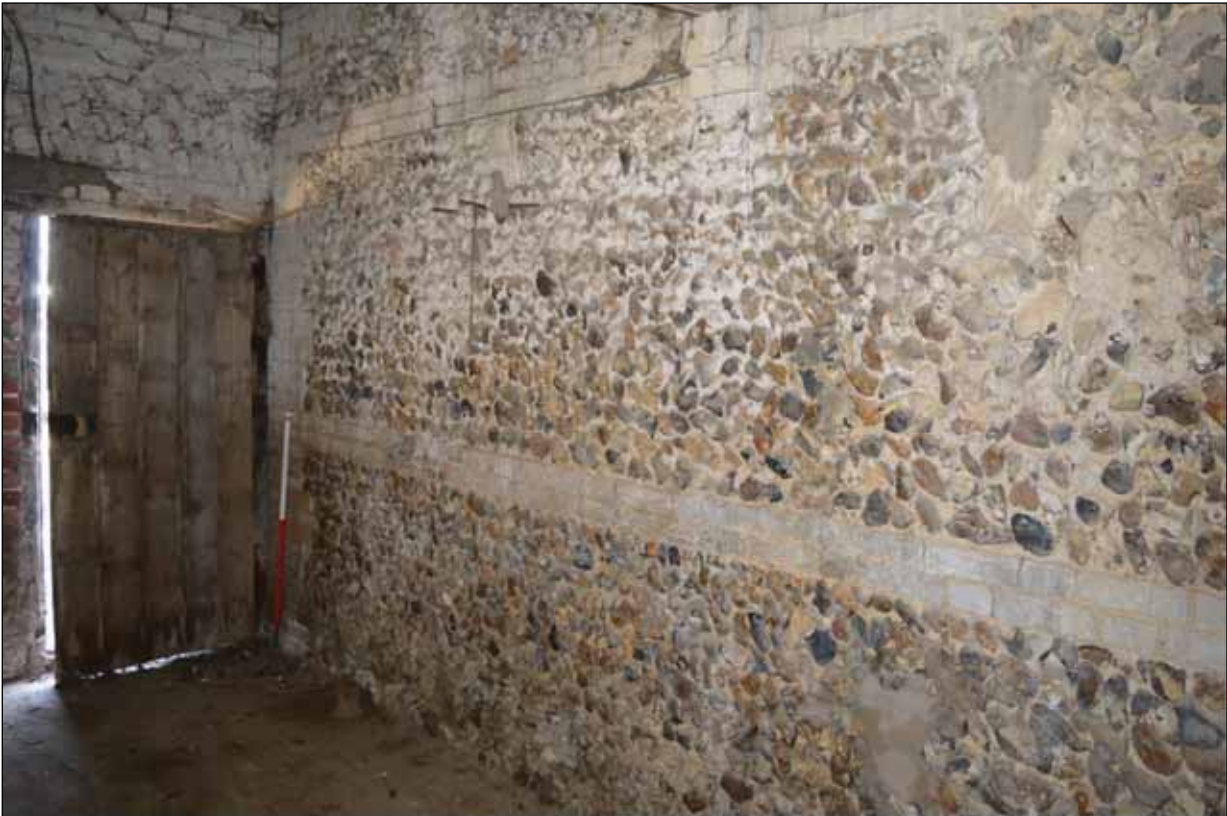
Plate 92: External wall of Building 6 viewed internally from Building 6a
