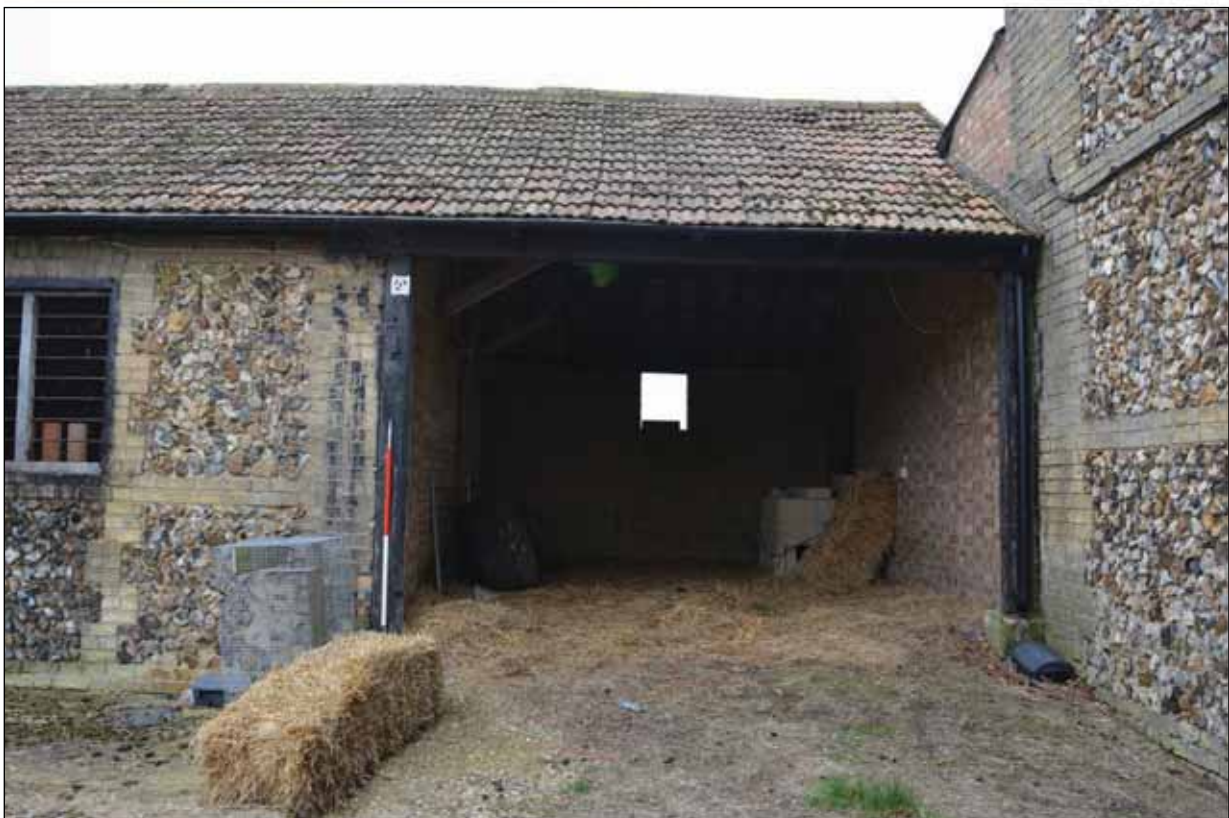
Plate 101: Courtyard view of Building 7 viewed from the north-east
