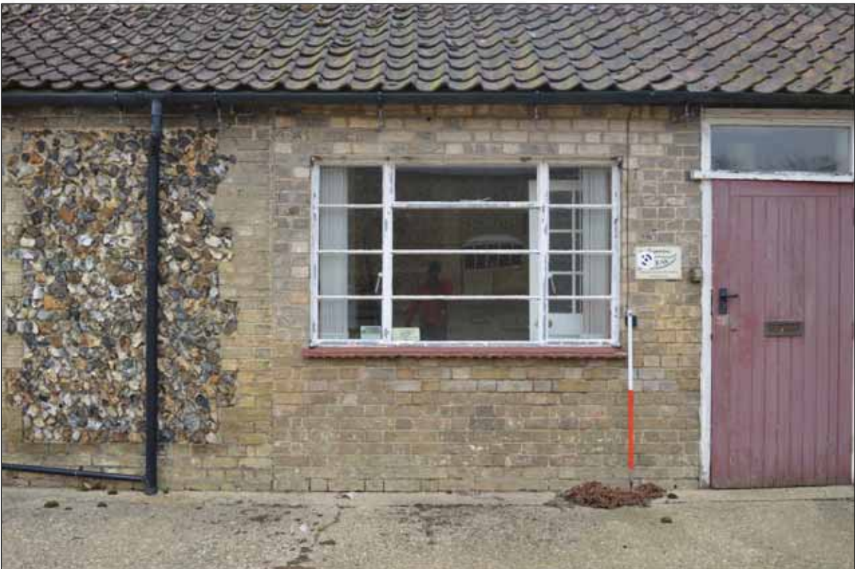
Plate 43: Building 5 - Crittal style metal window to the courtyard viewed from the north-west
