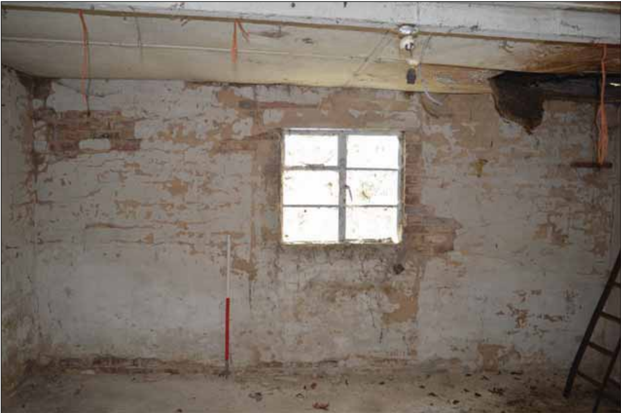
Plate 142: Building 11 - Metal window and south-west facing wall viewed internally
