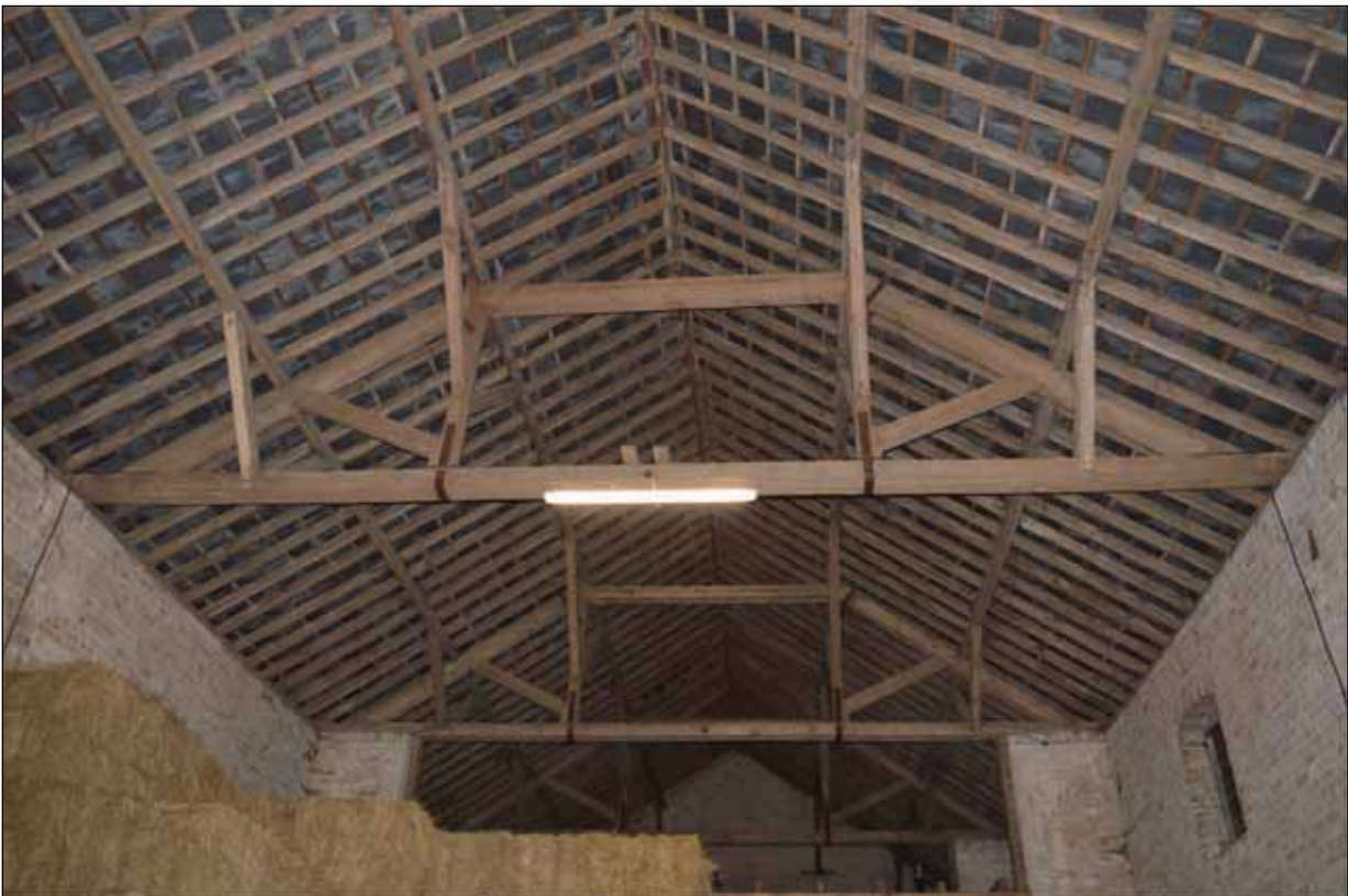
Plate 127: Building 8 - Detail of trusses resting on brick piers
