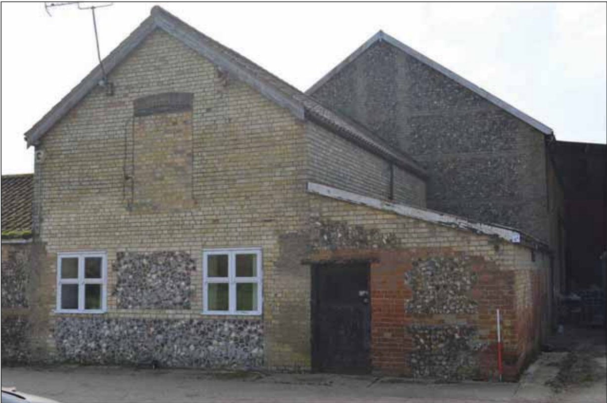
Plate 85: Building 6a viewed from the north-east
