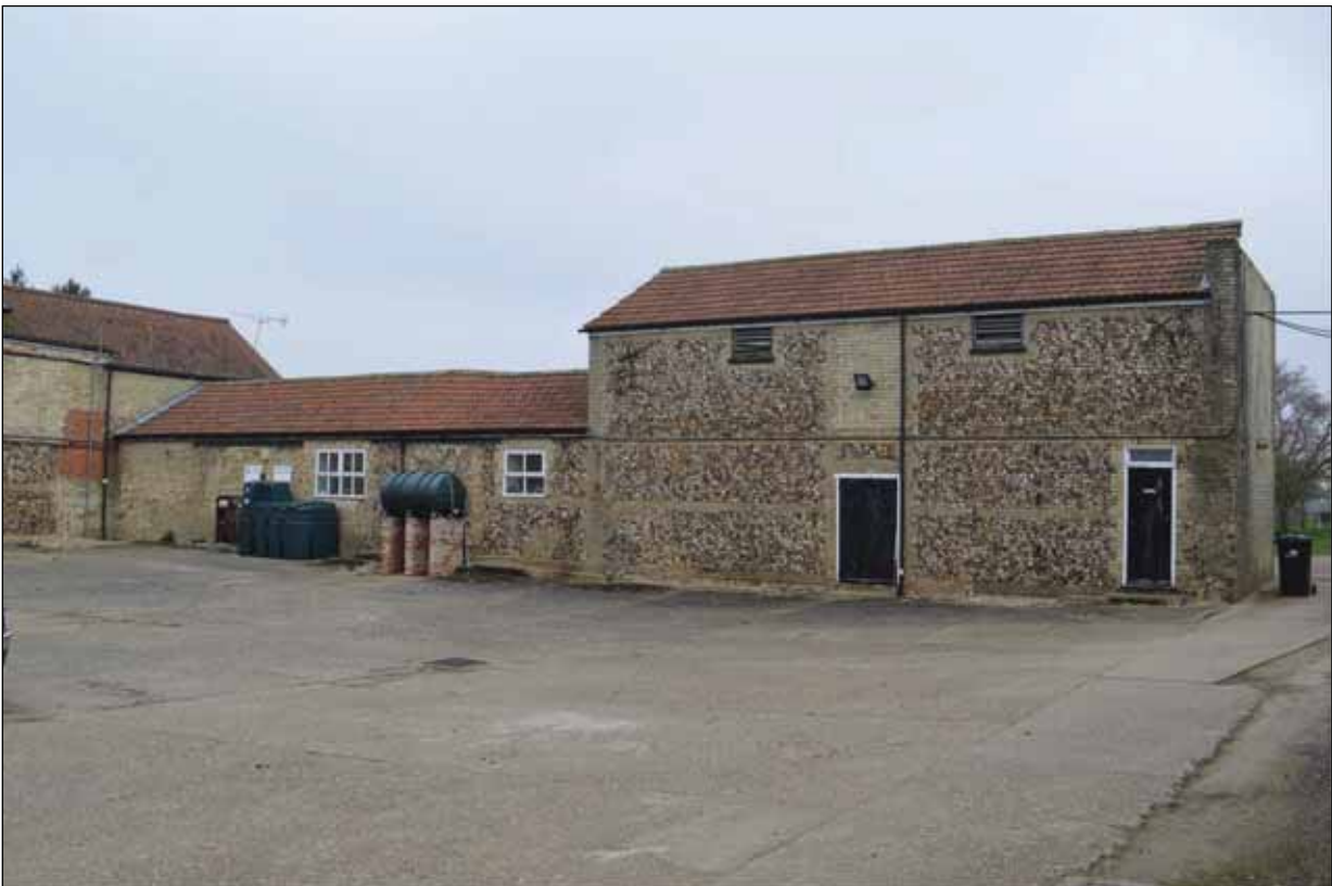
Plate 63: Building 6 - Courtyard view of building viewed from the south-west
