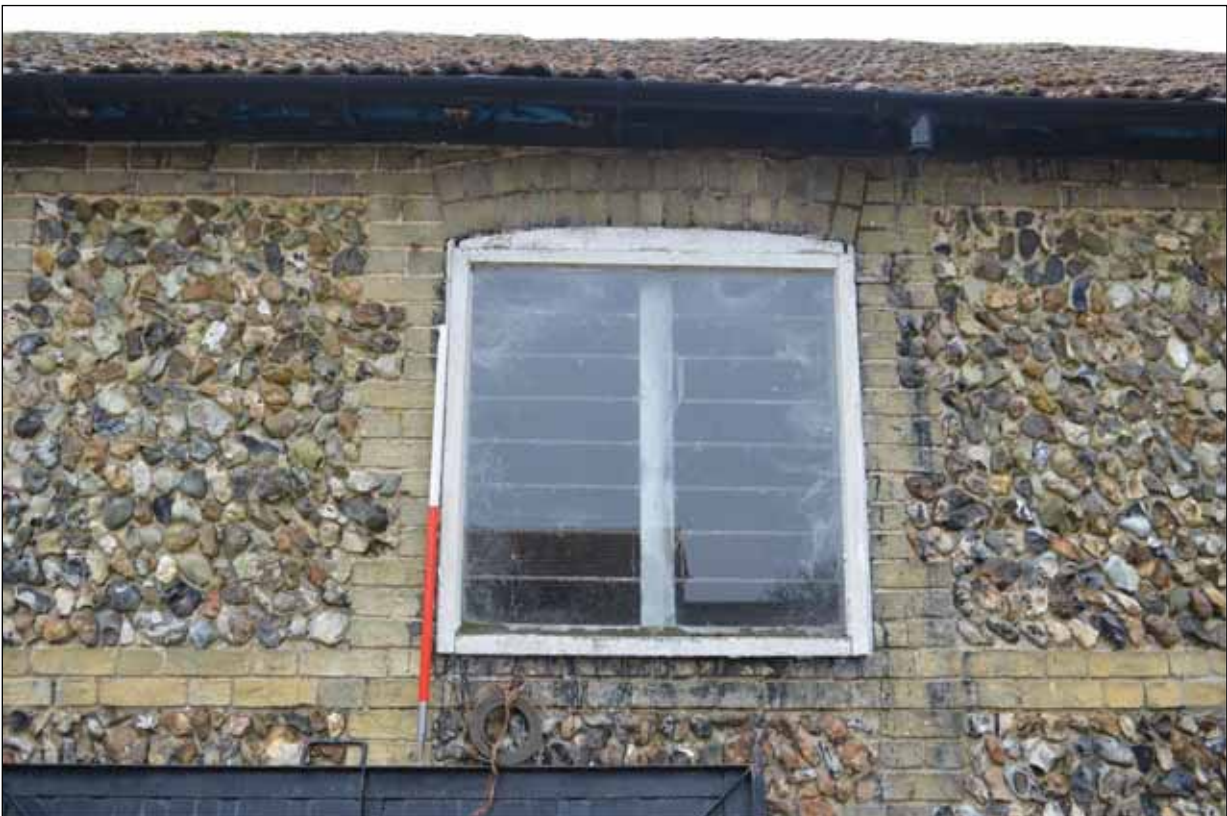
Plate 29: Building 4 - Wooden casement to the north-east elevation
