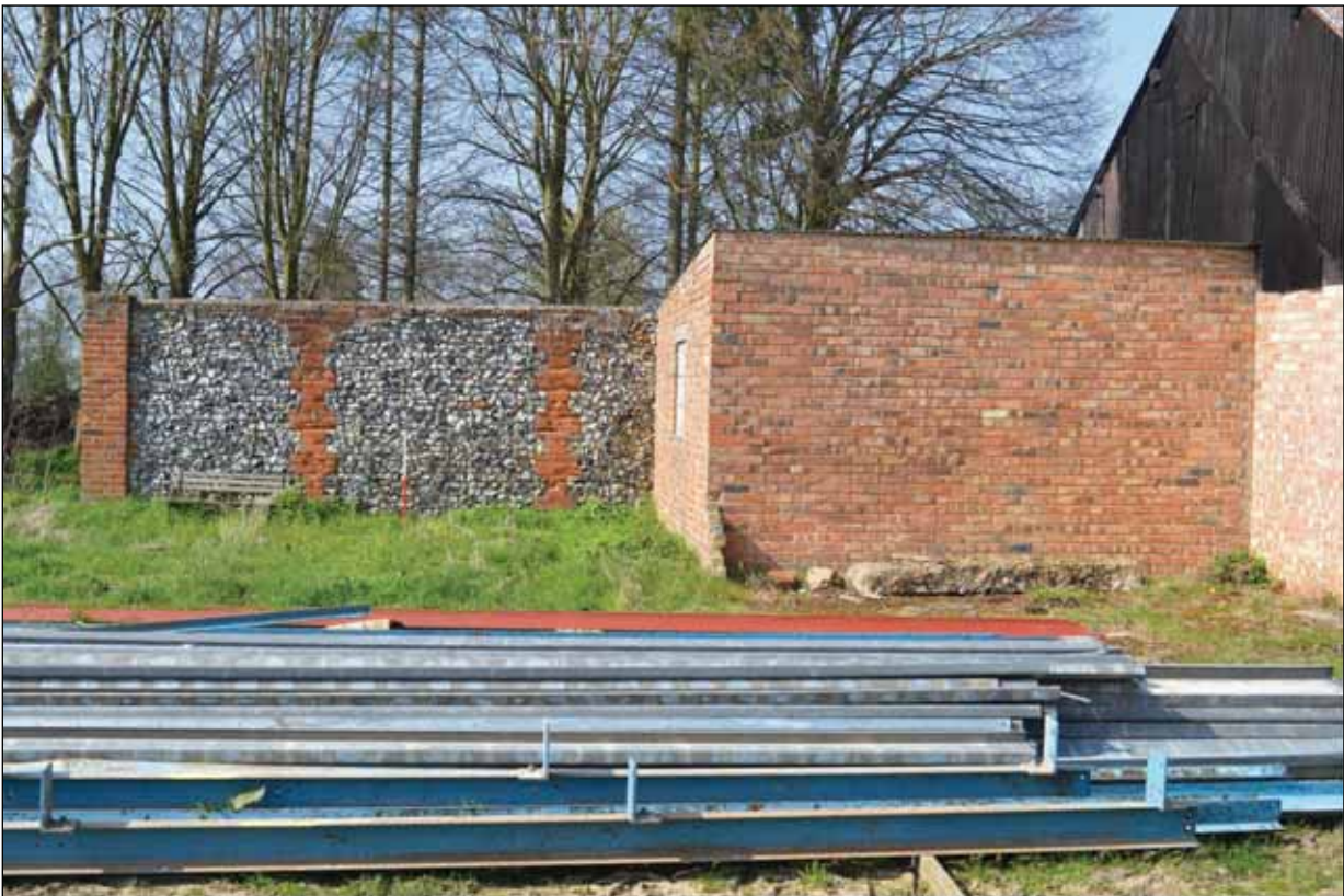
Plate 136: Building 11 and perimeter wall viewed from the south east
