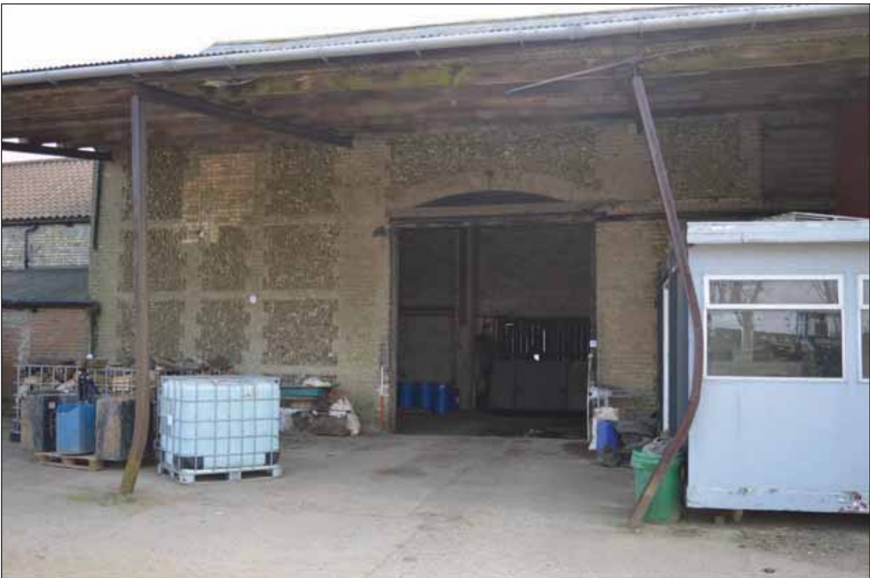
Plate 115: Building 8 - Double doorway to north-west elevation
