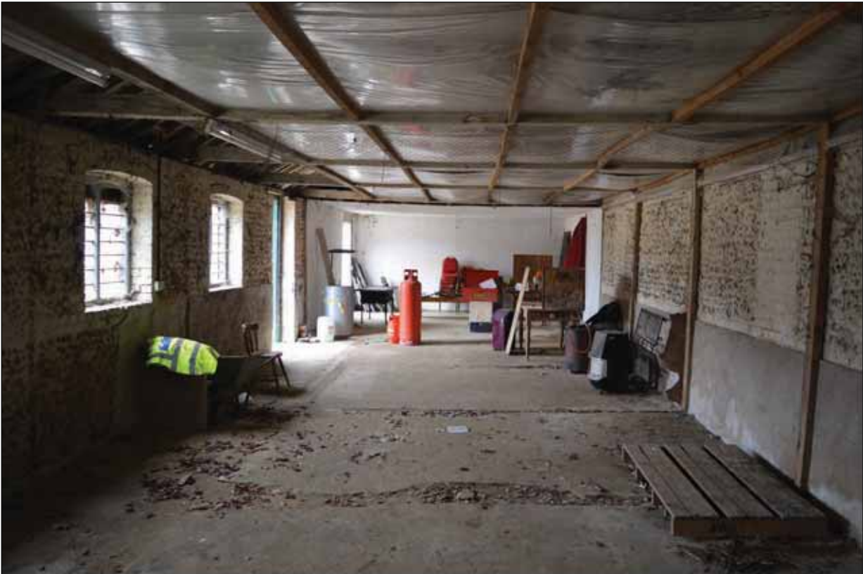
Plate 32: Building 4 - Internal view of the eastern end of the building
