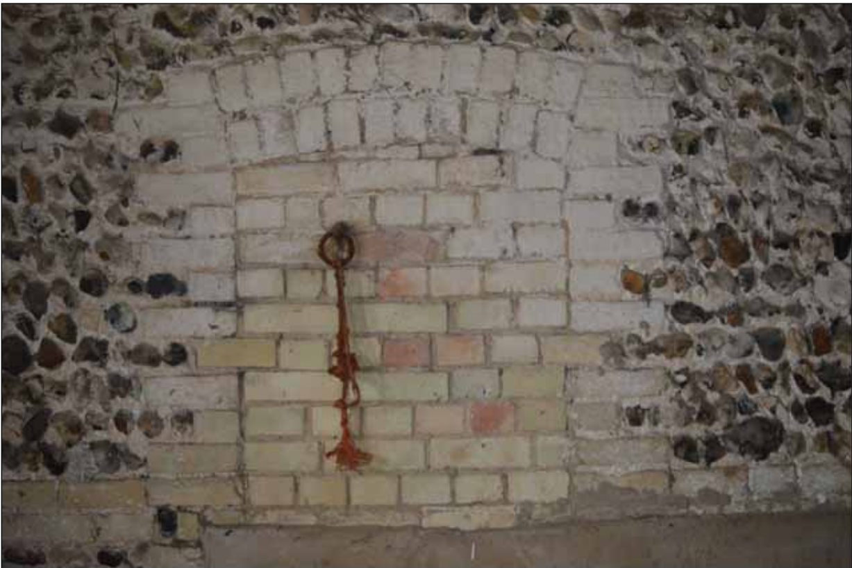
Plate 38: Building 4 - Detail of blocked window located to the rear wall of the building
