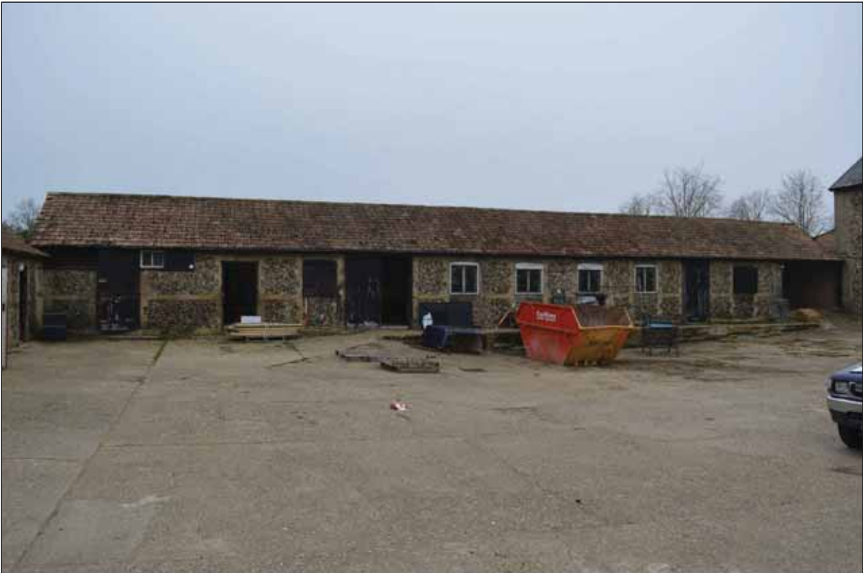
Plate 14: Courtyard aspect of Building 4 viewed from the north-east
