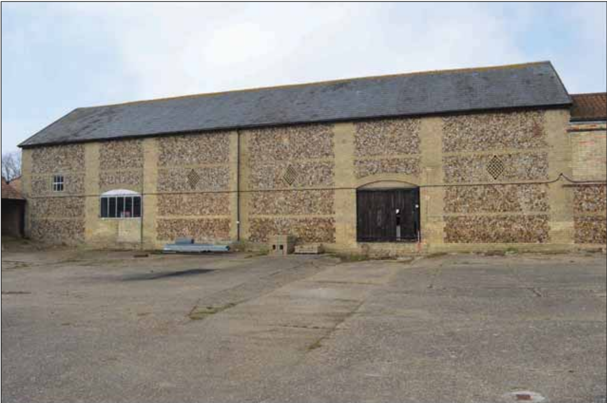
Plate 108: Courtyard view of Building 8 viewed from the north-east
