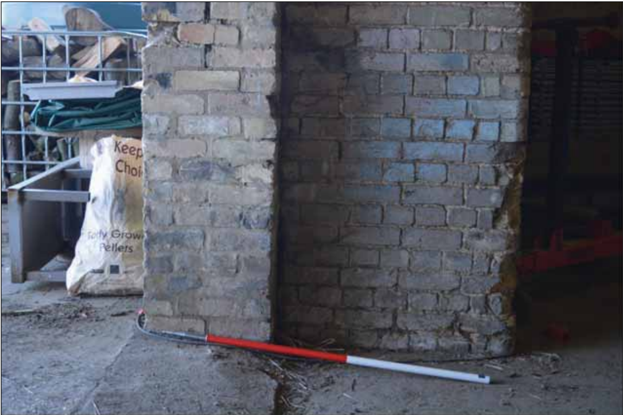
Plate 120: Building 8 - Detail of brickwork
