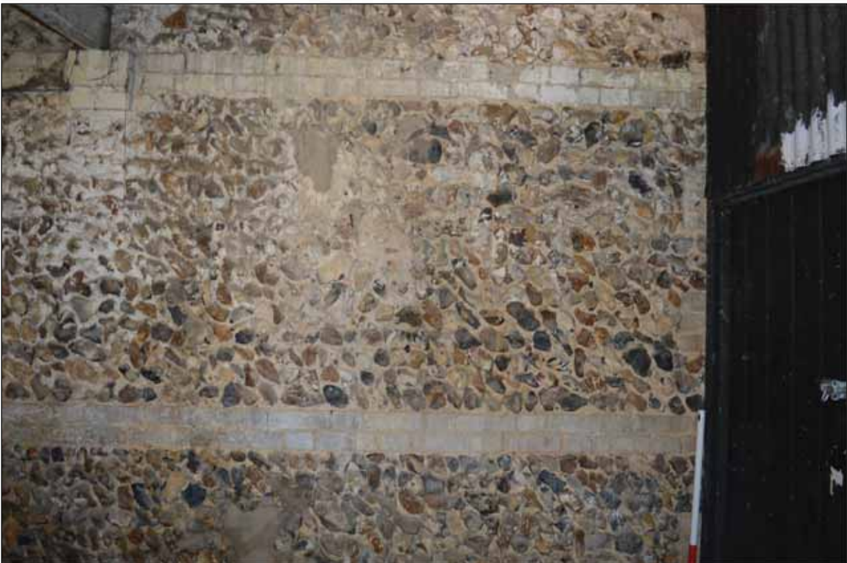
Plate 93: Detail of flint with brick lacing to the external wall of Building 6a
