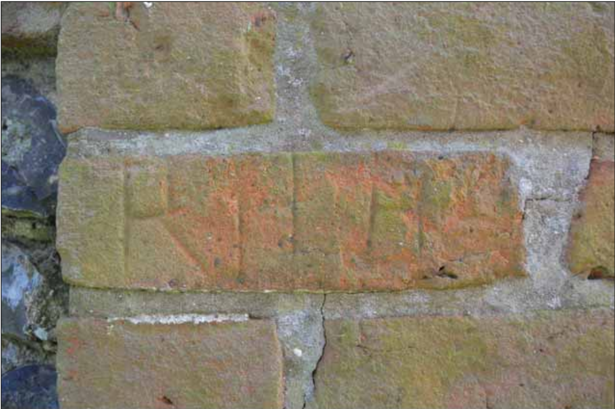
Plate 138: Detail of graffiti on the north west facing elevation of Building 11
