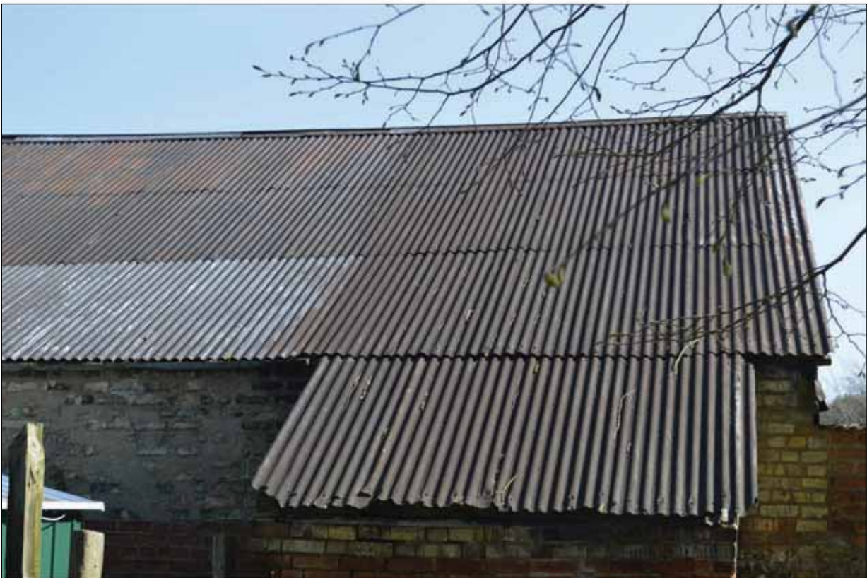
Plate 7: Building 1 - Corrugated iron roof viewed from the west
