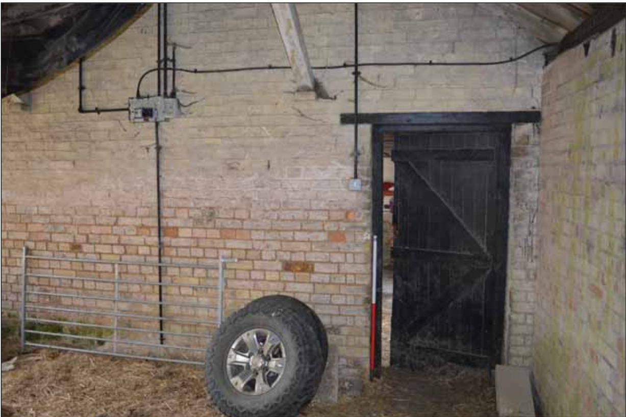
Plate 103: Door to Building 4 from Building 7 viewed from the north-west
