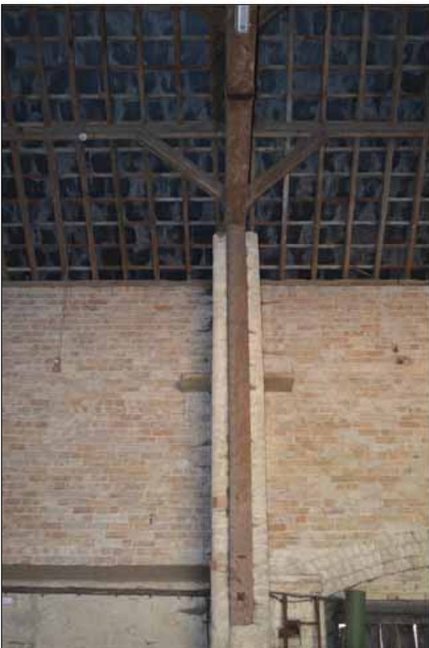
Plate 121: Building 8 - Detail of brick pier and roof structure to south-east elevation
