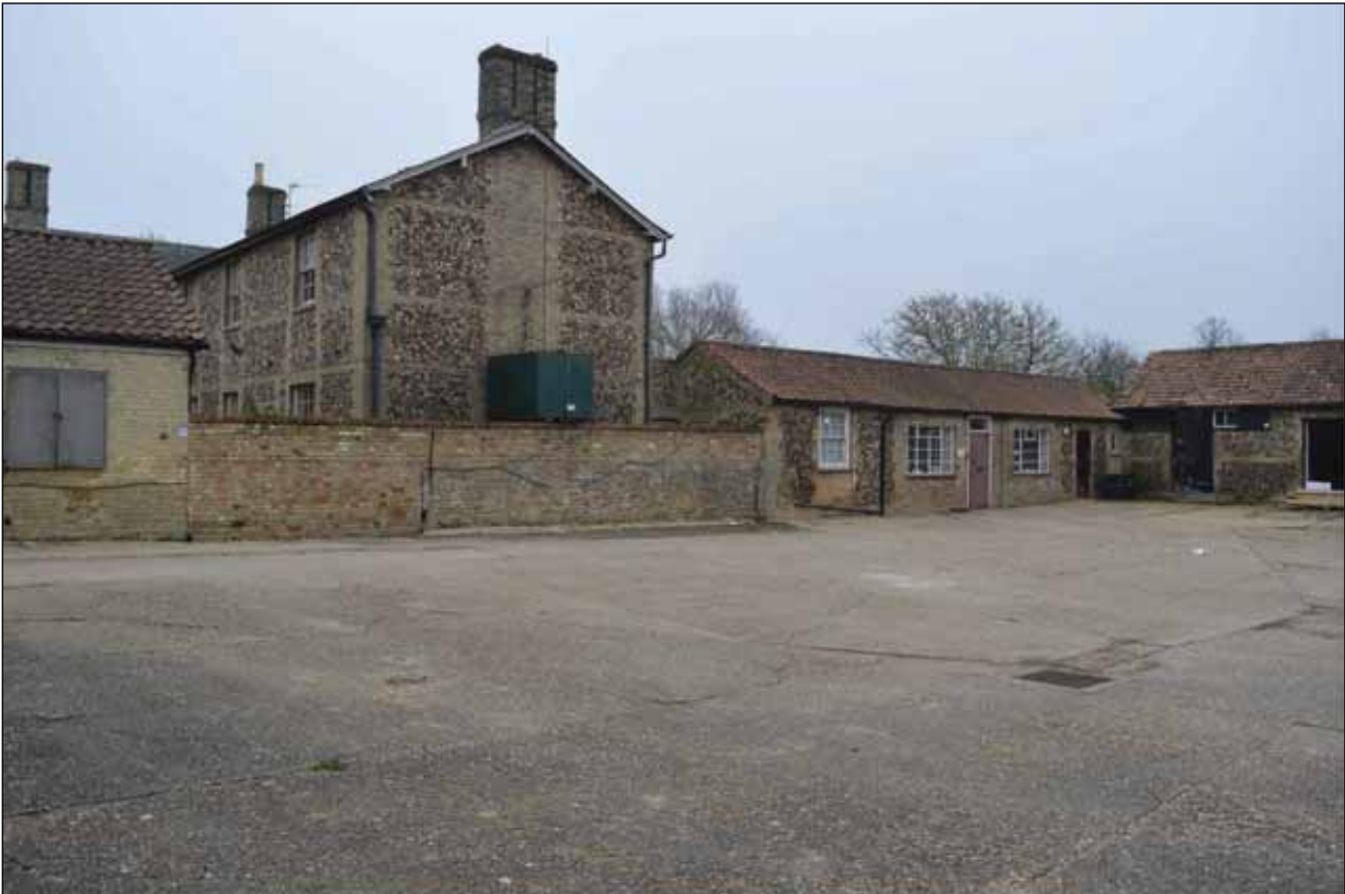
Plate 40: Building 5 - Building in relationship with the former farm house viewed from the courtyard
