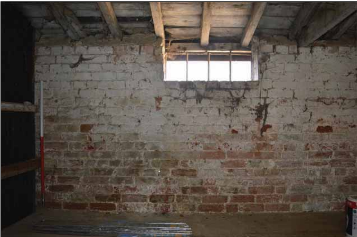
Plate 91: Building 6a - Internal view of window and brick wall to north-west elevation
