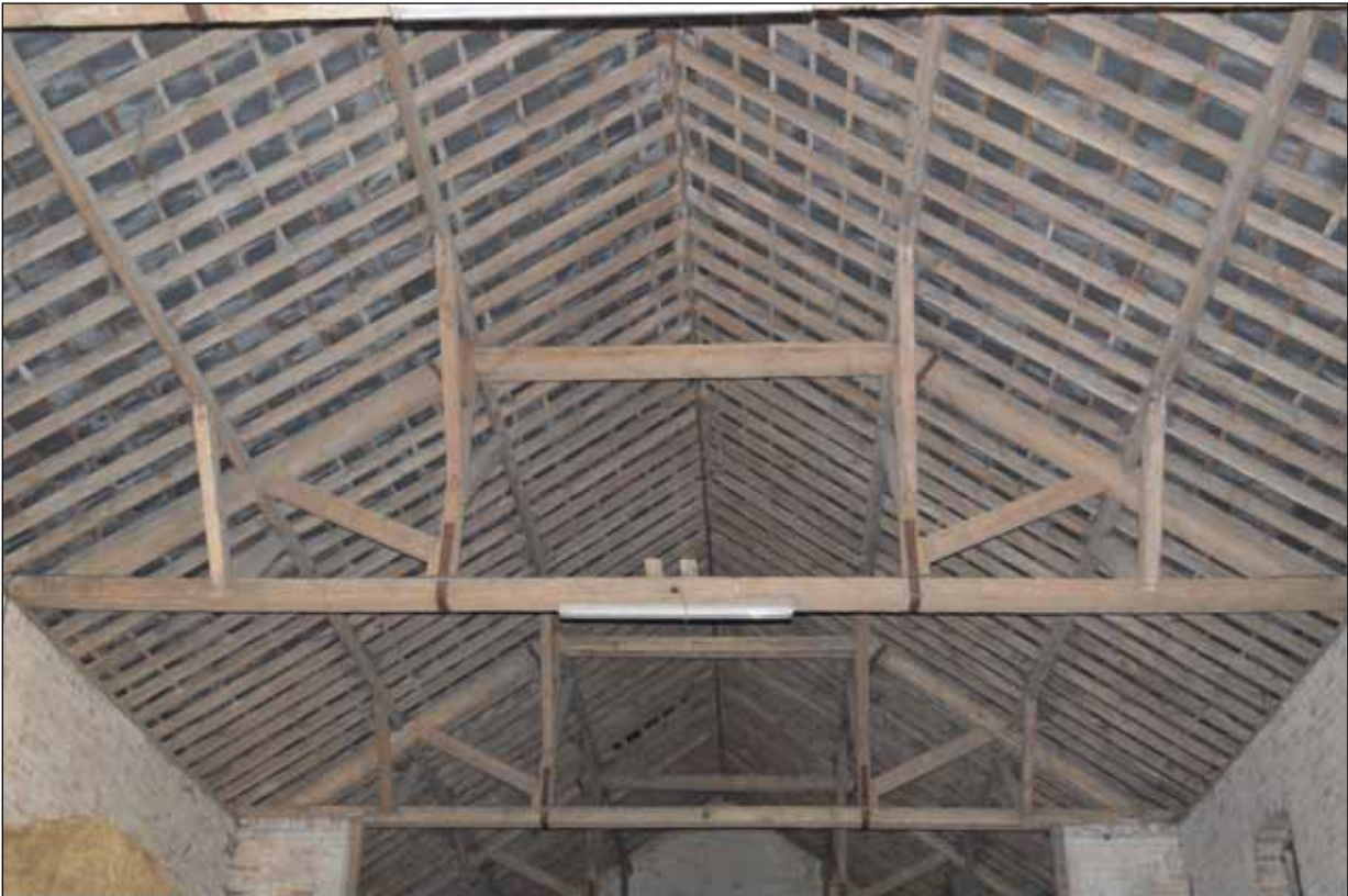
Plate 126: Detail of trusses and roof structure to Building 8 viewed internally
