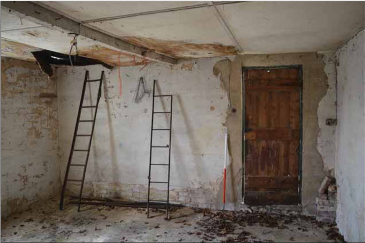
Plate 140: Door to the north west wall of Building 11 viewed internally
