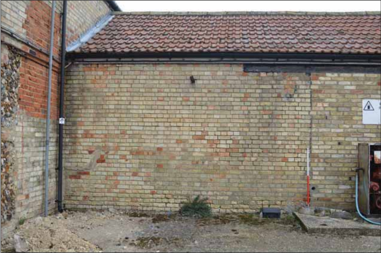
Plate 70: Building 6 - Detail of in-filling
