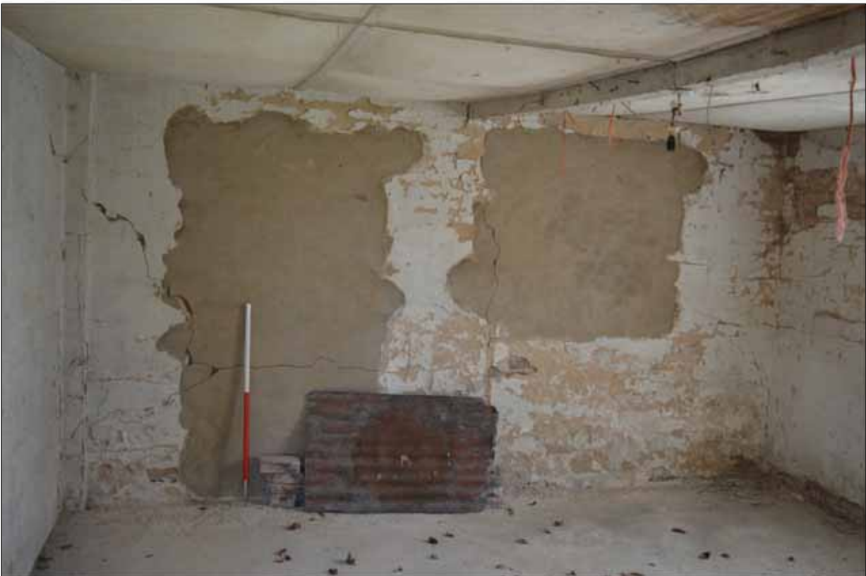
Plate 139: Building 11 - Blocked window and doorway on south-east wall viewed internally
