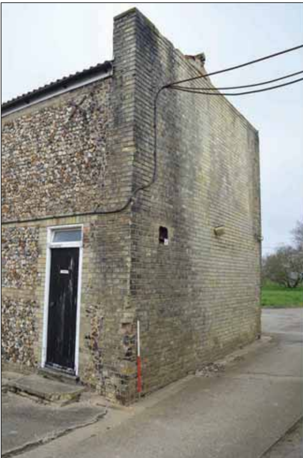
Plate 71: South-east facing wall at the end of Building 6 viewed from the south
