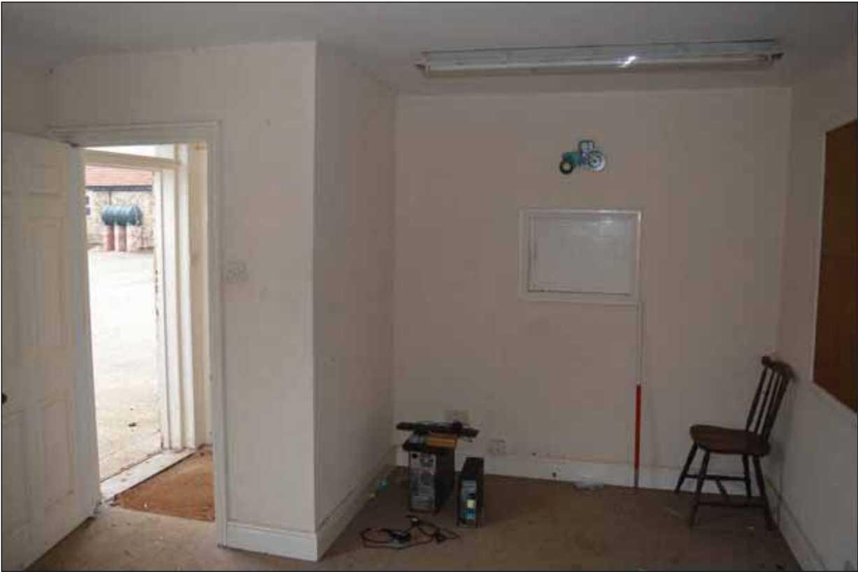
Plate 54: Building 5 - Foyer and wall of office
