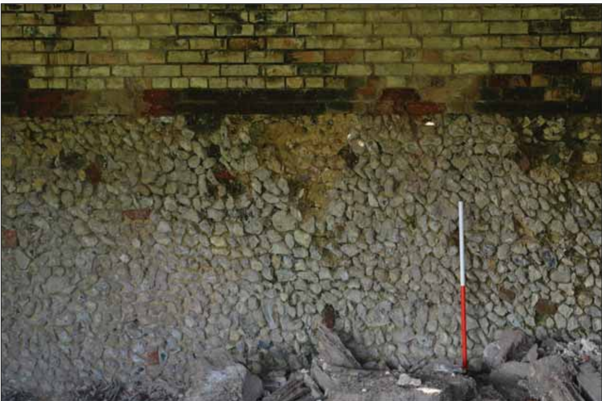
Plate 13: Building 1 - Detail of rear wall
