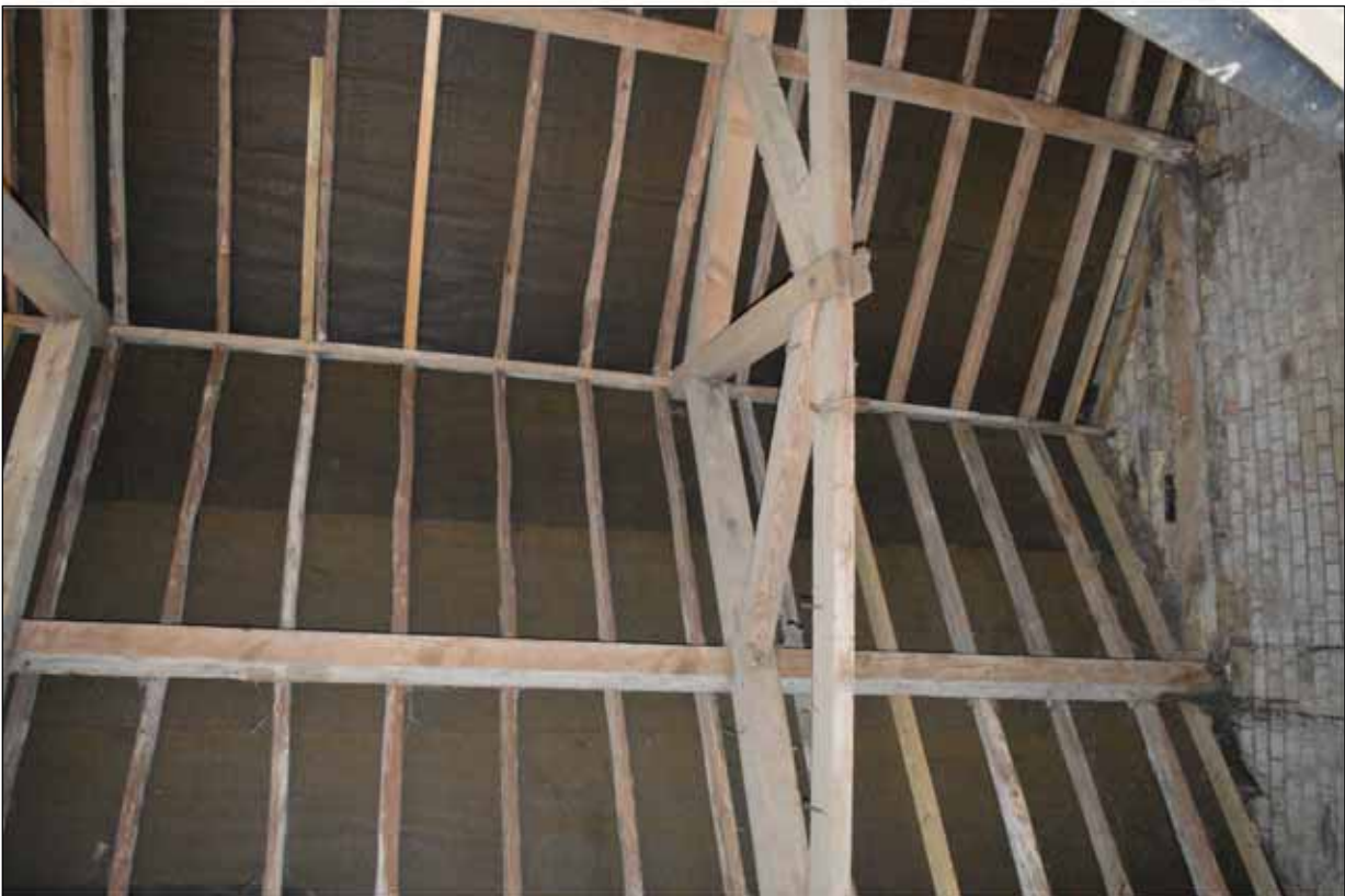
Plate 79: Modern re-roofing to Building 6
