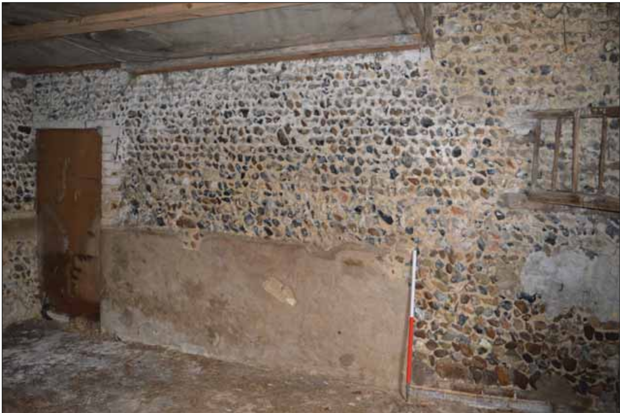
Plate 18: Building 4 - Internal view of the western wall
