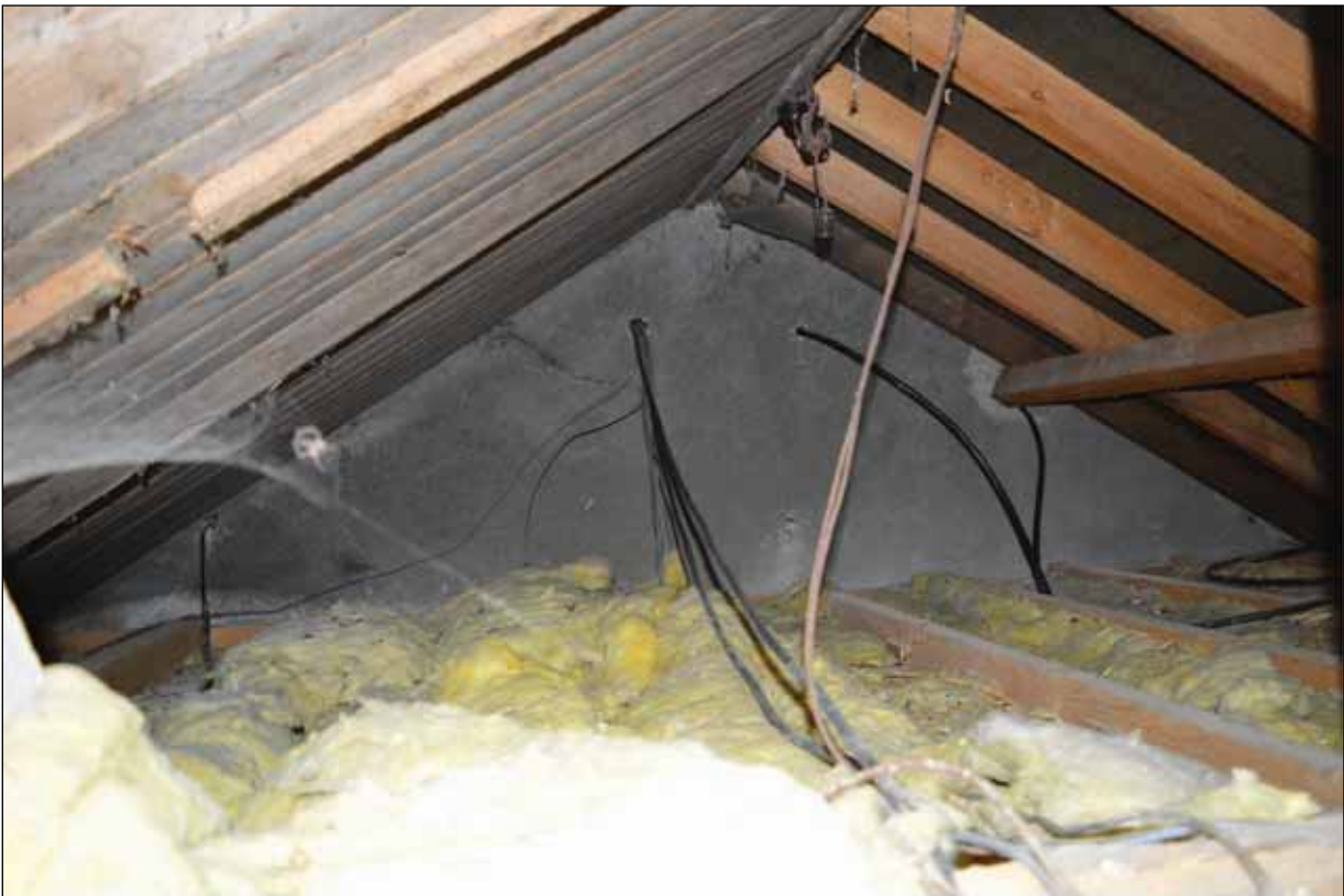
Plate 58: Building 5 - Detail of modern roof
