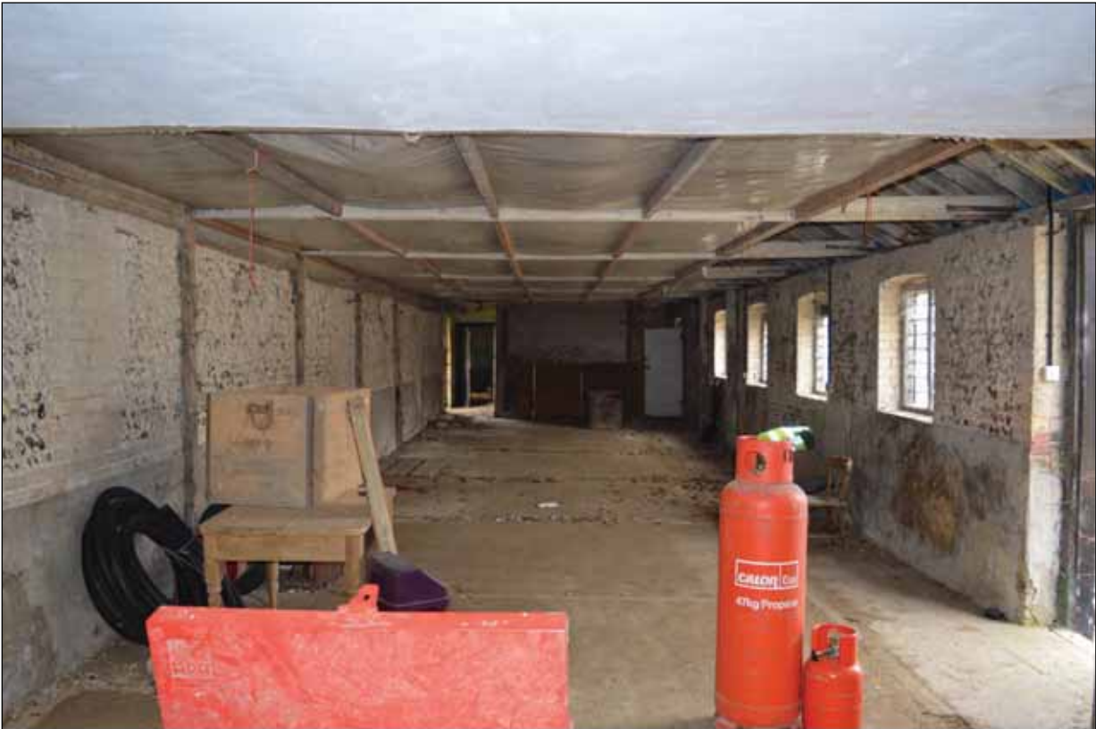
Plate 30: Building 4 - Internal view of the western end of the building
