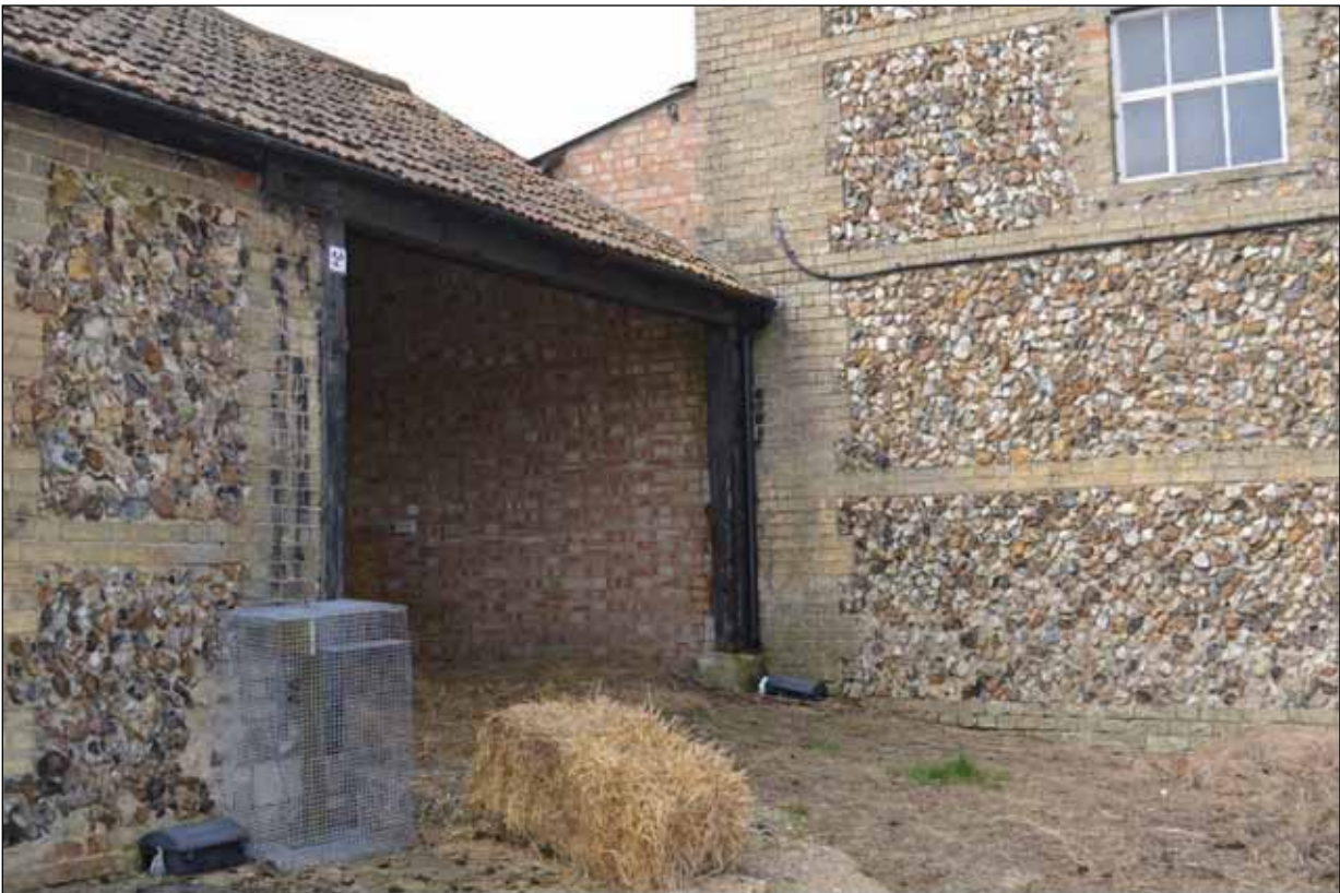
Plate 102: Building 7 adjoining Building 8 viewed from the north-east
