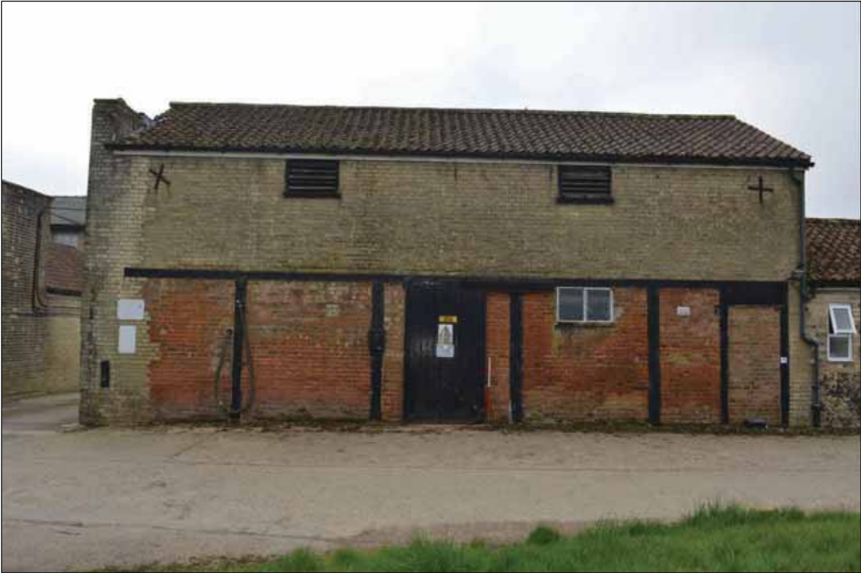
Plate 74: North-east facing elevation of Building 6
