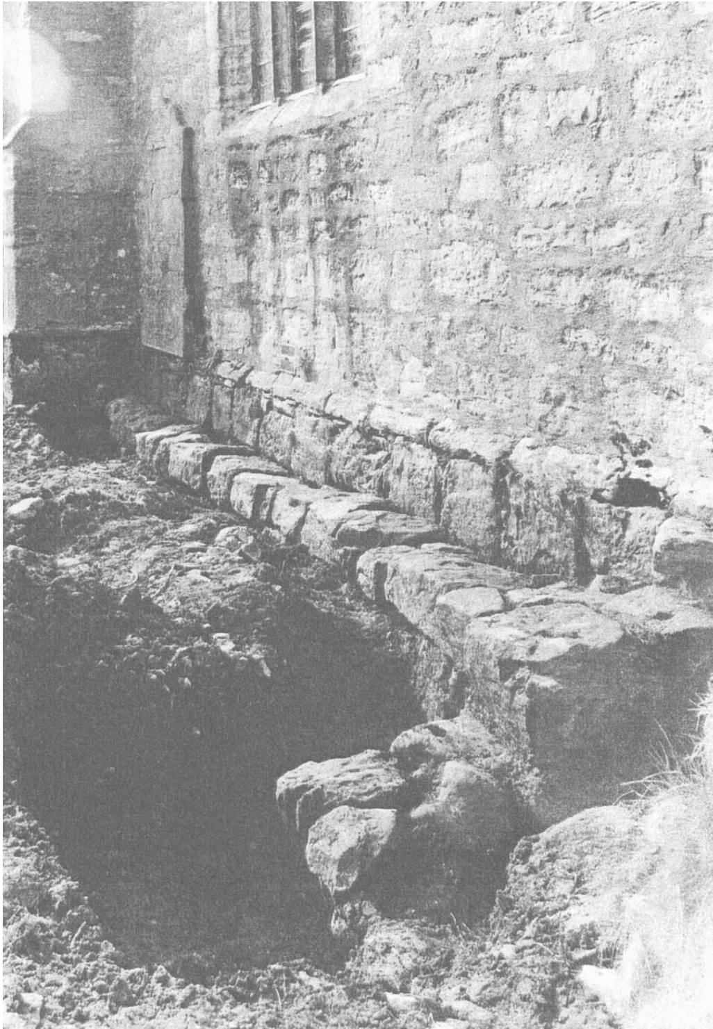
Plate 4: Photograph of external foundations of south side of Nave, Orton Church (from Cumbria County Council 1986)
