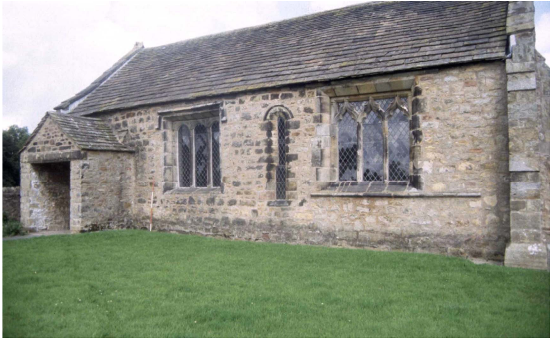
Plate 1: The south external elevation, looking north-west
