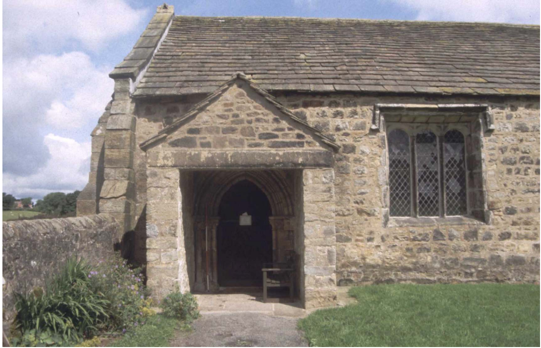
Plate 5: The porch, looking north
