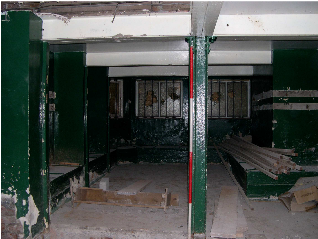
Plate 11: Concrete benches 15 and ceiling 14 in Room 6
