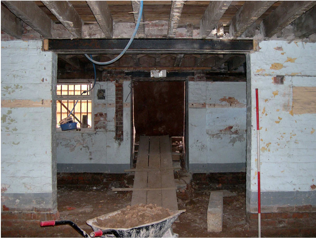
Plate 10: Doorway 02 and remodelled fireplace 05 in Rooms 1 and 2
