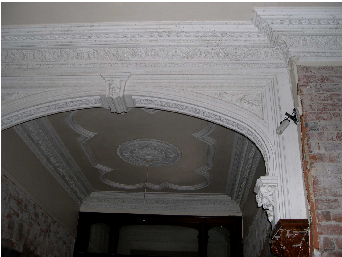
Plate 13: Arch detail in Room 9
