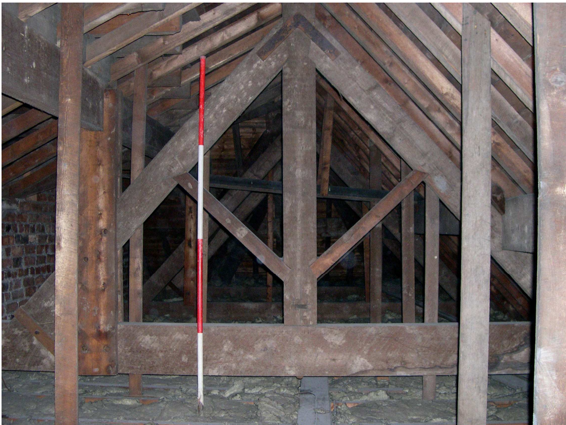
Plate 9: Truss within the western section of the roof space
