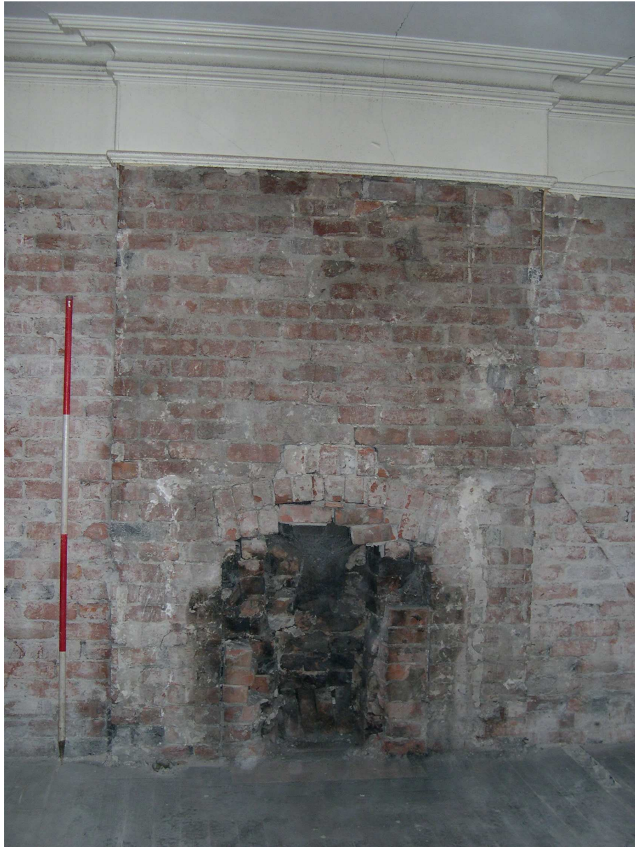
Plate 24: Blocked fireplace 49 in Room 23
