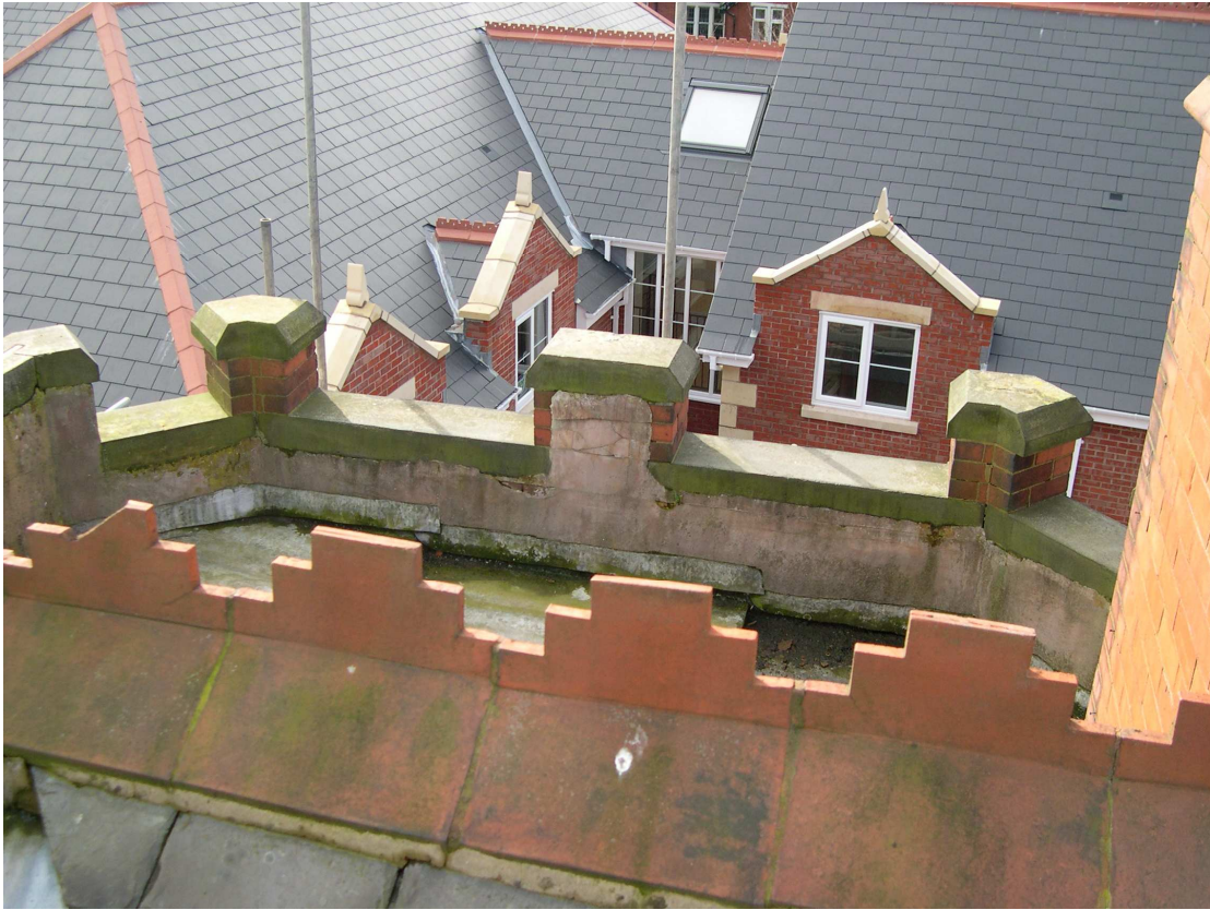
Plate 8: Parapet on the south side of the west part of the roof
