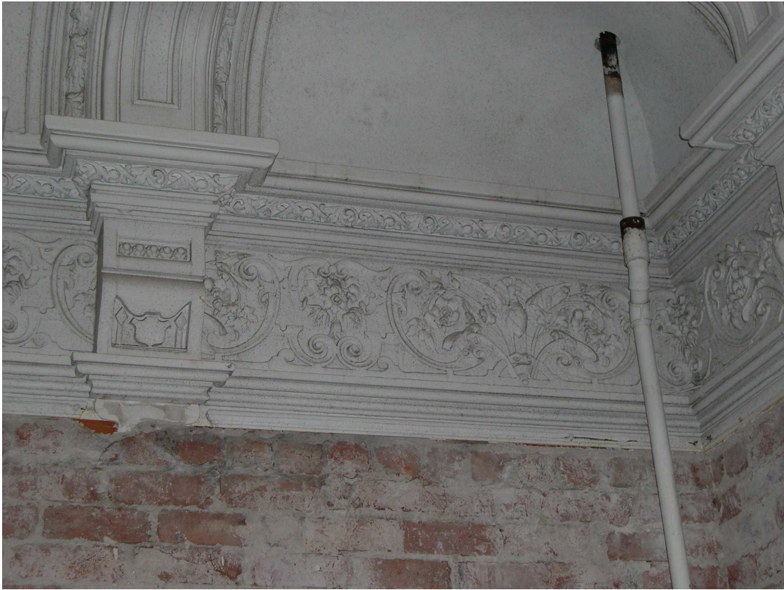
Plate 12: Cornice detail in Room 8
