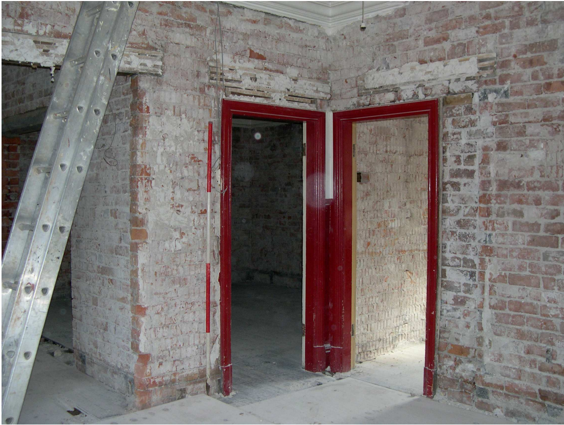
Plate 23: Remodelled doorway 40 and grooved brick wall 39 in Room 19
