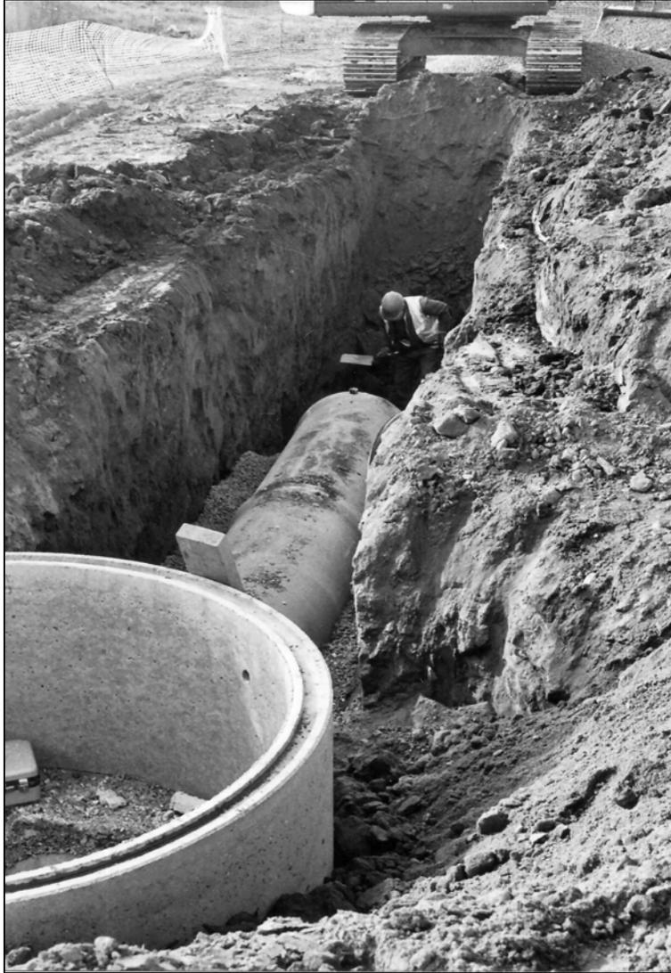
Plate 8: Excavation of the pipetrench for the main sewer under Phase 1 of the watching brief investigations
