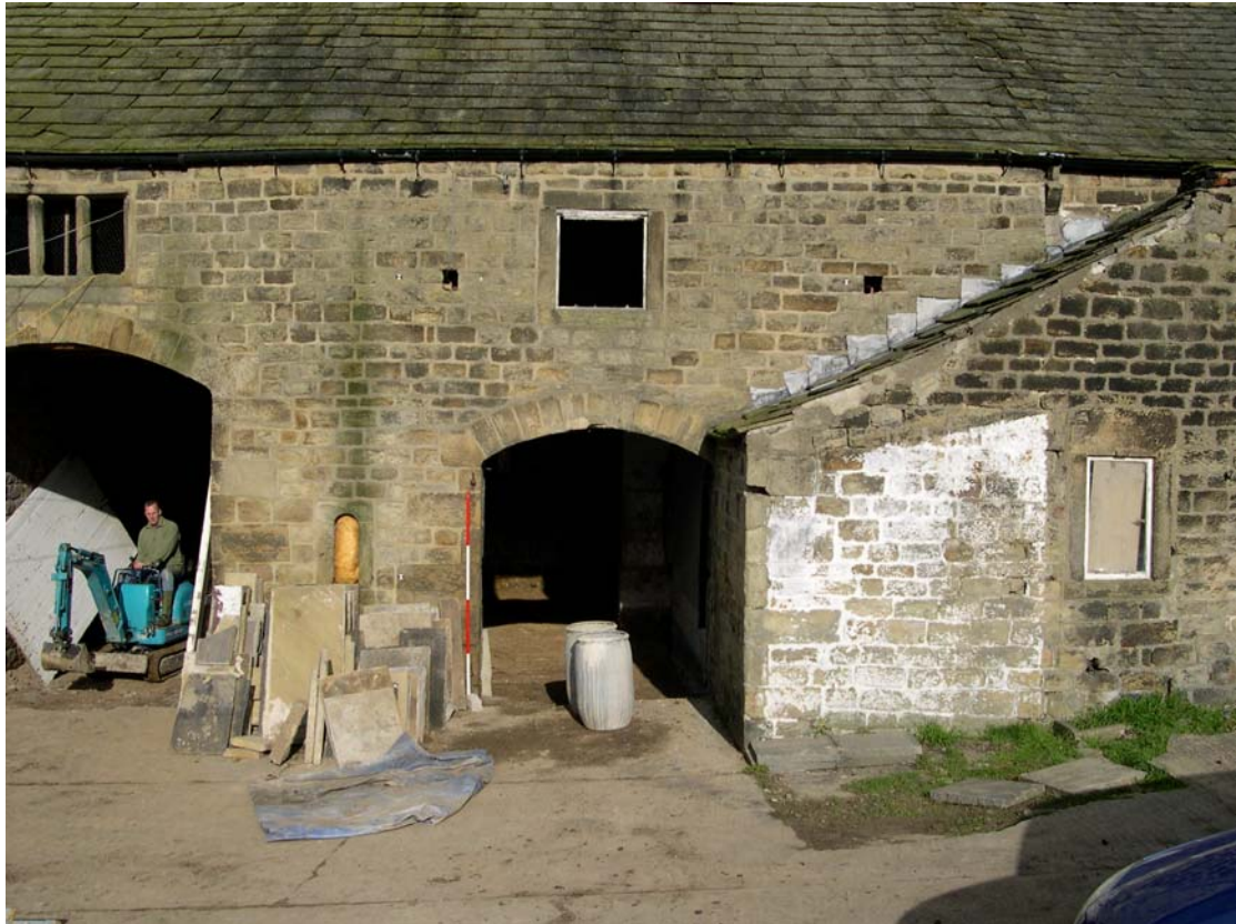
Plate 32: South elevation of the barn, eastern end
