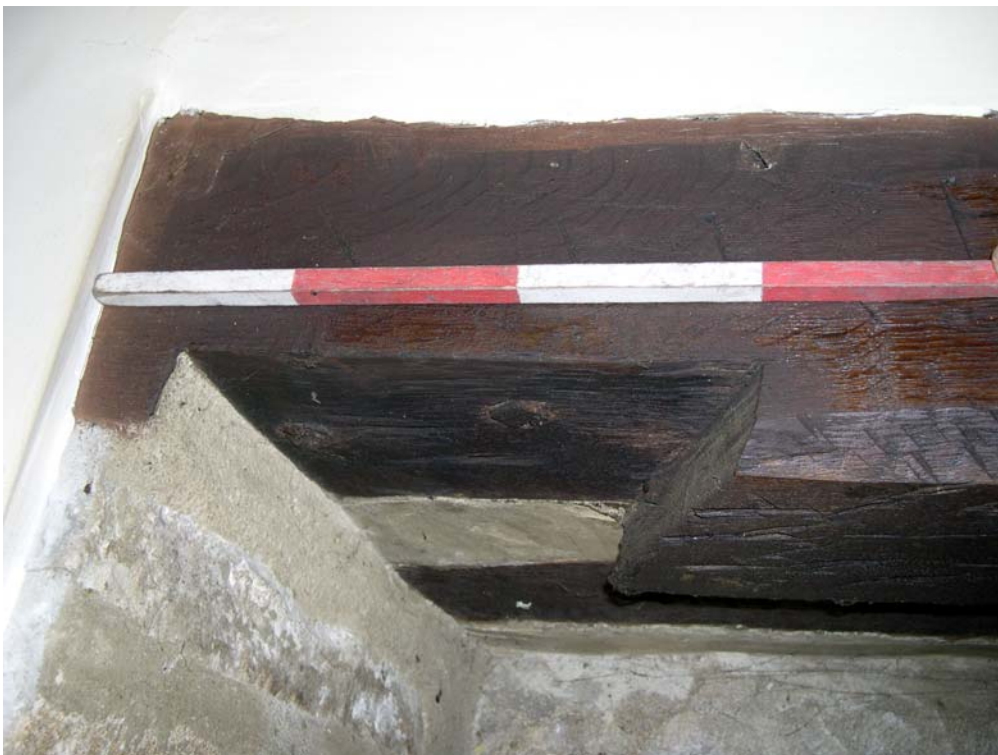
Plate 11: Re-used lintel above farmhouse door
