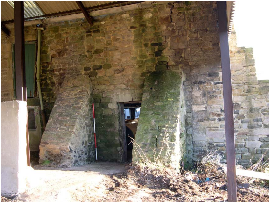
Plate 39: Buttresses on external northern elevation of attached cow-shed
