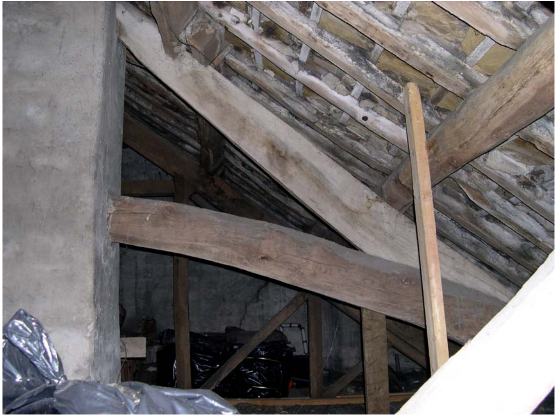
Plate 18: Additional principal rafters within roof-space over farmhouse outshut
