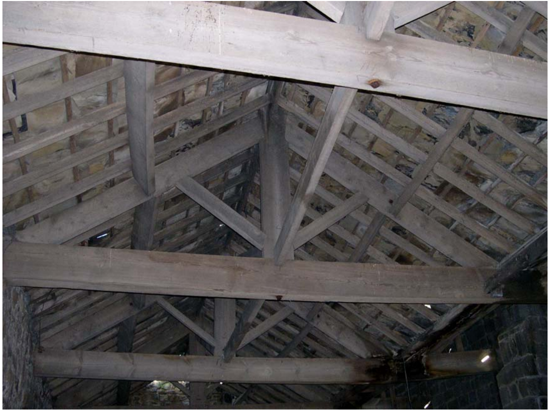
Plate 44: Roof trusses in attached cow-houses
