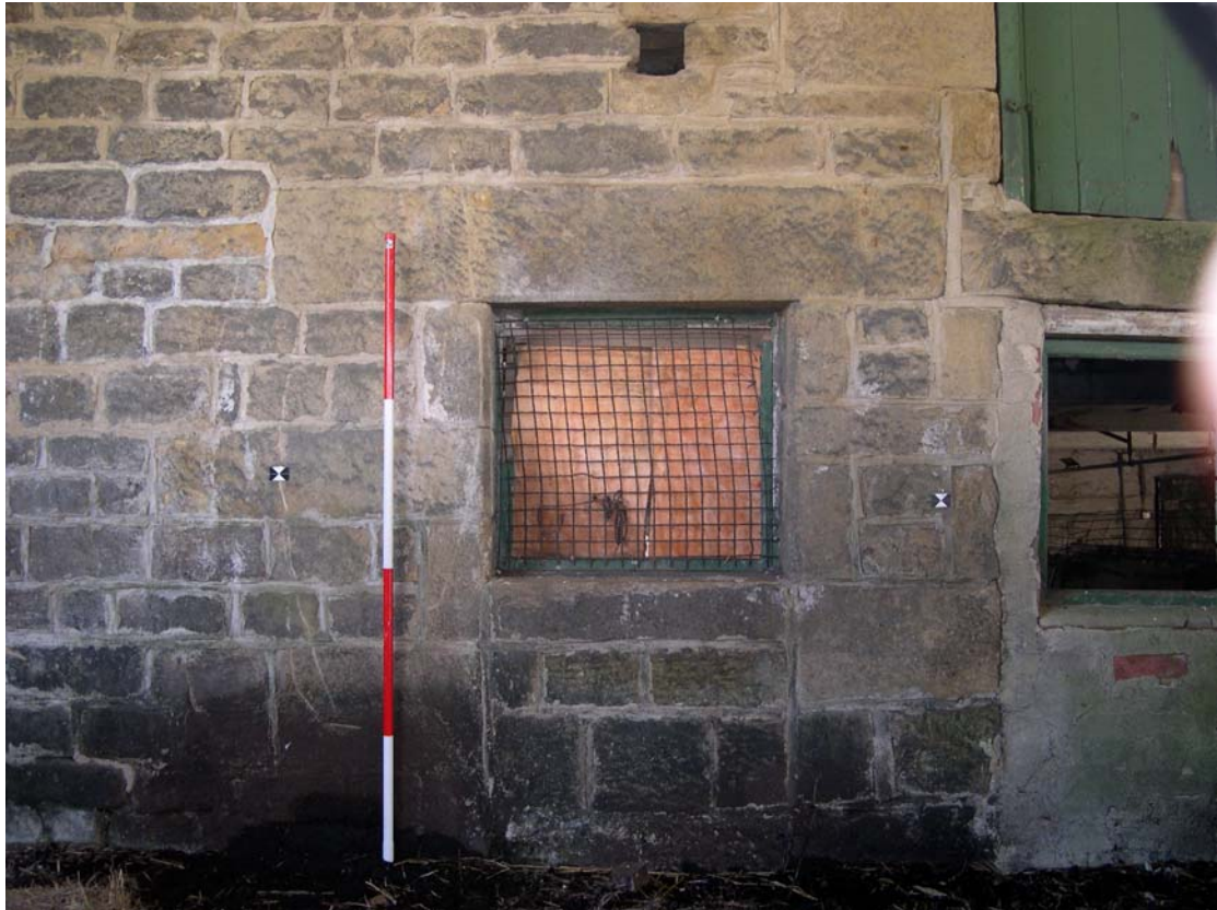
Plate 24: Remodelled doorway in north elevation of the cow-house
