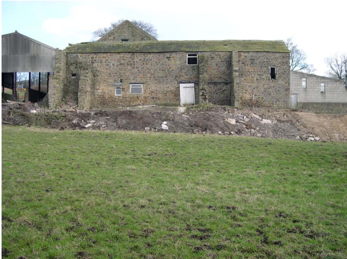
Plate 40: Buttresses on external western elevation of attached cow-sheds
