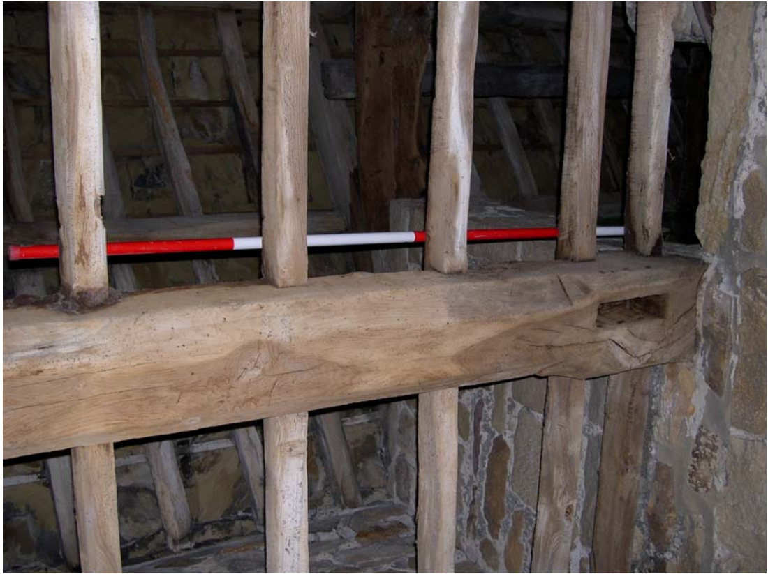
Plate 30: Mortise within re-used beam in the barn porch
