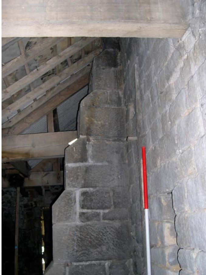
Plate 28: Upper part of arcade buttress by west external elevation of the barn
