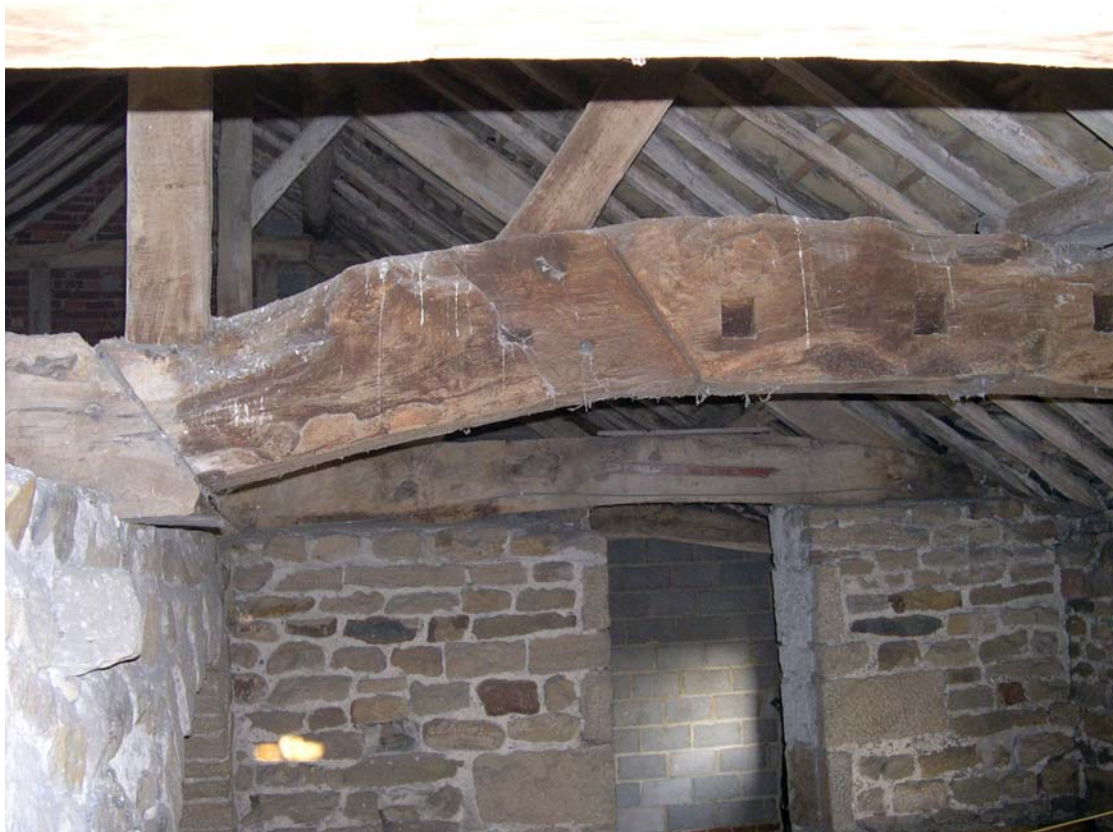
Plate 35: Scarf joint over arcade plate and redundant joints in tie-beam
