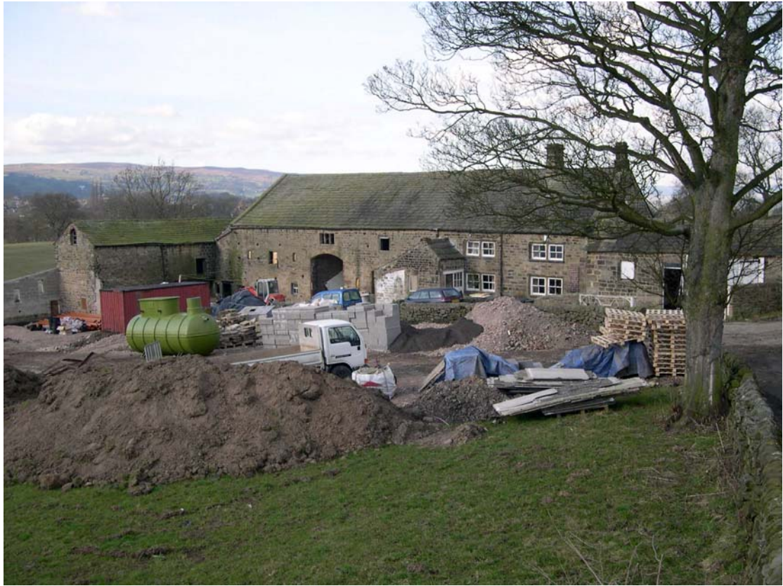
Plate 6: View of site from south-east
