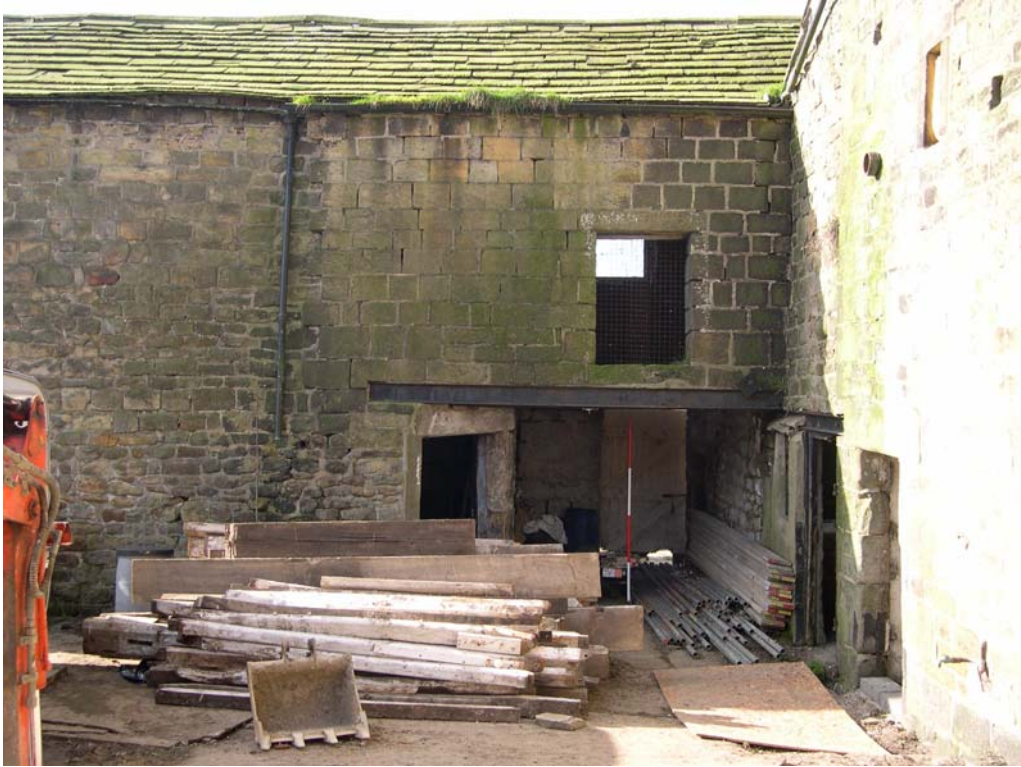
Plate 42: East elevation of attached cow-houses
