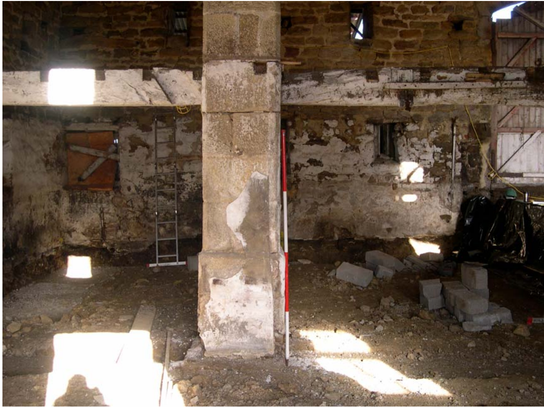
Plate 26: Lower south part of western arcade column
