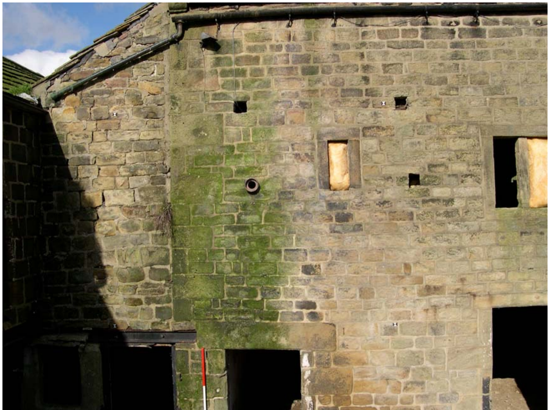
Plate 19: Sockets and rectangular vents in south elevation of the barn
