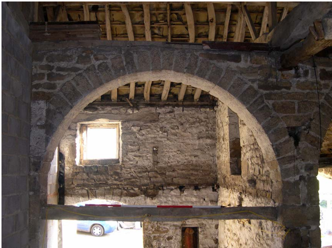
Plate 33: Bridging joist across the face of the arcade
