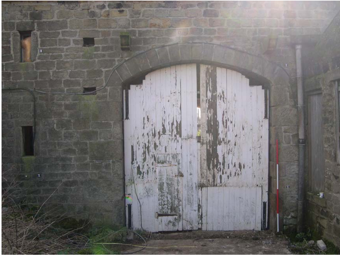
Plate 20: Wagon-door in north elevation of the barn
