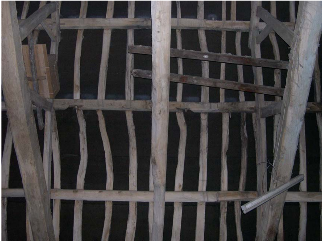
Plate 36: Re-used purlins, and rafter detail in the barn
