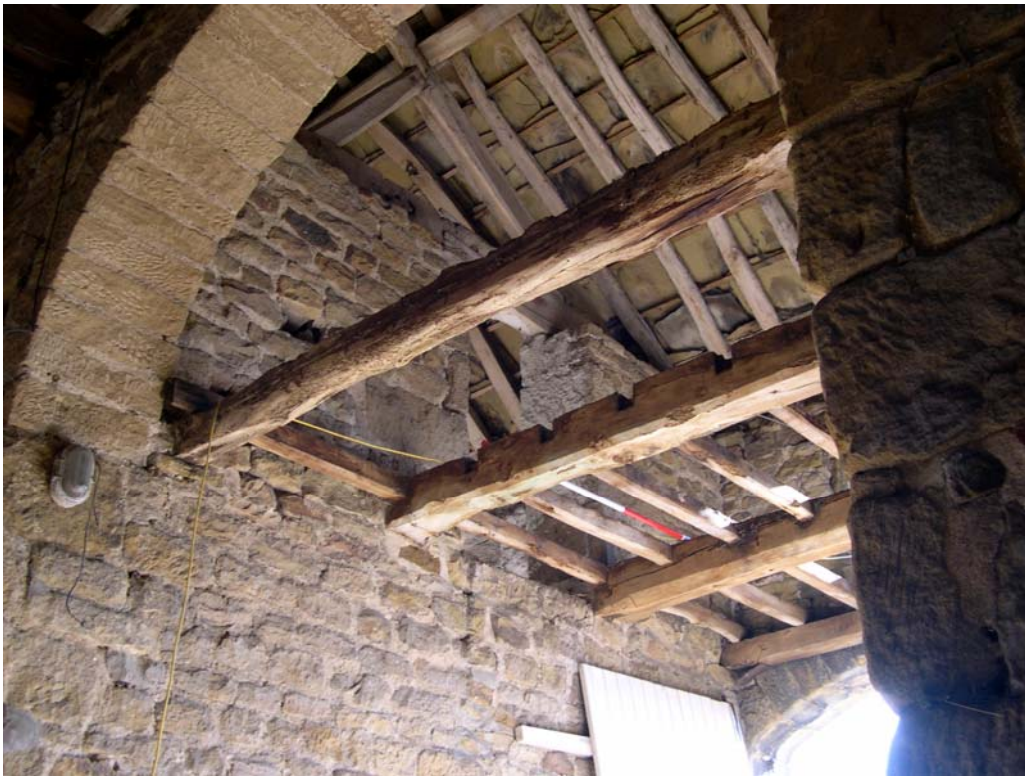
Plate 29: Re-used beams supporting floor joists in the barn porch
