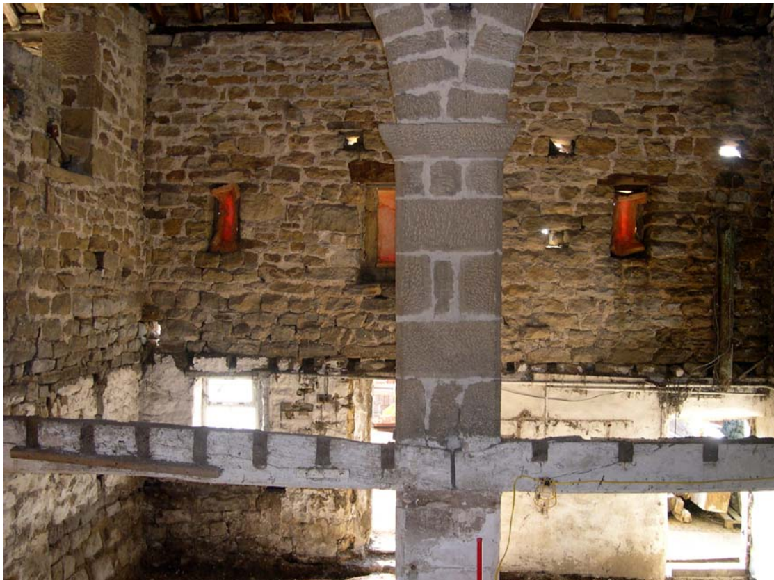
Plate 27: Upper north part of western arcade column, showing chamfered impost
