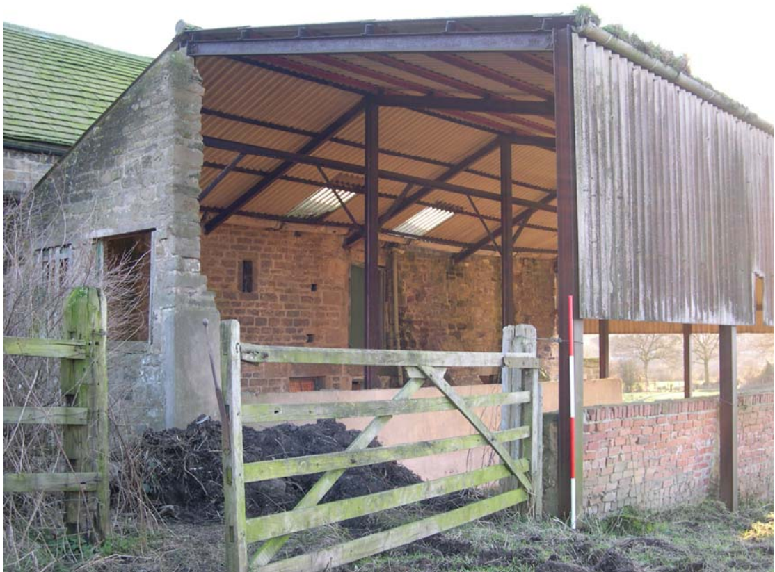
Plate 37: Twentieth century shelter shed attached to northern side of the barn
