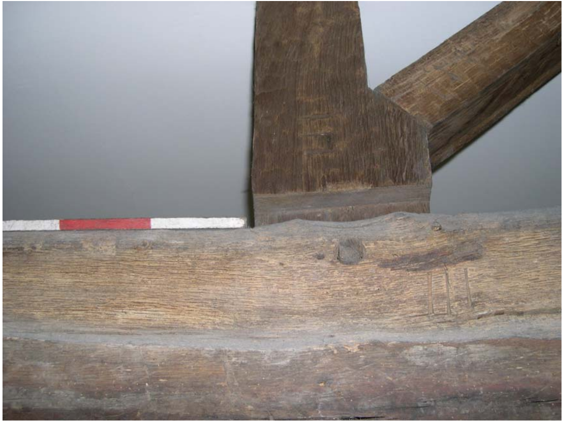
Plate 16: Assembly marks on farmhouse truss
