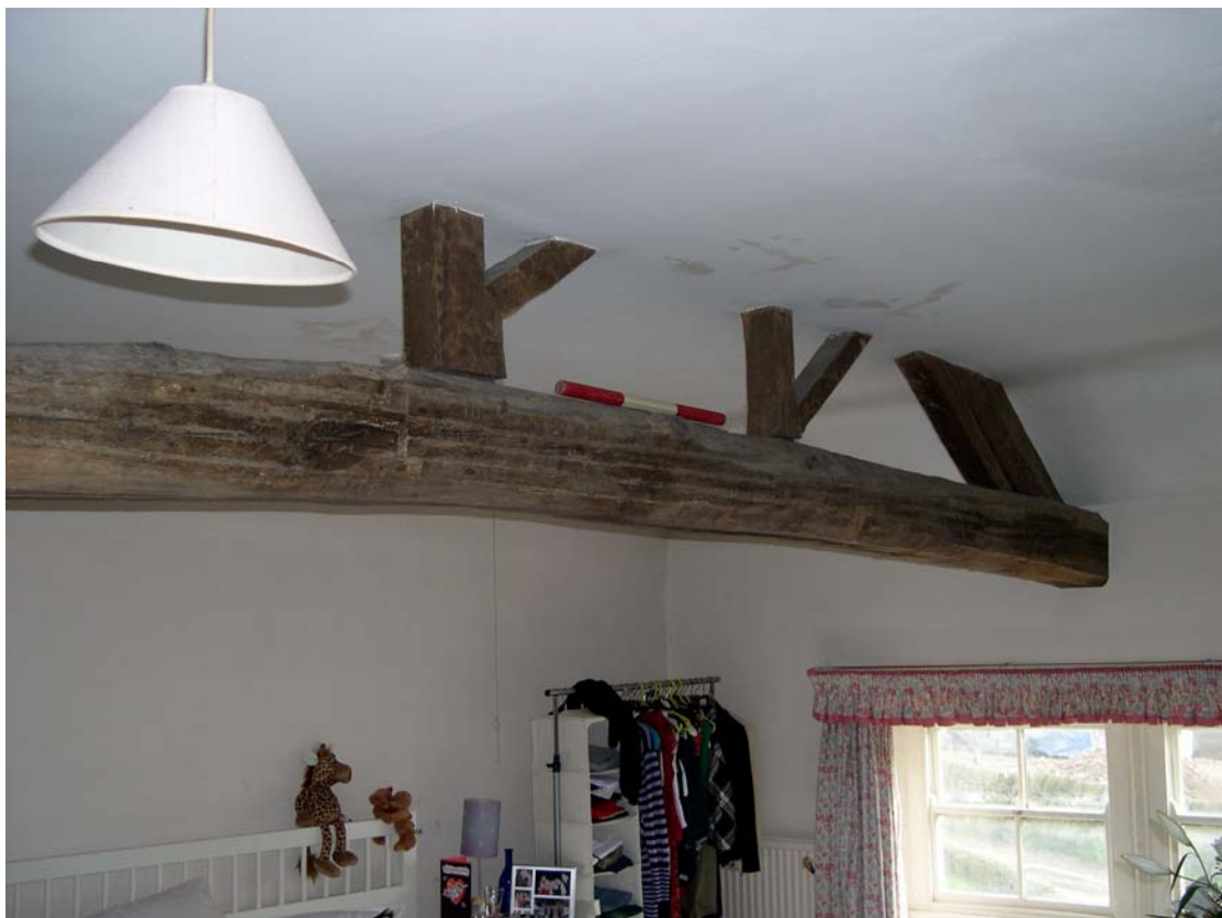
Plate 15: Queen and princess posts in farmhouse truss
