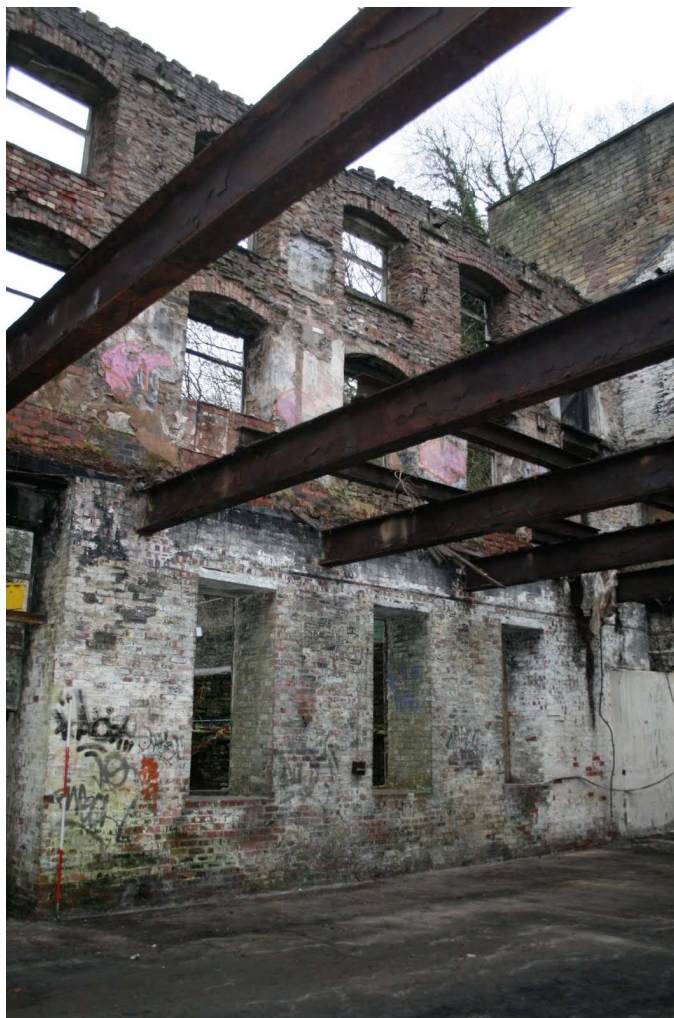
Plate 32: Western bays of south elevation, Building I, showing refaced ground floor
