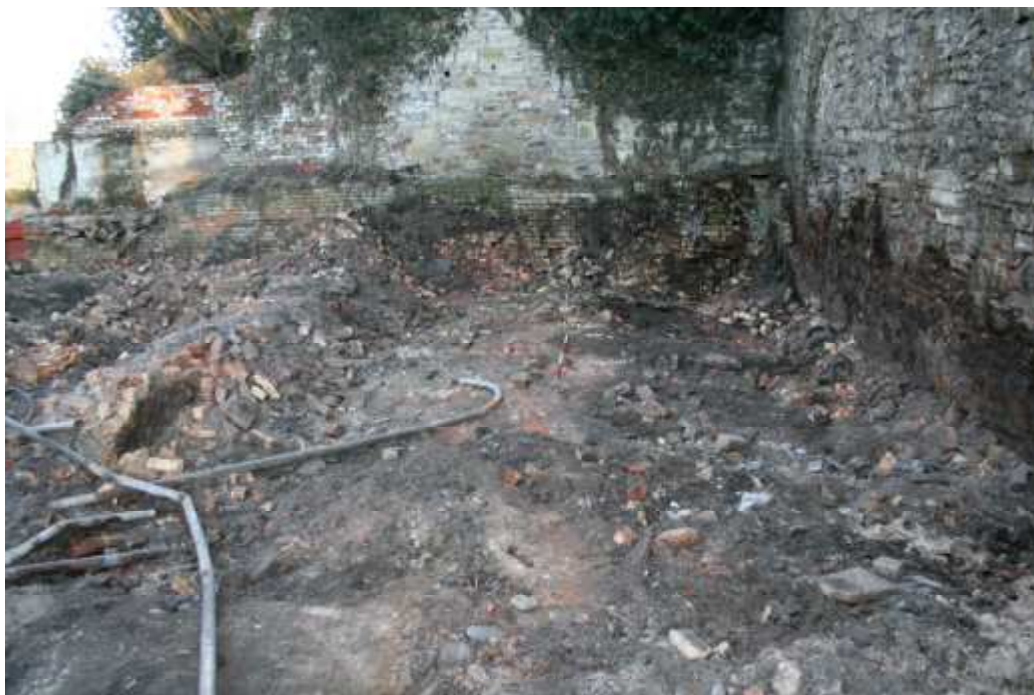
Plate 35: Footprint of Building E following demolition
