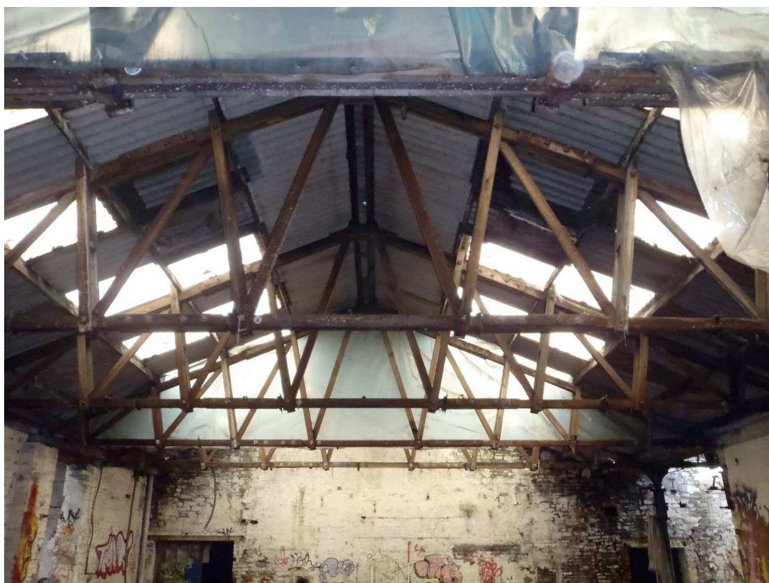
Plate 15: Rooftrusses within Building Q,
