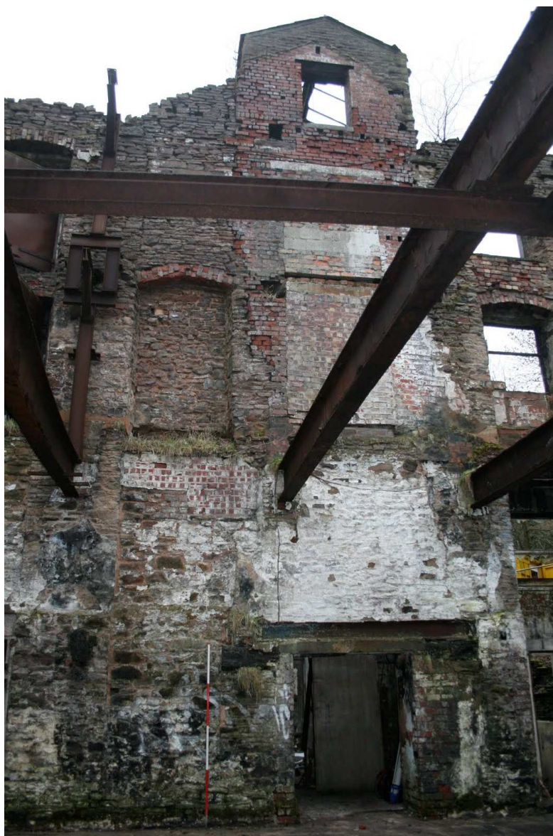
Plate 30: Bays 7 and 6, south elevation, showing blocked doorways and brick hoist tower J
