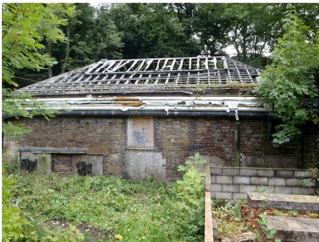
Plate 13: Front elevation of Building P, with raised ground level in the foreground
