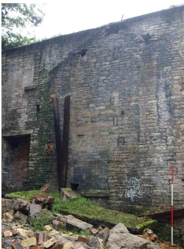
Plate 4: Wall scar of Building D on northern elevation of Building E
