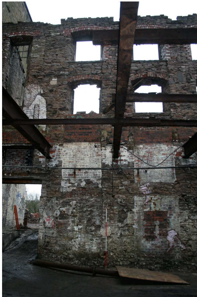
Plate 17: North internal elevation, Building I, with diminishing wall thickness and window size, blocked apertures and narrow upper Bay 1 window
