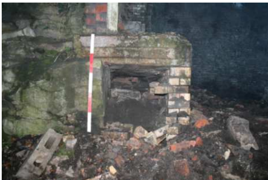
Plate 37: Flue on boiler bench, and at rear (right) of both visible beds into main flue
