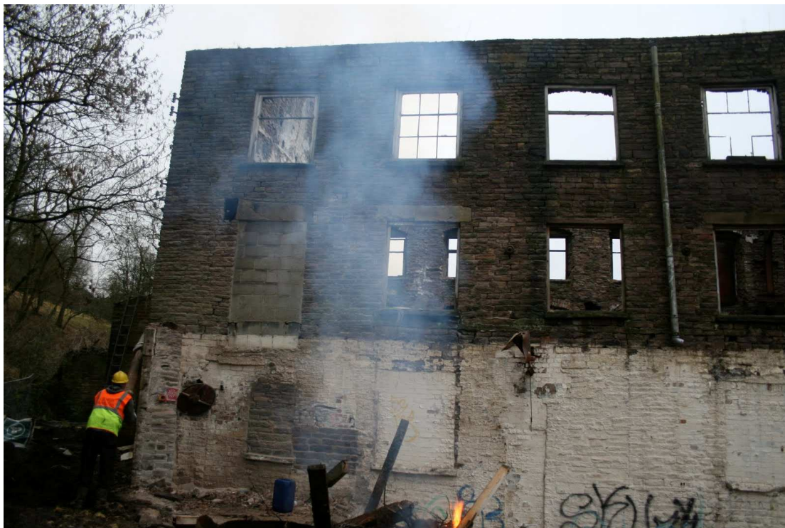
Plate 18: Eastern end of north elevation, Building I, with remodelled aperture in end bay
