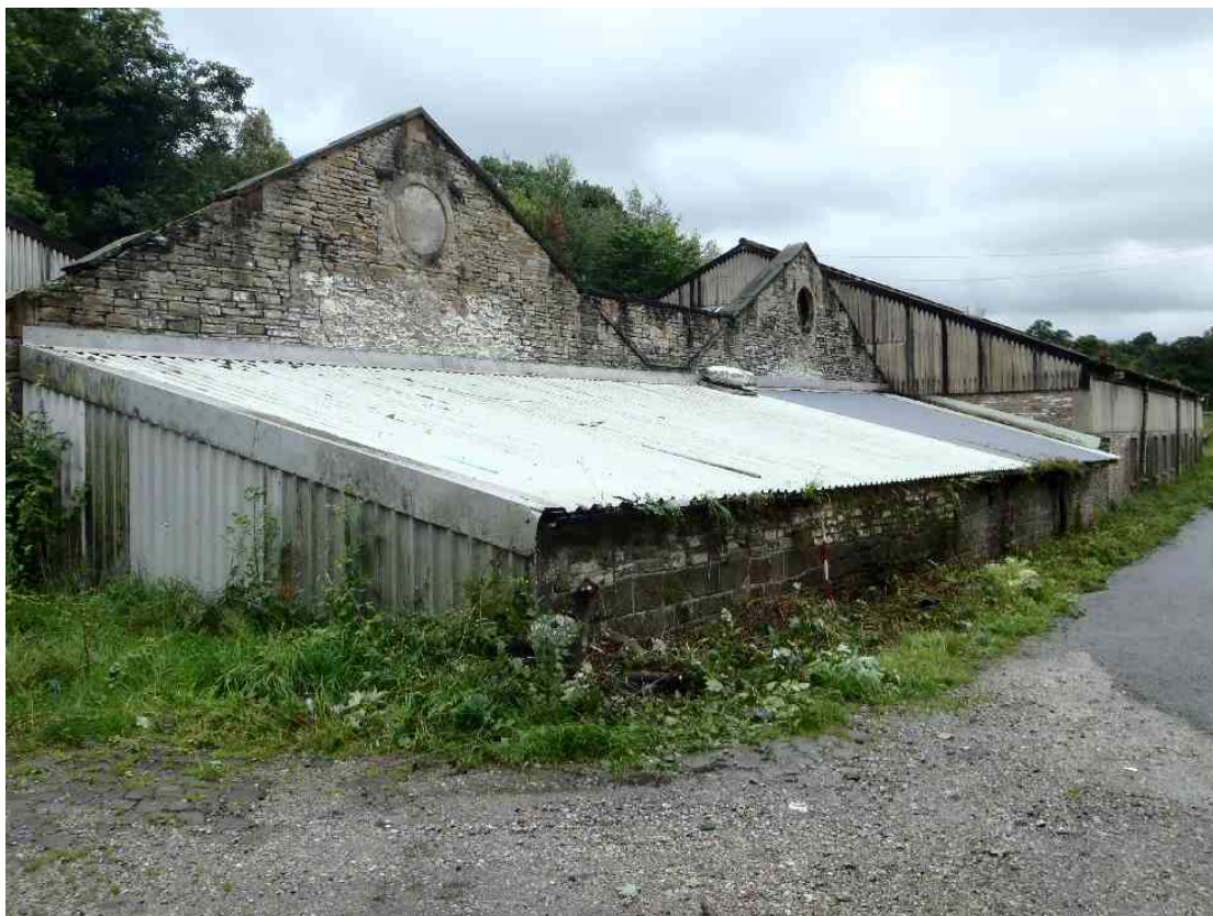
Plate 14: West elevation of Building R, western gables of Building Q above
