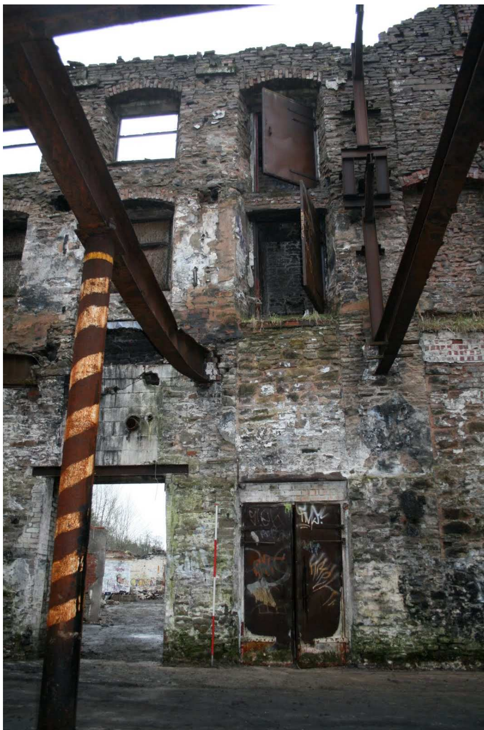
Plate 28: Bay 8, south elevation, Building I, showing doorways into stair tower J
