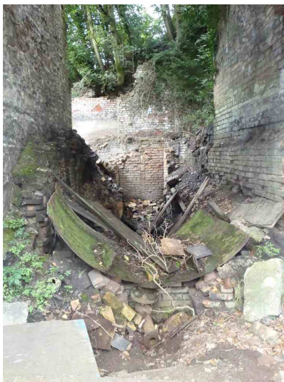
Plate 6: In-situ remains of a Cornish boiler, Building E
