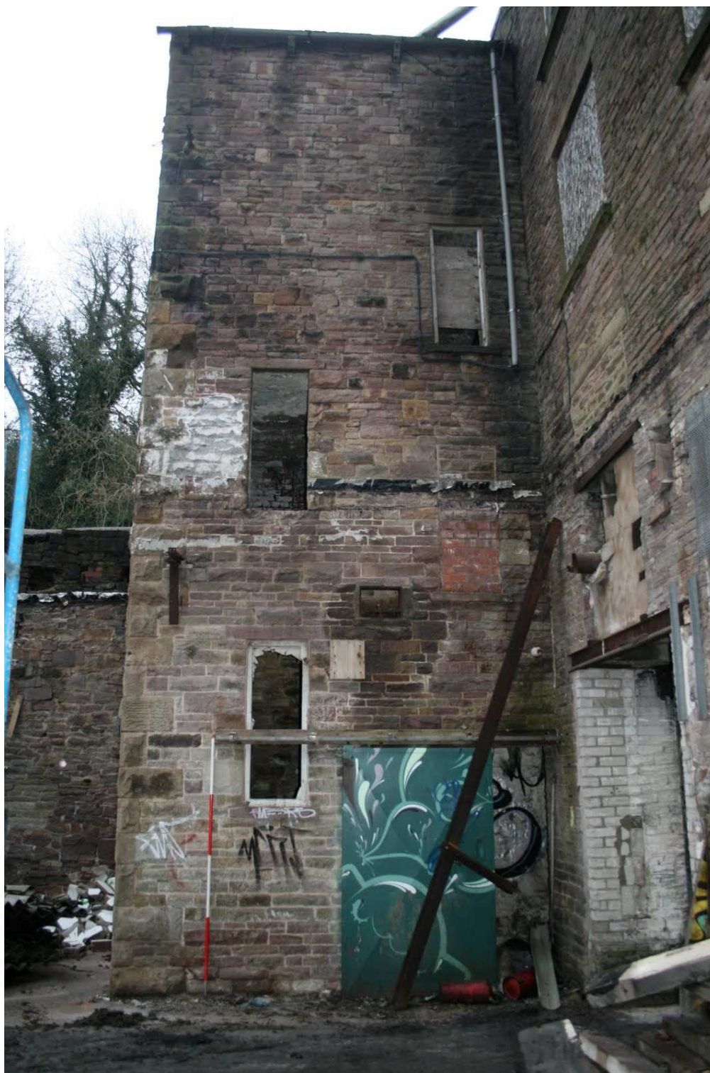
Plate 29: East wall of stair tower with landing windows and two inserted bearing boxes
