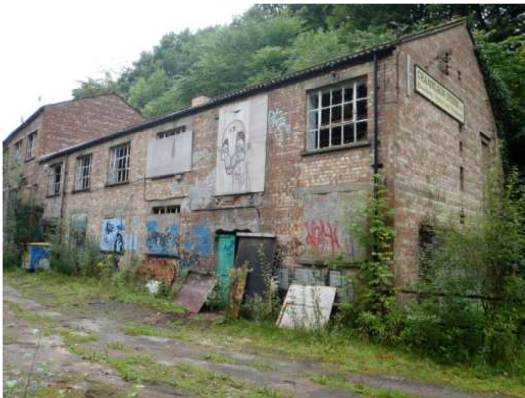
Plate 2: East elevation of Building A, with Building B to the rear
