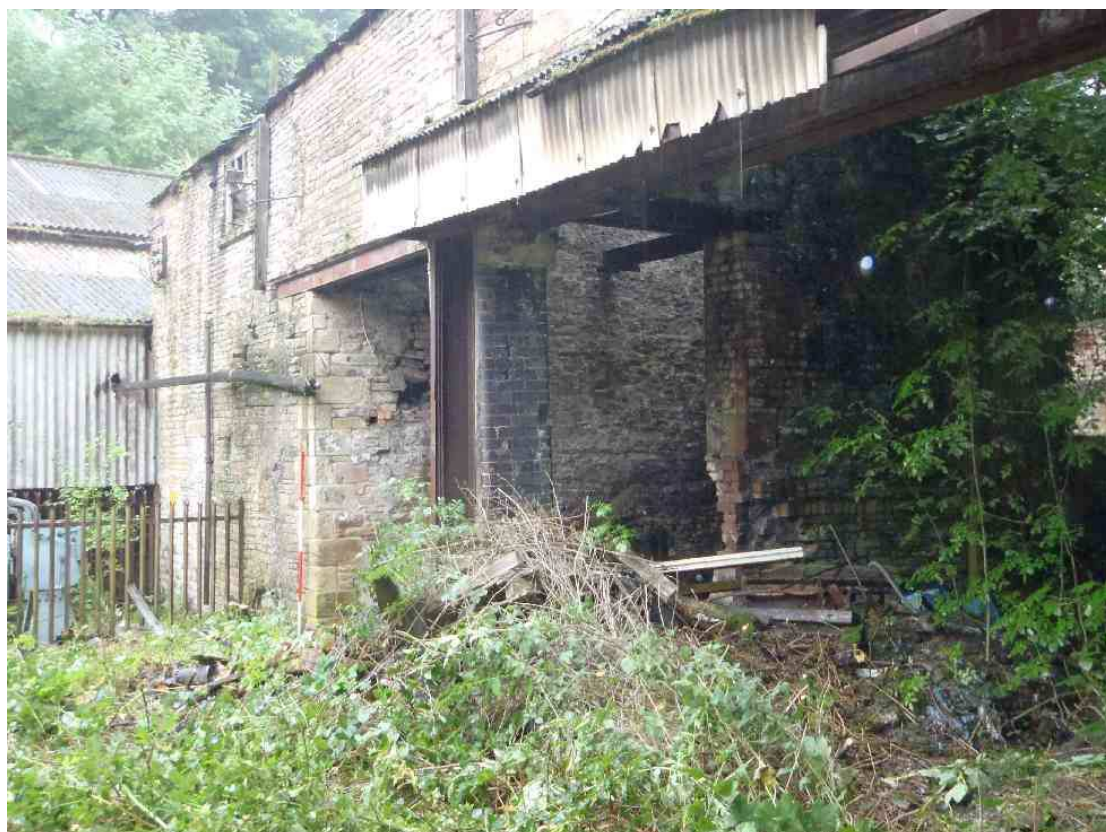
Plate 8: Open frontage of boiler house in eastern part of Building E
