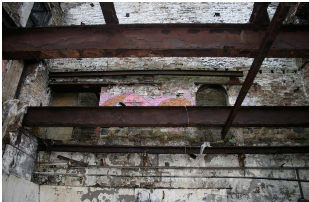
Plate 21: Apertures inserted into the western gable of the spinning block, into Building H
