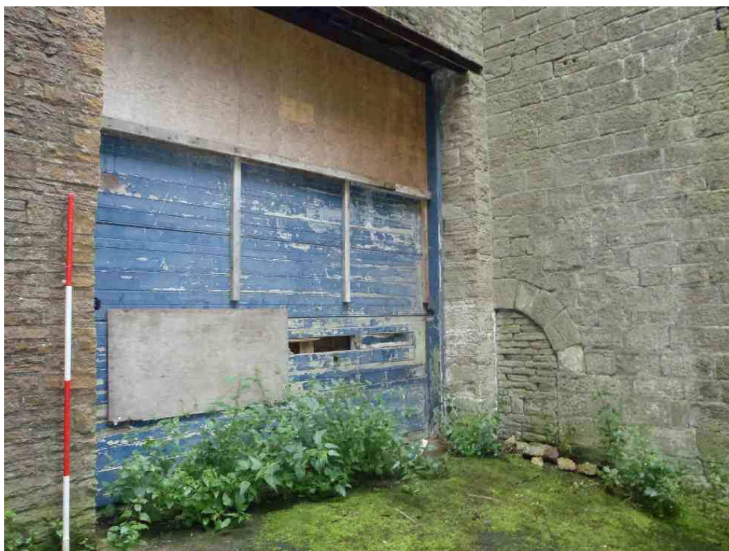
Plate 11: South elevation of Building G, with blocked aperture in west elevation of Building H
