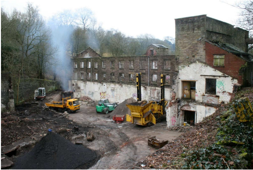
Plate 16: General view of the spinning block, Building I, and wheel house Building H
