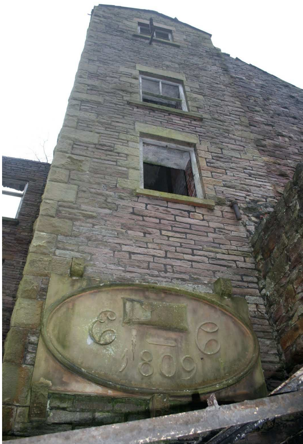
Plate 31: Southern elevation of hoist tower, J, with repositioned datestone of 1809
