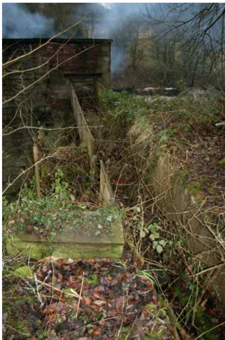
Plate 34: Detail of iron-sheet trough from reservoir into wheel house
