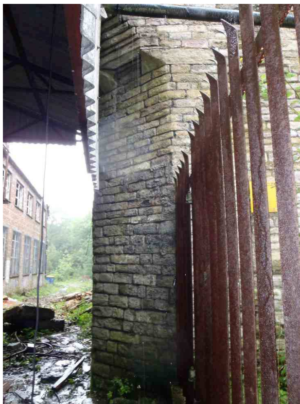
Plate 7: Chamfered ground floor return of Building E
