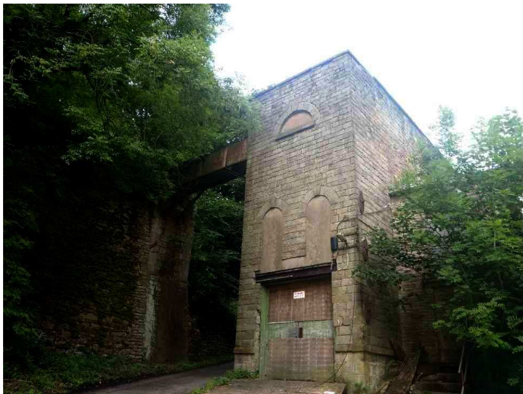
Plate 33: Large 1850s wheel house, with cast iron trough supplying water from a reservoir
