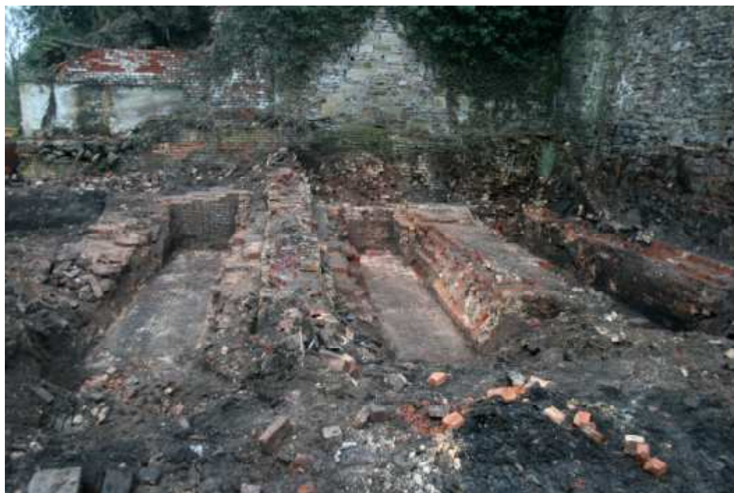
Plate 36: Three boiler beds with partially intact benches observed below Building E
