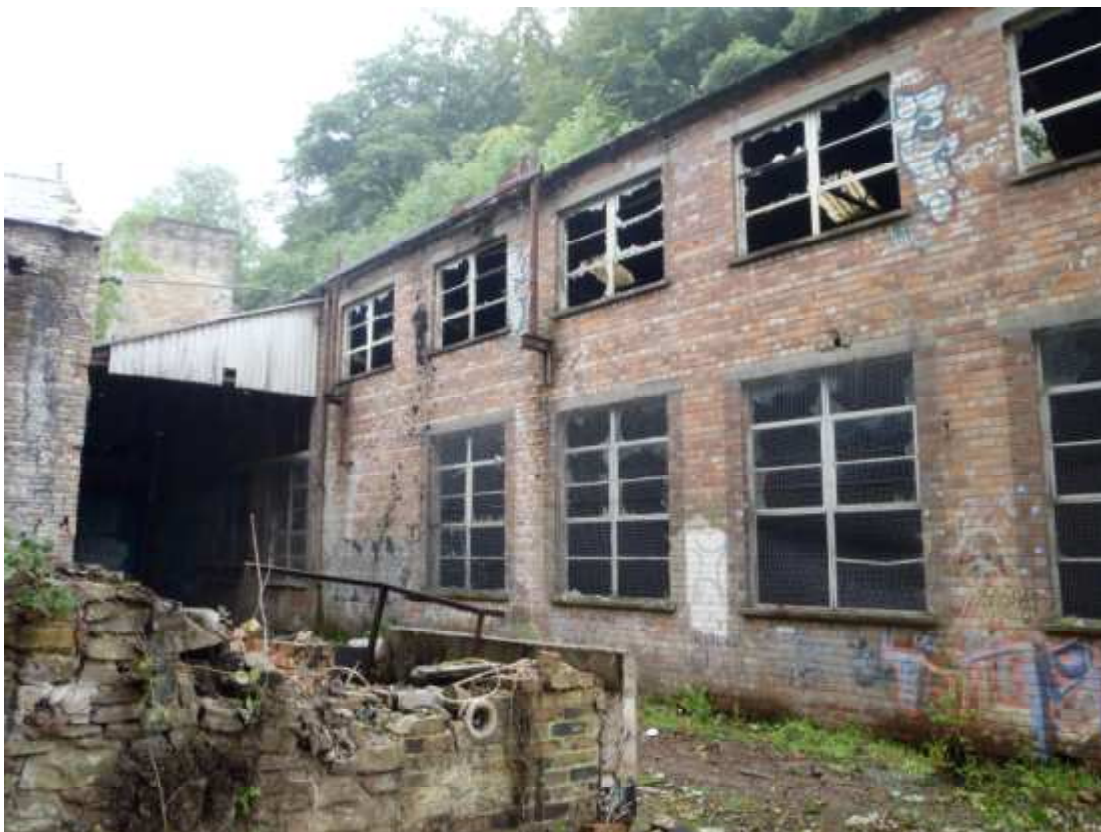
Plate 3: East elevation of Building B, with canopy to building F behind
