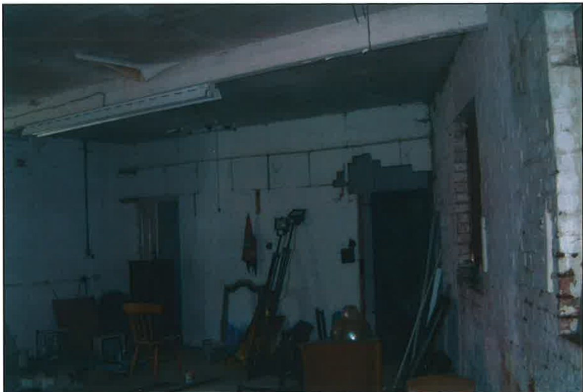
Plate 17: OAU 10 East view of shopfitter's first floor administration area
