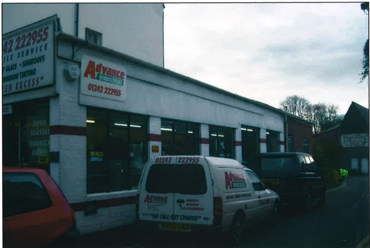
Plate 21: OAU 17 North elevation
