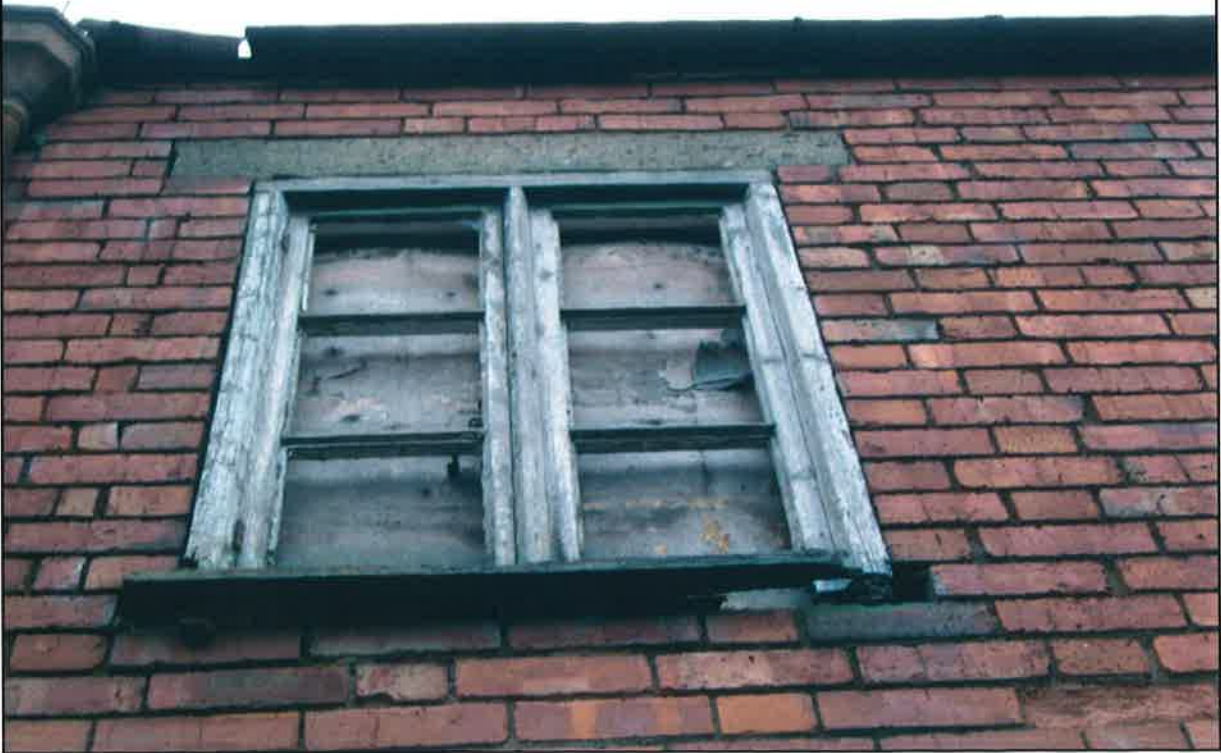
Plate 7: OAU 10 South elevation, first floor window
