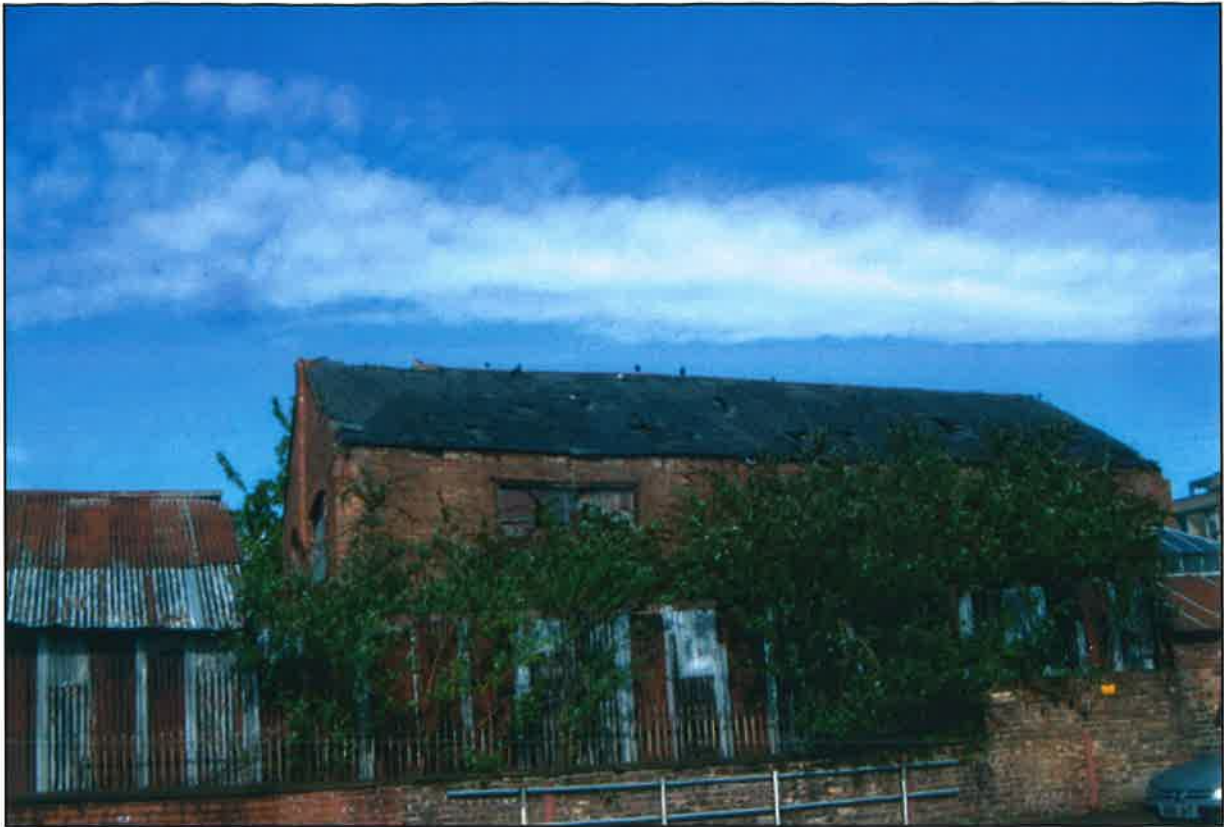
Plate 5: OAU 10 Warehouse, east elevation
