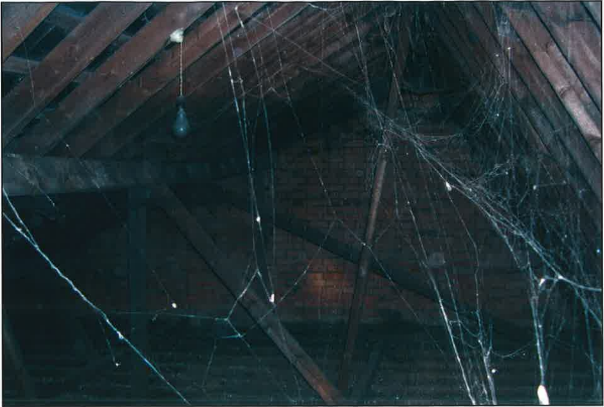
Plate 18: OAU 10 West view of roof
