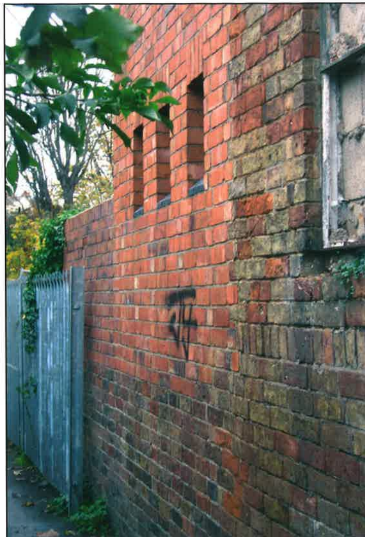
Plate 8: OAU 10 South elevation, showing later extension to west
