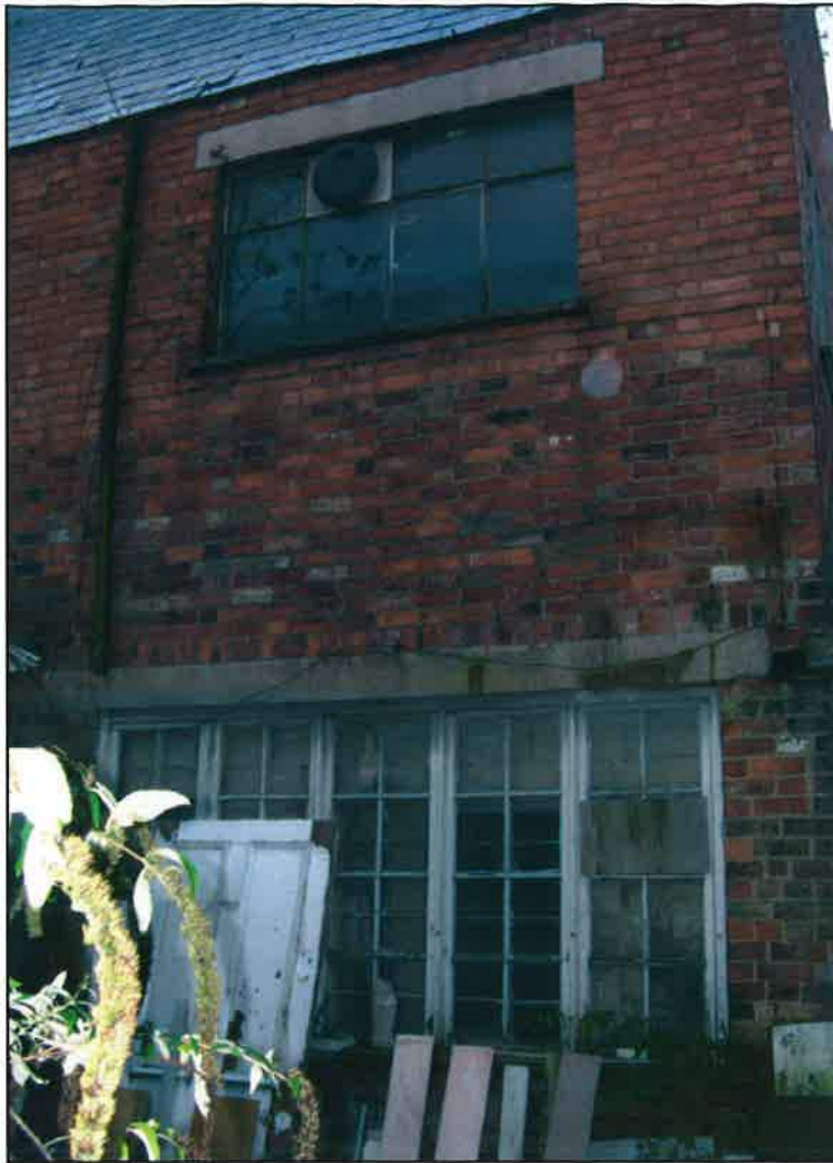
Plate 9: OAU 10 North elevation, showing phasing of brickwork
