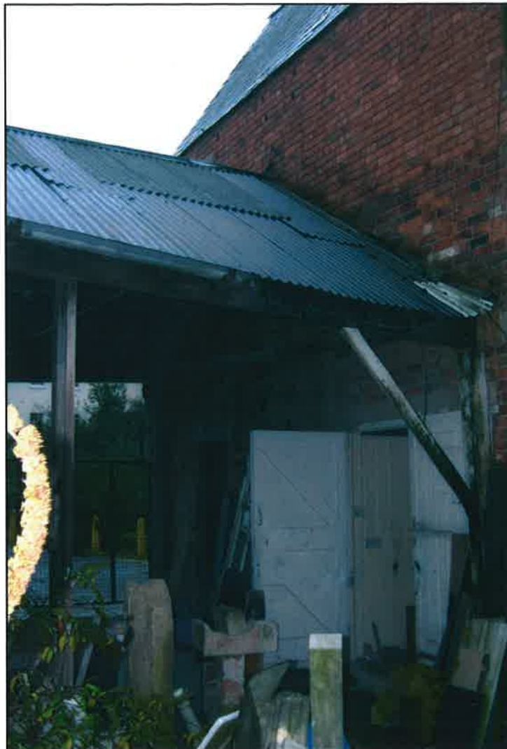
Plate 19: OAU 10 External covered courtyard area to the east
