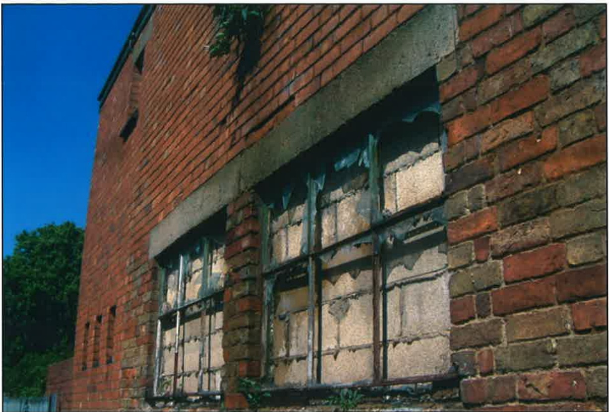
Plate 6: OAU 10 South elevation, ground floor windows
