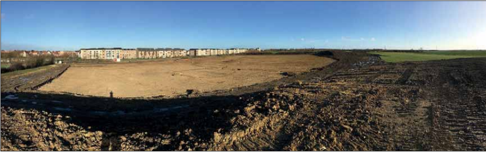
Plate 1: Panoramic Photo of Site 4i fully stripped, looking north-west
