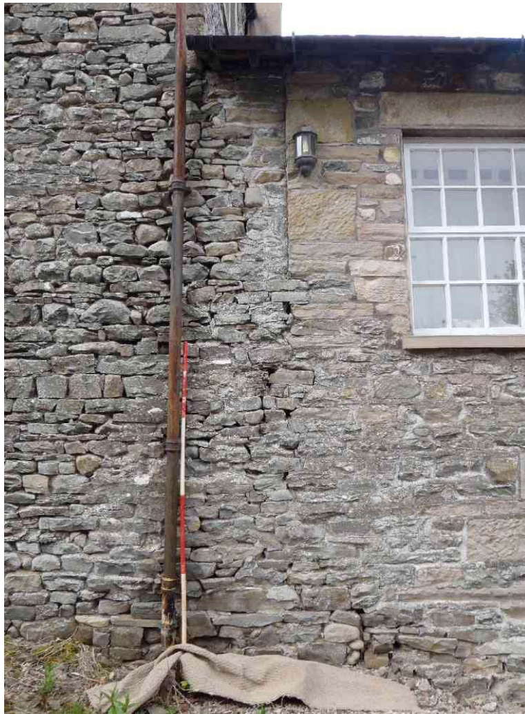
Plate 6: Quoins abutting the east end of the warehouse, suggesting it was originally detached at this end
