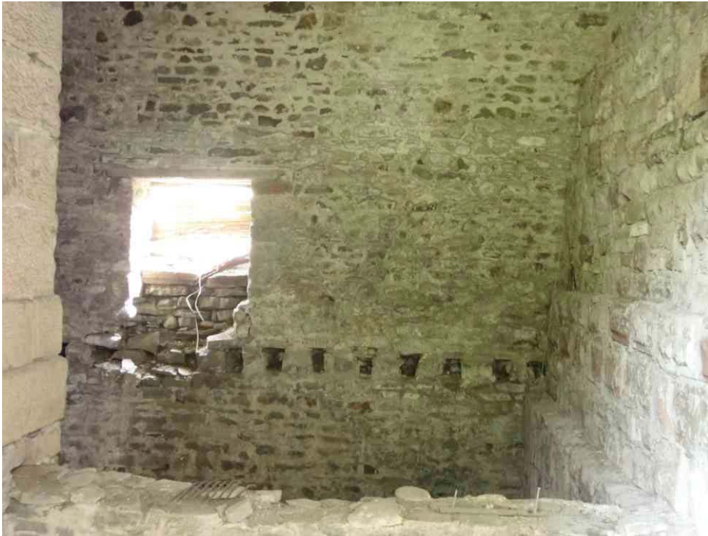
Plate 15: The joist sockets and associated sill within the adjoining wall, indicative of a former floor, first floor (east end)
