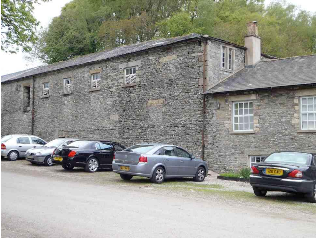
Plate 3: The south elevation of the warehouse, showing blocked windows and a central line of repair
