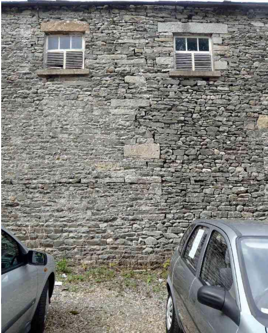
Plate 5: Line of rebuild or repair in the north elevation
