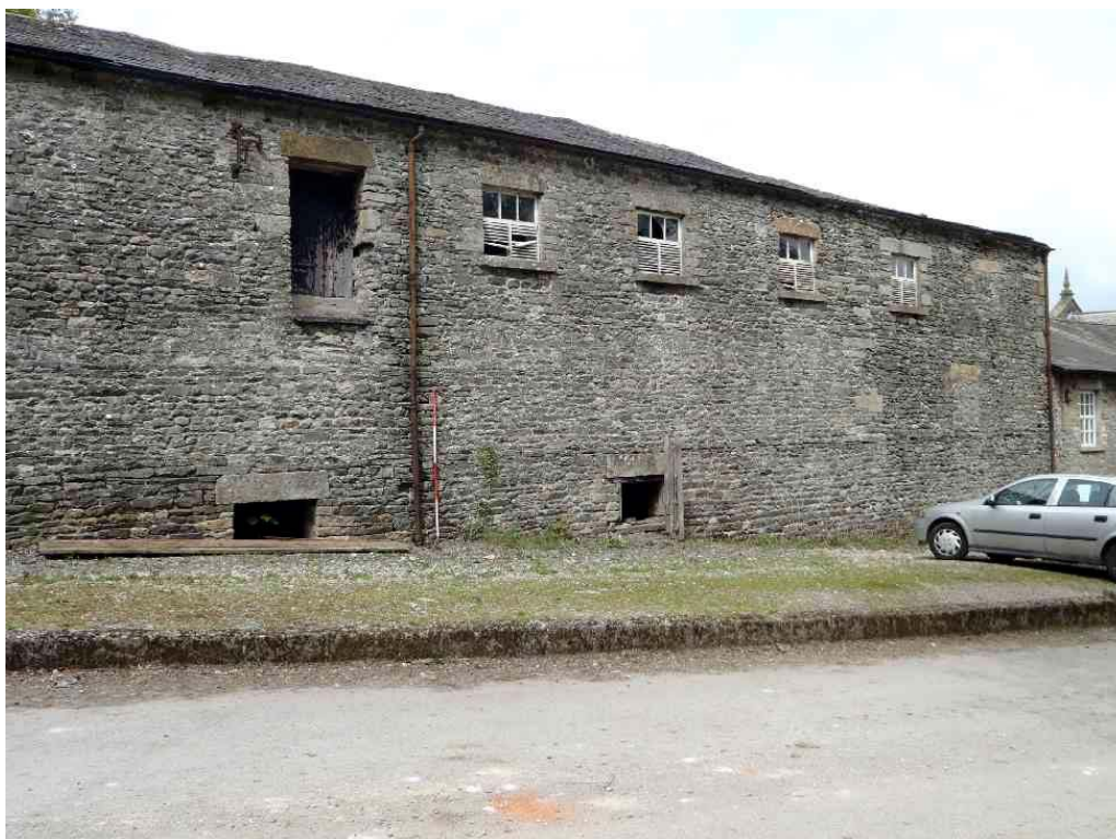
Plate 4: General view of the south elevation of the warehouse
