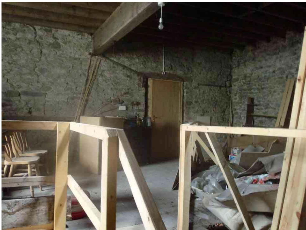
Plate 16: East end of the first floor with doorway into the adjoining building
