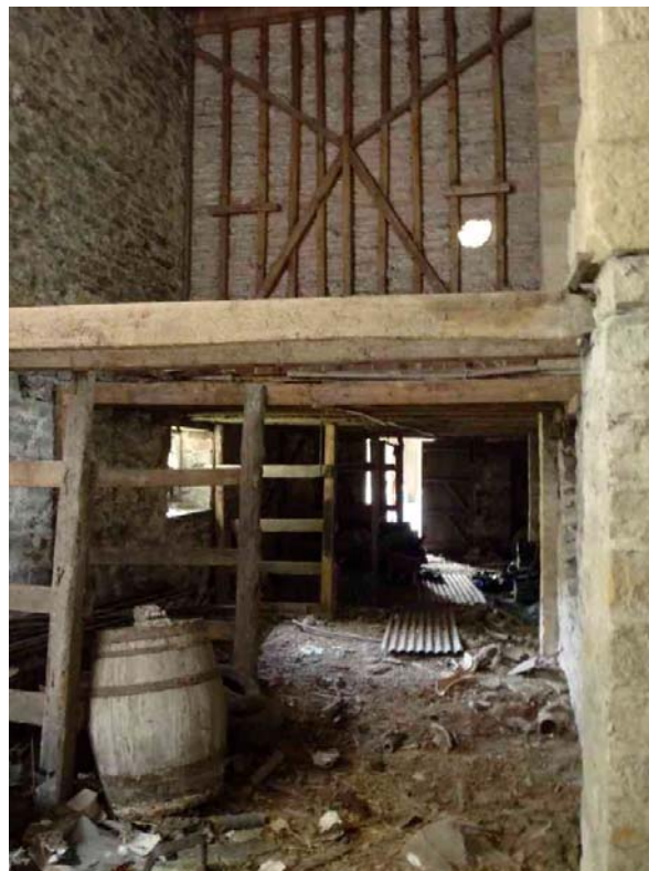
Plate 14: Northern half of the ground floor, showing timber storage bays, and the self-contained room above
