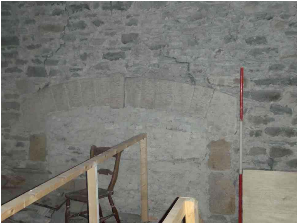
Plate 17: Voussoirs of blocked arch in the dividing wall between the east and west ends of the warehouse, at first floor height
