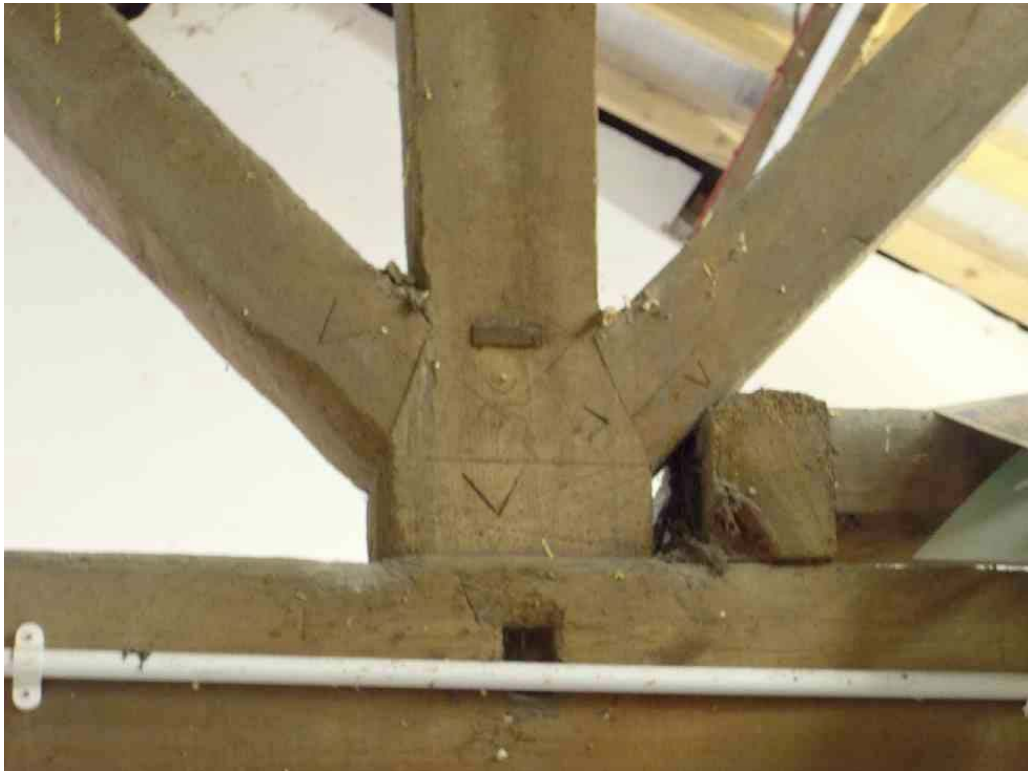
Plate 21: Truss within the mill marked on the upper face with a 'V'
