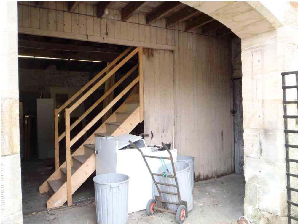
Plate 10: View through ground floor entrance to warehouse, east end
