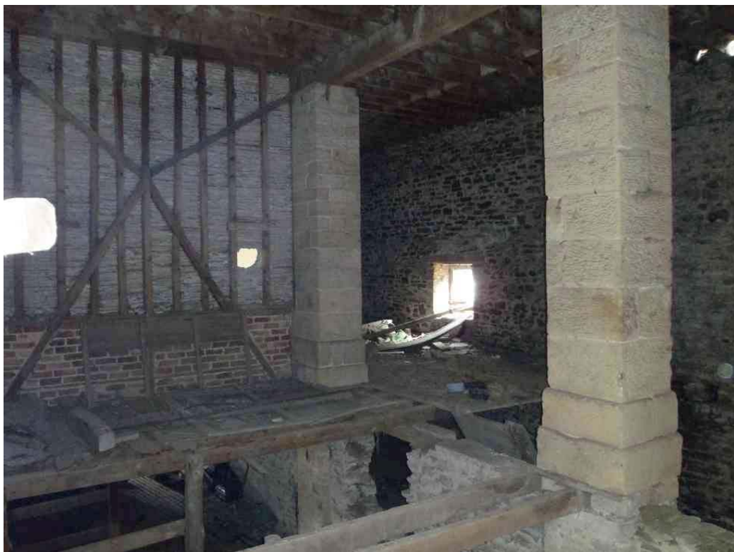
Plate 18: First floor viewed from safe access at the east end. The partition wall is part of the self-contained room relating to the former north range
