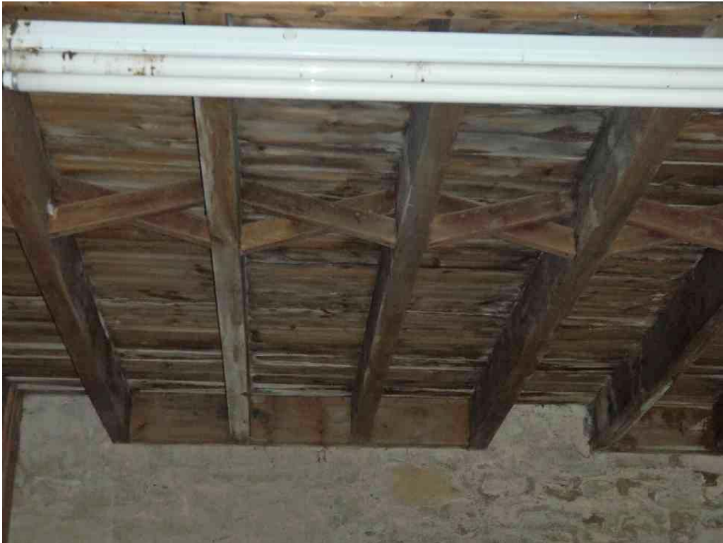
Plate 13: Herringbone struts between first-floor floor joists
