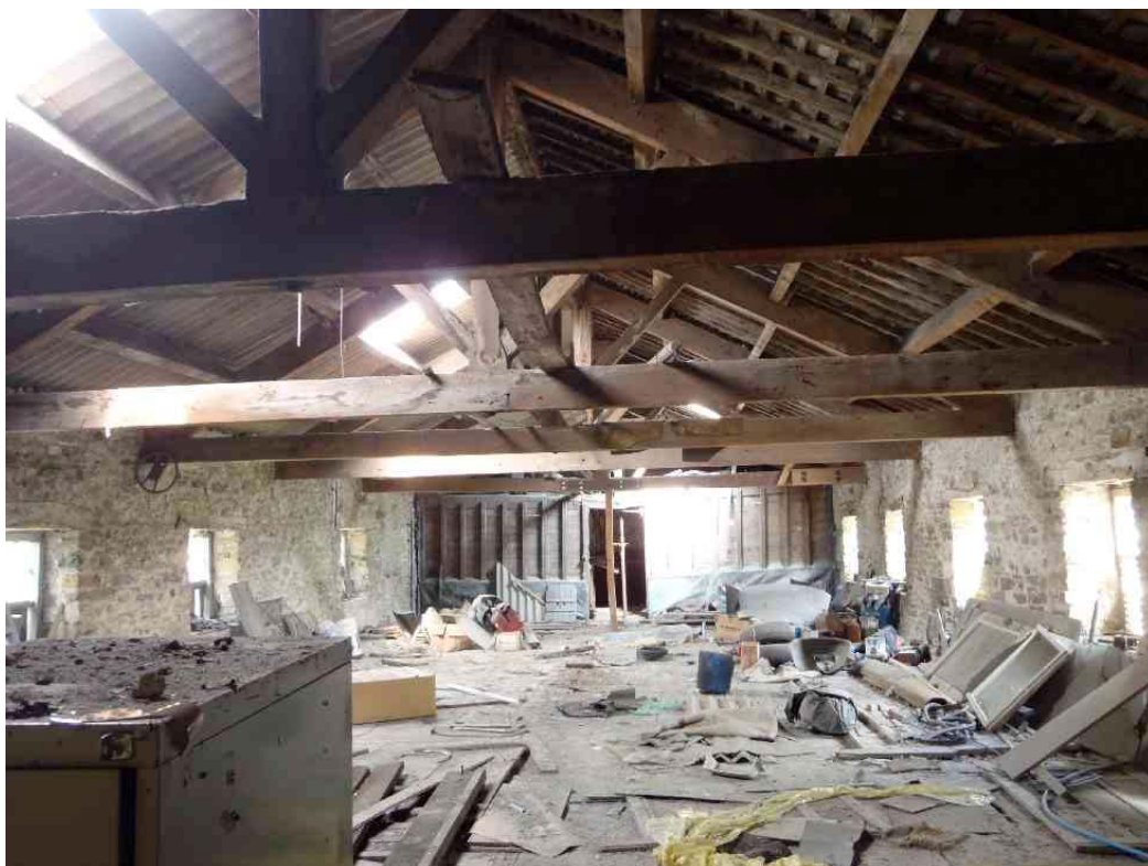
Plate 20: Second floor of the warehouse showing timber partition room at far end
