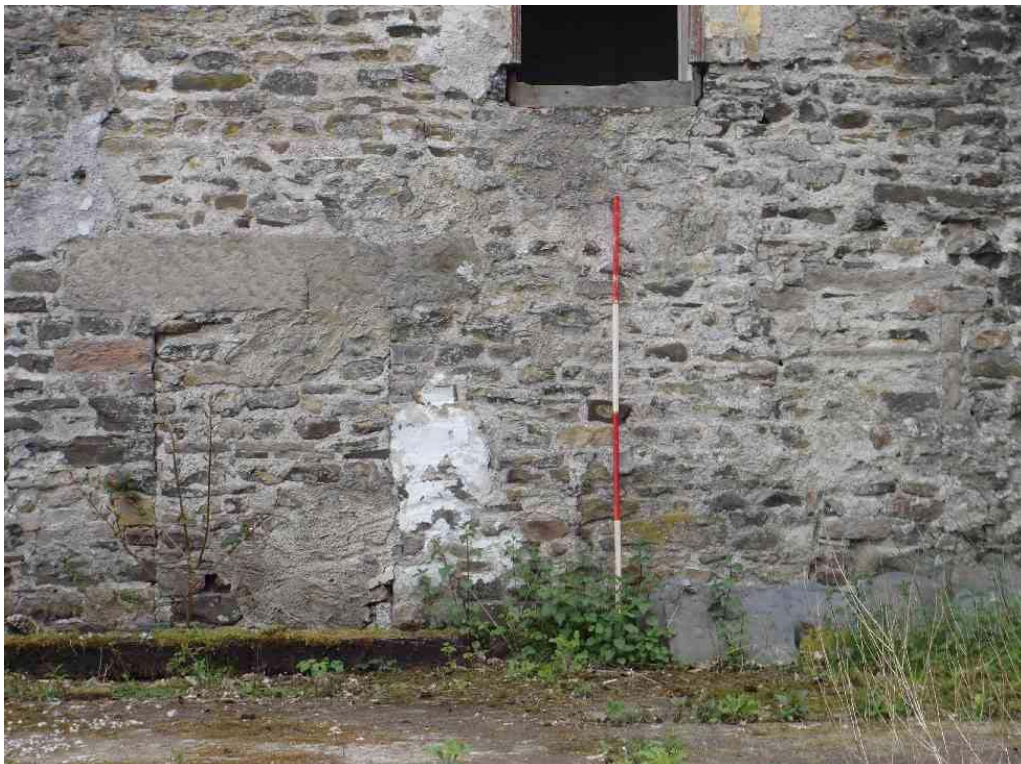
Plate 8: Blocked door and window within front elevation, with the entrance to self-contained first floor room just visible above
