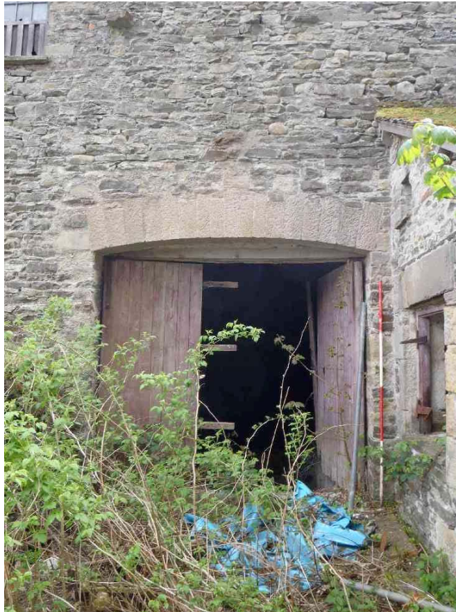
Plate 9: Segmental arch doorway into main first floor room, west end
