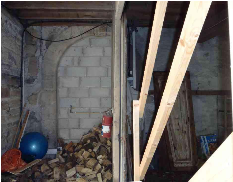
Plate 11: Blocked arch in the east elevation of the warehouse
