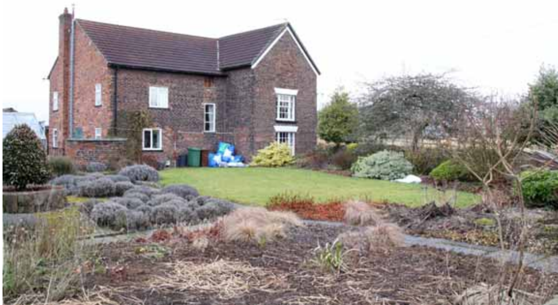
Plate 3: Rear view of farmhouse showing projecting wing with sash windows, new gable to the north-west
