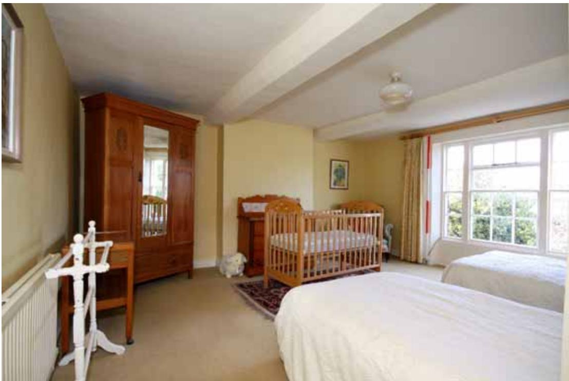
Plate 10: Second bedroom with large sash window and run-out stop chamfered beams
