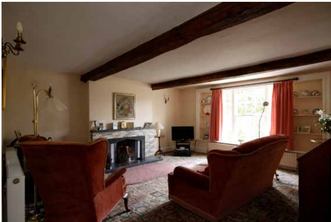
Plate 7: Living room showing sash window with wide decorative surround, and exposed beams
