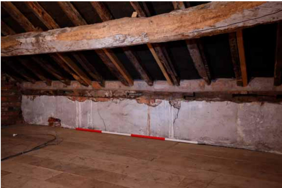
Plate 12: Detail of wall plate with edge-halved, scarf joints, and new brickwork above
