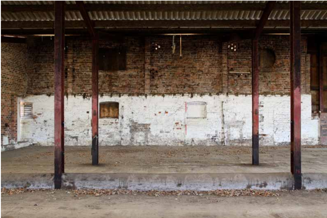
Plate 32: Internal elevation of Building 2 within Building 6, showing the sockets for the floor joists
