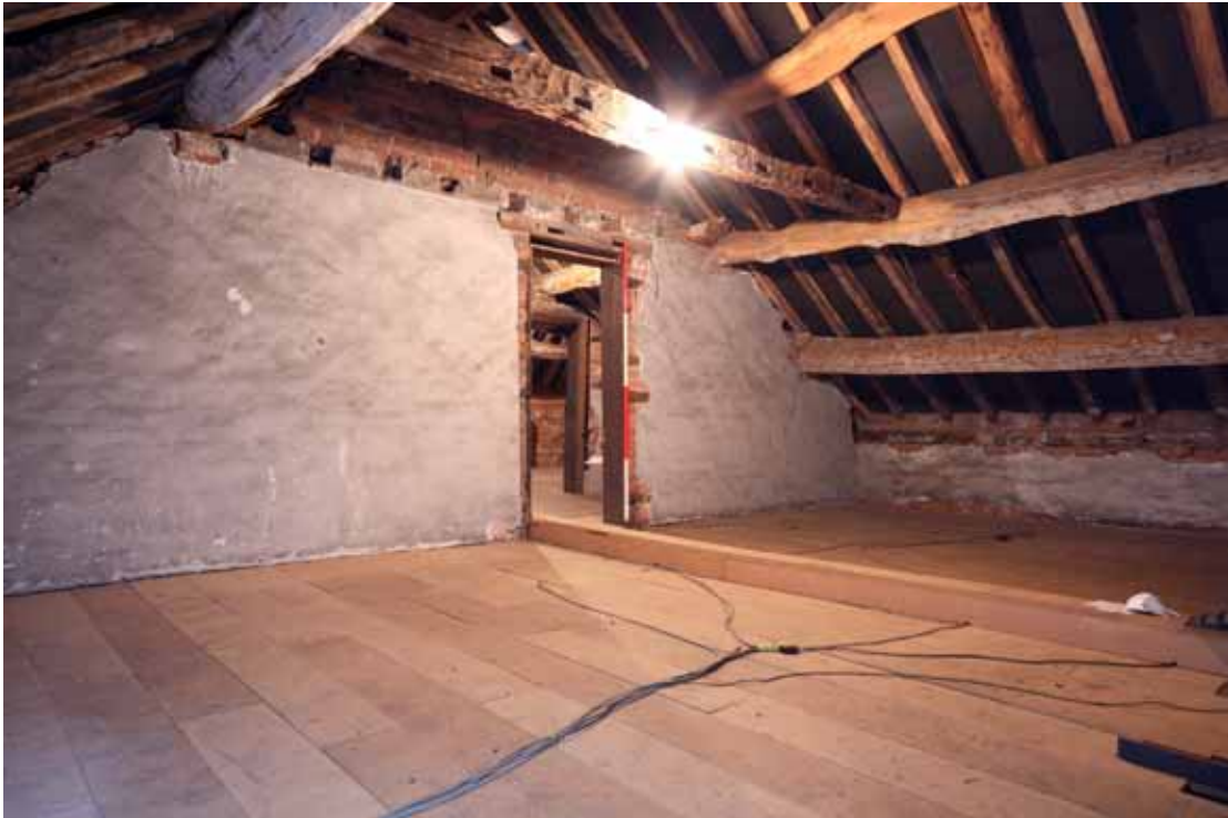
Plate 11: Attic space showing sockets for ceiling joists within the tie-beam and brickwork
