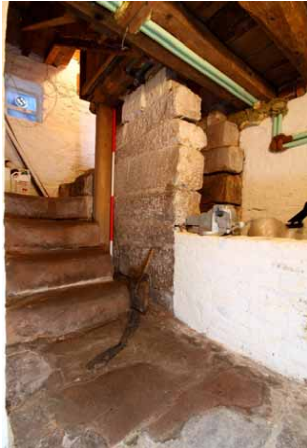
Plate 16: Detail of staircase in the cellar
