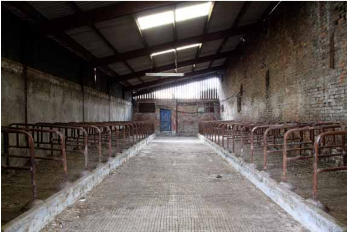
Plate 24: Rear wall of the barn (Building 1) with blocked doorway just evident
