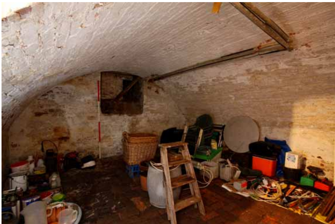
Plate 17: Cellar with coal chute in front wall
