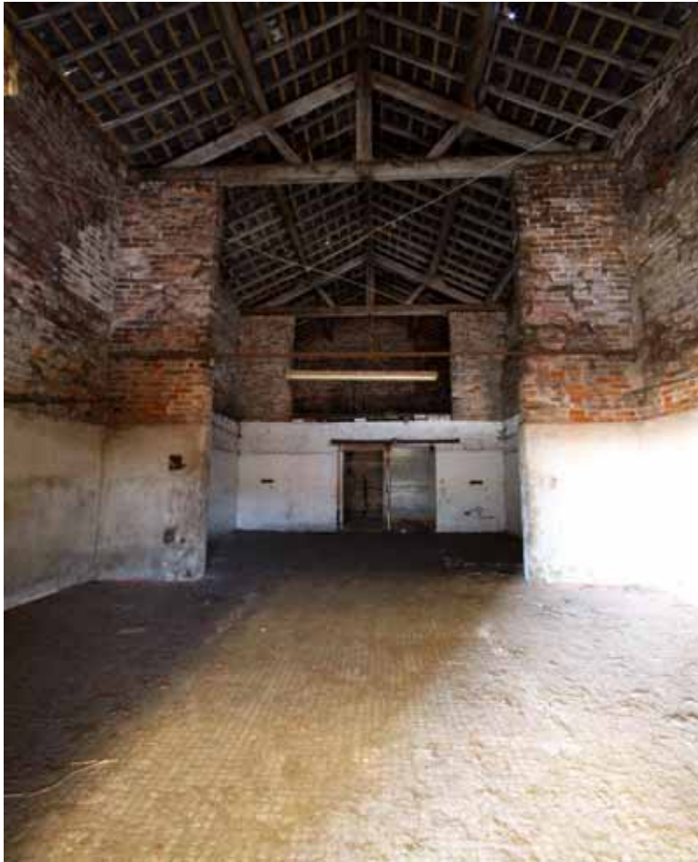
Plate 28: Open interior of the barn (Building 1) showing king-post trusses supported on brick buttresses
