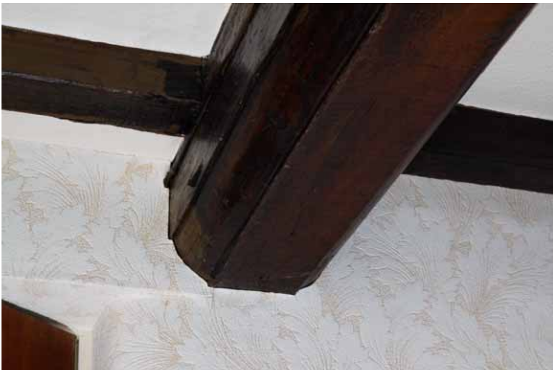
Plate 6: Detail of an ovolo-chamfered beam
