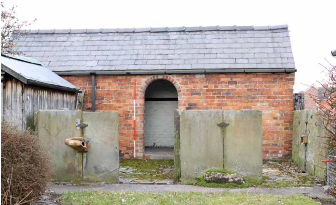
Plate 19: Pigsty with original ceramic feed hoppers in external pen walls
