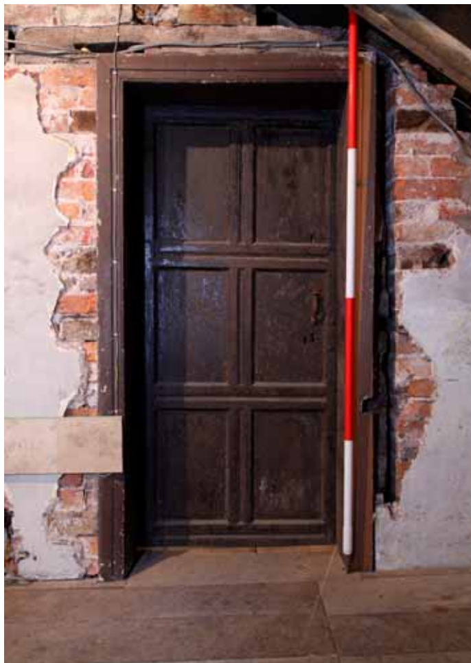
Plate 15: Detail of door in the attic
