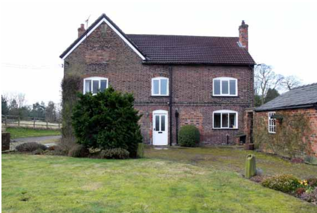
Plate 2: Front elevation of the farmhouse, one of the blocked doorways is evident, as is the blocked window at attic floor level, and the datestone
