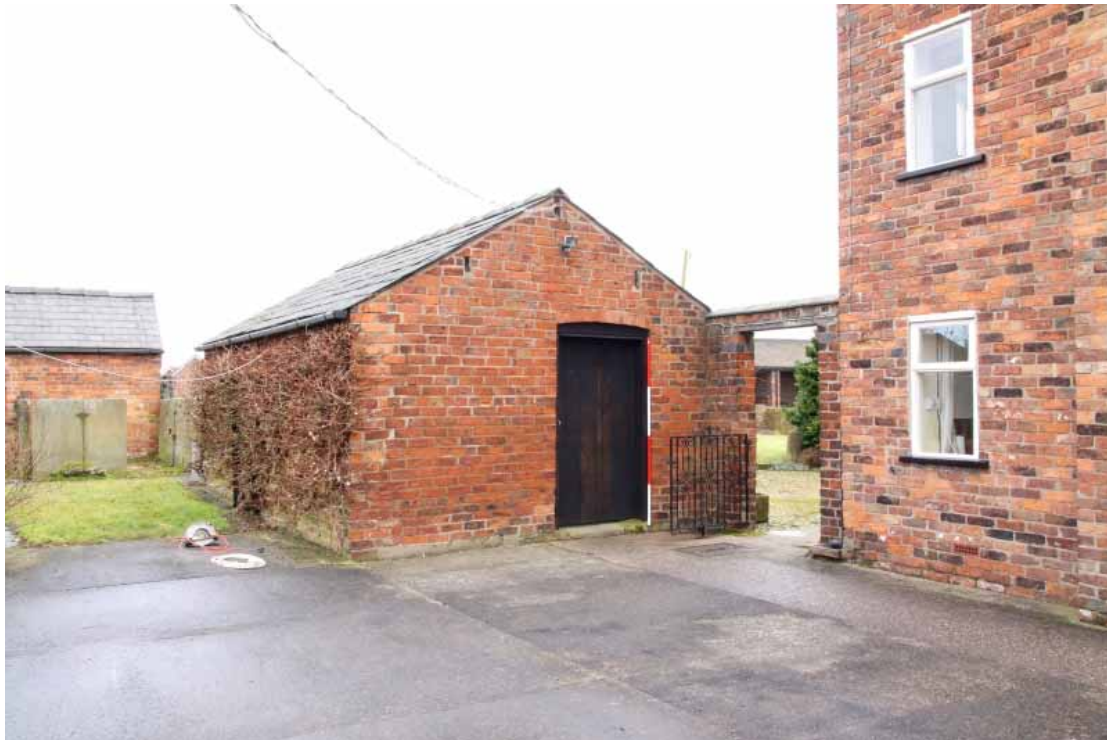
Plate 20: Garage with roof purlins evident in elevation
