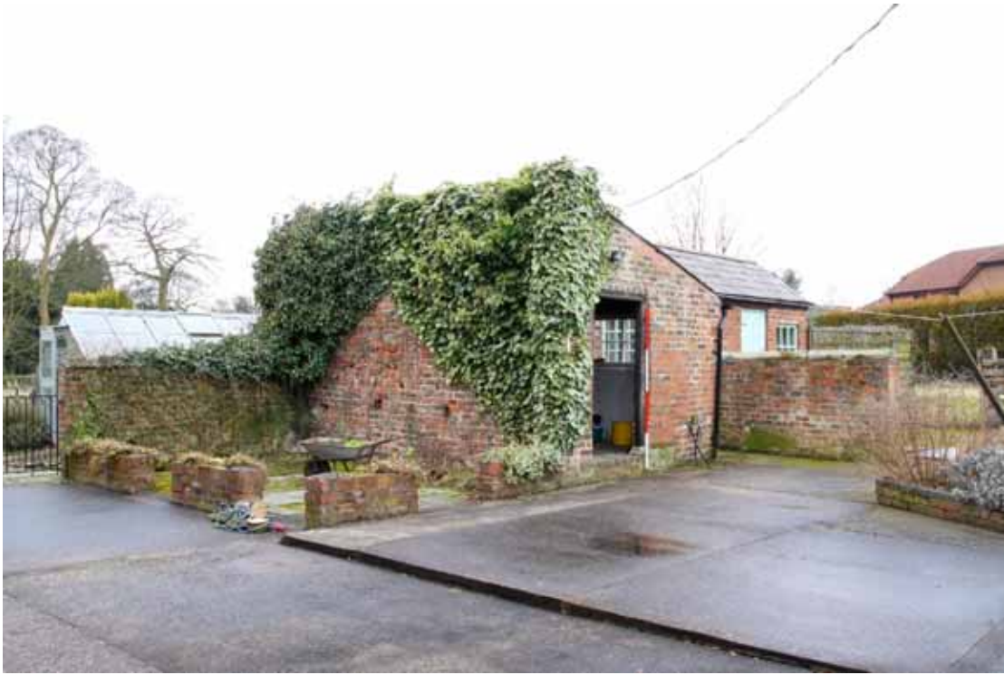
Plate 18: The brick outbuilding formerly attached to the farmhouse
