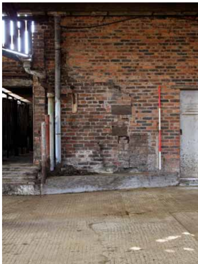
Plate 31: Rear elevation of Building 4, showing the short section of Building 2, and the sandstone pads for an original door jamb
