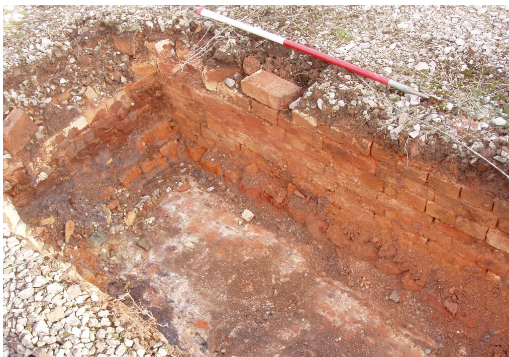
Plate 4: Northern end of TP 101, showing the brick walling (top), stacked brick mass (left) and underlying concrete layer
