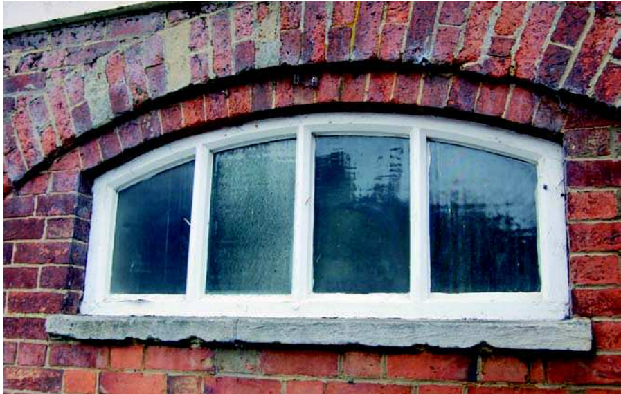
Plate 5: Window in north elevation
