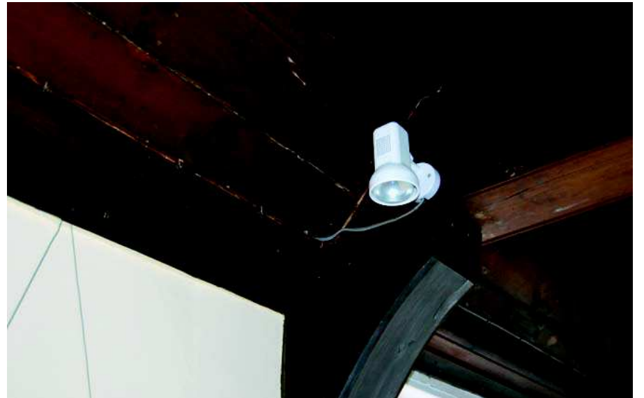
Plate 24: Detail on corbel in roof structure
