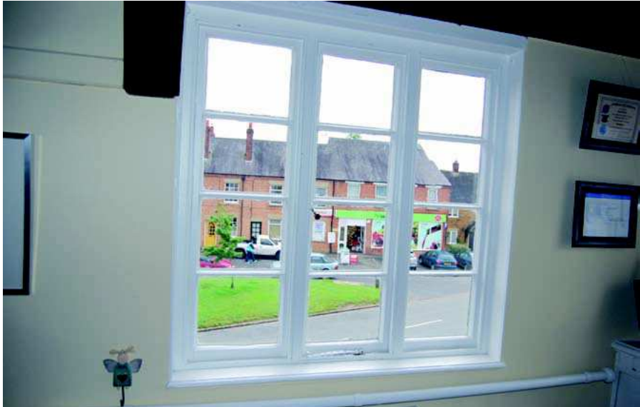
Plate 21: Window in east wall
