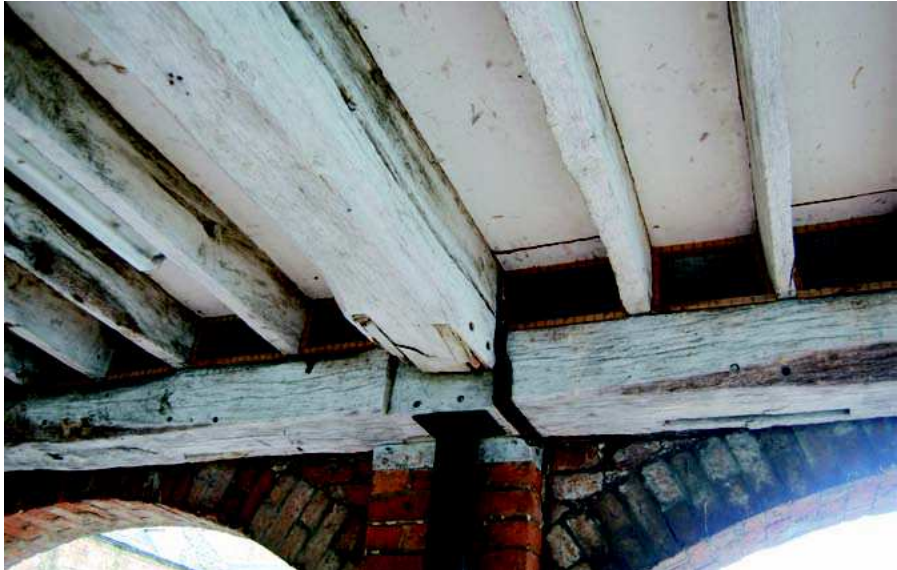
Plate 9: Details in underside of first floor
