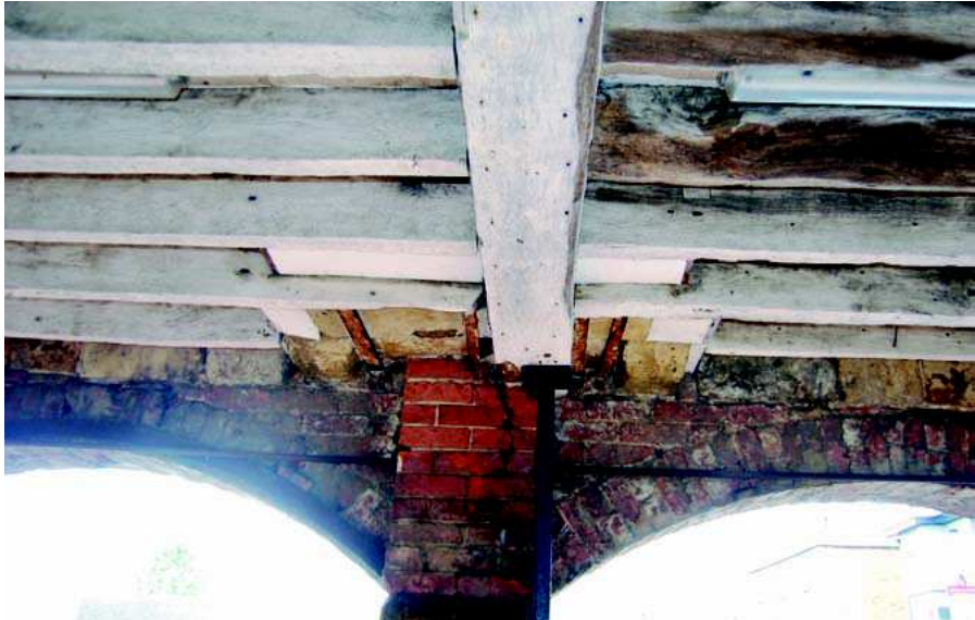
Plate 13: Underside of hearth in south wall
