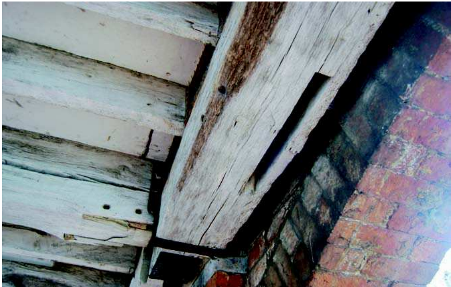
Plate 11: Empty mortice in underside of first floor
