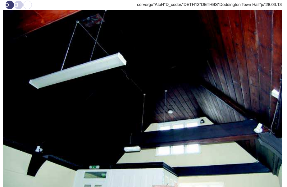
Plate 22: General view of roof
