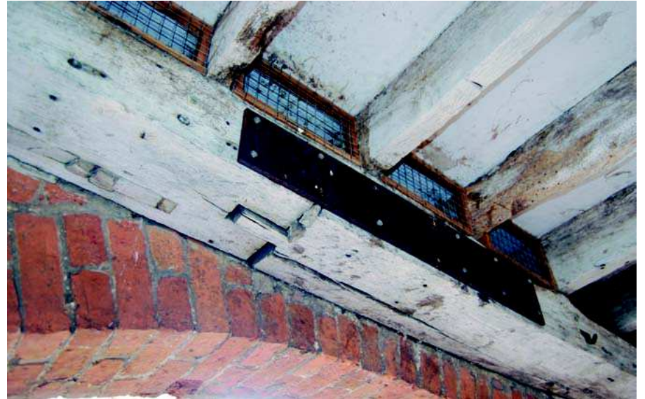
Plate 10: Scarf joint and metal strengthening in first floor
