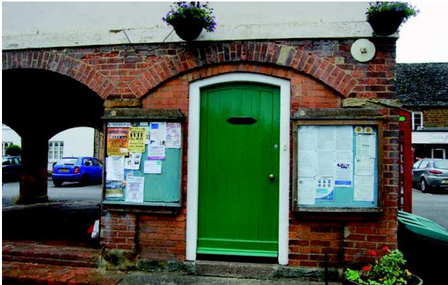
Plate 7: Door in east elevation
