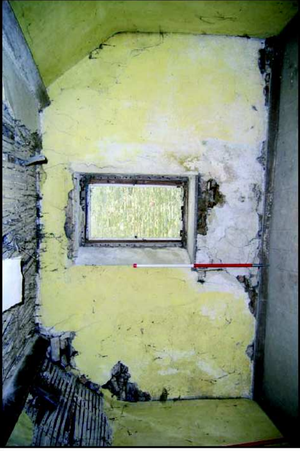
Plate 30: Attic, South gable end, looking south
