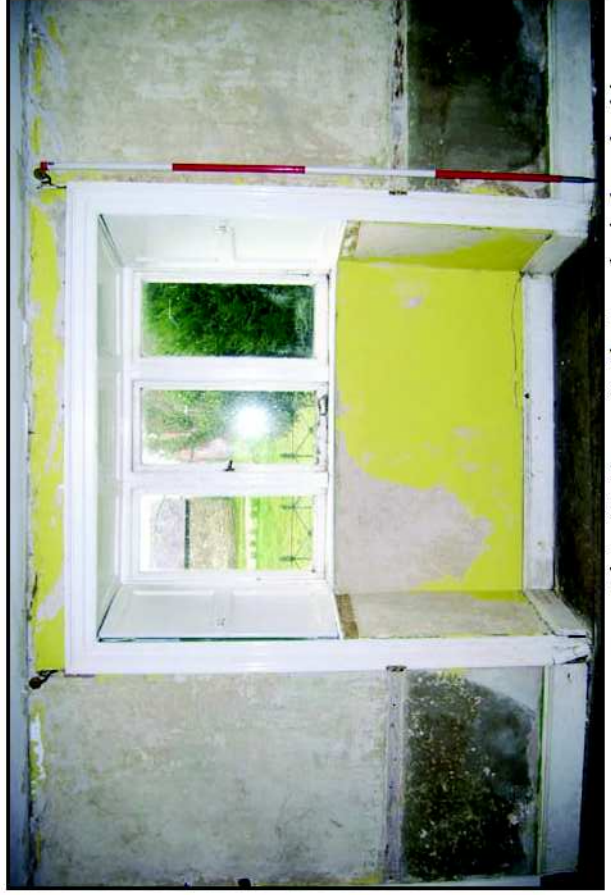
Plate 19: Room 8, Shuttered window, looking west
