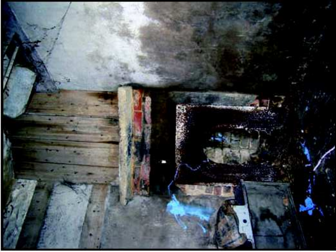
Plate 33: Outbuildings, Fire place in outbuilding, looking north east
