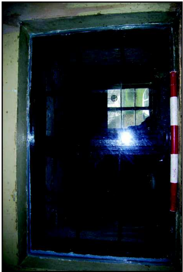
Plate 15: Room 5, Internal casement window, looking west
