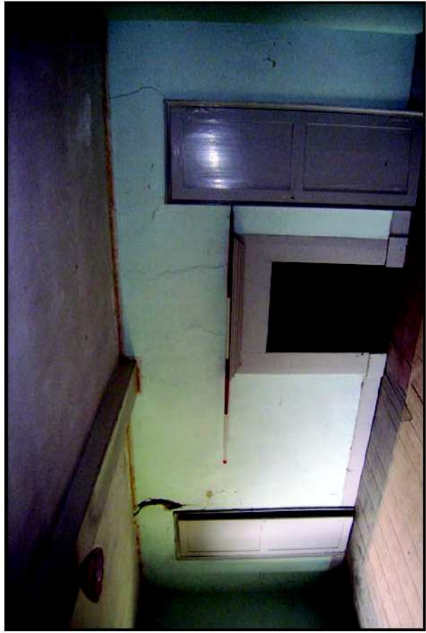
Plate 27: Room 14, North wall, looking north west
