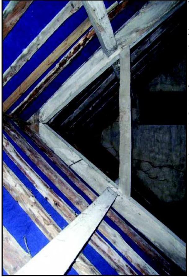
Plate 31: Attic, Roof structure, looking north
