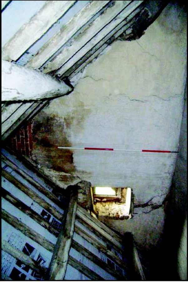
Plate 29: Attic, North gable end, looking north
