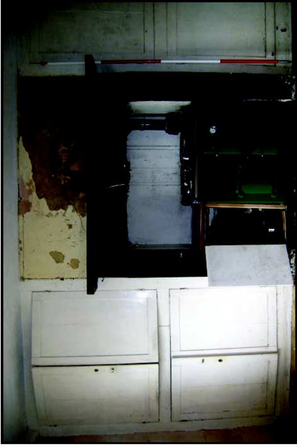
Plate 14: Room 5, South wall
