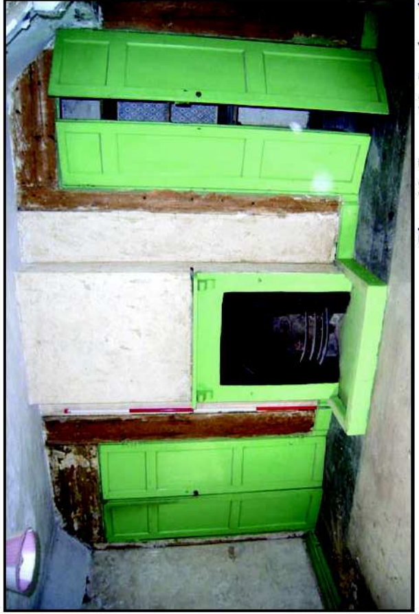
Plate 23: Room 10, South wall
