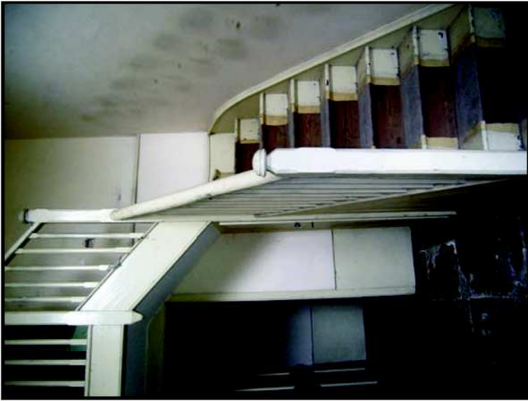
Plate 21: Hallway, Stairs, looking south east
