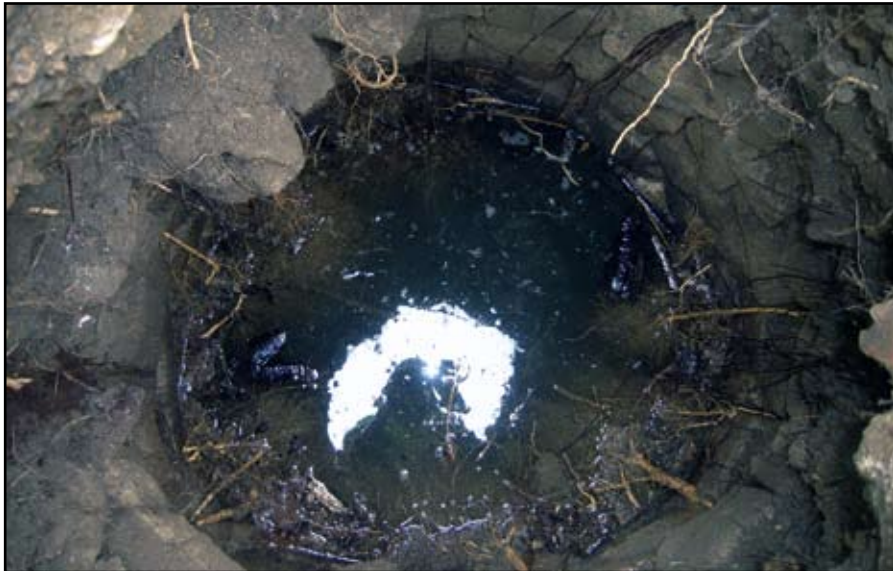
Plate 7: Close-up view showing walls of well
