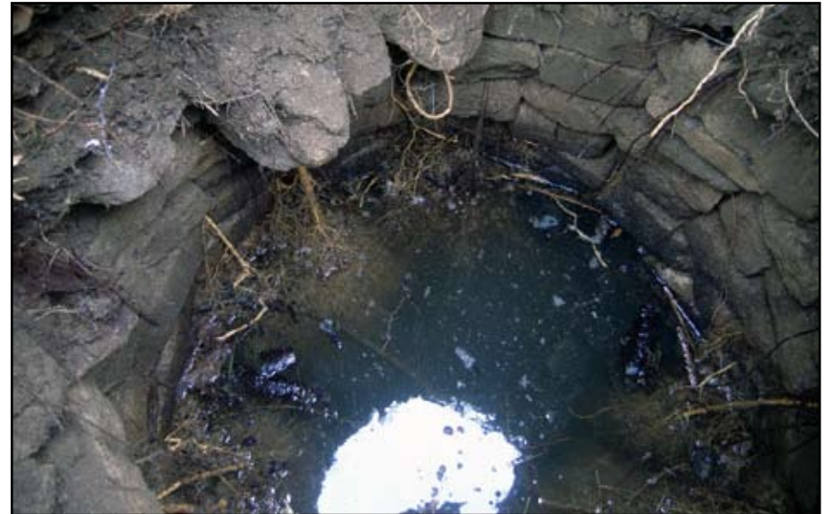
Plate 8: Close-up view showing walls of well
