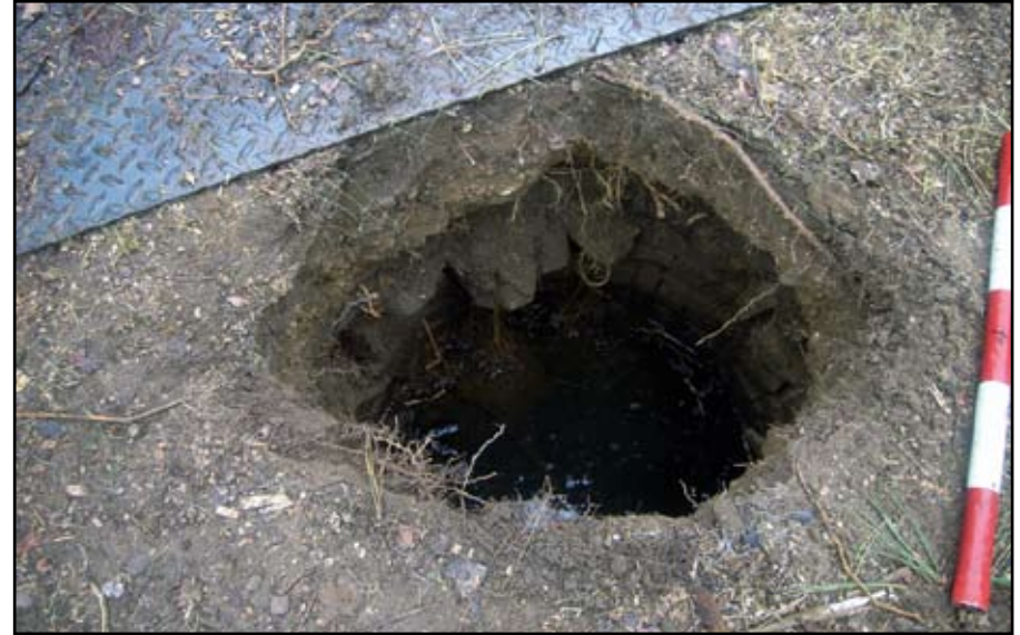
Plate 6: Hole in ground surface showing exposed well
