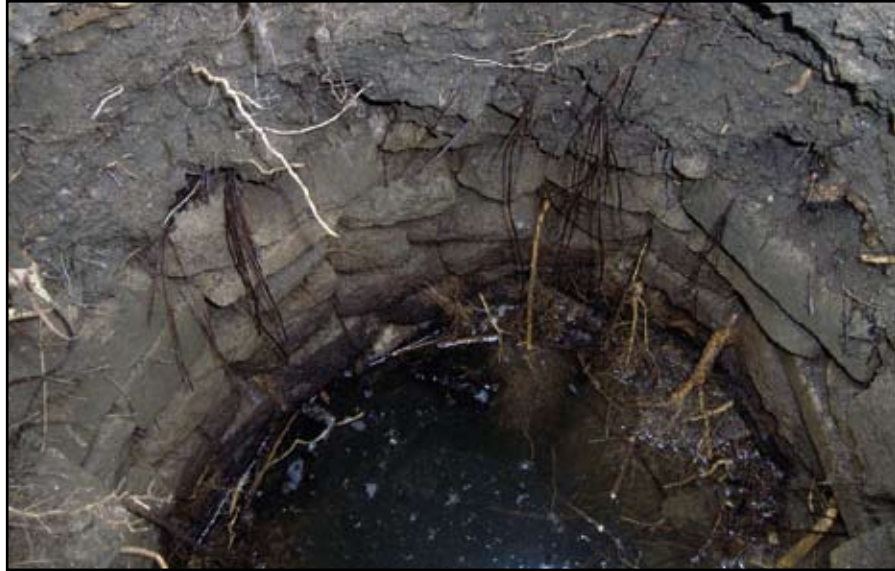
Plate 9: Close-up view showing walls of well
