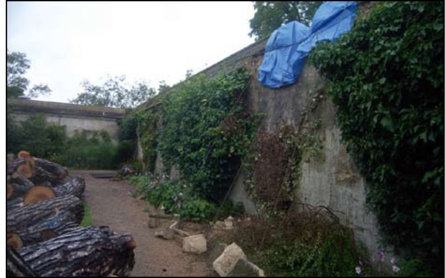
Plate 2: Wall showing damaged area where tree collapsed
