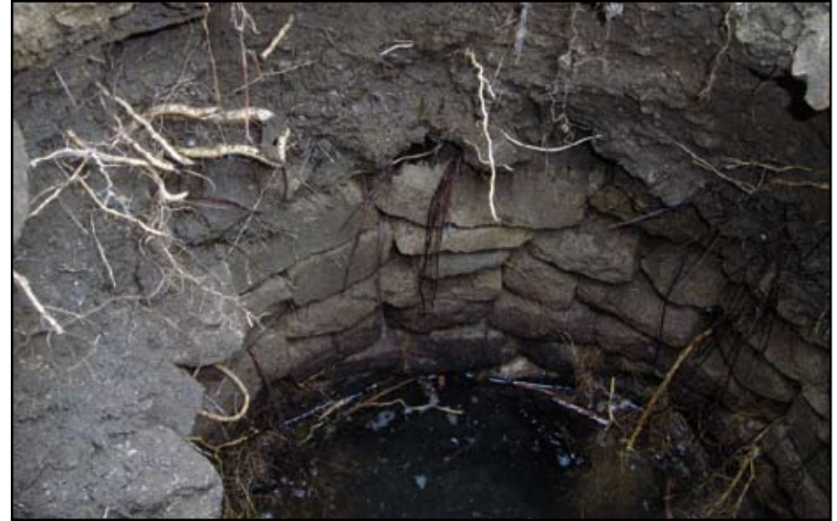
Plate 10: Close-up view showing walls of well
