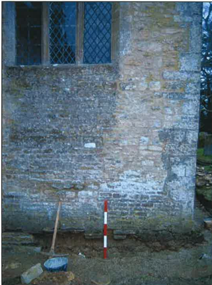
Plate 6: External view of blocked doorway?
