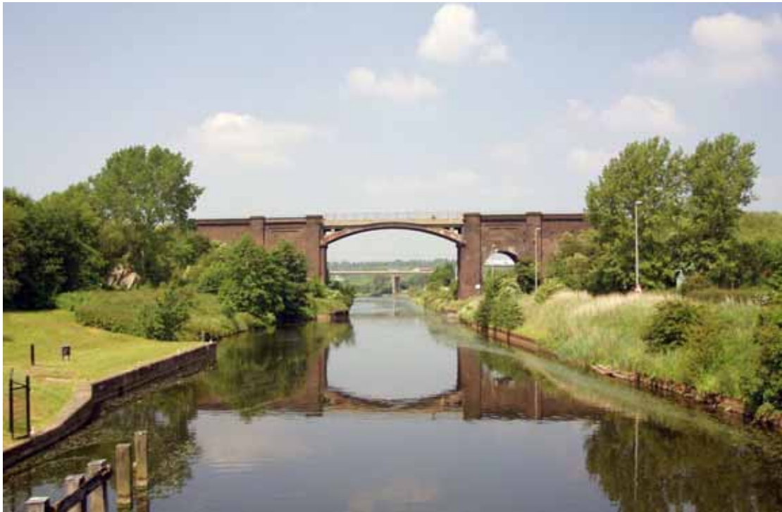
Plate 1: Frodsham viaducts 53 and 54 (Site 1 ) facing north-west
