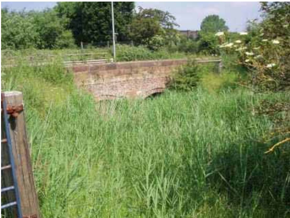
Plate 6: Sutton Bridge (Site 24 ) facing north-west
