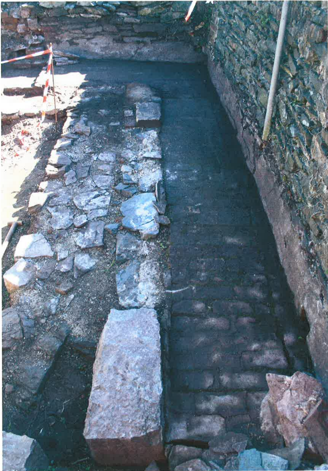
Plate 10: Southern side of the stack, showing walkway and additional single-skin wall
