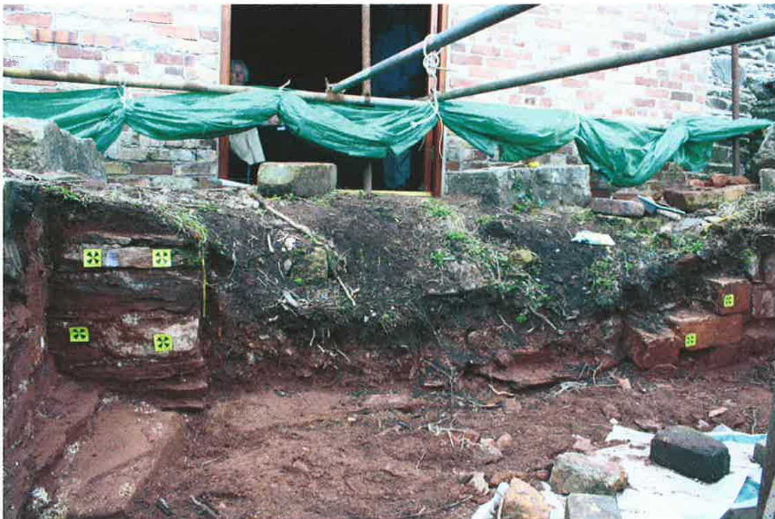
Plate 4: Doorway in western elevation, providing access to charging house
