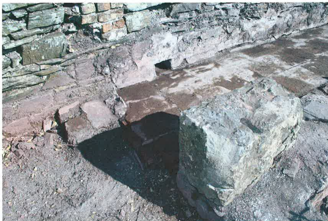
Plate 9: North-western corner of the walkway, showing the projecting quoin and drain hole in the parapet wall
