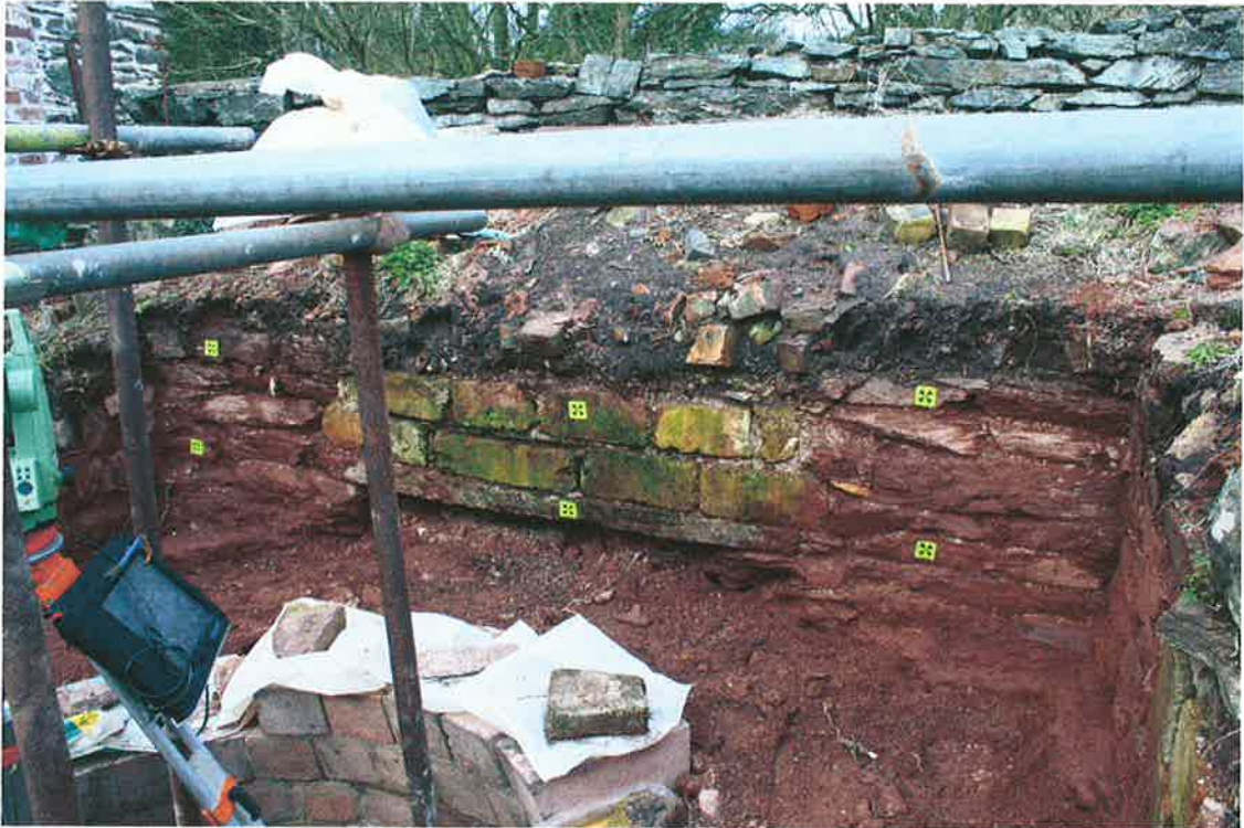
Plate 1: North elevation of the furnace stack, showing the overburden atop the wall
