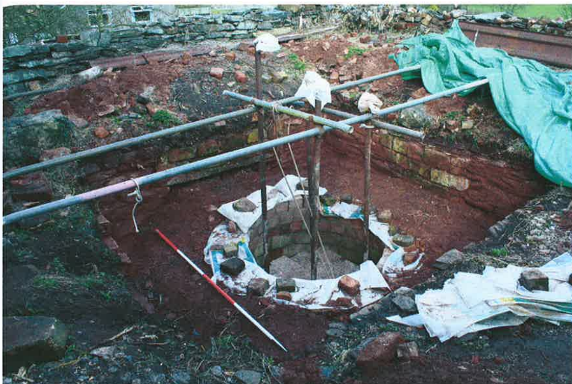
Plate 6: View across the top of the furnace in April 2007, showing iron lintel in the north elevation of the stack wall
