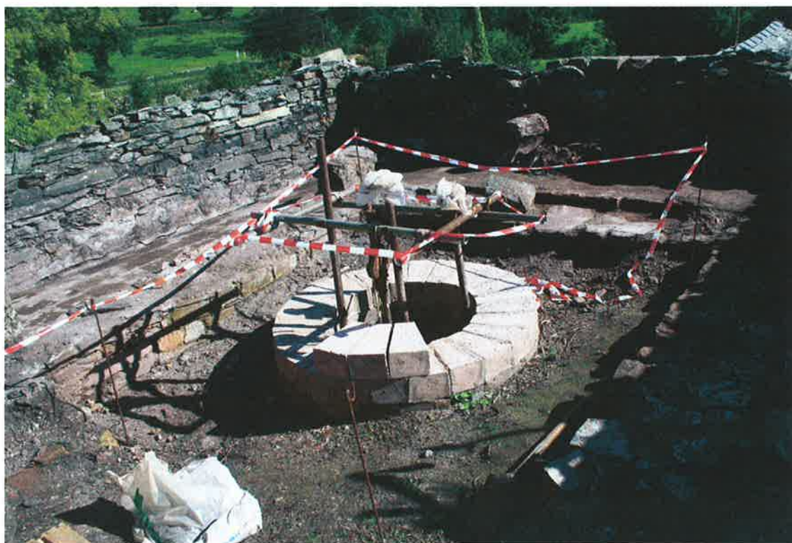
Plate 7: View looking north across the top of the furnace in September 2007, following the removal of overburden from the walkway
