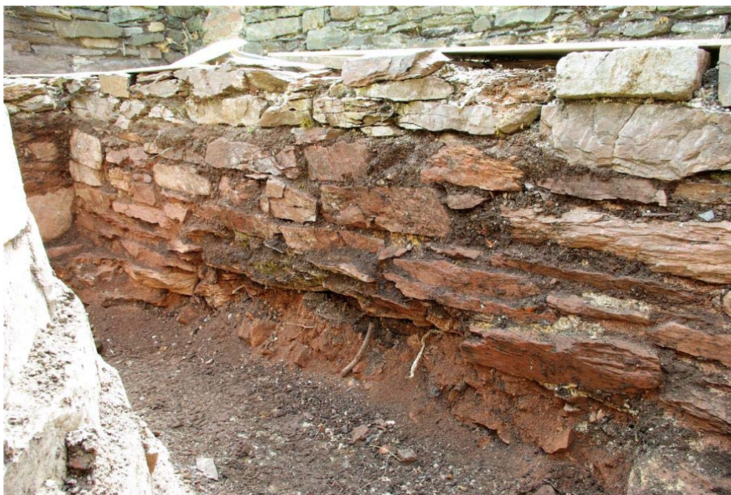
Plate 6: Aperture in the south elevation (Elevation 3) of the interior of the stack wall
