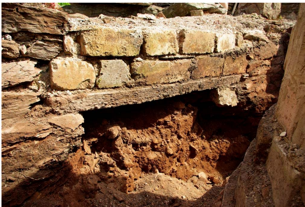
Plate 3: Aperture in the north elevation (Elevation 1) of the interior of the stack wall showing collapsed material
