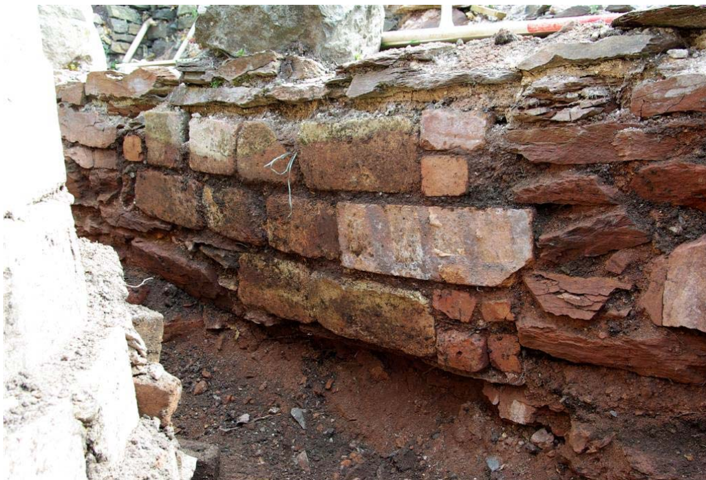
Plate 5: Aperture in the east elevation (Elevation 2) of the interior of the stack wall
