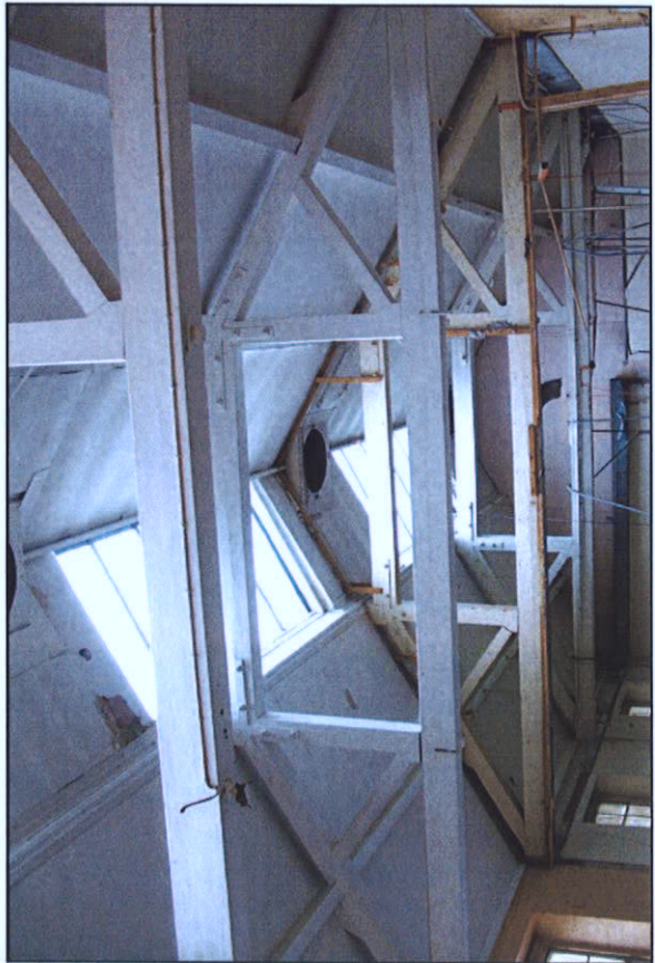
Plate 51: Laundry, Queen post roof trusses looking south east.
