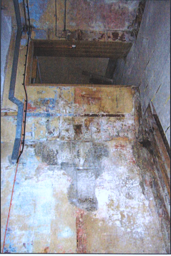
Plate 6: Block 1, Interior of west extension, looking south east.
