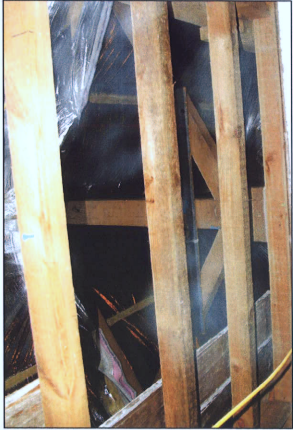
Plate 35: Block 5, primary king post truss and secondary ceiling joists.
