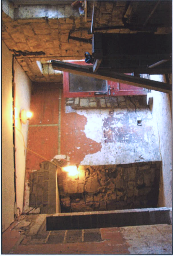
Plate 8: Block 1, ground floor room of south east extension.
