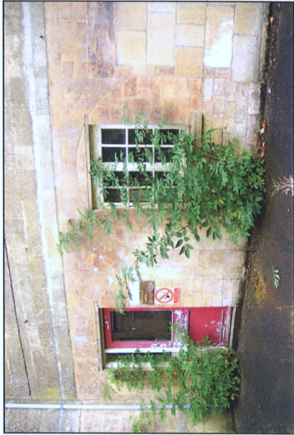
Plate 27: Block 4, blocked arches in west wall.
