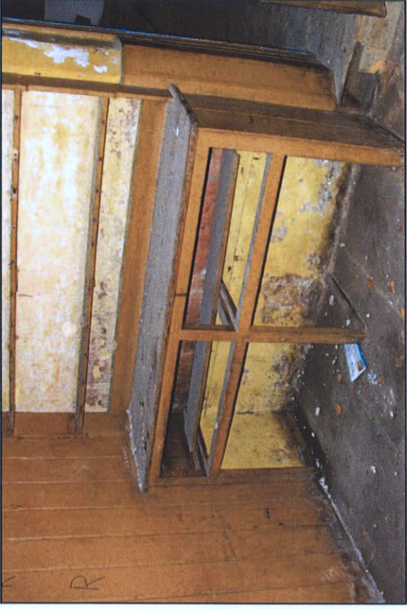
Plate 14: Block 2, fitted cupboard in ground floor room looking south.
