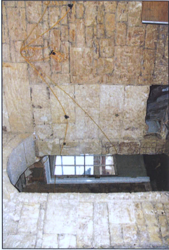
Plate 7: Block 1, arch and blocked doorway in central room after stripping out.
