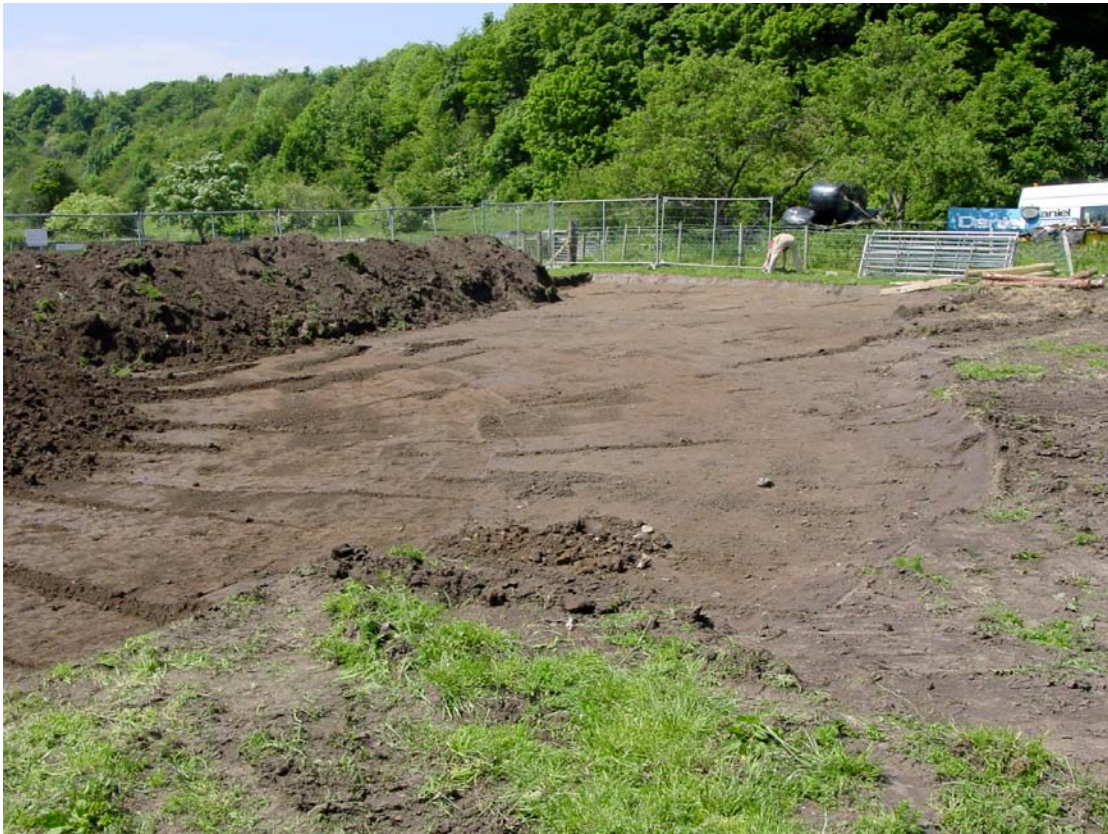
Plate 1: Area of Topsoil stripping
