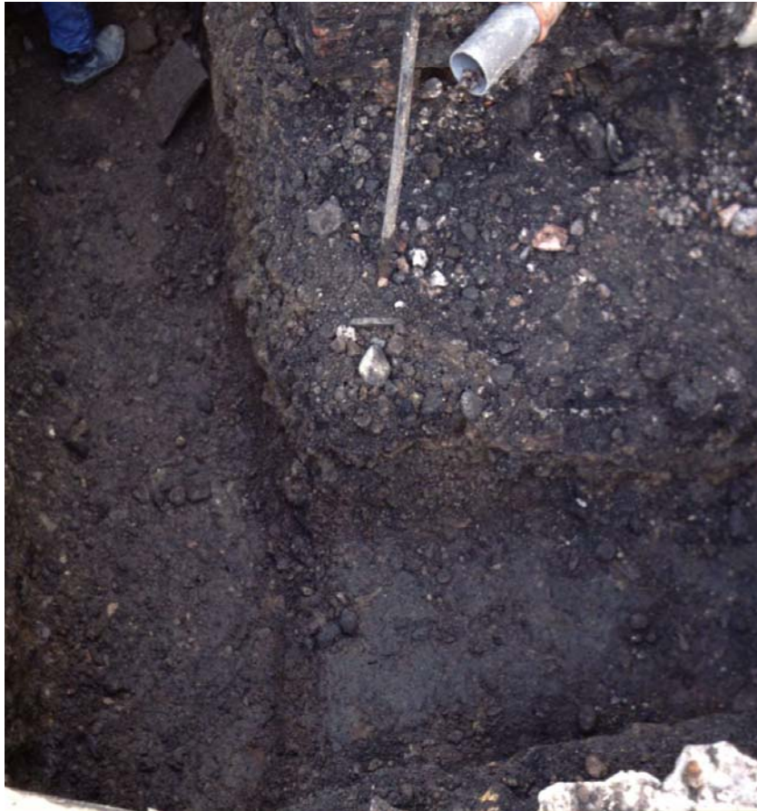
Plare3: Plan shot of excavated footing trench
