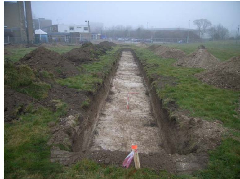
Plate 2: Trench 2 looking NW (1x2m and 1x1m scale)
