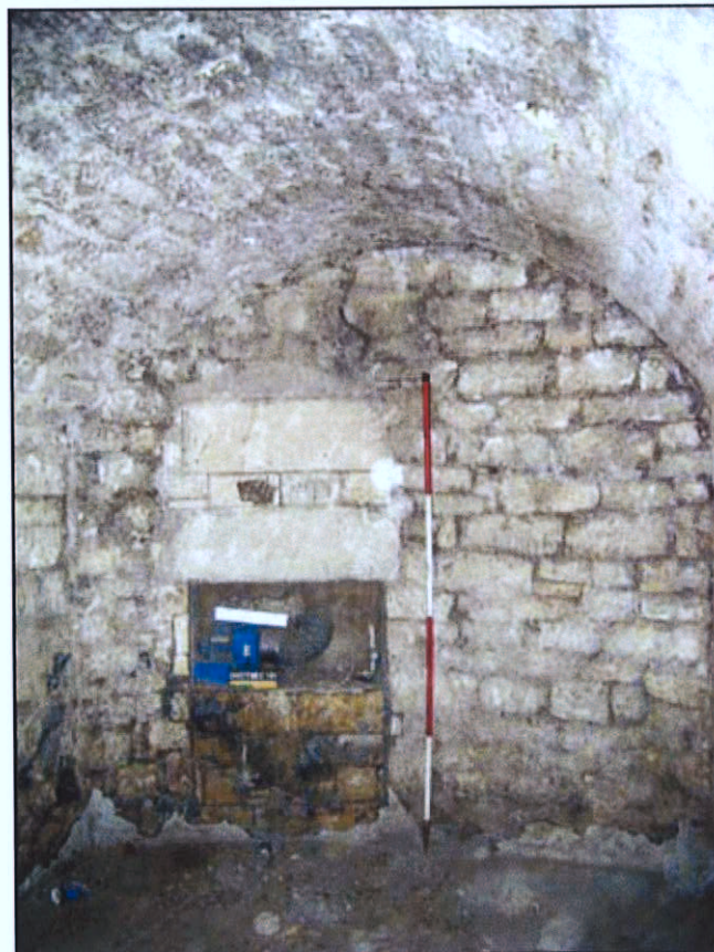
Plate 11: Octagon Vault Room 6 Blocked Fireplace (154)
