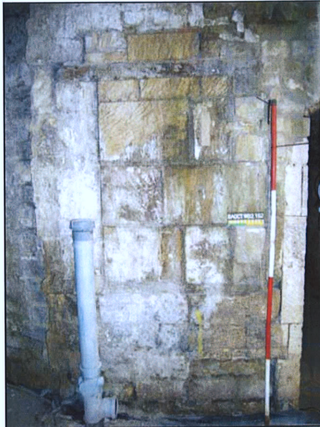
Plate 10: Octagon Vault Room 5 Blocked Window (152)
