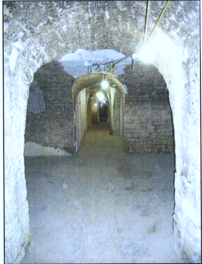
Plate 6: Octagon Vaults corridor and Tramway (123) looking towards Milsom Street
