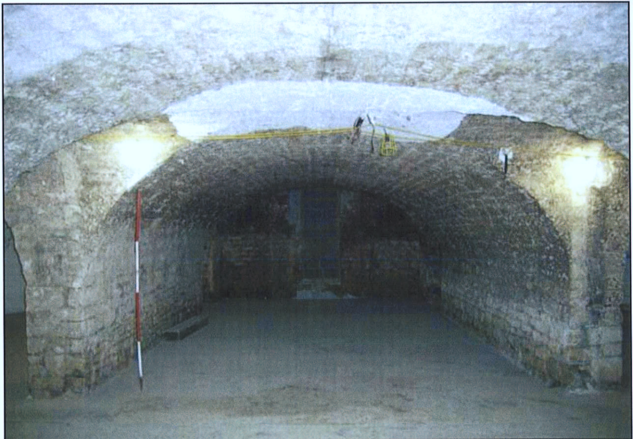
Plate 7: Octagon Vault Room 3 looking north-west
