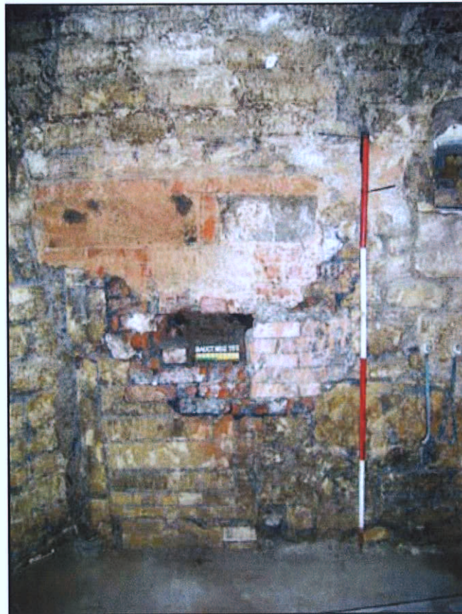
Plate 9: Octagon Vault Room 5 Blocked Fireplace (155)
