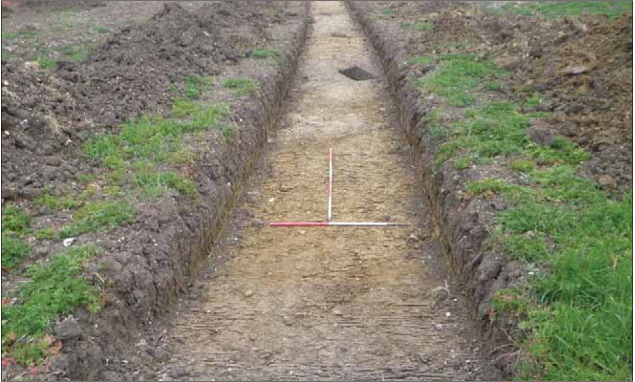
Plate 7: Trench 11, view from south-east
