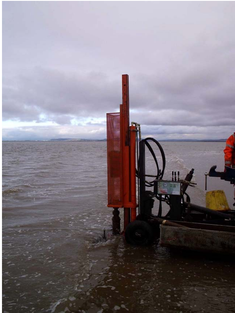
Plate 2: Working Shot of mechanical corer at Heysham
