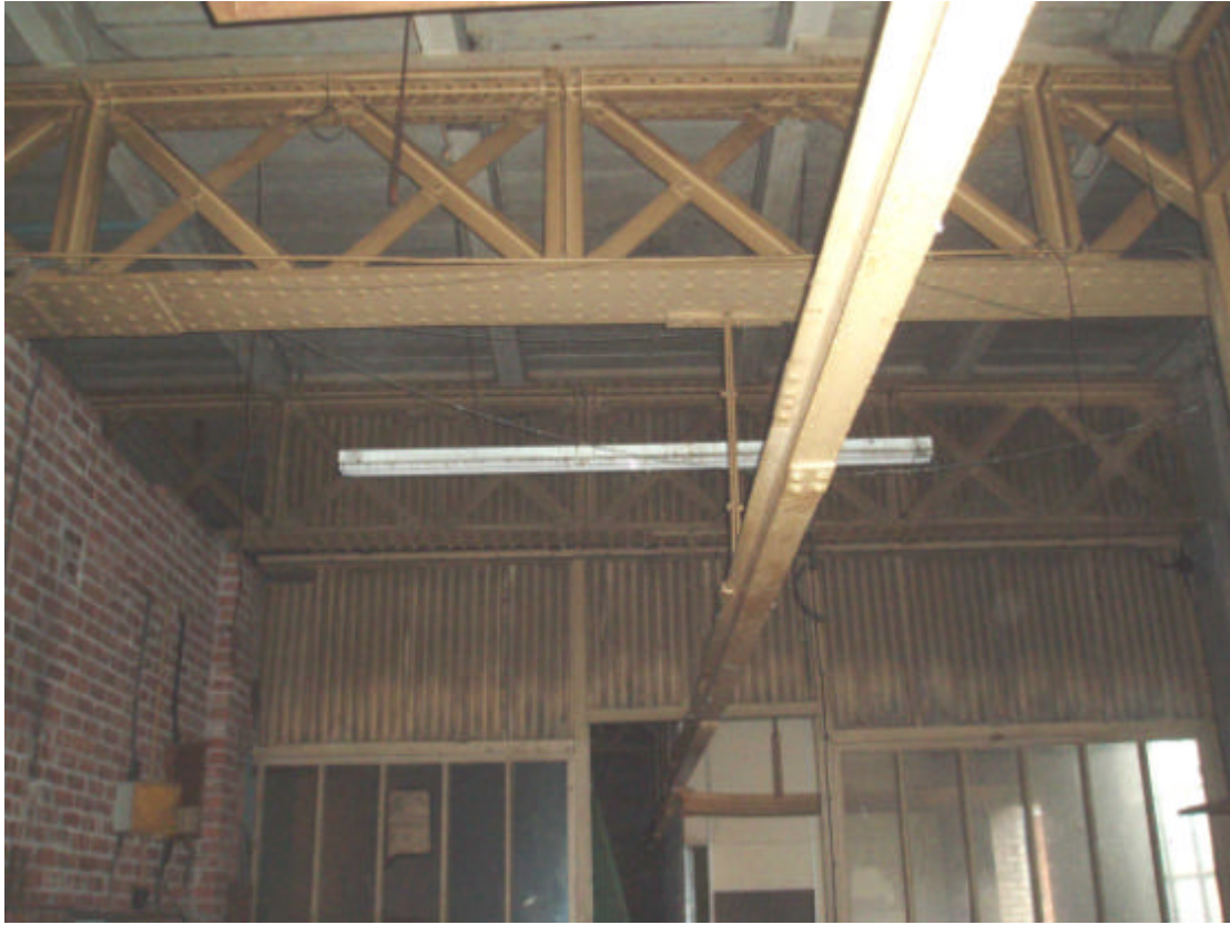
Plate 7: Girder rails running below ceiling of ground floor in Building 5, looking south
