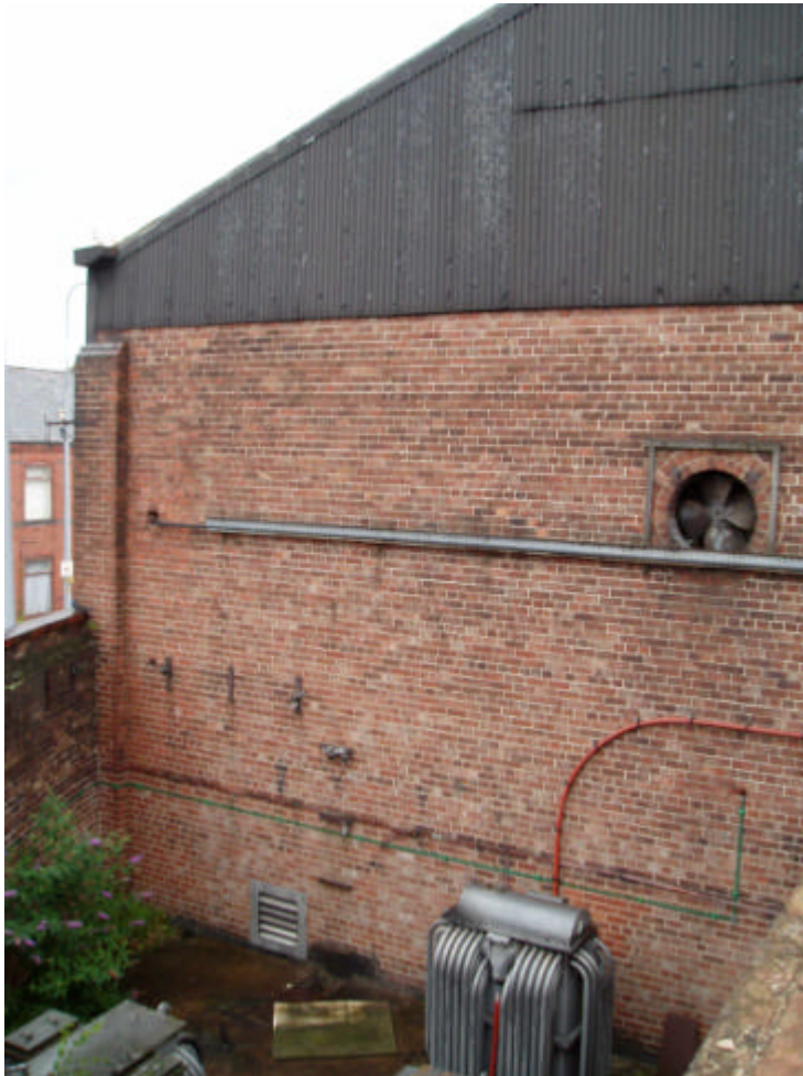
Plate 44: West elevation of Building 8
