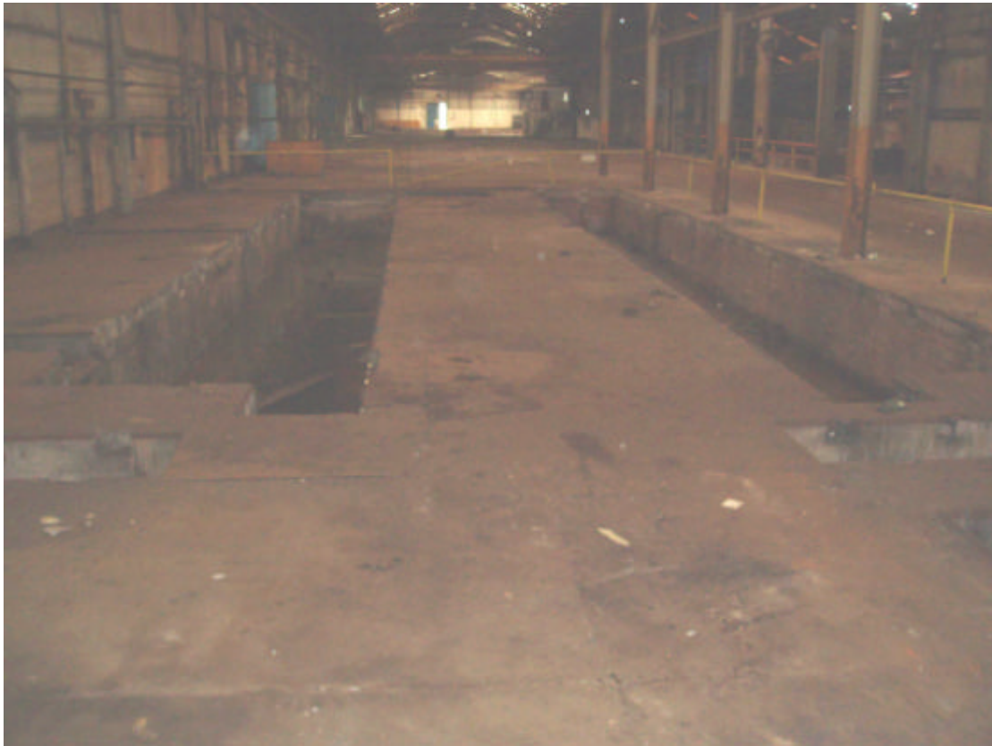
Plate 33: Concrete tanks in Building 7
