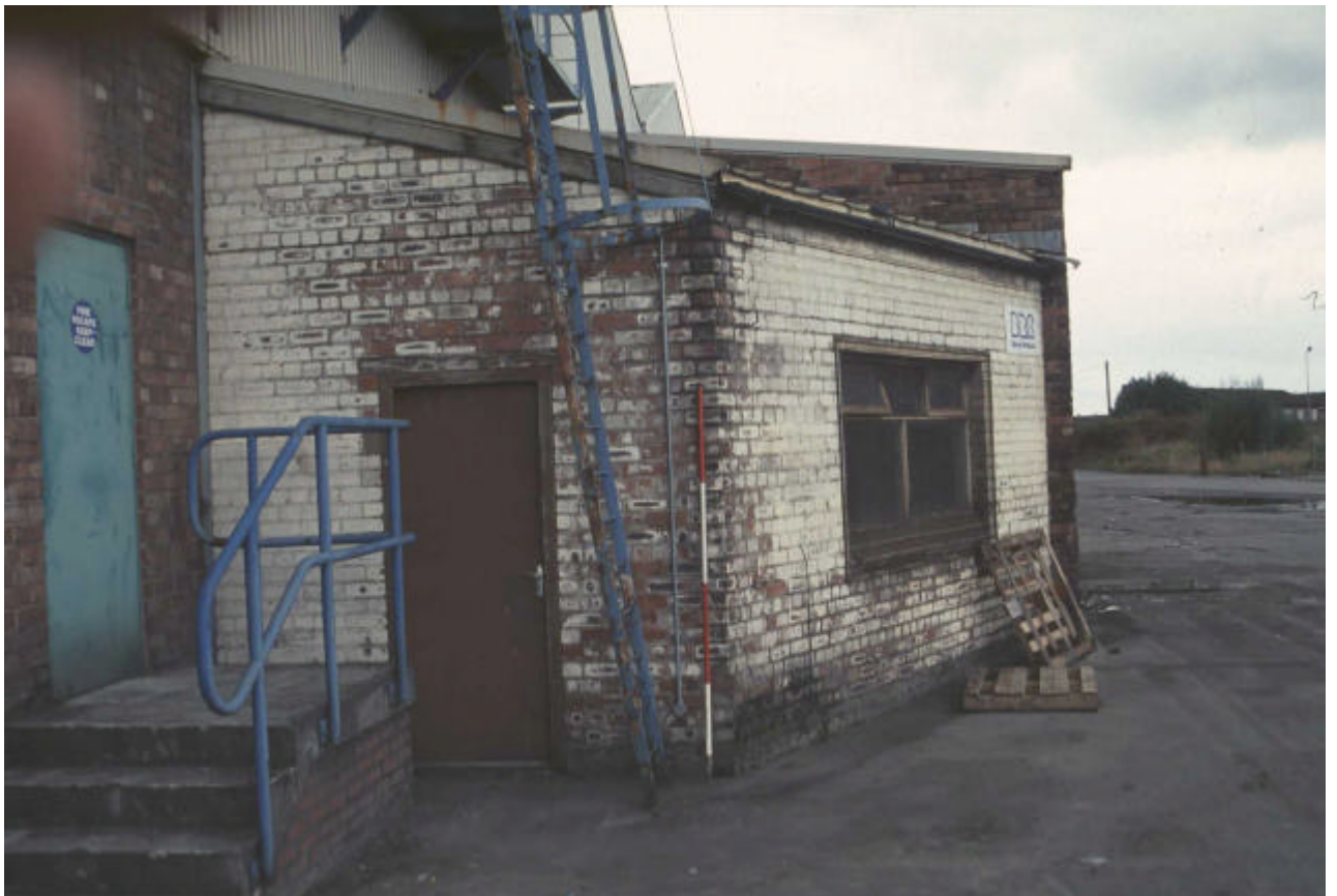
Plate 26: General view of Building 13, looking north
