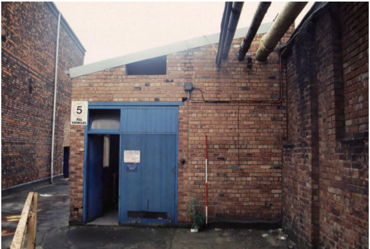
Plate 38: North elevation of Building 4
