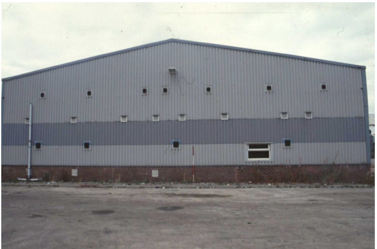
Plate 40: South elevation of Building 10
