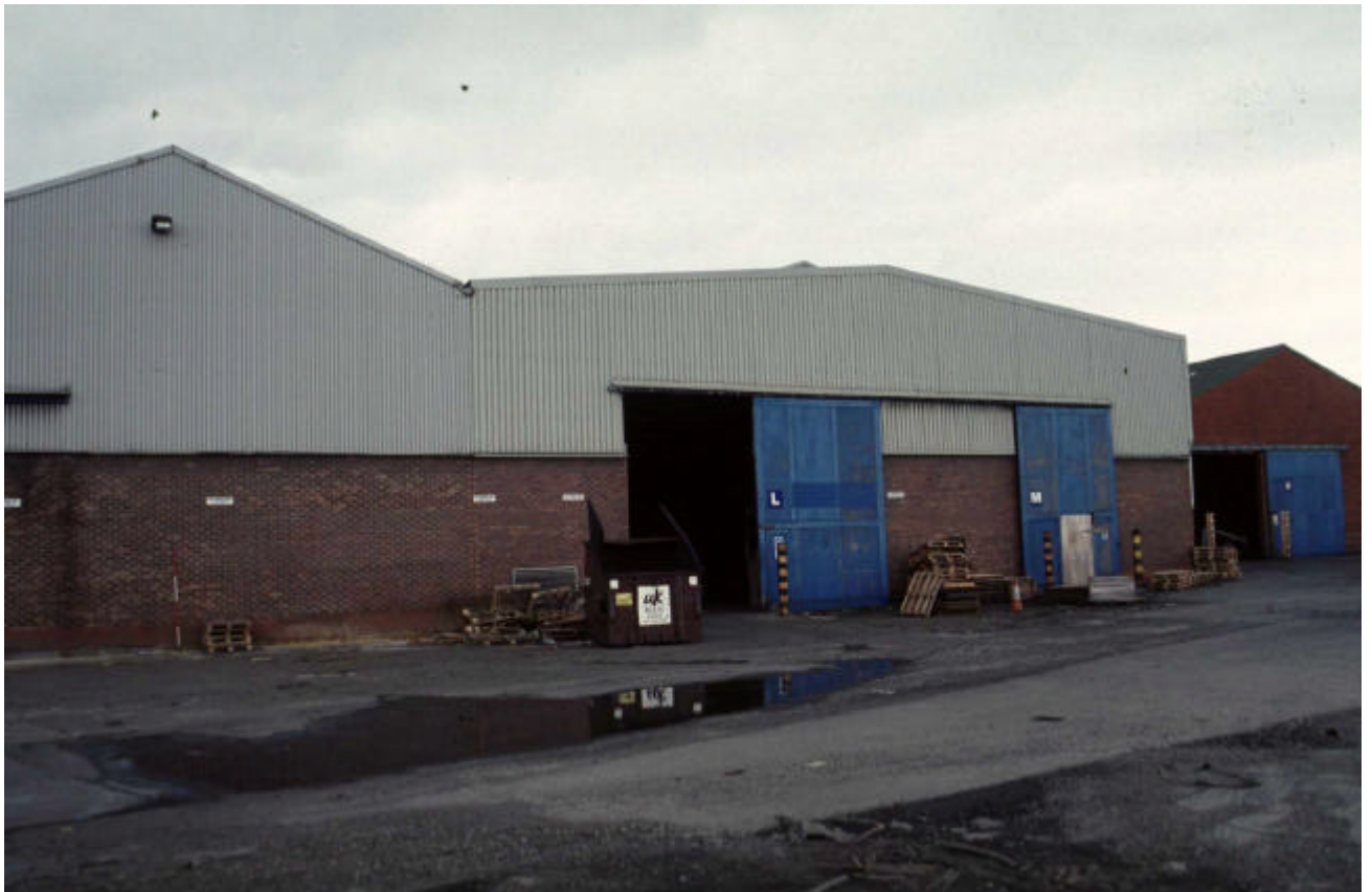
Plate 24: East elevation of Buildings 7 and 8
