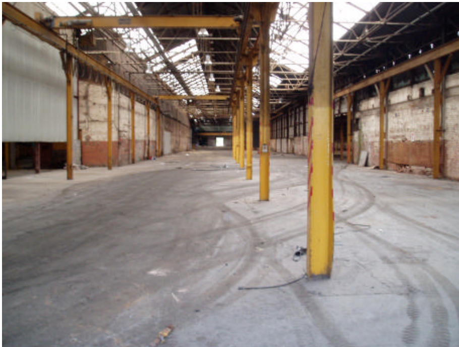
Plate 20: Interior of Building 7, looking east
