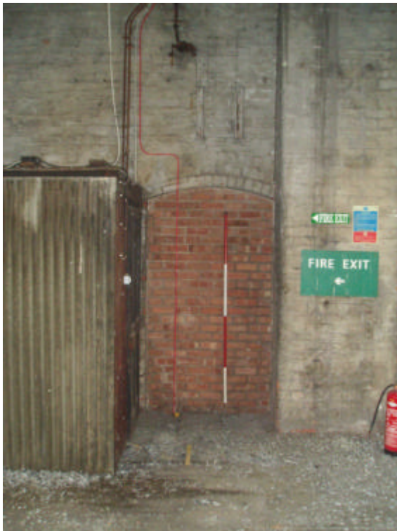
Plate 14: Blocked window within the east wall of Building 5
