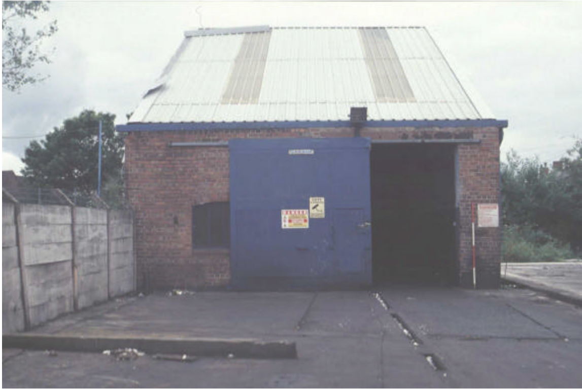
Plate 41: East elevation of Building 11
