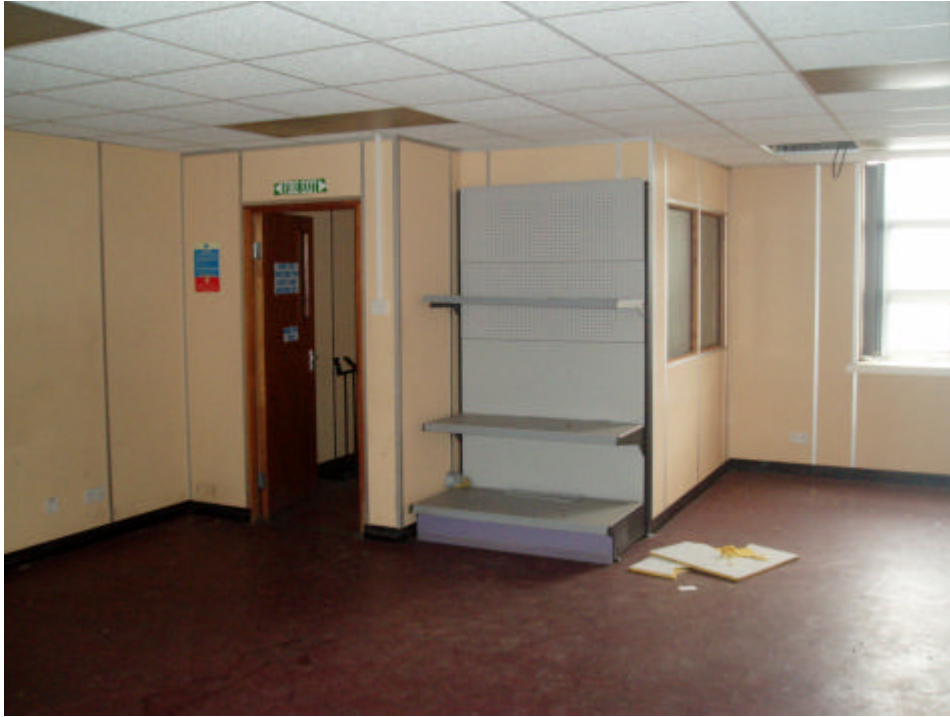
Plate 15: Office within the west end of Building 5
