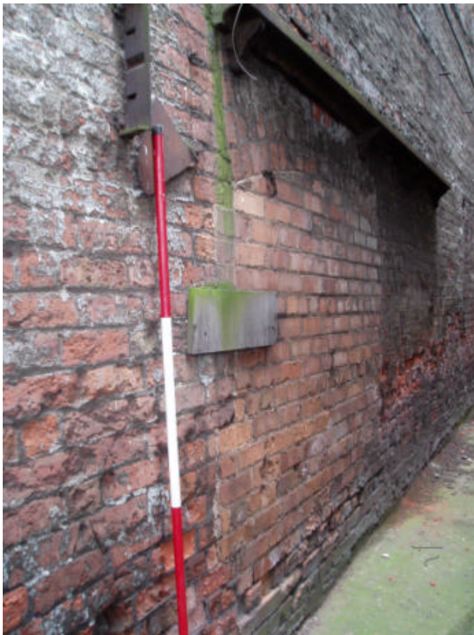
Plate 16: Blocked doorway along east external elevation of Building 5
