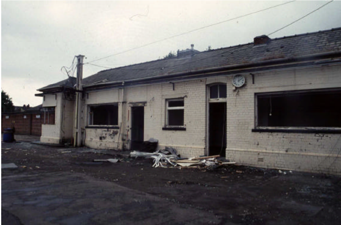
Plate 35: East elevation of Building 1, looking south/west
