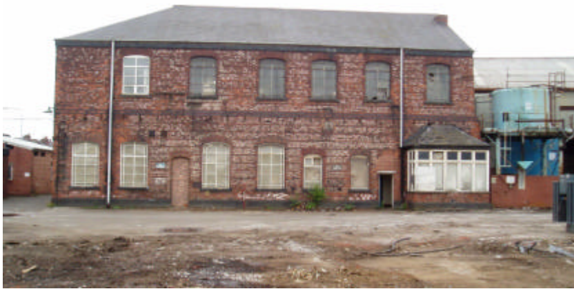
Plate 1: General view of Building 5, looking north
