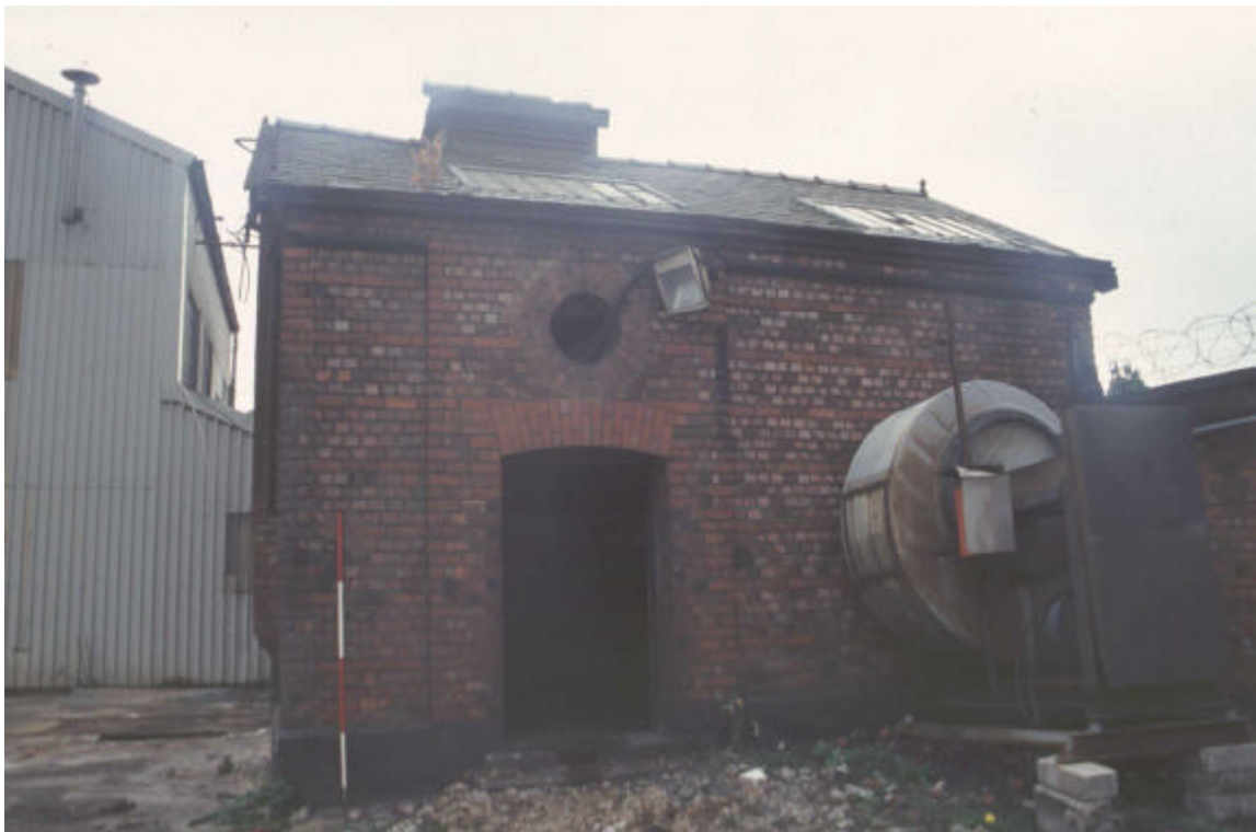
Plate 36: North elevation of Building 2
