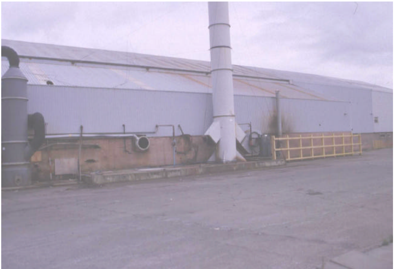
Plate 22: South (centre) elevation of Building 6
