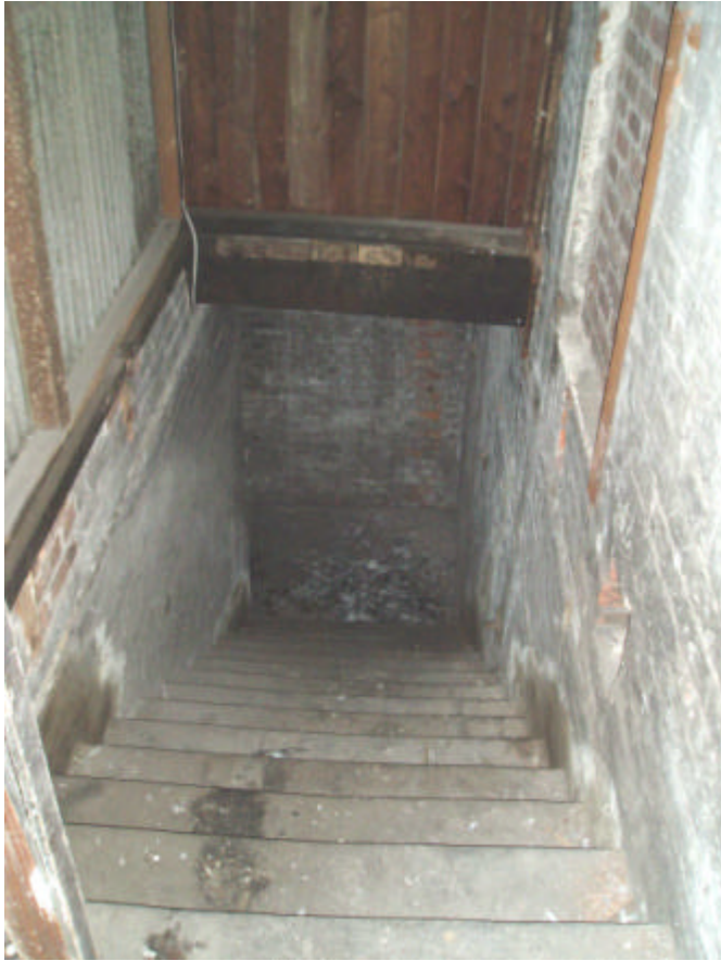
Plate 13: Fire exit stairs to the ground floor along the east end of Building 5
