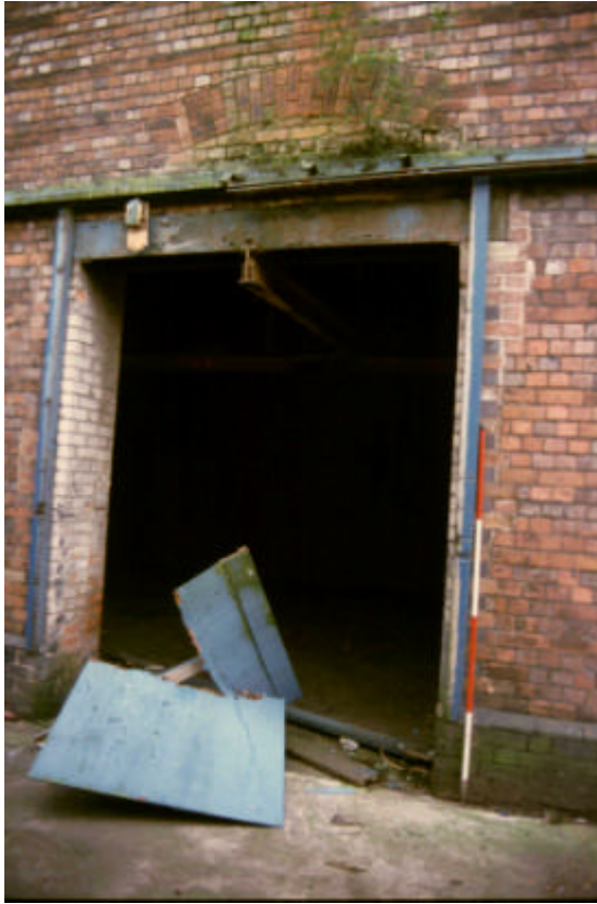
Plate 5: Loading bay along north external wall in Building 5
