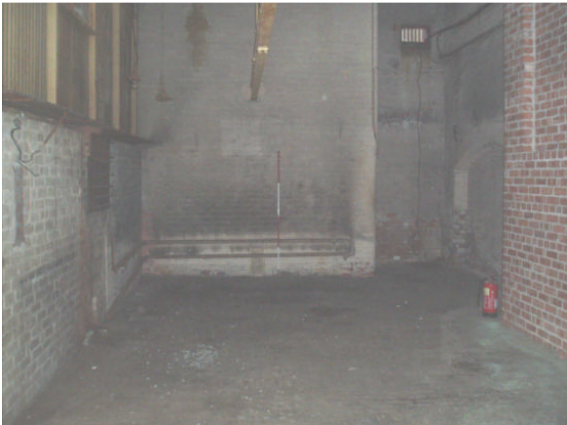
Plate 6: View of north room interior in Building 5
