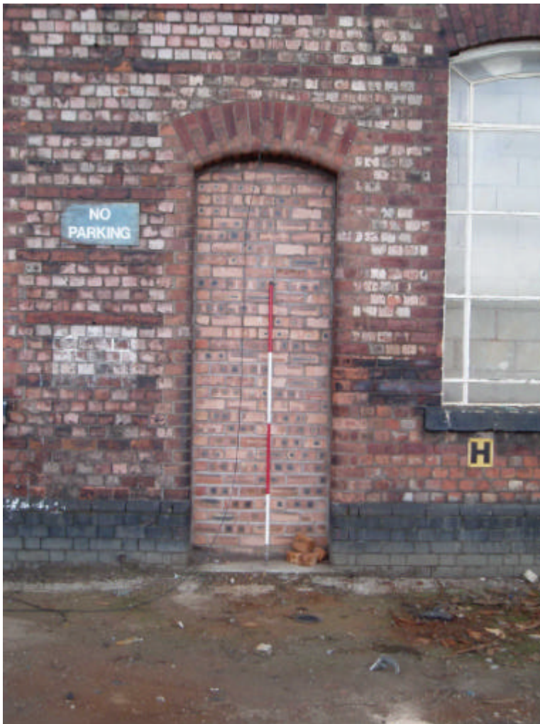
Plate 2: Blocked doorway at west end of south external elevation of Building 5
