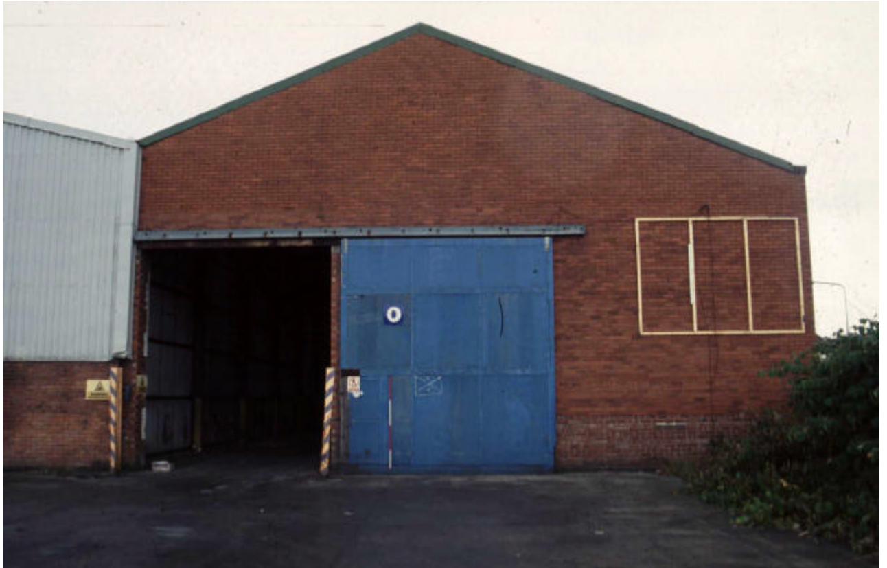
Plate 25: East elevation of Building 8
