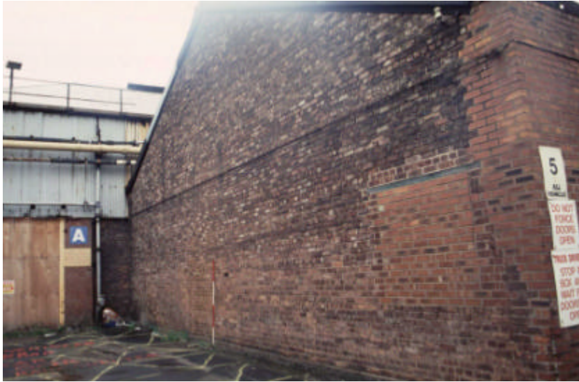
Plate 43: West elevation of Building 14
