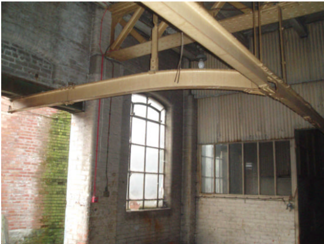
Plate 8: Girder rails running below ceiling of ground floor in Building 5, looking north
