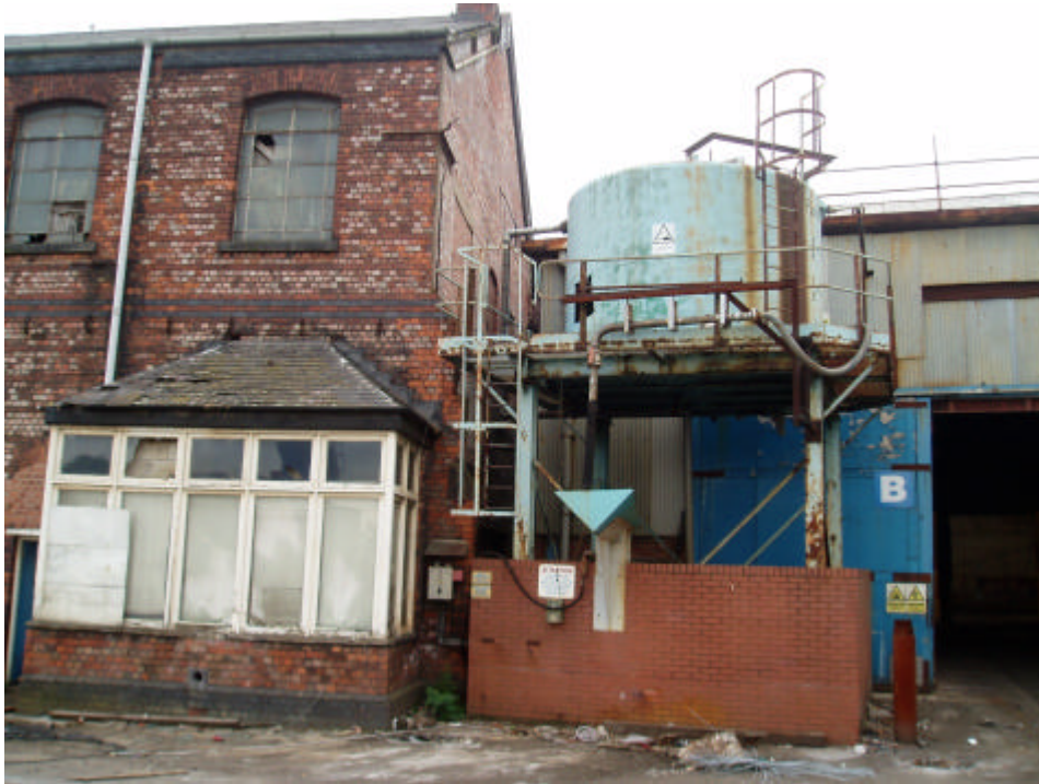
Plate 17: Porch attached to the east end of Building 5
