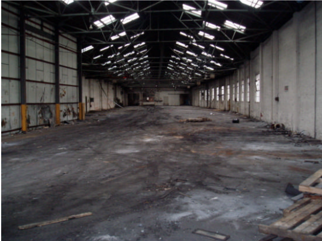
Plate 29: Interior of Building 8, looking west
