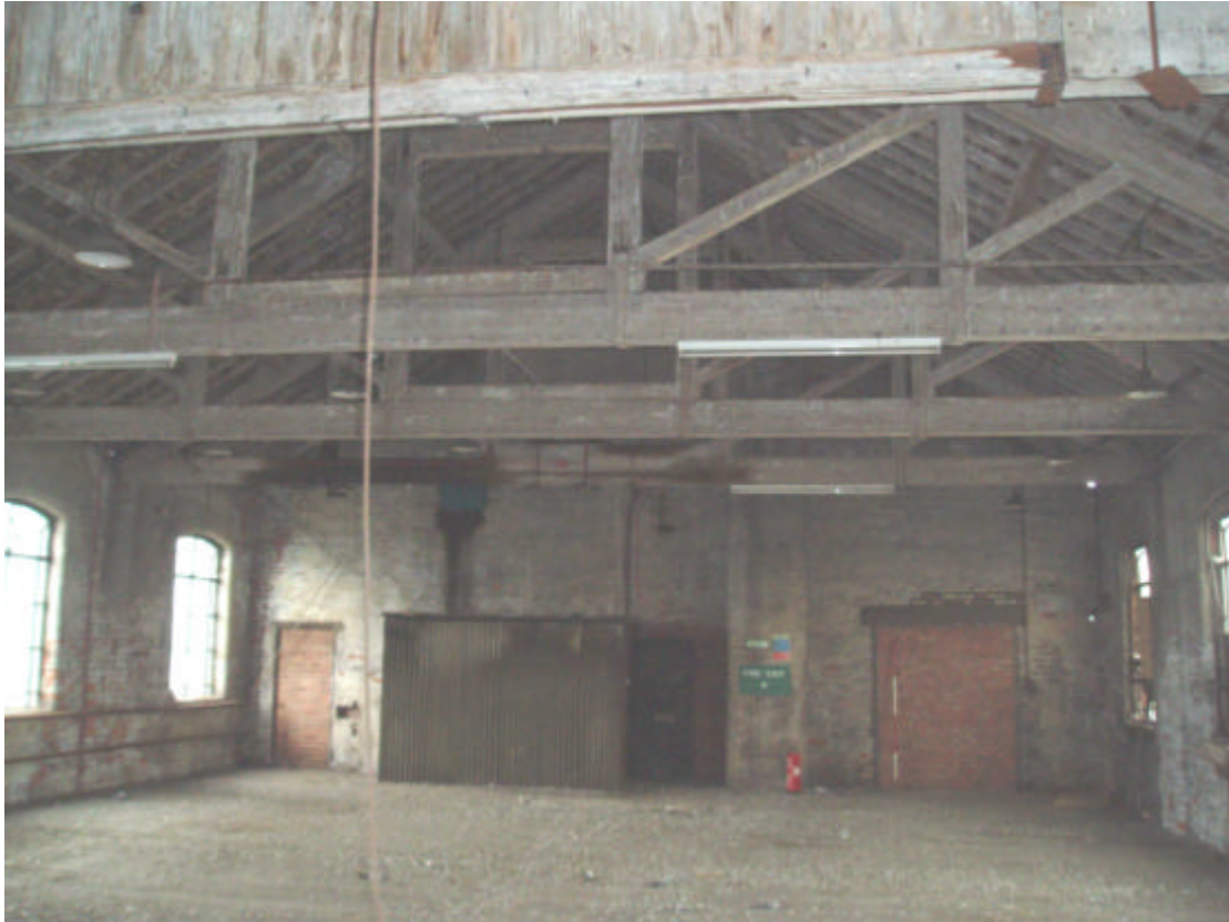
Plate 11: First floor ceiling in Building 5
