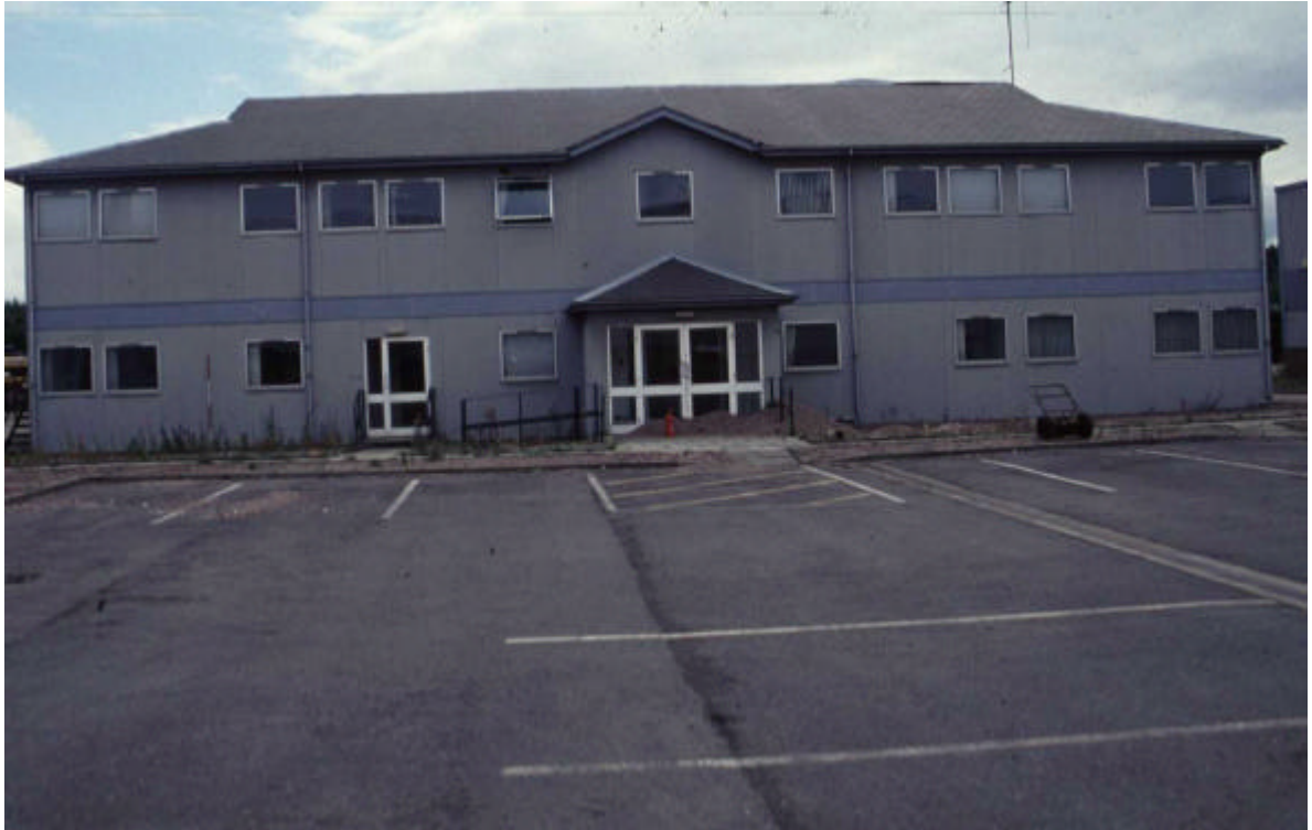
Plate 37: North elevation of Building 3
