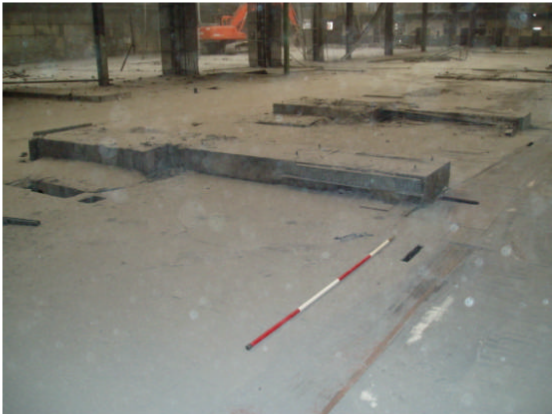
Plate 32: Machine platforms in Building 7
