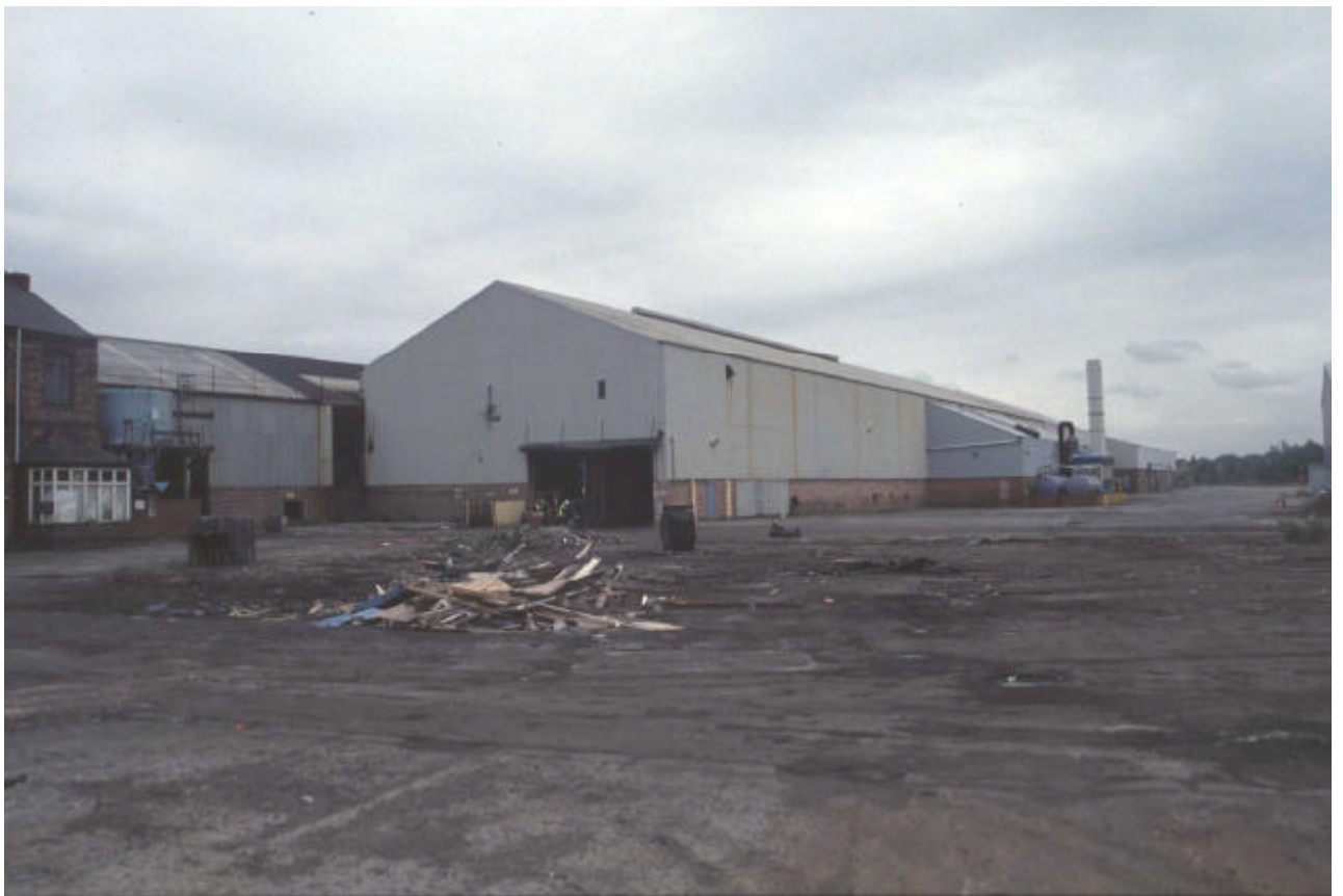
Plate 28: General view of Buildings 6 and 7, looking north/east
