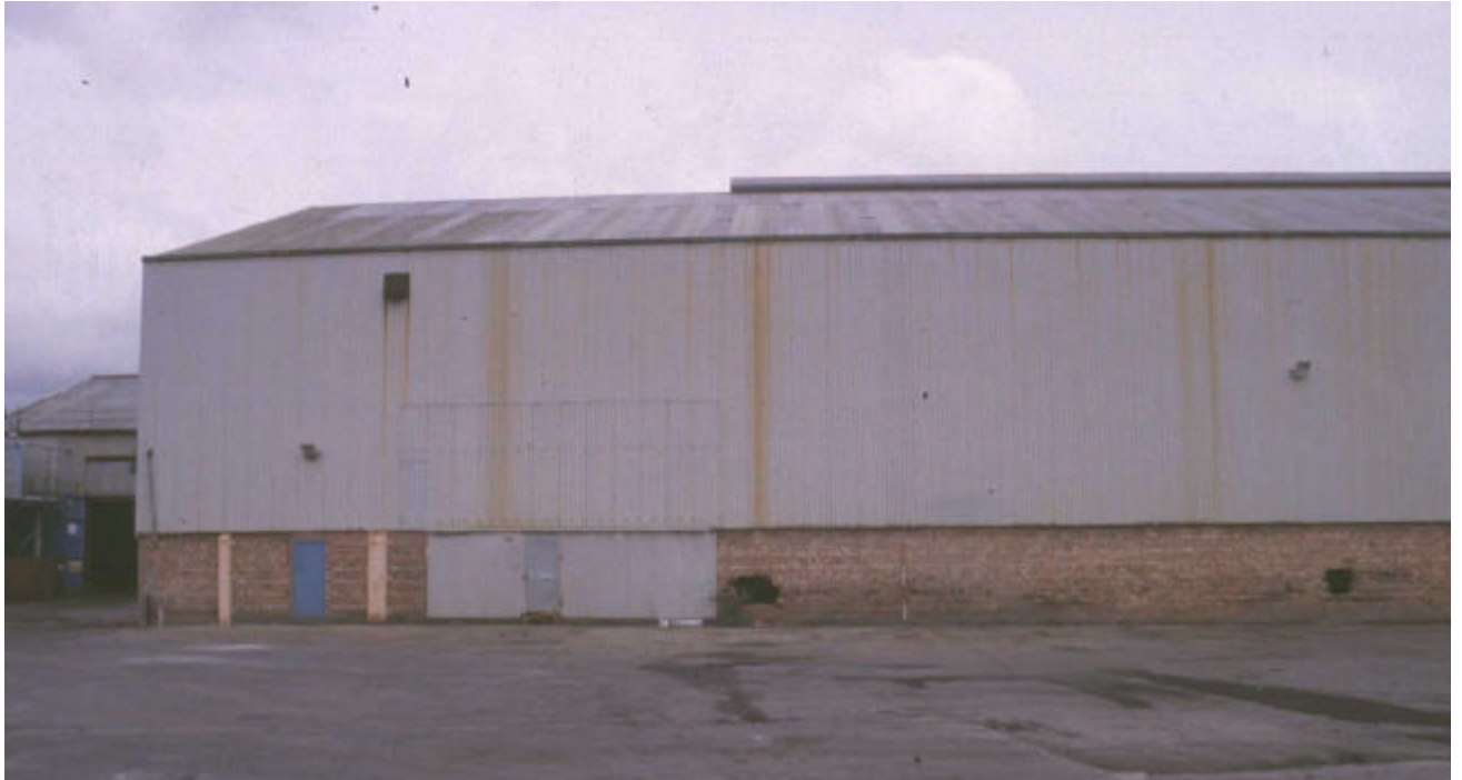
Plate 21: South (west) elevation of Building 6
