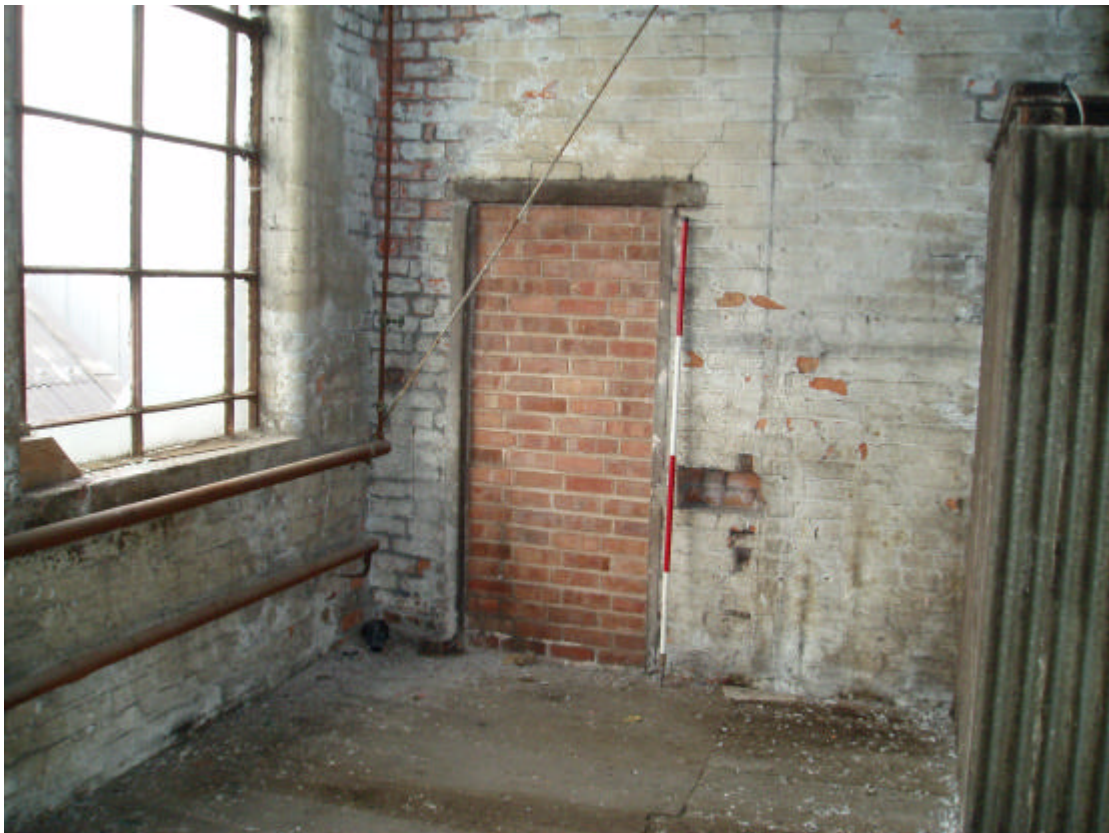
Plate 12: Blocked doorway within the east wall of Building 5
