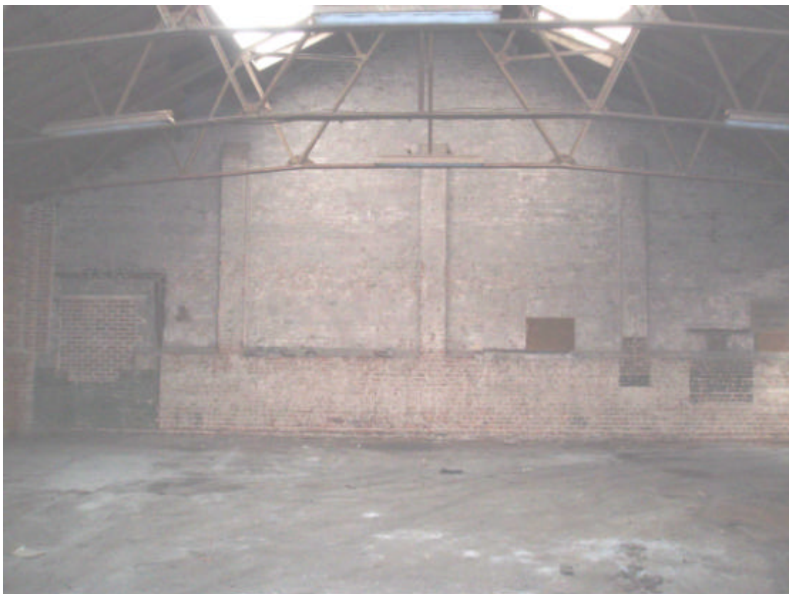
Plate 34: Internal east wall elevation in Building 8
