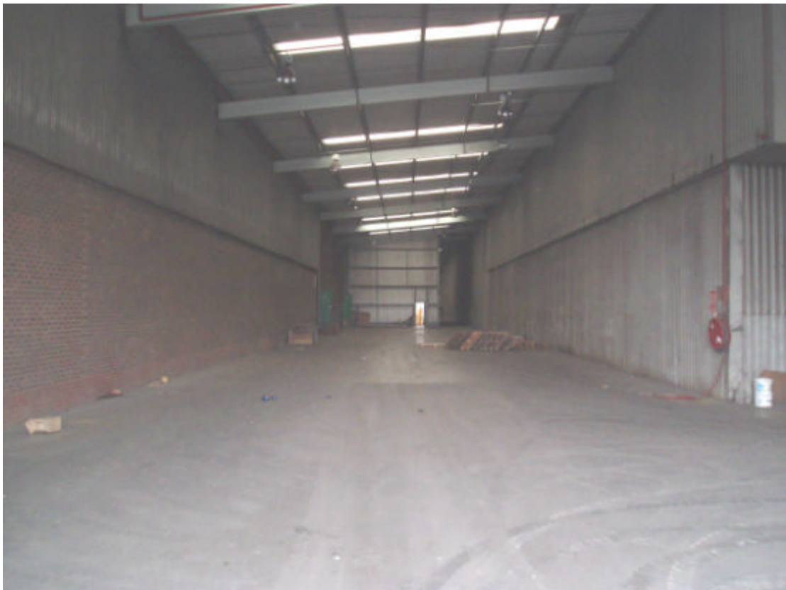
Plate 30: Interior of Building 6, looking south
