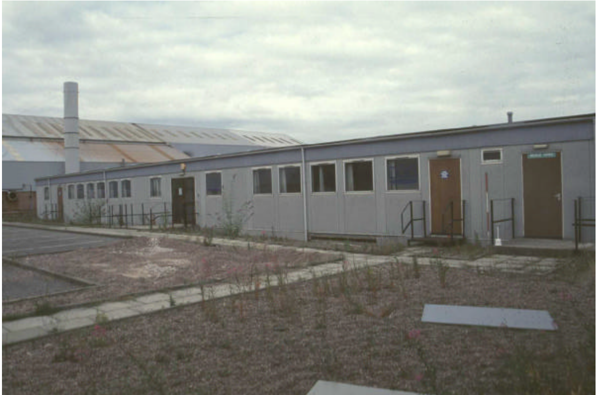
Plate 39: West elevation of Building 9
