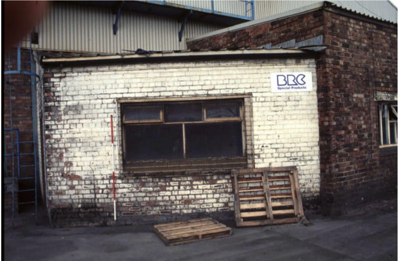
Plate 27: East elevation of Building 13
