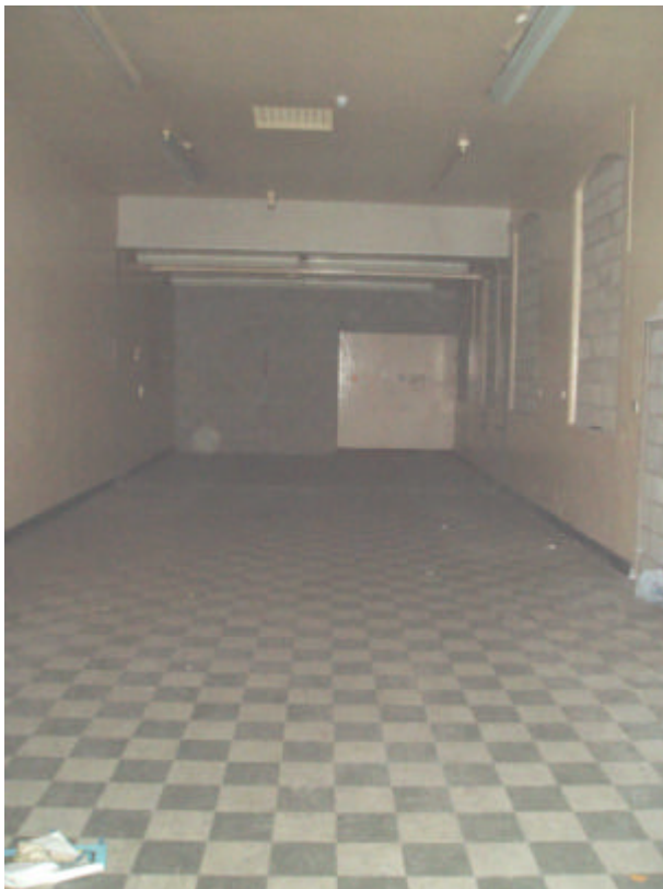
Plate 10: Ground floor interior of the south room in Building 5
