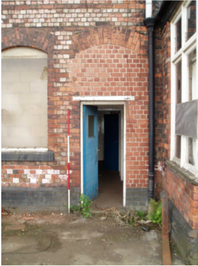
Plate 3: Doorway at east end of south external elevation of Building 5
