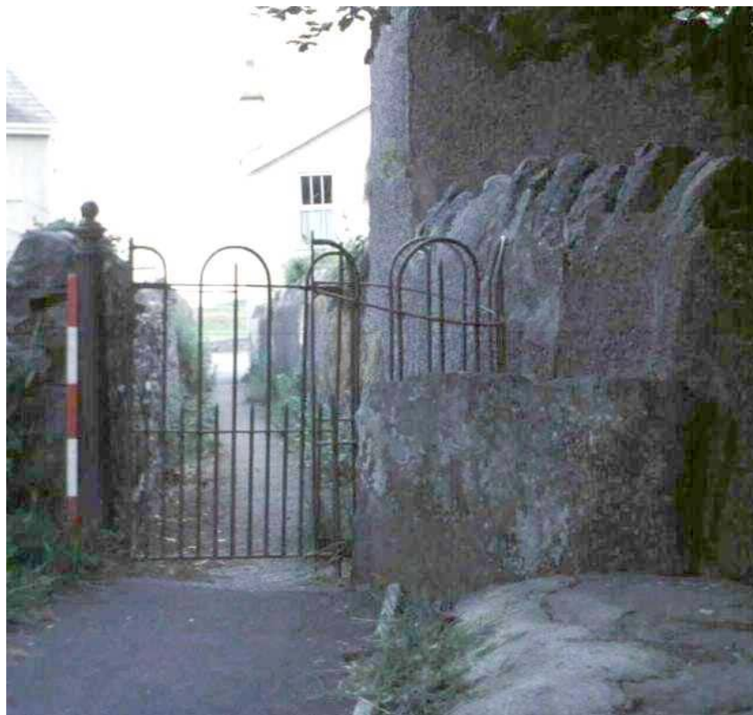
Plate 8: Site 10, kissing gate
