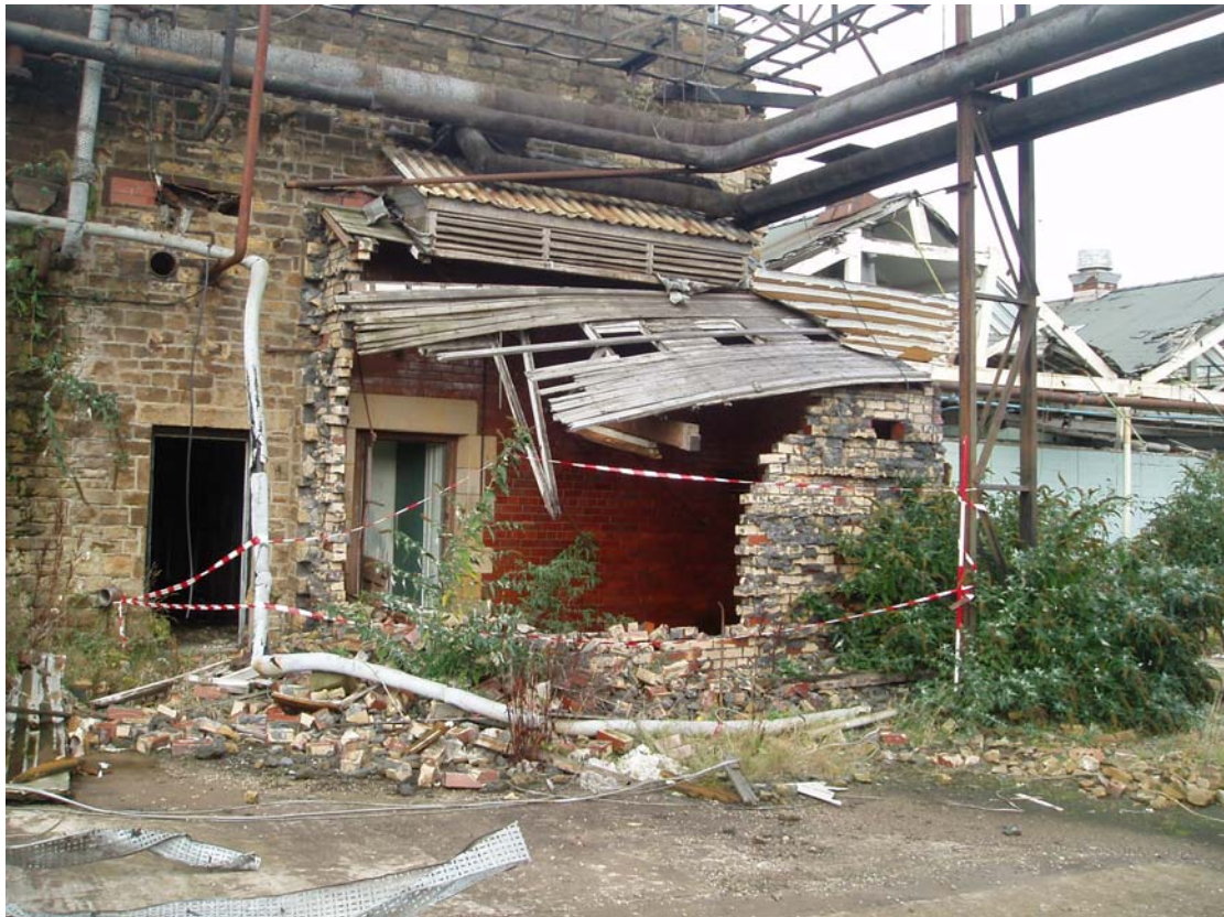
Plate 8: The damaged south end of Structure 22 , looking northeast
