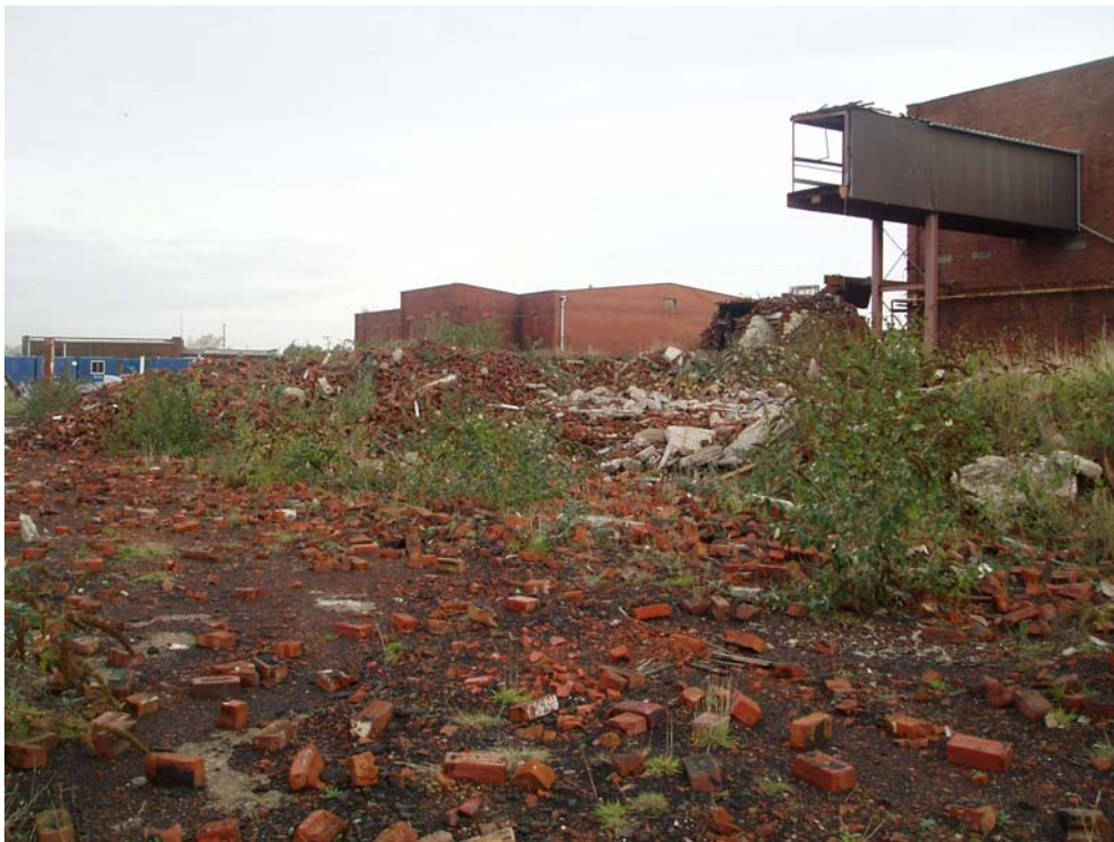
Plate 10: The demolished remains of Structures 32 and 33 with 31 beyond, looking north
