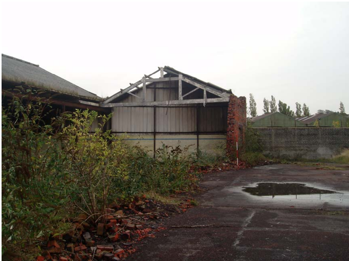
Plate 6: The damaged remains of Structure 20 , looking south
