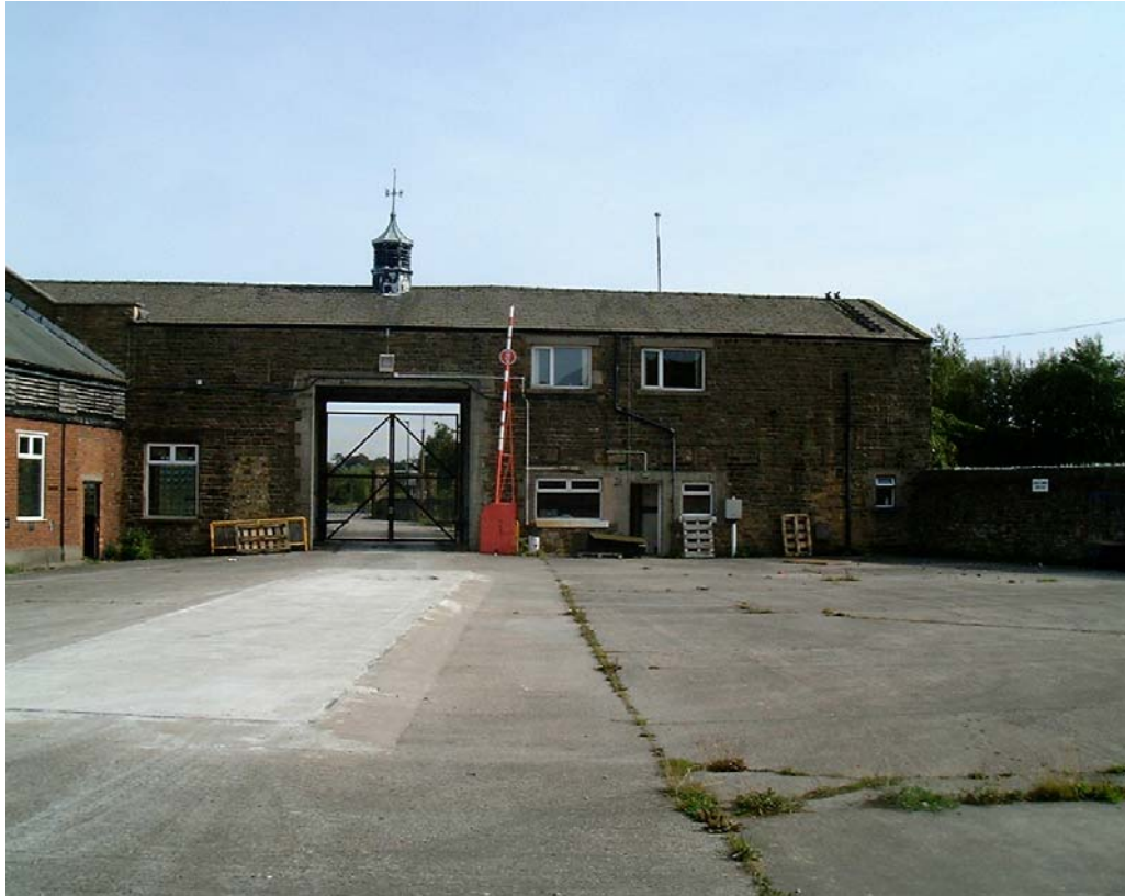
Plate 25: Structure 1 , looking east (after OA North 2002)
