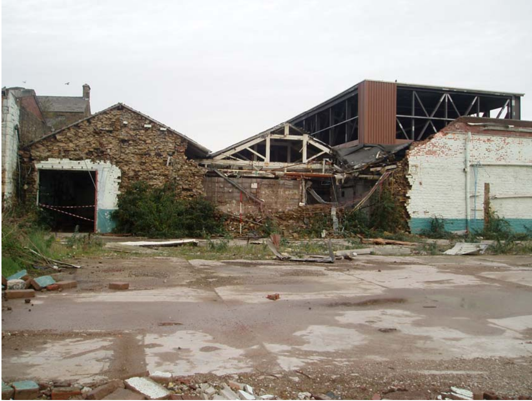
Plate 22: Structure 23 , looking north
