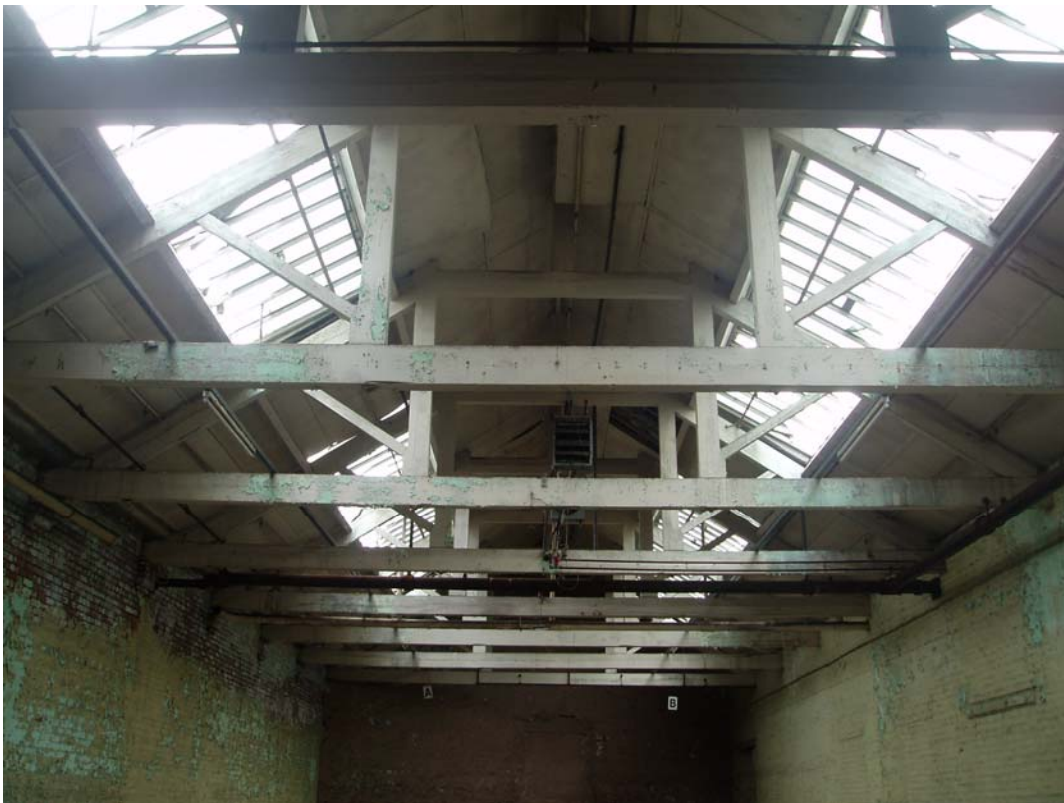
Plate 2: Trusses in Structure 4, looking south
