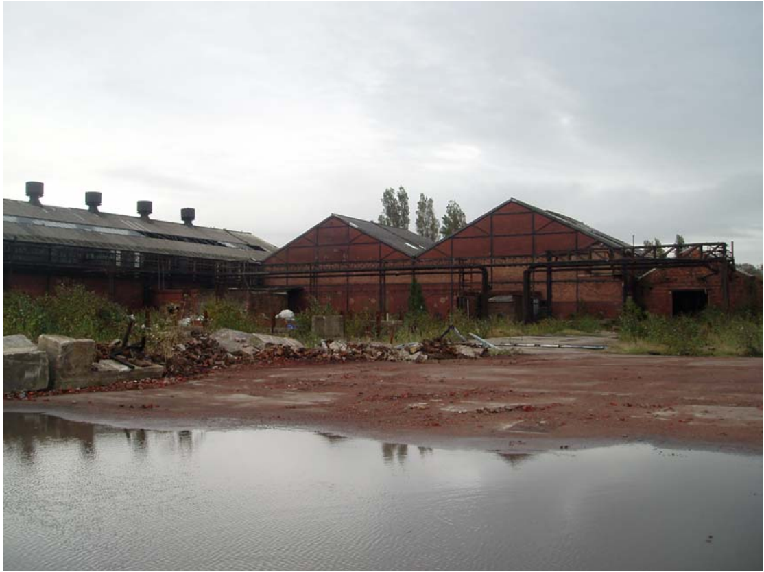
Plate 18: Structures 18 and 19 , looking south
