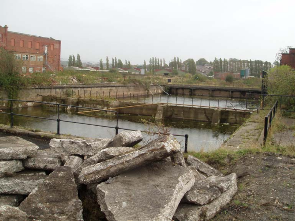
Plate 14: Structure 34 , looking south-east
