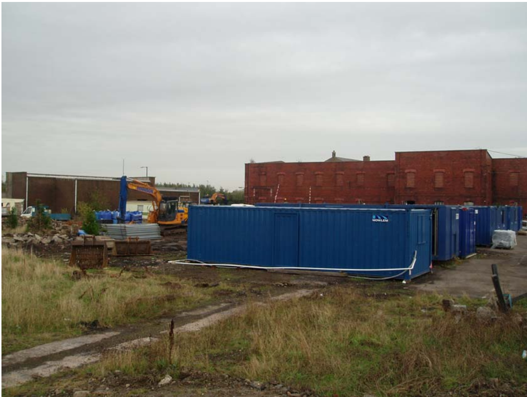
Plate 23: Structures 27 and 29 , looking northeast
