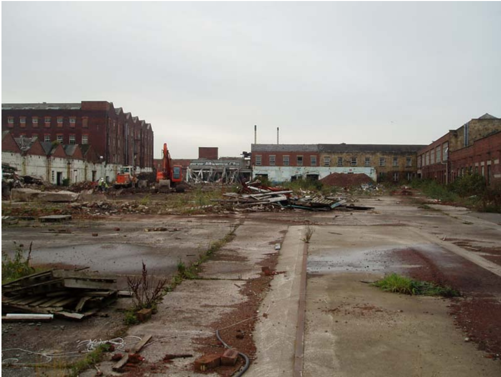
Plate 1: The site of Structures 3, 5-8 and 12-13 following demolition, looking west
