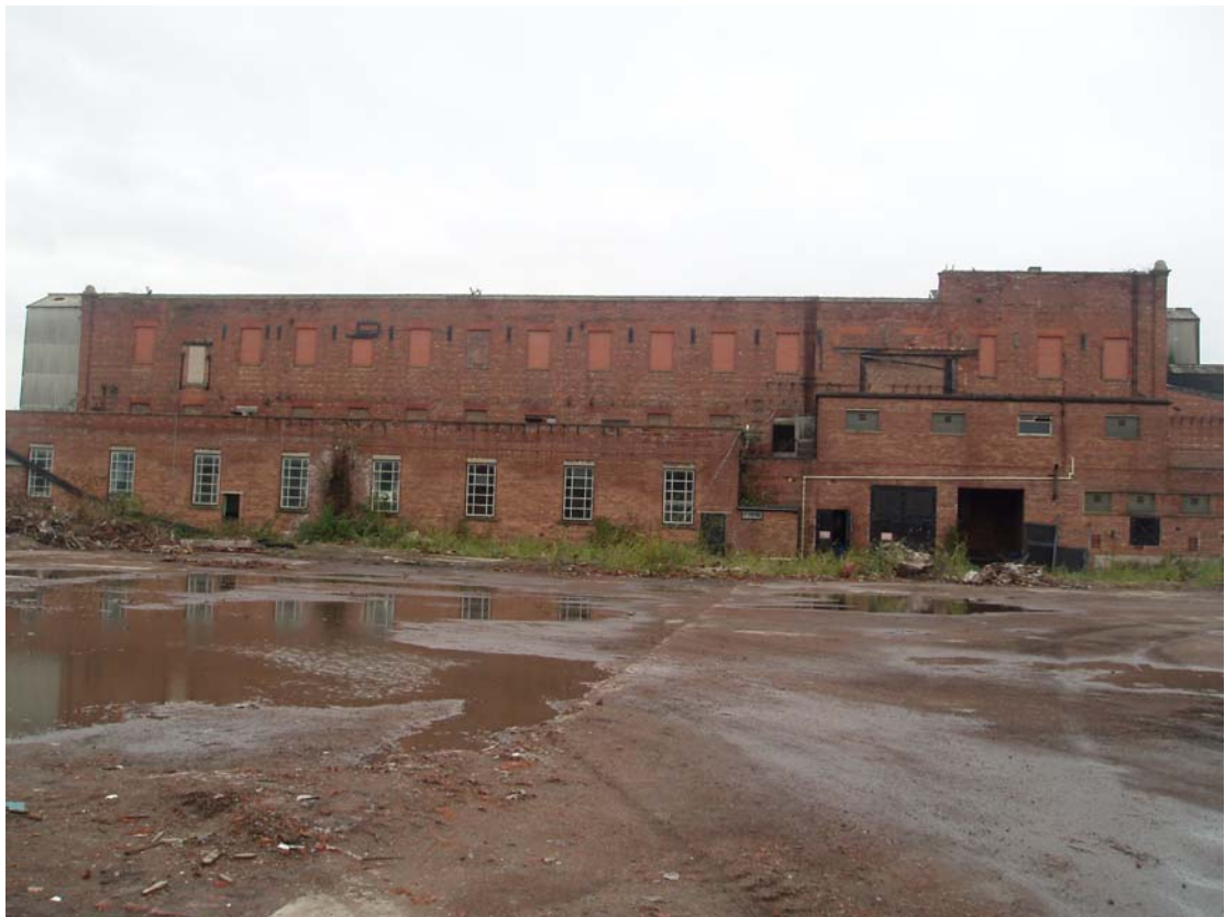
Plate 19: Structure 31 , looking west
