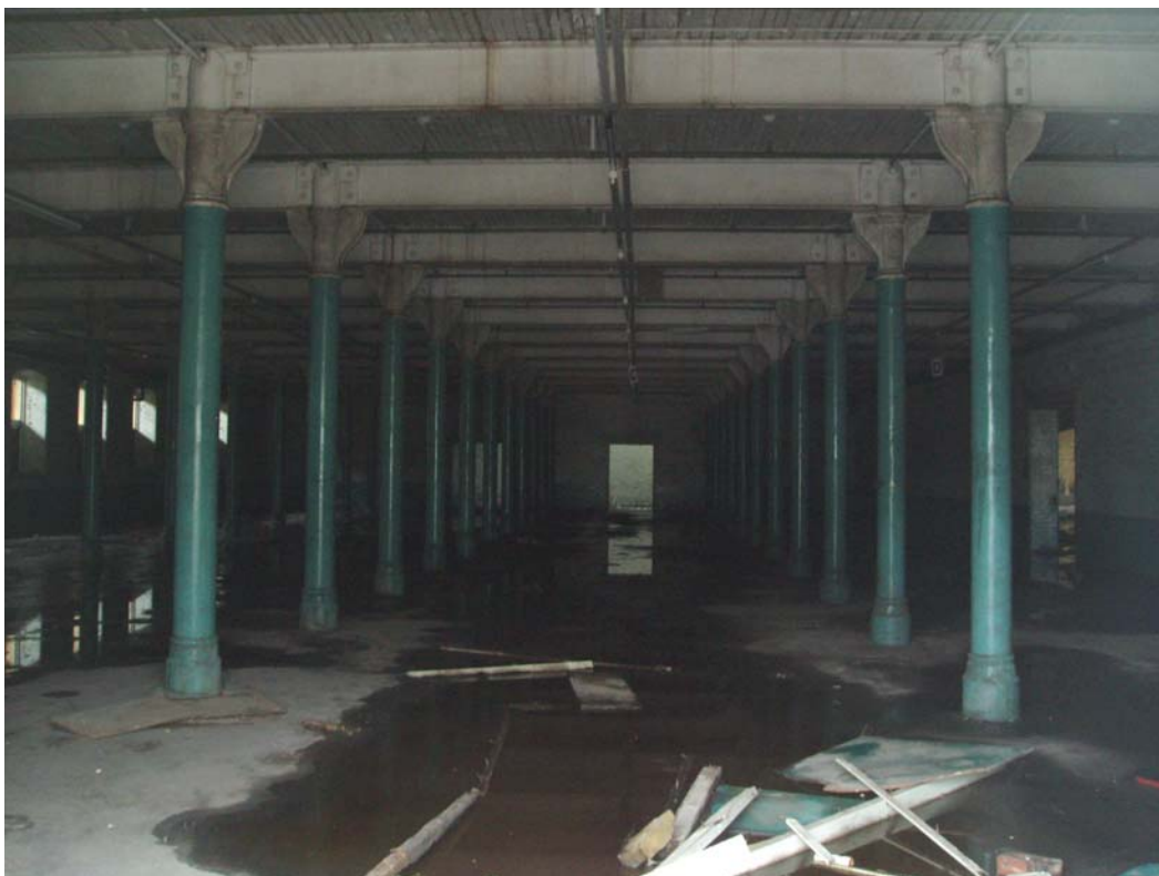
Plate 17: The columns within Structure 11 , looking south
