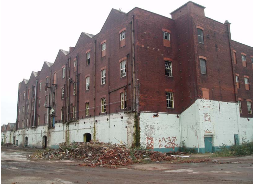
Plate 3: General view of Structure 11 , looking southeast
