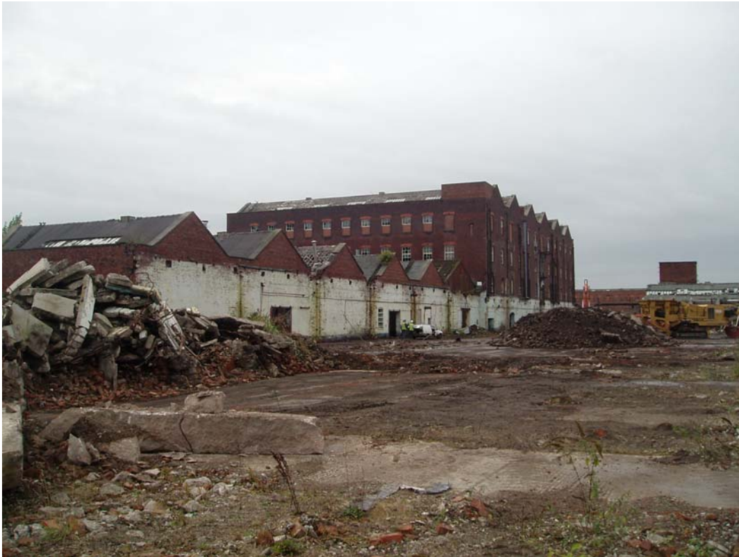
Plate 16: General view of Structures 4 , 9 and 11 , looking south-west
