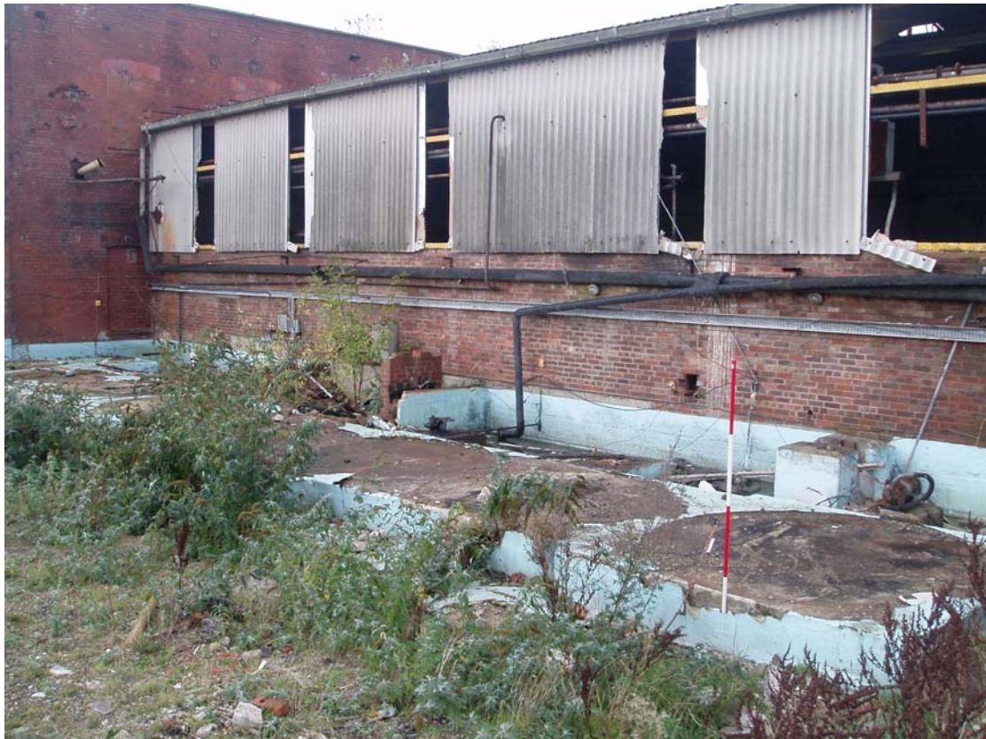
Plate 15: Engine bases at the south end of Structure 25 , looking north-west
