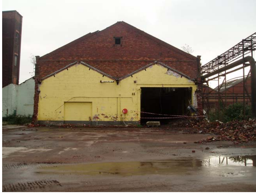
Plate 7: The damaged remains of Structure 21 , looking south
