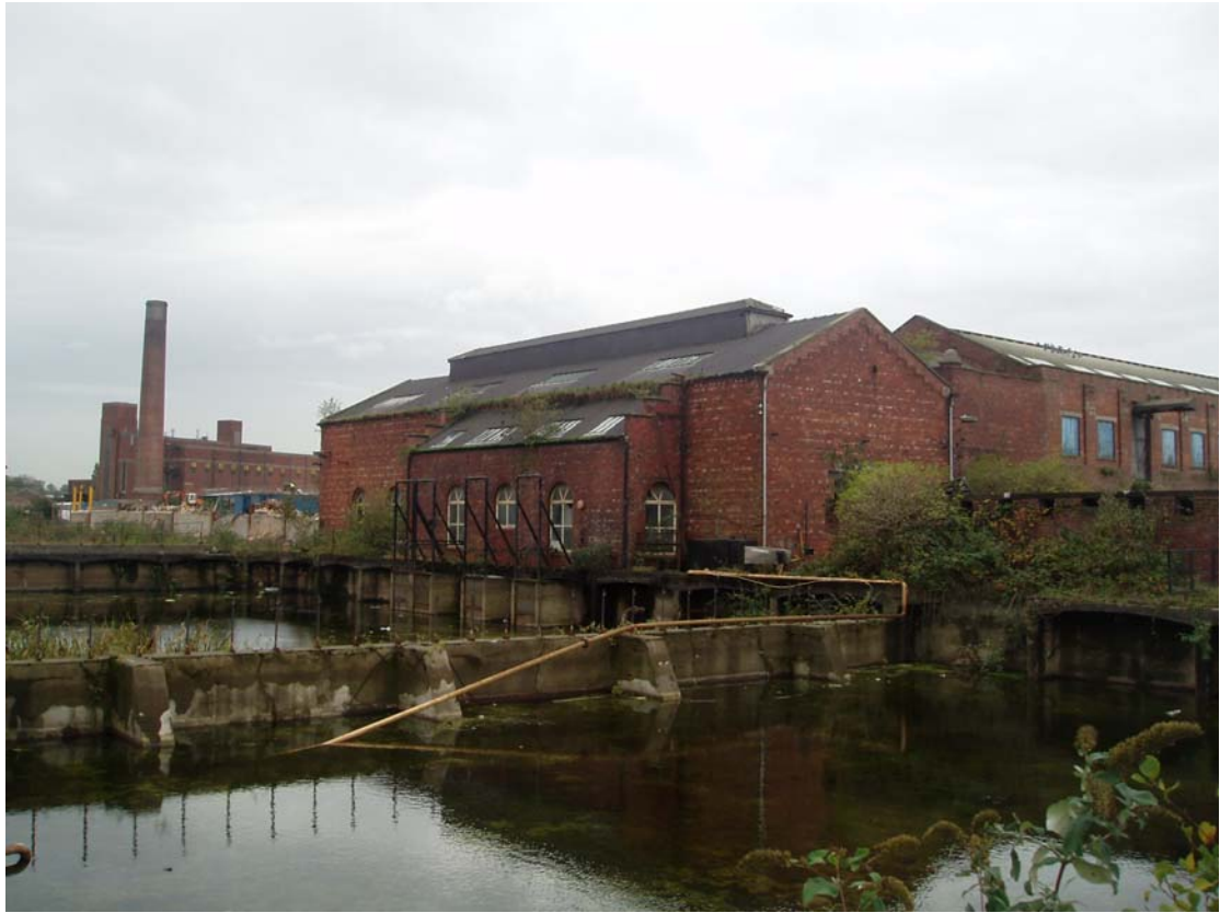
Plate 20: Structure 36 , looking south-west
