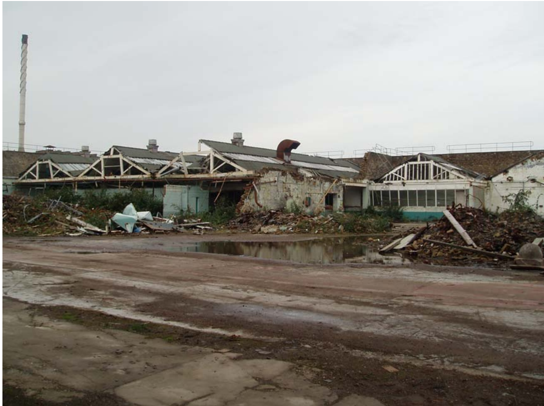
Plate 5: The damaged remains of Structure 17 , looking northwest
