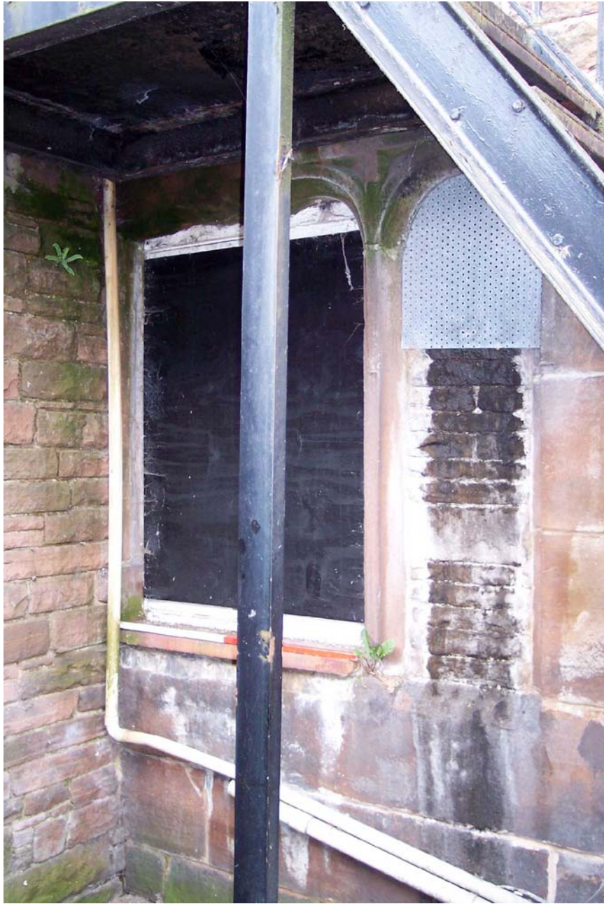
Plate 7: Relocated arched window, external south elevation (Room 4)
