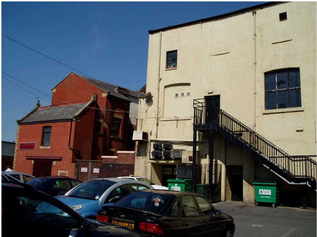
Plate 16: The rear of Buildings 6, 7 and 8, looking north-west
