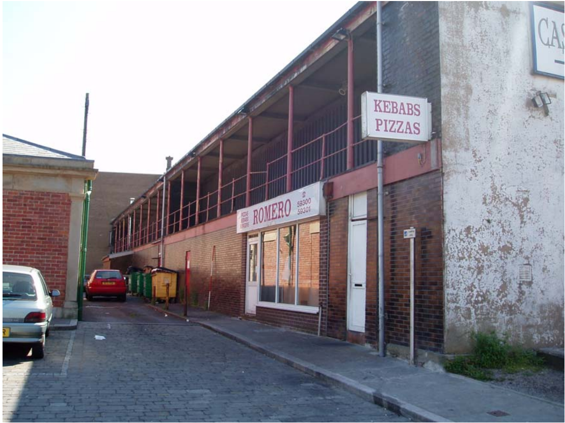
Plate 13: Building 5, looking south-east
