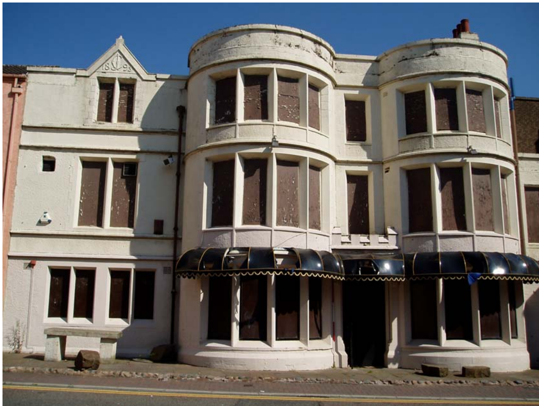
Plate 10: Building 2 looking north
