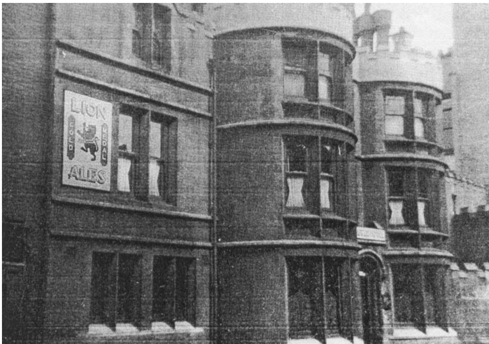
Plate 8: An early view of the Castle Hotel (after Baggoley 1996, 65)
