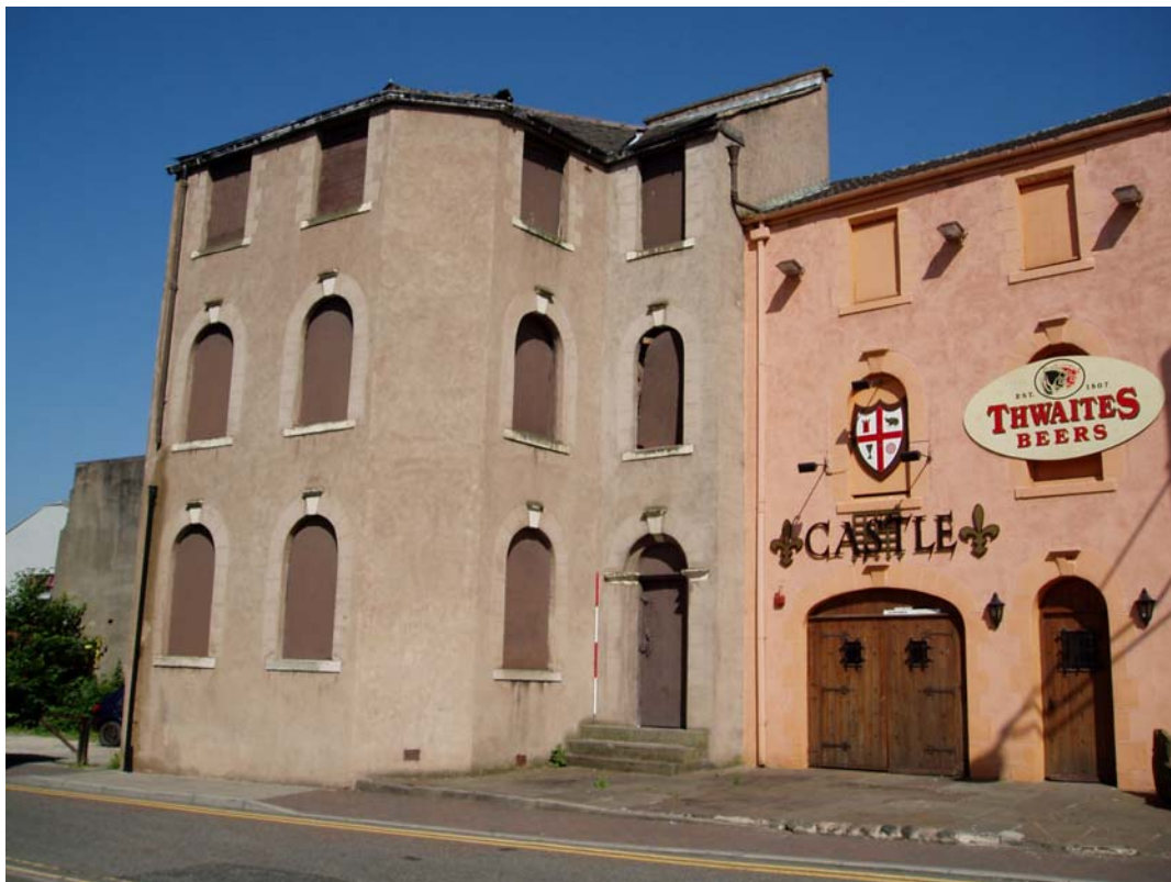
Plate 12: Building 4, looking north-west
