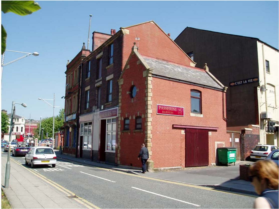
Plate 15: Buildings 7 and 8, looking north-east
