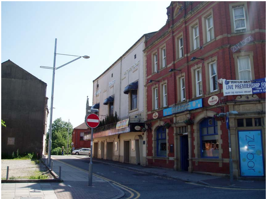
Plate 14: The ZY Bar, formerly the Dun Horse, and Building 6, looking south-east
