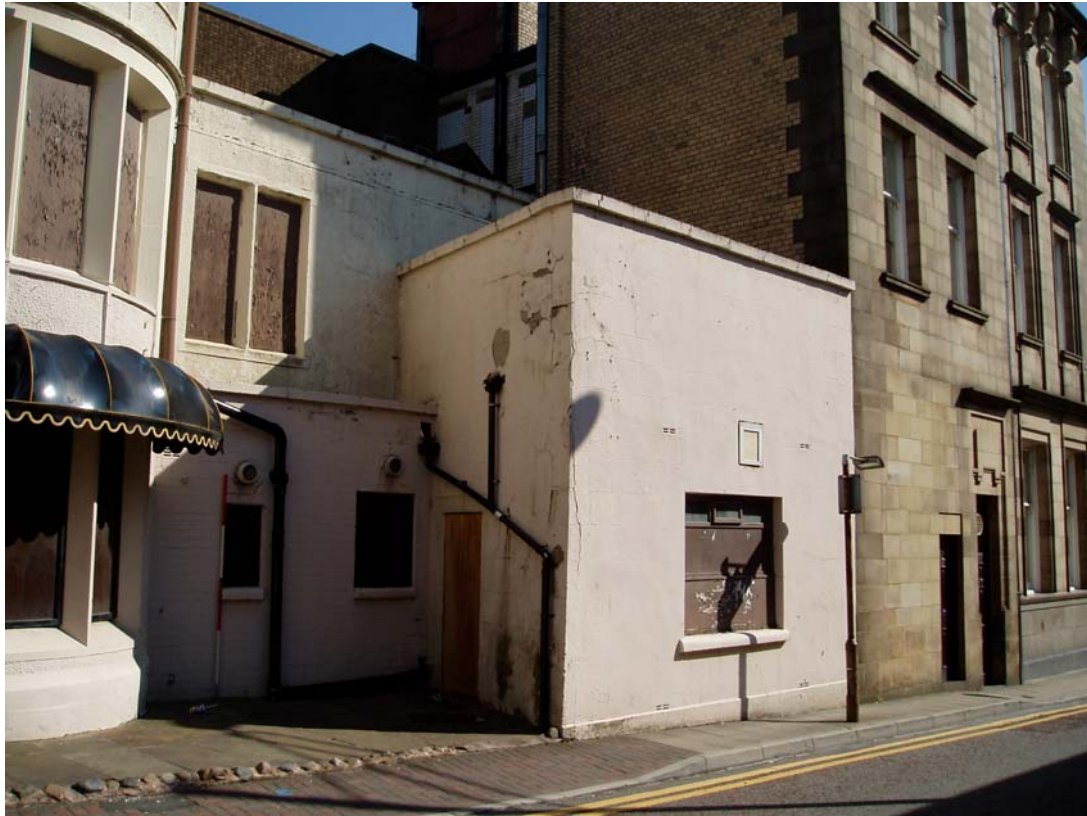
Plate 9: Building 1, looking north-east
