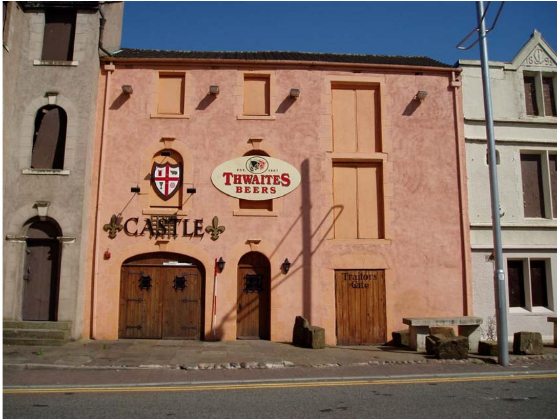
Plate 11: Building 3, looking north
