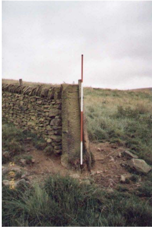
Plate 17: Site 84 , Field 18, gatepost, looking north-east
