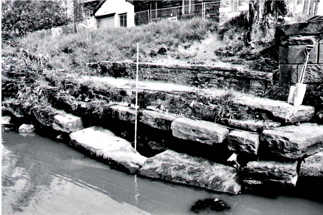
Plate 8: North-west-facing view of the north bank of the Reedyford Weir site
