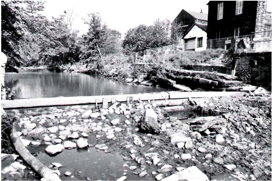
Plate 1: North-west facing view of Reedyford Weir
