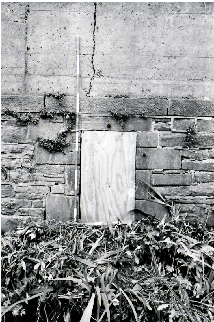
Plate 12: Detail of the blocked out-fall at the Romney Avenue site
