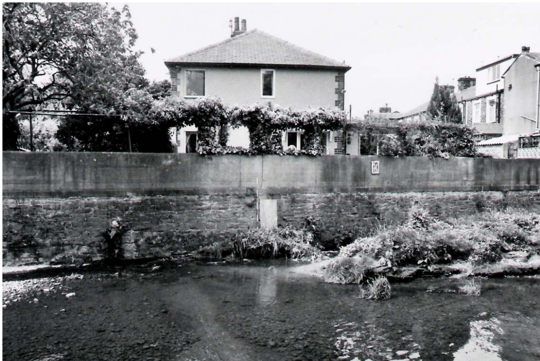
Plate 11: Retaining wall at the Romney Avenue site
