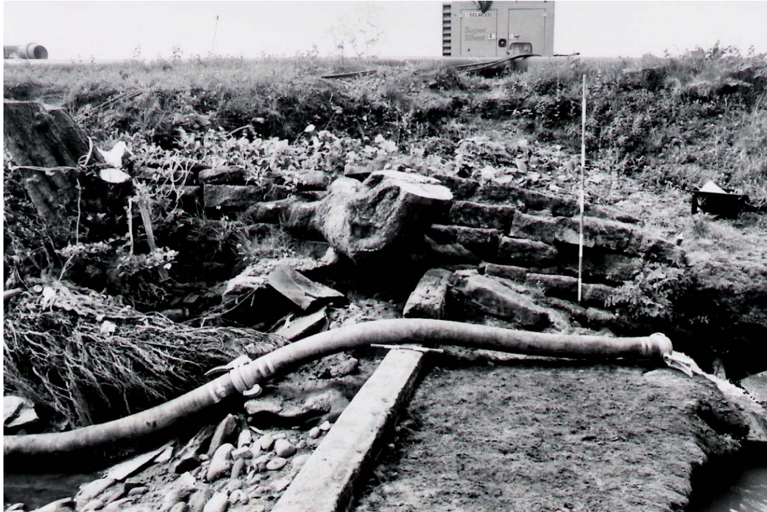
Plate 10: South-facing view of the south bank of the Reedyford Weir site
