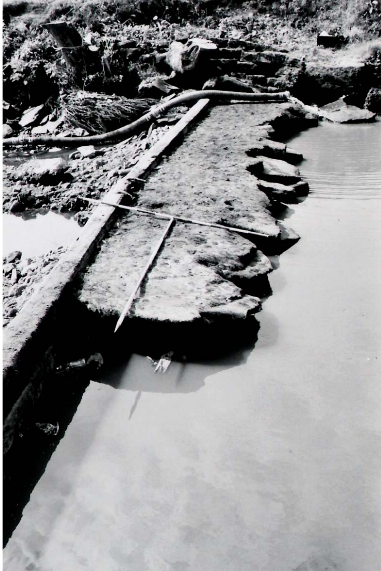
Plate 5: The concrete platform on the western side of Reedyford Weir
