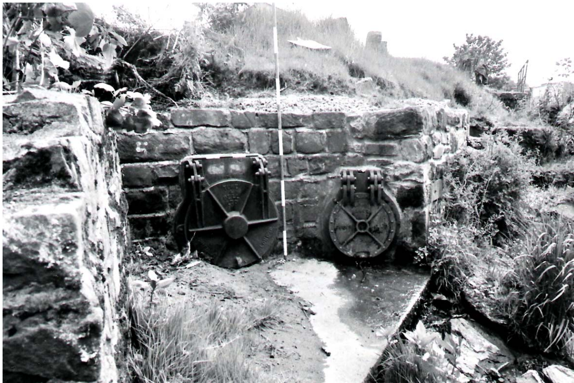
Plate 9: Out-falls on the north bank of the Reedyford Weir site
