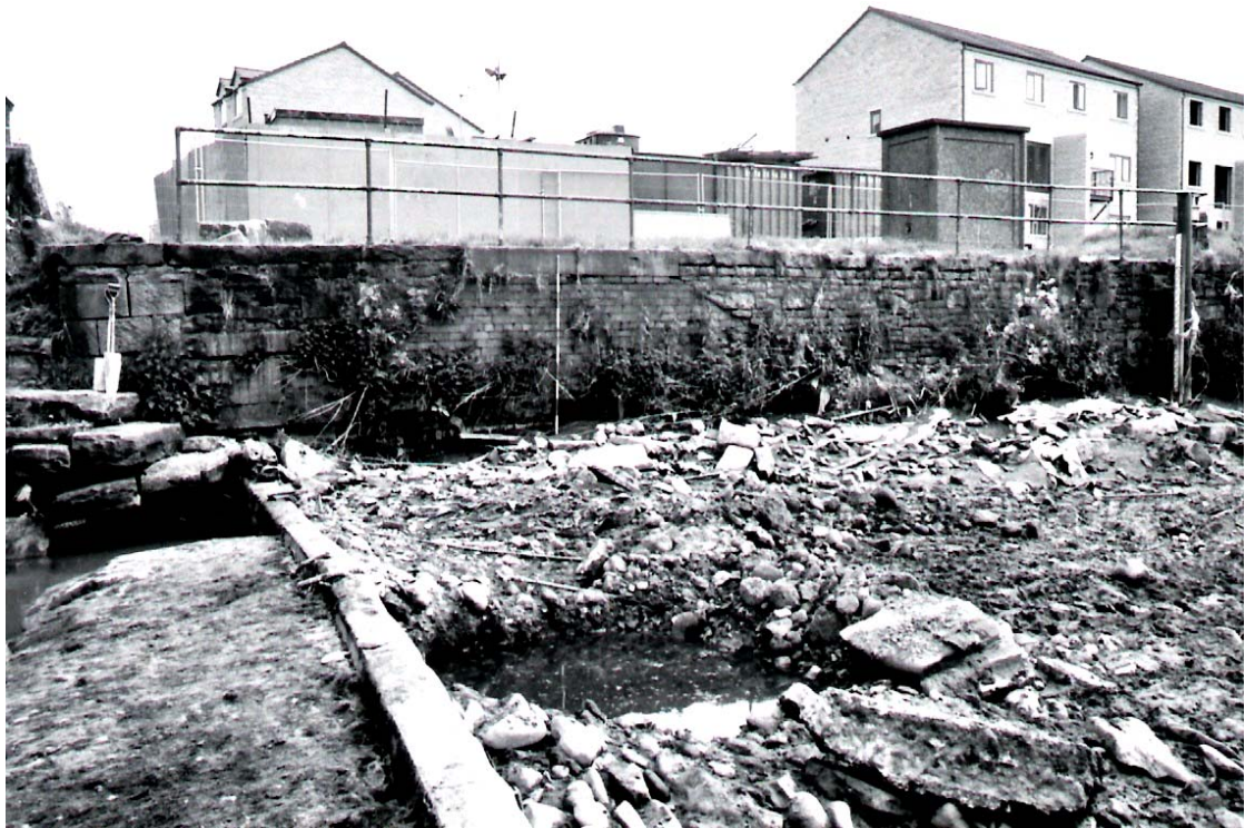
Plate 6: North-facing view of the retaining wall on the north bank of the Reedyford Weir site
