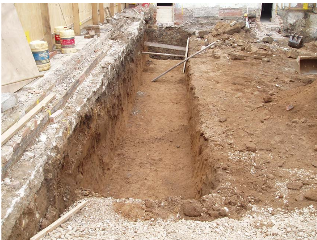
Plate 4: Oblique view of north-facing section showing the cellar wall of 33-35 Penny Street
