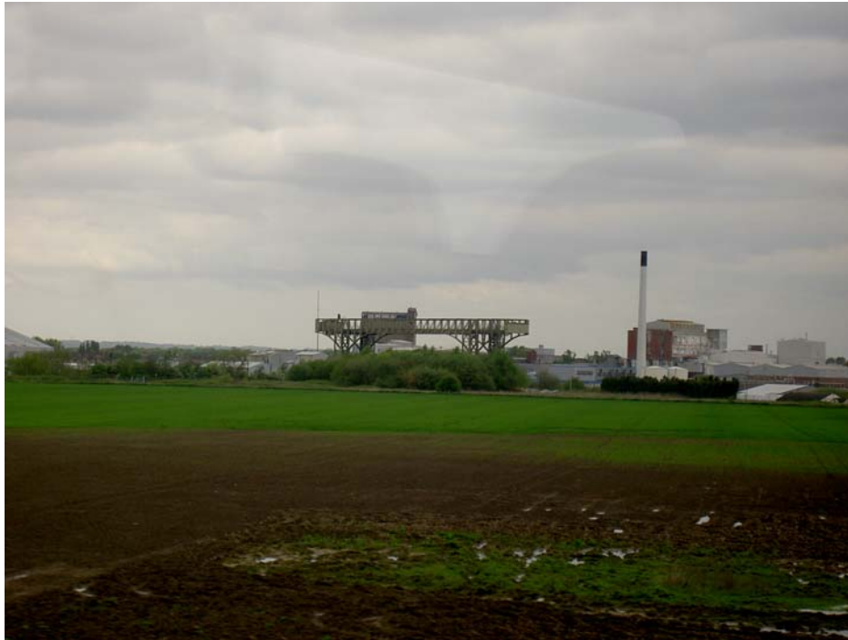
Plate 1: Part of the east (Arpley Meadows) half of the proposed development area, with the transporter bridge (Site 06) in the background, facing north-west
