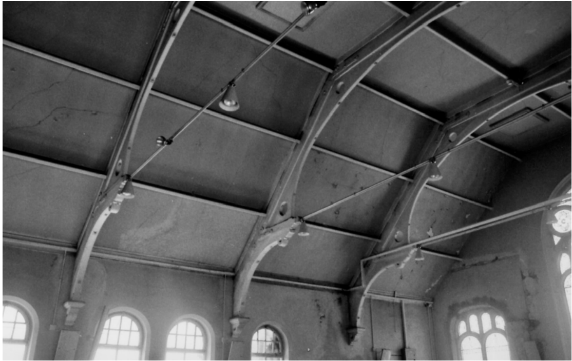
Plate 9: Detail of the Hammerbeam Trusses in the First Floor Chapel
