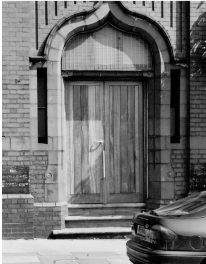
Plate 5: Detail of one of the Entrances on the West Elevation
