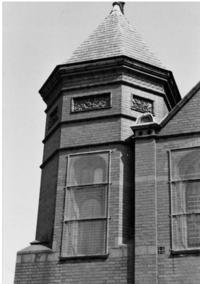
Plate 8: Detail of the Octagonal Tower at the North-West Corner of the Building
