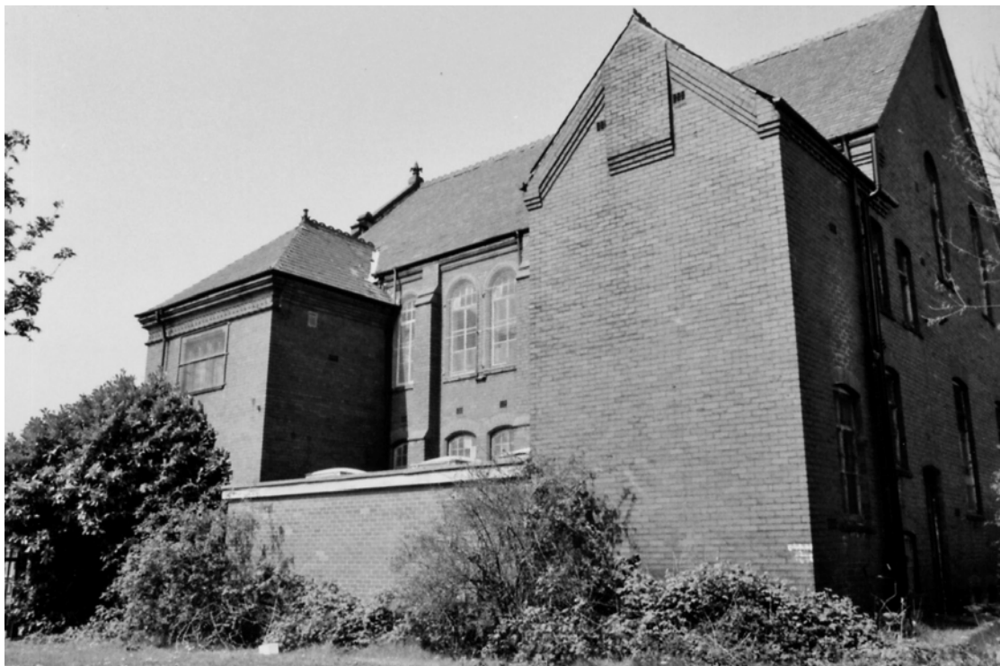
Plate 2: The South-Facing Elevation of the Church
