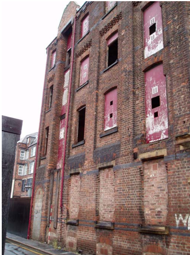
Plate 3: West-facing elevation of Building 1, showing blue-brick string courses
