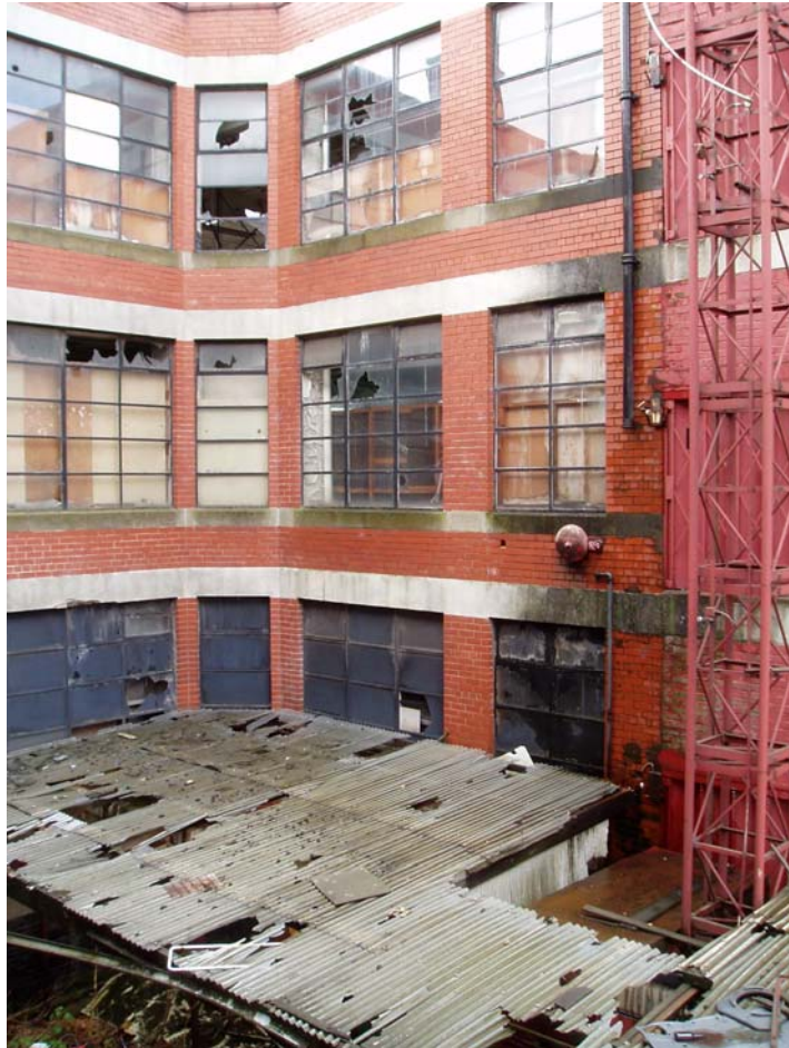
Plate 30: Steel-framed hoist to the west of the staircase in the northern wing of Building 3
