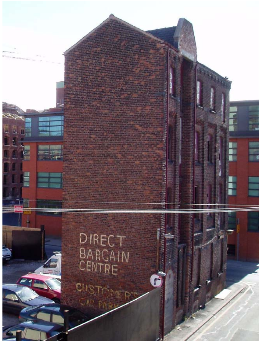
Plate 10: North-facing elevation of Building 1
