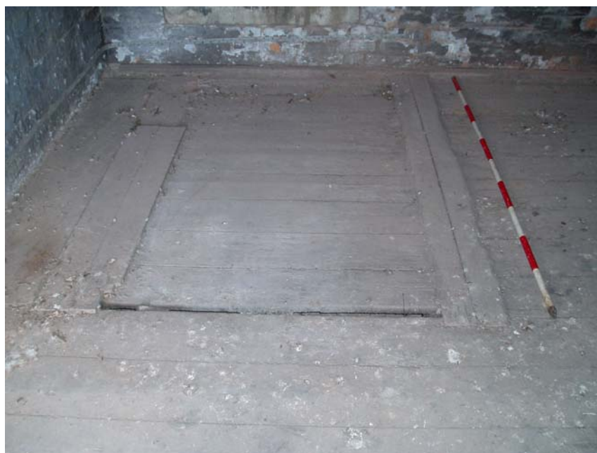
Plate 11: Trap door on 3 rd floor of Building 1
