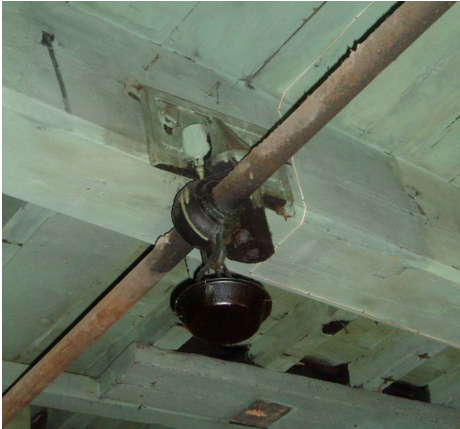
Plate 14: Line-shaft supporting hangers attached to the southern side of the ground floor ceiling beams, complete with oil-drip trays
