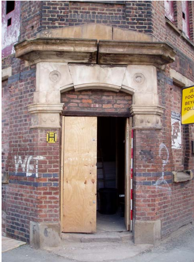
Plate 2: The main door of Building 1, showing the triangular sandstone frontal above a segmental sandstone bed, supported on moulded sandstone door jamb capitals
