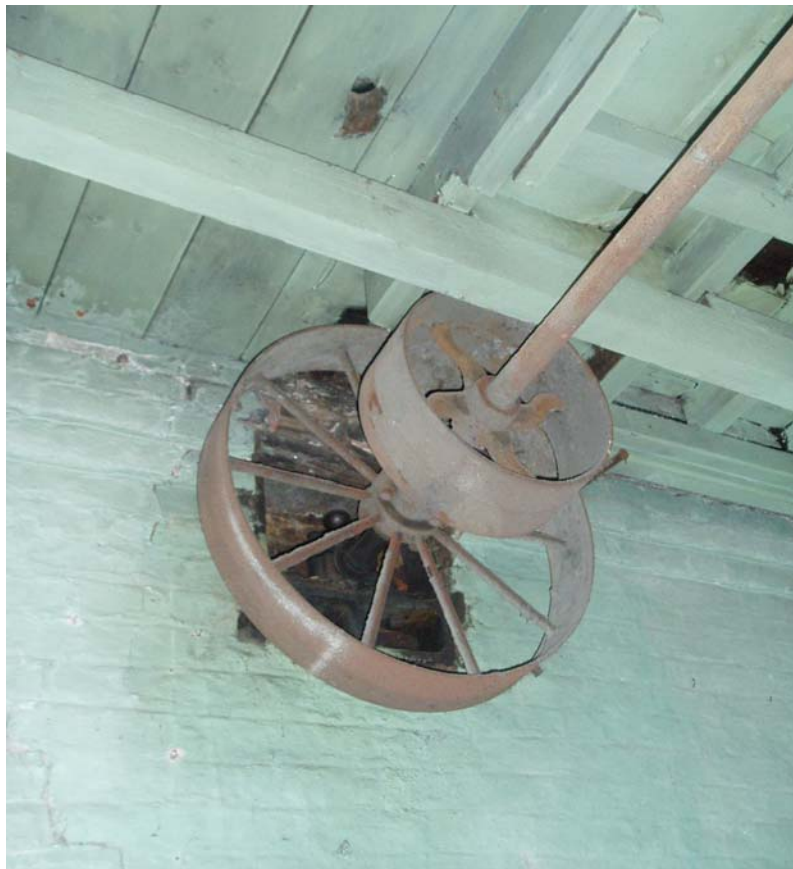
Plate 13: Line-shaft flywheel and bearing box in party wall
