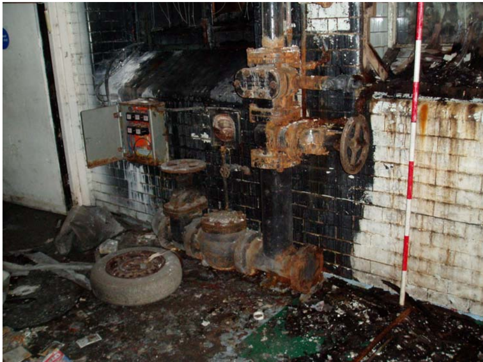
Plate 31: Detail of sprinkler valves in basement of Building 3
