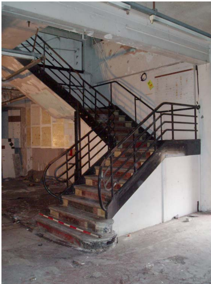
Plate 29: Detail of staircase against south elevation of ground floor in Building 3
