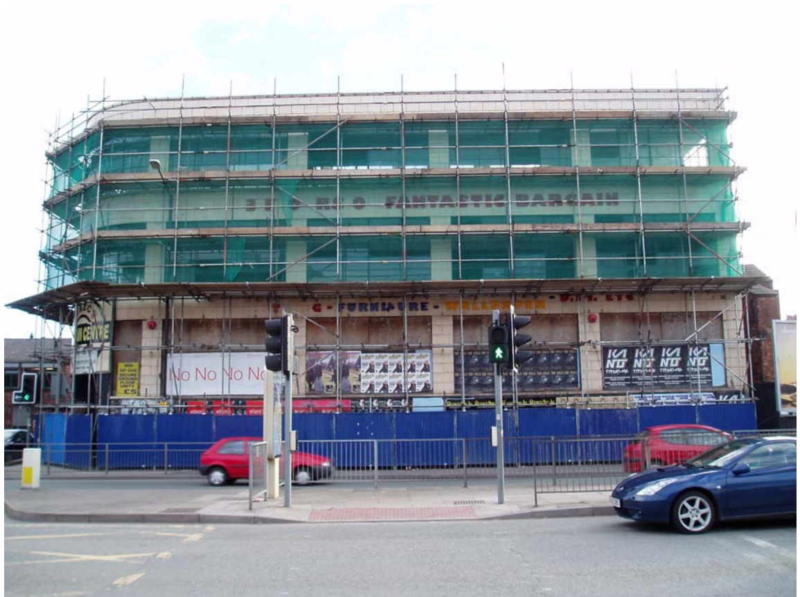
Plate 26: General view of Building 3 across Great Ancoats Street
