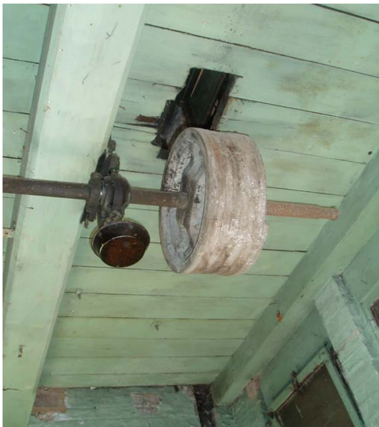
Plate 15: Aperture in ground floor ceiling for belt drive
