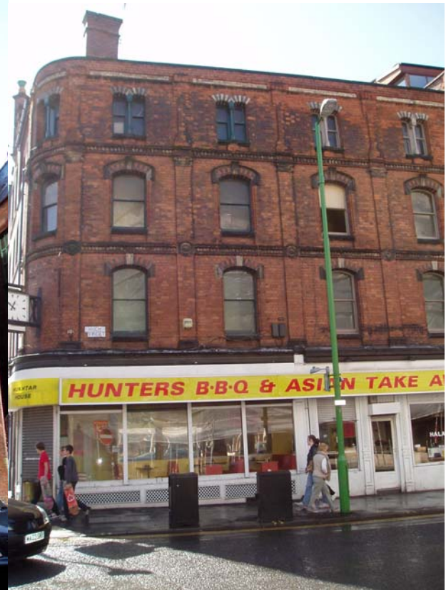
Plate 37: 1870s building on corner of Thomas Street and High Street
