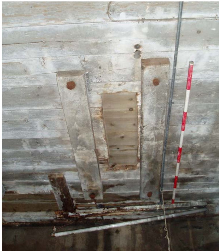
Plate 25: Detail of evidence for power transmission within ground floor of Building 2
