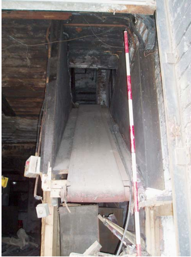
Plate 24: Looking west at conveyor belt between ground and 1 st floor of Building 2
