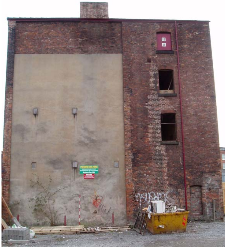
Plate 8: East-facing elevation of Building 1
