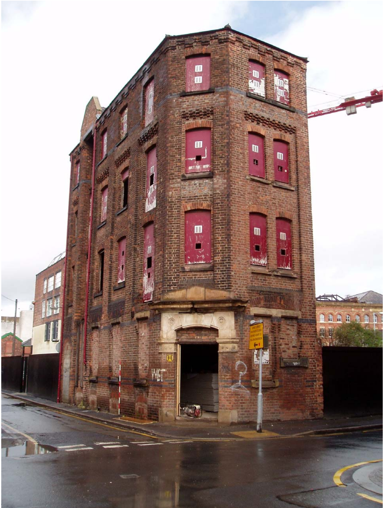
Plate 1: General view of Building 1, looking north, showing the main entrance to the building
