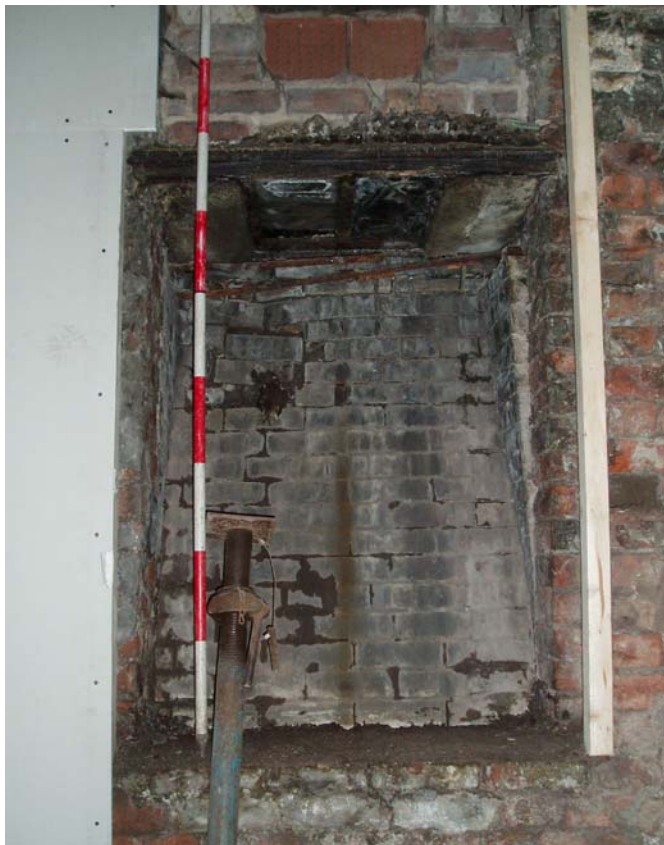
Plate 5: Cast-iron treads over the cellar-light apertures in Building 1
