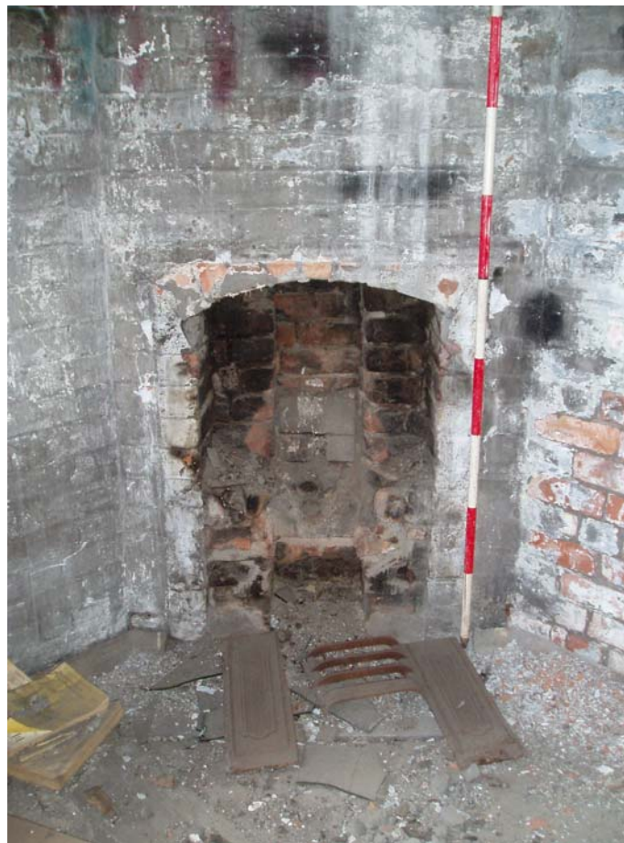
Plate 23: Fireplace in eastern bay of 2 nd floor
