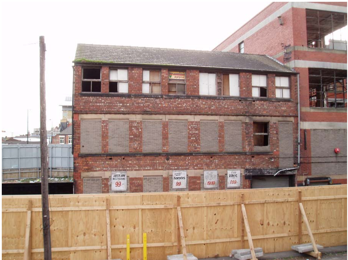
Plate 16: East-facing elevation of Building 2
