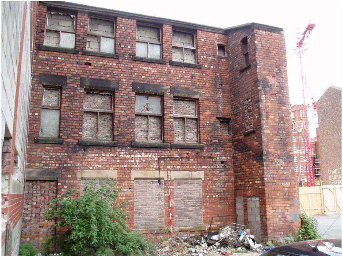
Plate 18: West-facing elevation of Building 2, showing original toilet tower
