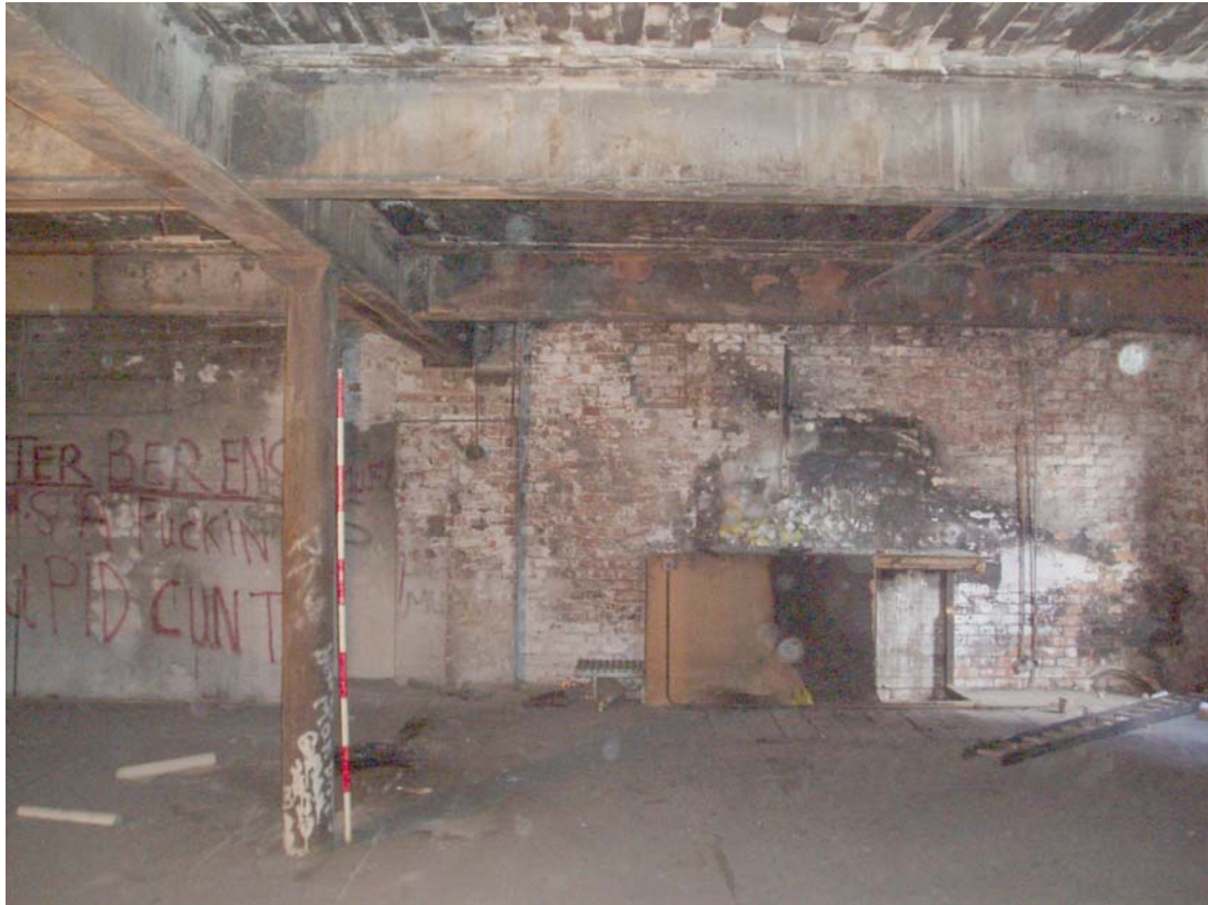
Plate 22: General view of Building 2, 1 st floor
