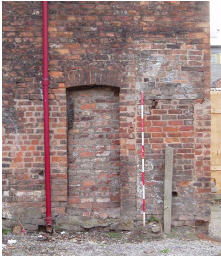
Plate 9: Two blocked doors at ground floor level of the northern bay
