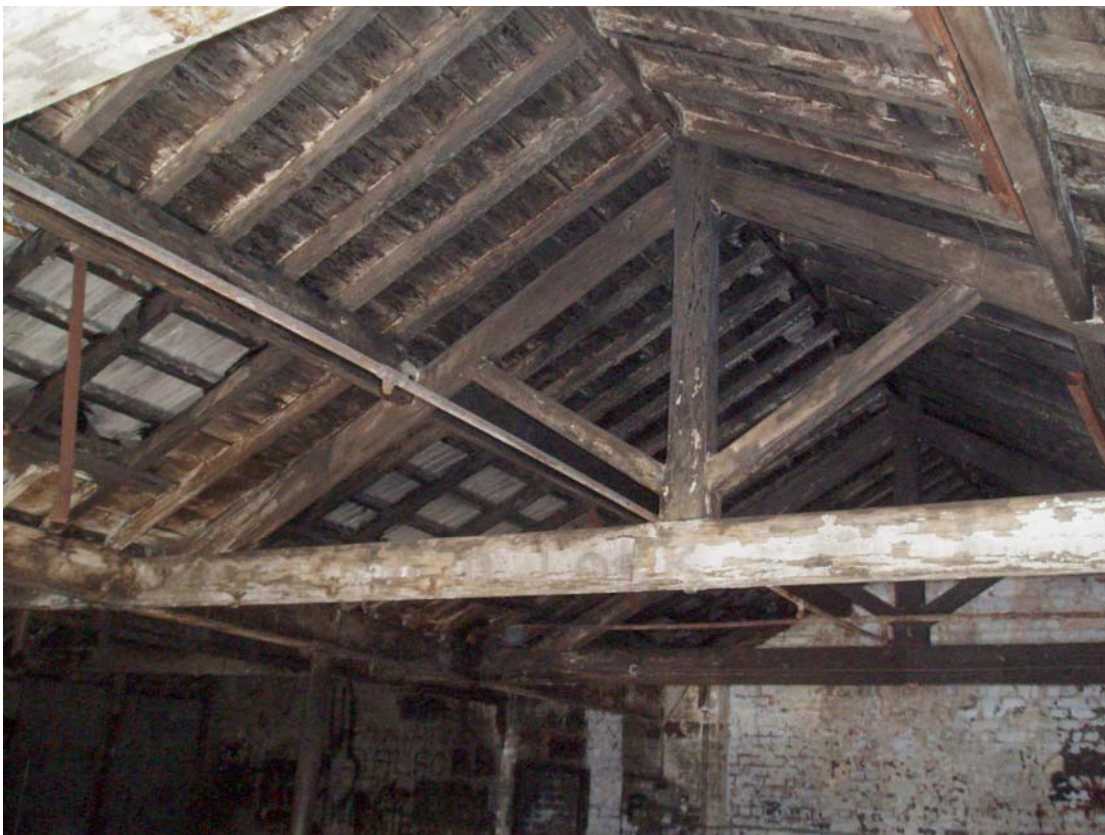
Plate 21: Roof truss detail of Building 2
