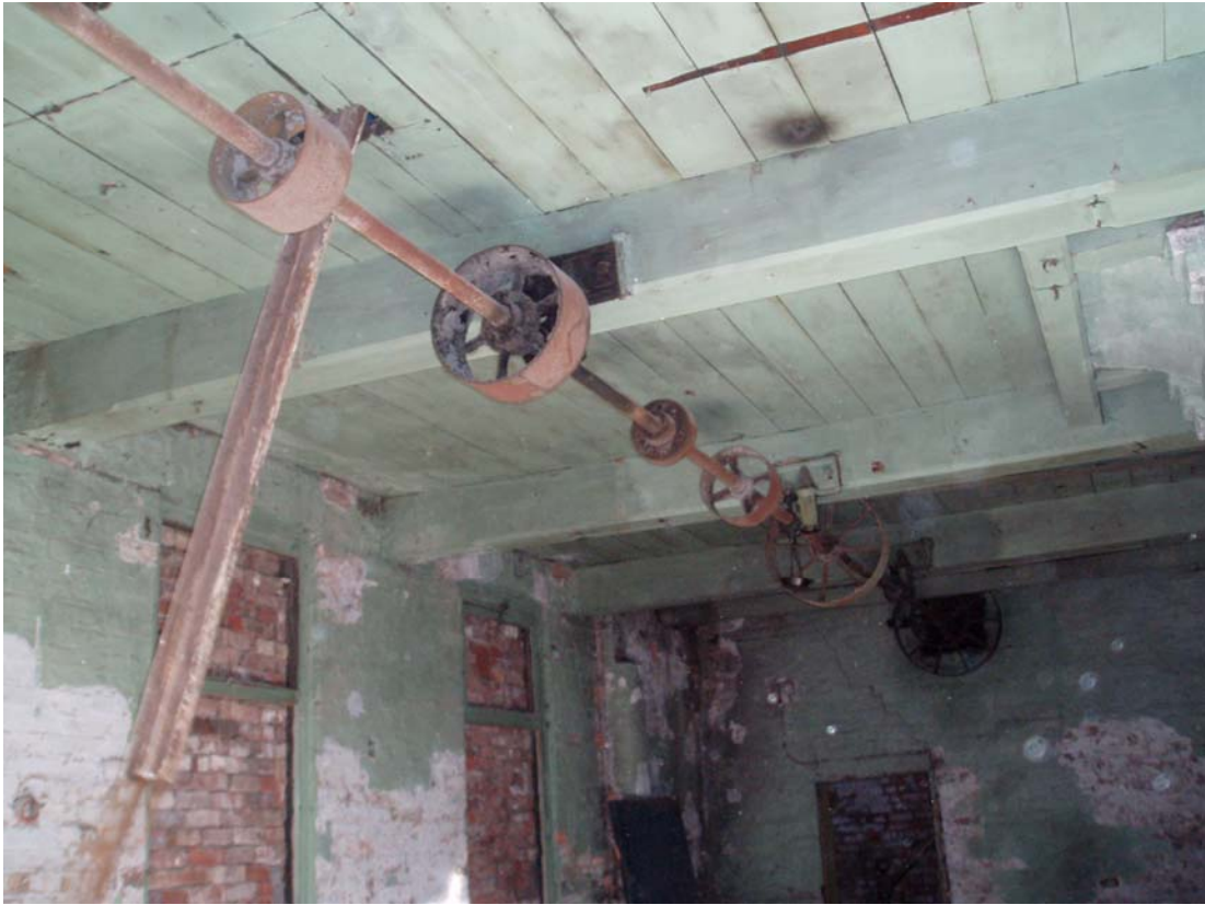
Plate 12: Line-shaft on ground floor of Building 1
