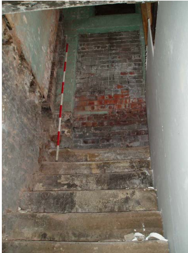
Plate 6: Sandstone steps into the cellar of Building 1, showing blocked doorway that formerly provided access to Jersey Street
