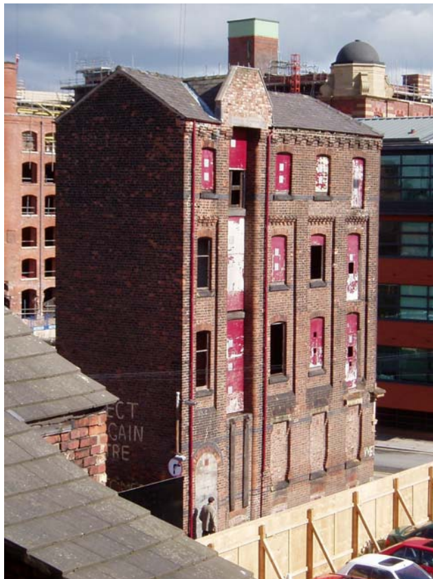
Plate 7: Looking north-east across Building 1, showing timber 'rubbing strakes' and projecting dormer in the roof
