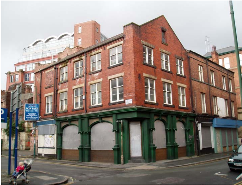
Plate 38: Late 19 th century warehouse on Turner Street
