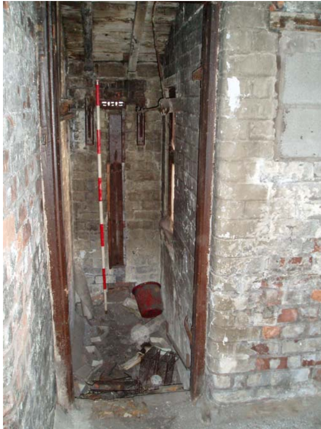
Plate 19: Internal detail of toilet tower on 2 nd floor of Building 2
