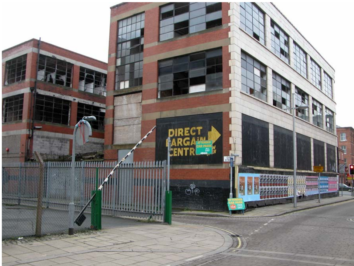
Plate 27: East-facing elevation of Building 3, fronting Gun Street
