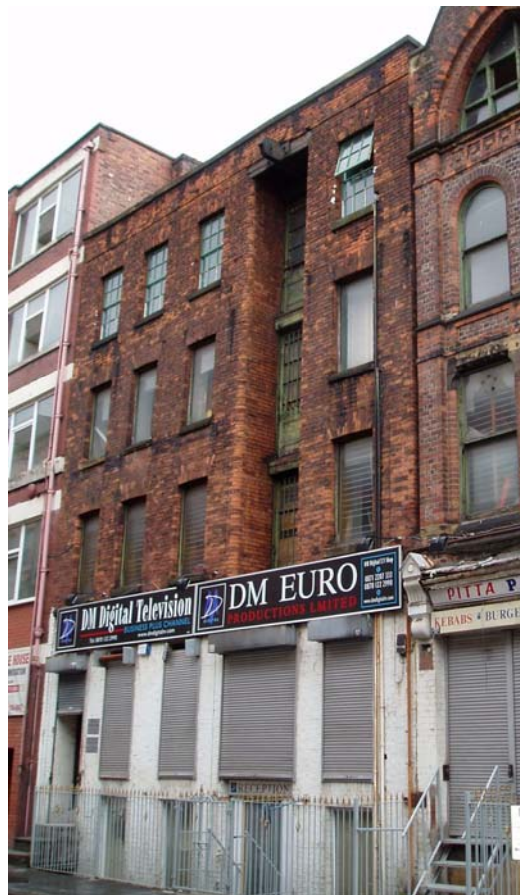
Plate 33: Mid-19 th century warehouse on Turner Street
