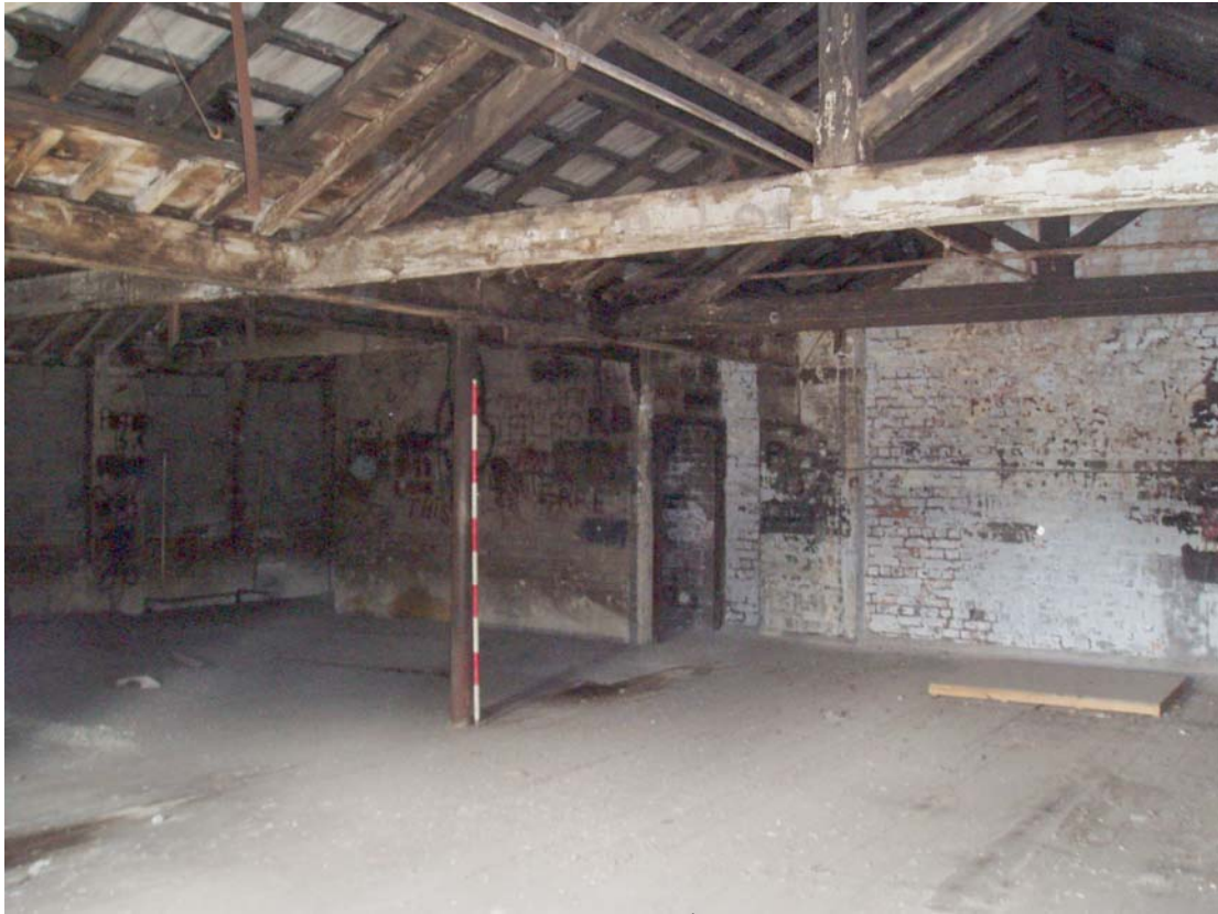
Plate 20: General view of 2 nd floor, Building 2
