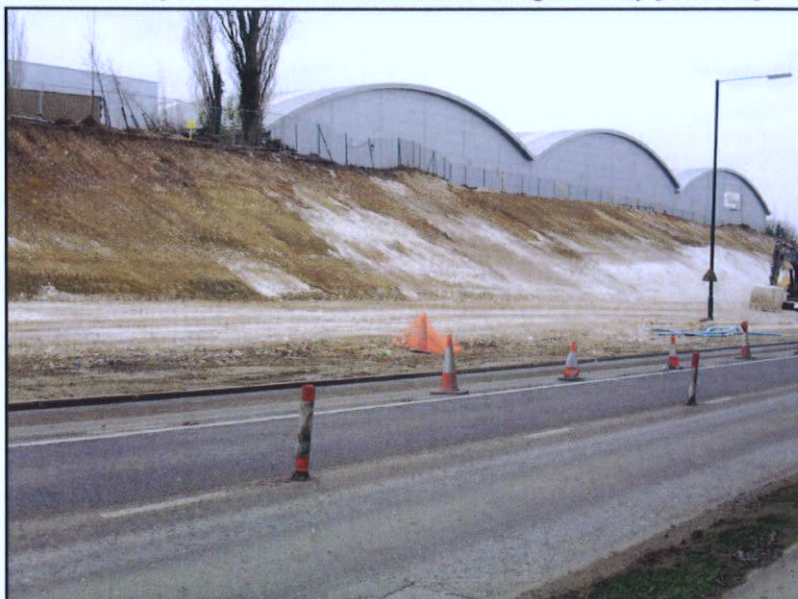
Plate 3. View westwards, covering sections 11 (nearest camera) to 15 showing valley bulge of chalk and coombe rock (see text)
