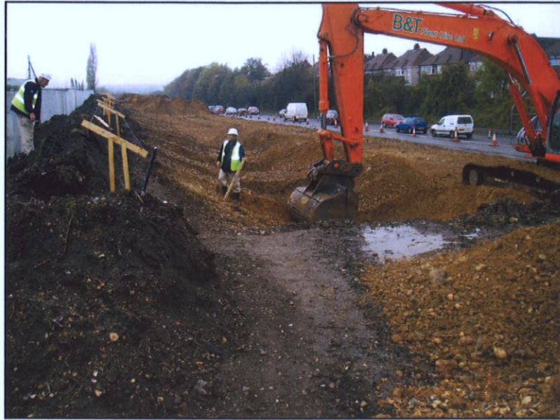
Plate 1: Groundworks in progress
