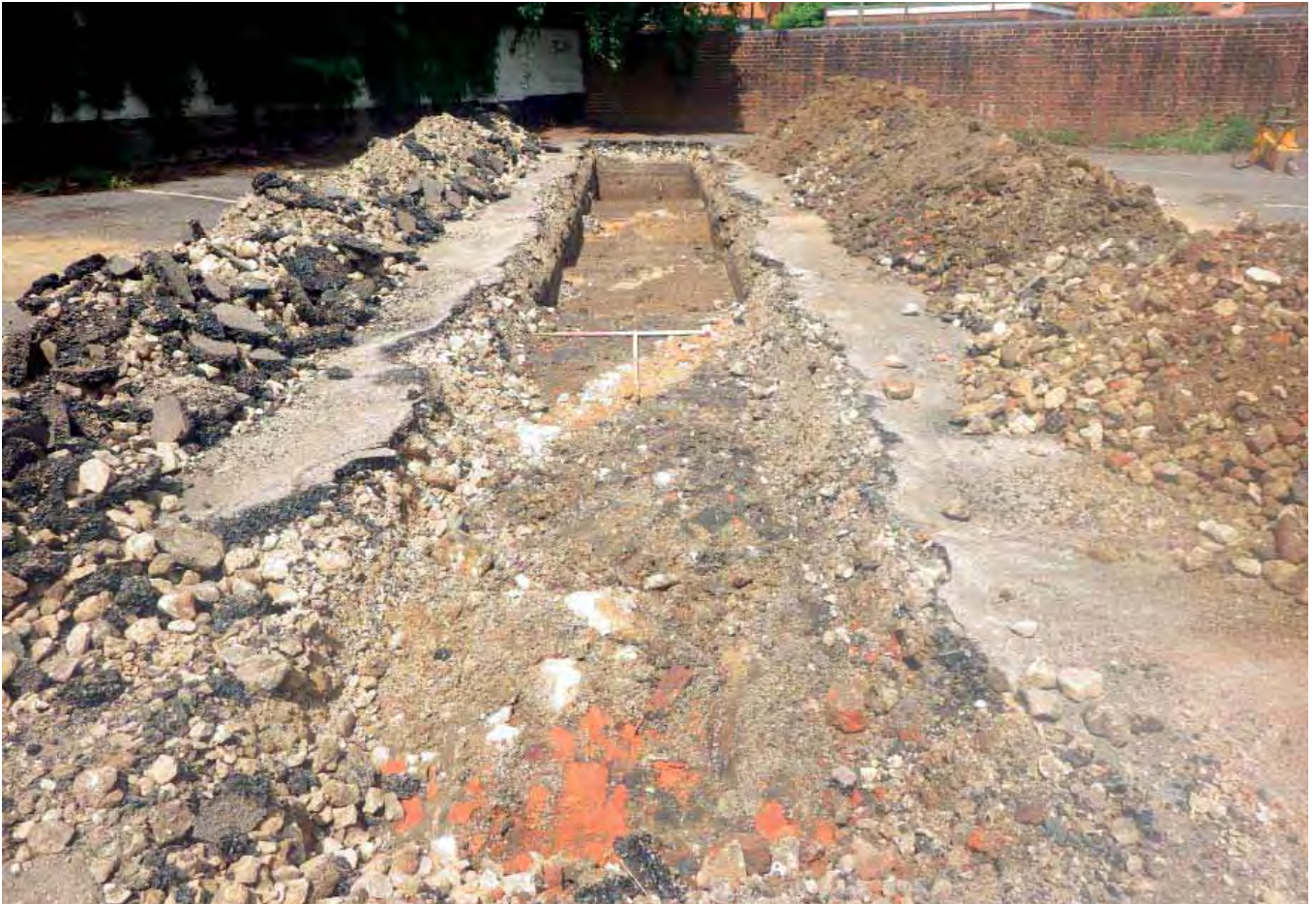
Plate 1 - Trench 1, view to NW
