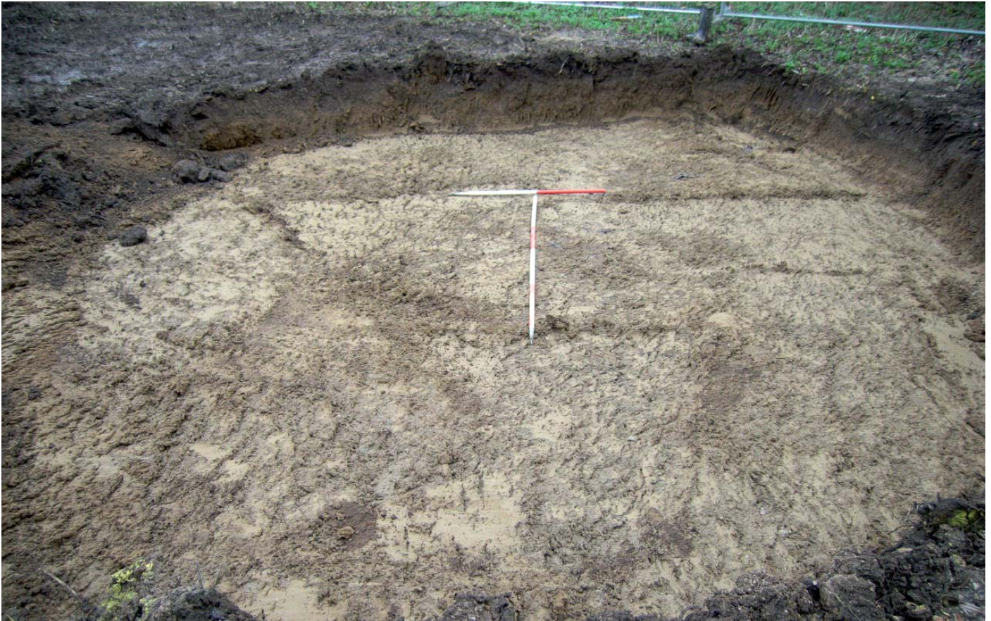
Plate 5: Attenuation pond, facing east.
