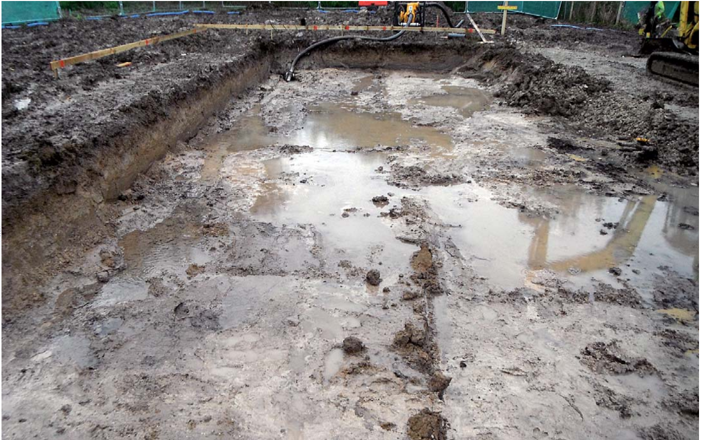
Plate 3: Substation area, facing south.
