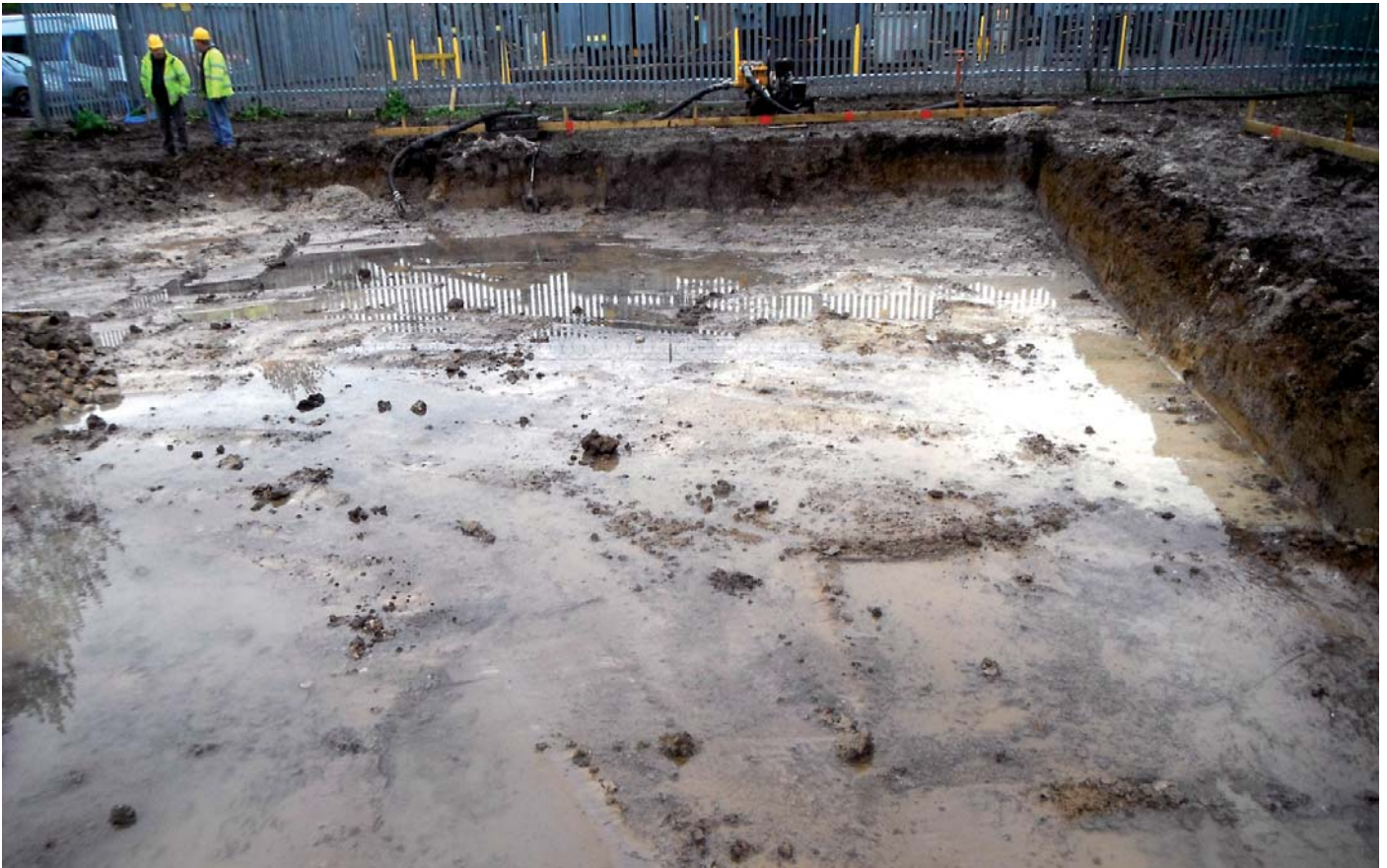
Plate 2: Substation area, facing north
