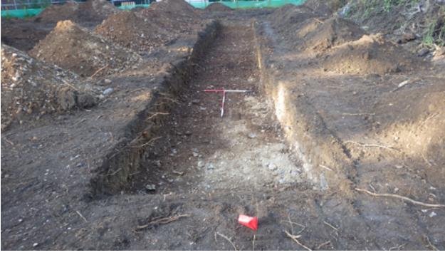
Plate 1: General shot of Trench 1, looking SW
