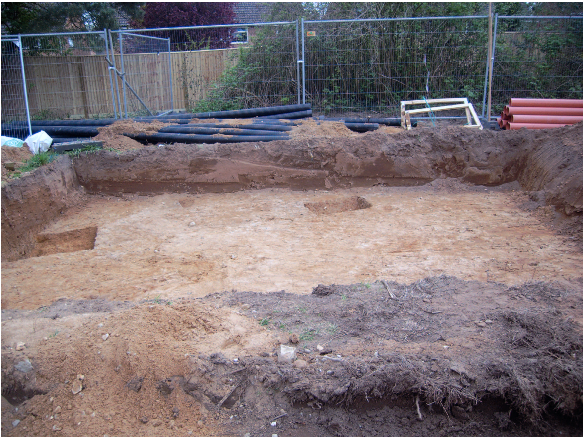
Plate 4: Soakaway pit RS3 from the north-west
