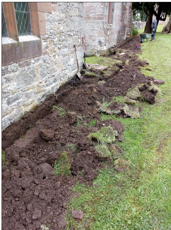
Plate 1: Oil delivery pipe trench looking south-west
