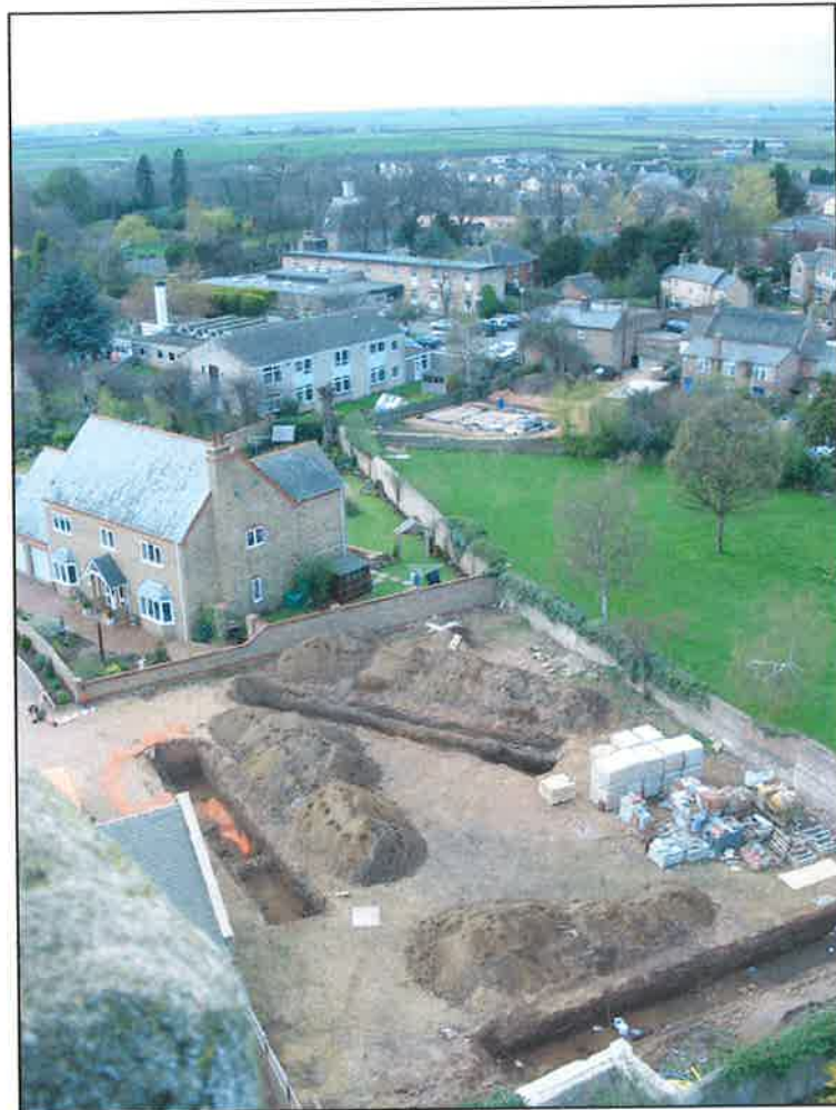
Plate 2 Location of trenches looking southwest
