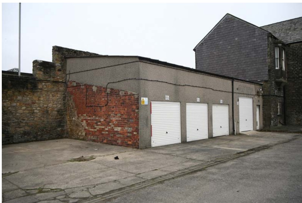
Plate 13: Example of a structure at the rear of the south perimeter wall (Site 04)
