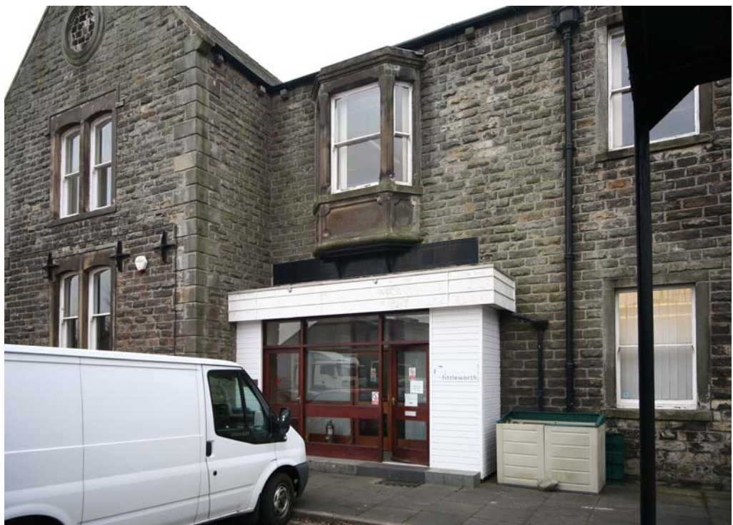
Plate 10: Oriel window supported by iron bracket set above the main entrance on the rear elevation
