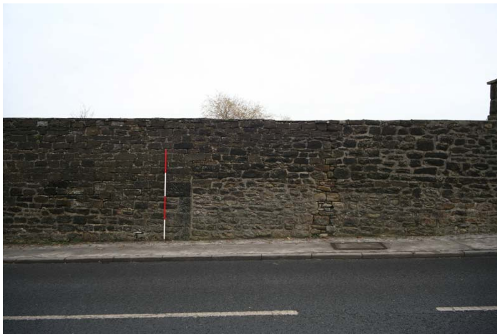
Plate 12: Stone perimeter wall (Site 04) to the south of the main office building showing phasing
