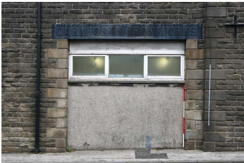
Plate 11: Entrance on the principal elevation showing the distinctive iron lintel bearing the name 'CARNFORTH IRON WORKS'
