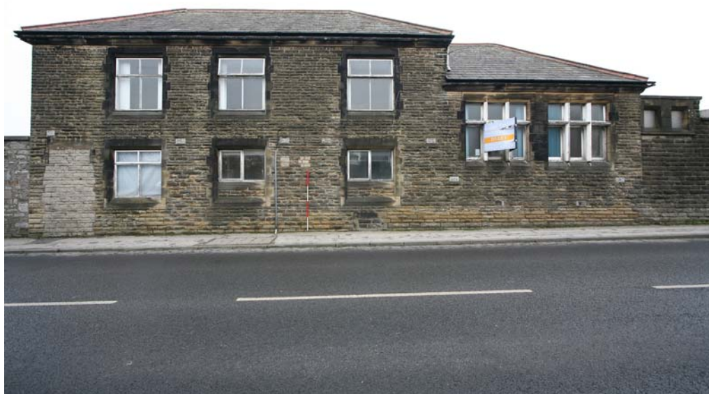
Plate 14: Front elevation of Iron Works Cottage showing the perimeter wall at the extreme right side and blocked door
