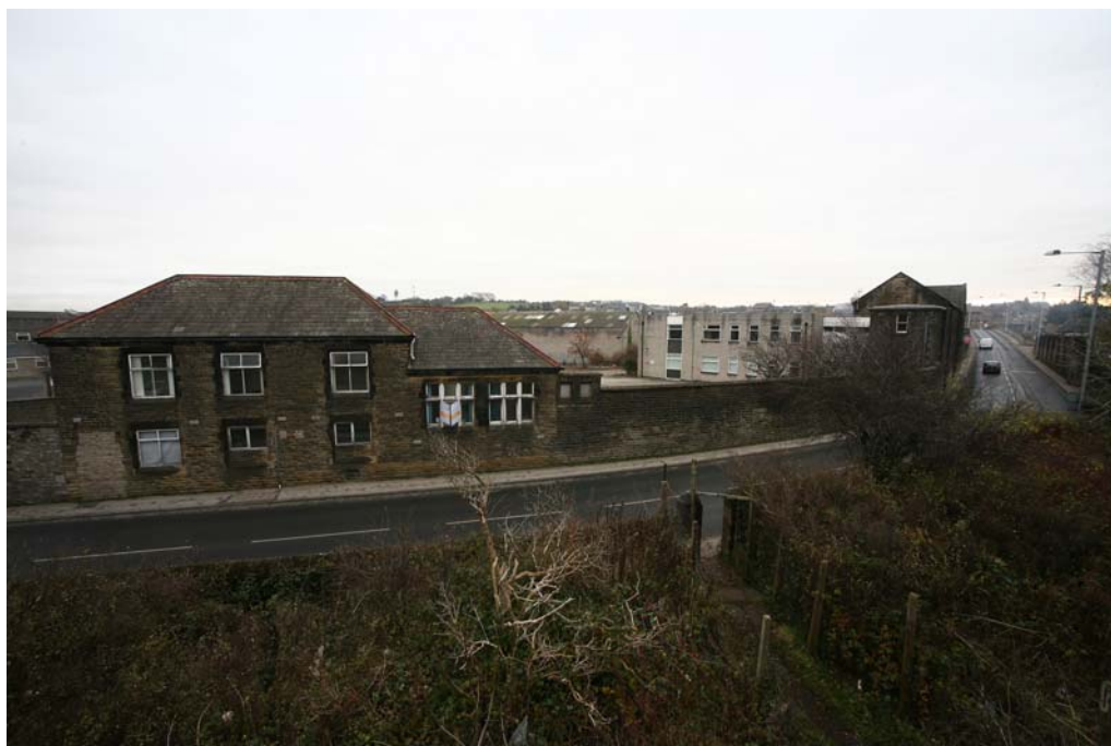
Plate 6: The north end of the site showing Iron Works Cottage (Site 02)
