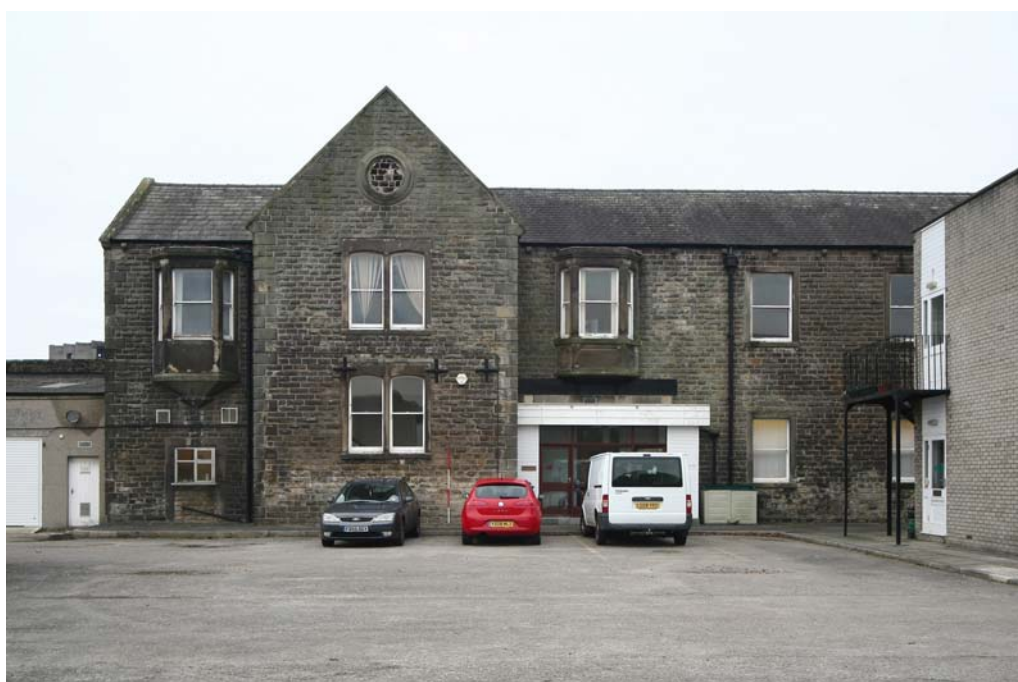
Plate 8: The rear elevation of the office range of the former iron works
