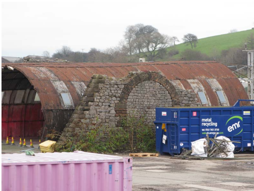
Plate 15: Example of stone elevated railway supporting wall (Site 05) at the south end of the site, close to the Lancaster to Carlisle Railway
