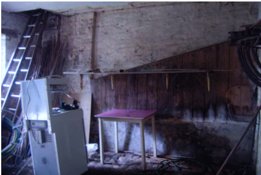
Plate 91: South wall of stable
