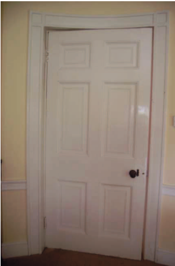
Plate 19: Dining room doors, facing north
