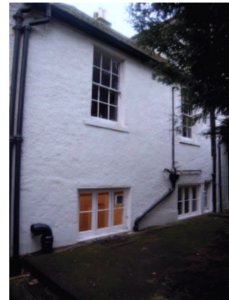
Plate 8: West elevation, Victorian extension
