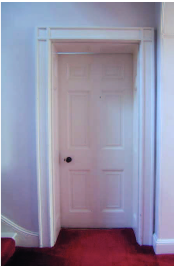
Plate 51: Bathroom door, facing north
