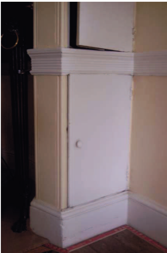
Plate 23: Dining room skirting board and dado rail
