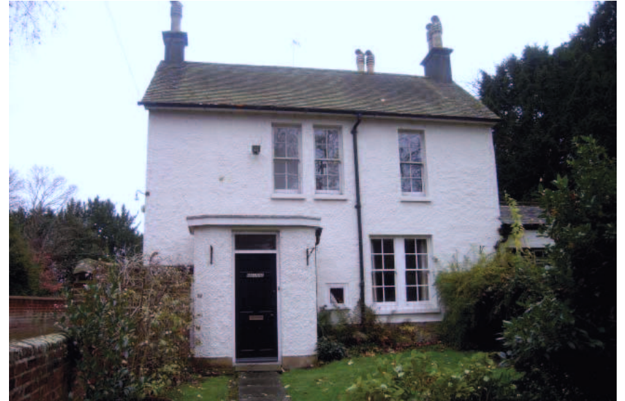
Plate 6: North elevation, Victorian extension
