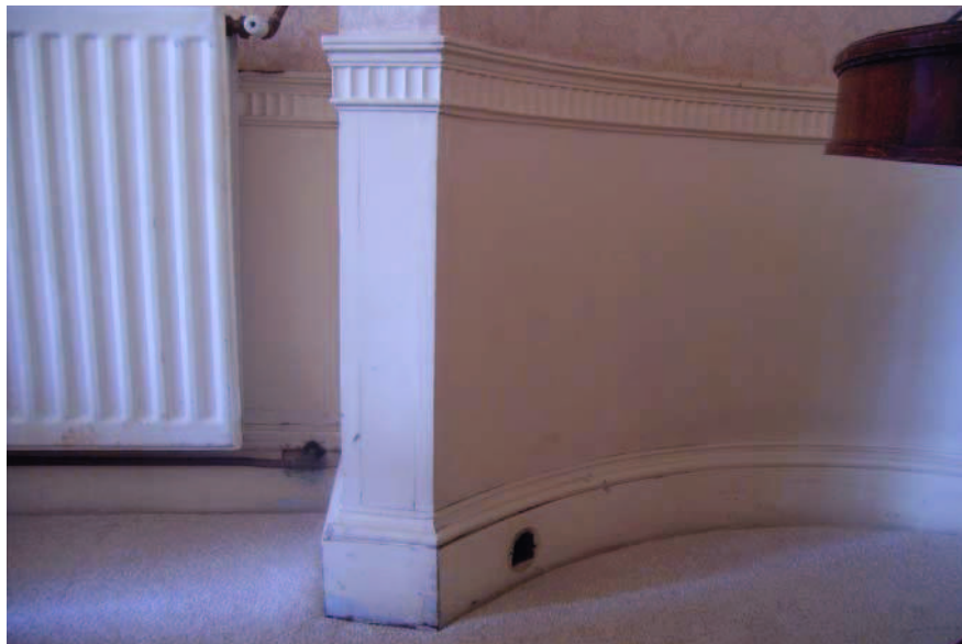
Plate 59: Drawing room skirting board and dado rail
