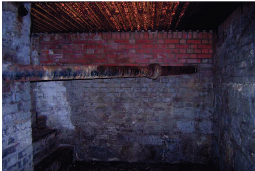
Plate 95: South wall of underground cellar
