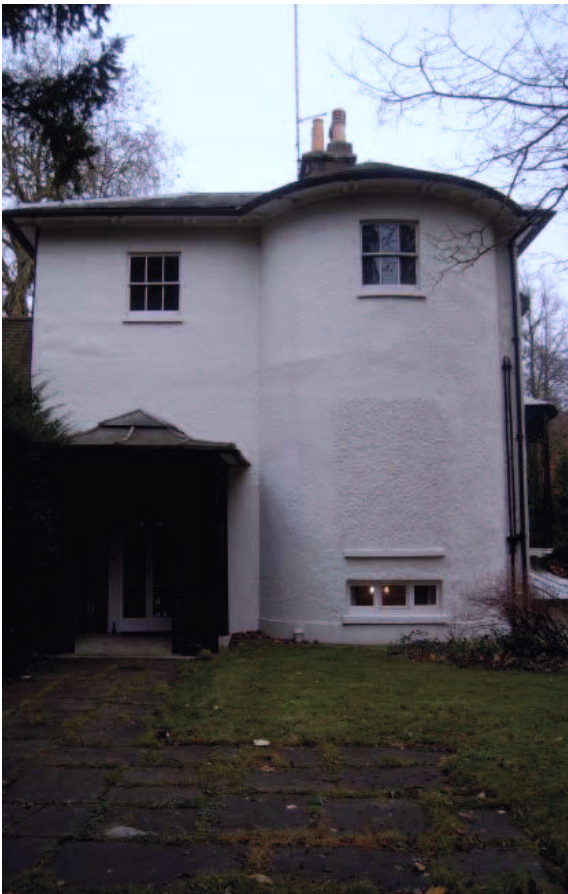
Plate 3: West elevation of Original House
