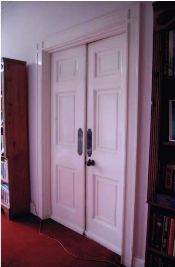
Plate 49: Drawing room doors, facing south-west
