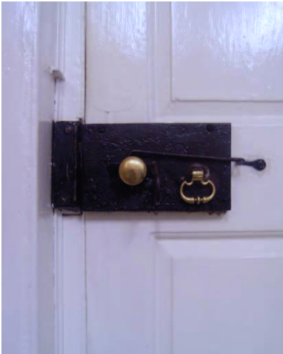
Plate 33: Kitchen door lockcase, facing north
